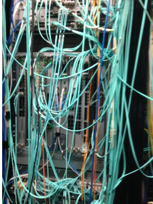
FIGURE 4 Cable clutter
