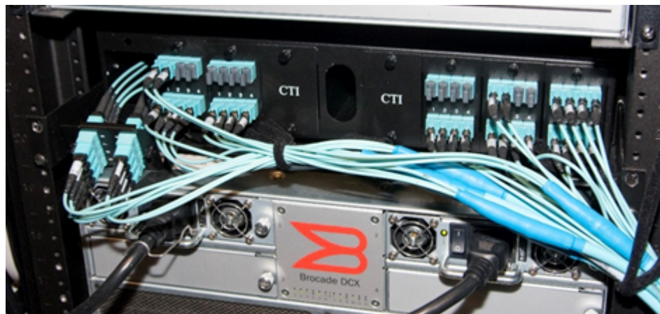
FIGURE 13 Device to Patch Panel Trunk Cabling
