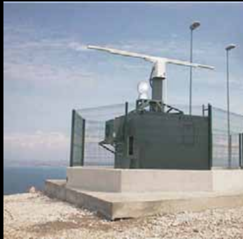
SURVEILLANCE RADAR SYSTEMS
