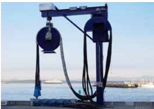
Photos feature cable on Cochran Marine's Cable Positioning Device, used to serve shore power
