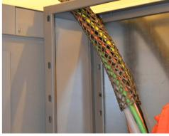
hearing about how even though they are plexed configurations, they pulled more easily through conduits than single conductor."
