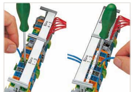
Sliding marking strips laterally.
