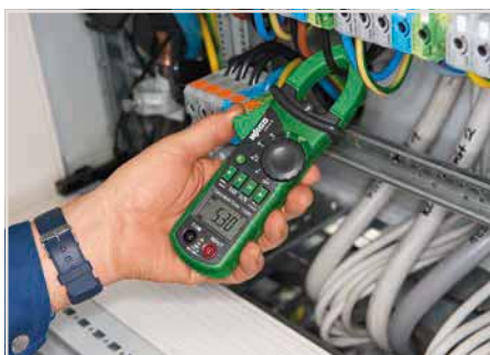
Voltage testing in switchgear cabinet
