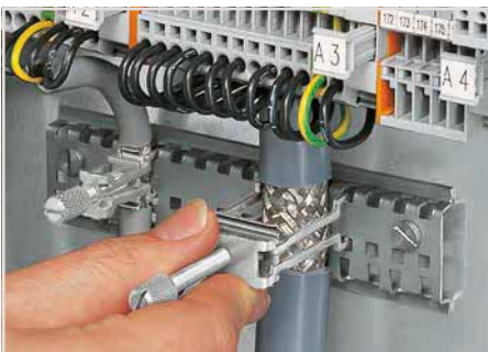
Fitting an additional clamping saddle.
