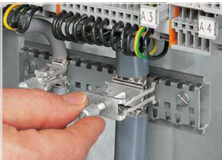
Tightening/removing a shield clamping saddle.
