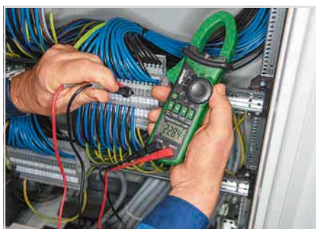
Current measurement in a switchgear cabinet
