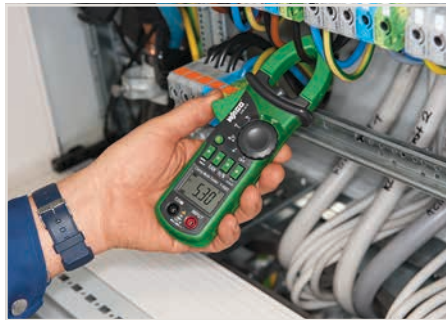
Voltage testing in switchgear cabinet
