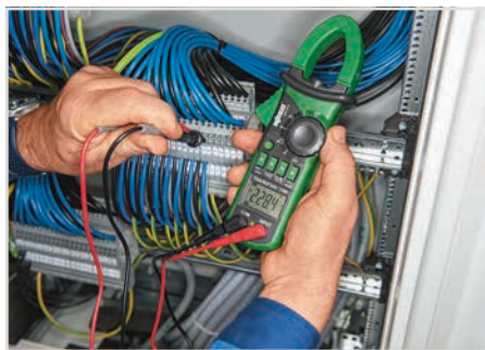
Current measurement in the switchgear cabinet
