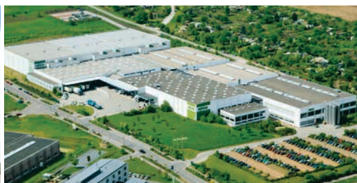
WAGO Sondershausen, Germany
