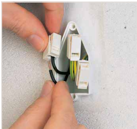
Wiring lighting connectors in a junction box.
