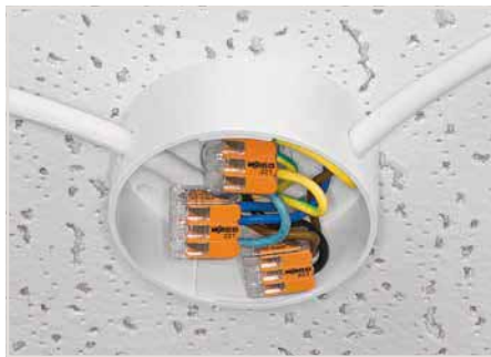
Lighting distribution in ceiling canopy
