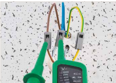
Testing via separate test ports.
