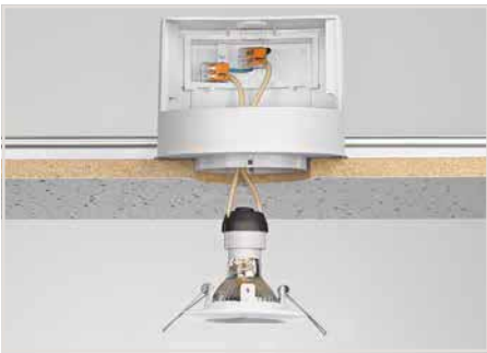
Custom low-voltage lighting system
