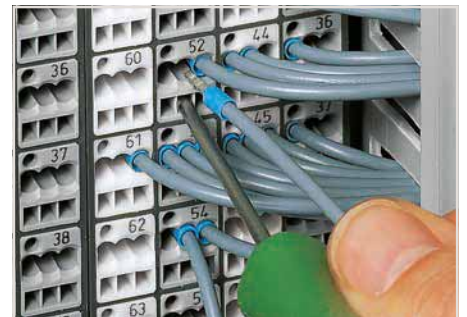
Terminating ferruled conductors via operating tool.
