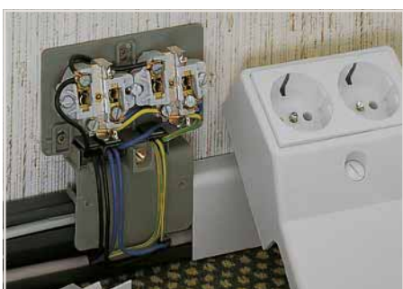
PUSH WIRE® junction box connectors used in a cable duct with double power outlet
