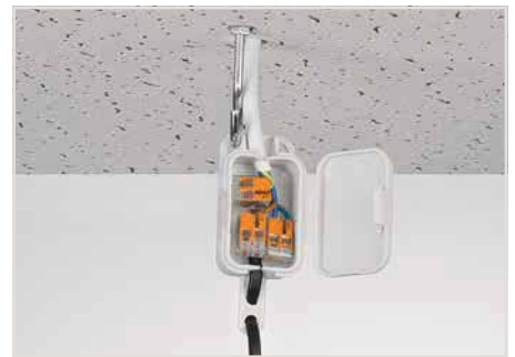
Pendant light connection in suspended ceilings
