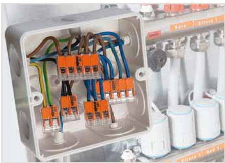
Wiring fine-stranded conductors in a junction box.
