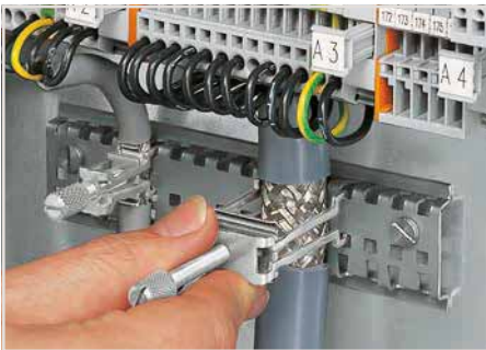
Fitting an additional clamping saddle.
