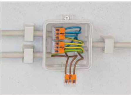
Wiring fine-stranded conductors in a junction box.
