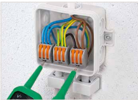
Testing via Profi-LED+ voltage tester (206-806).
