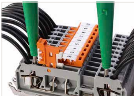
Testing with voltage tester.
