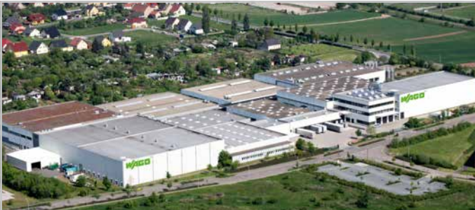
WAGO Sondershausen, Germany
