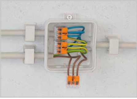
Wiring fine-stranded conductors in a junction box.
