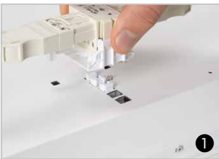
Position the T-connector within the two square recesses.
