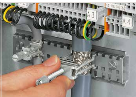
Fitting an additional clamping saddle.
