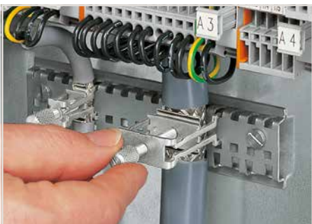
Tightening/removing a shield clamping saddle.
