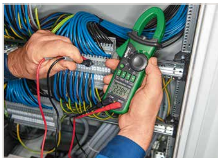
Current measurement in a switchgear cabinet
