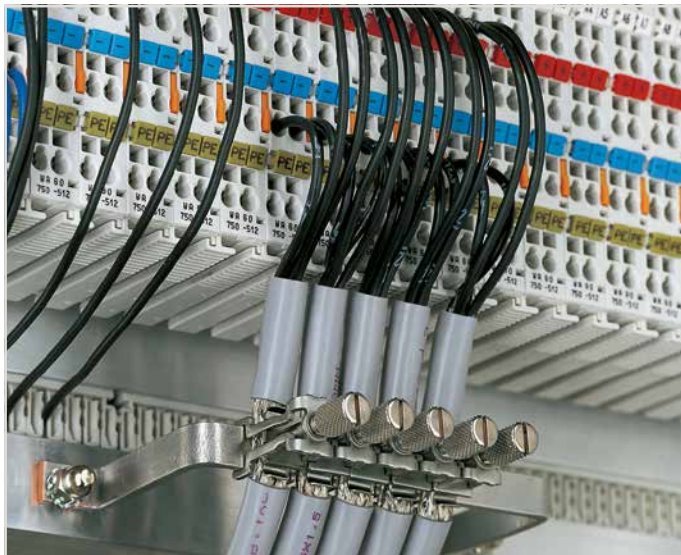
U-shaped (10 x 3) mm copper busbar
