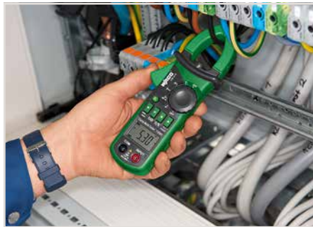
Voltage testing in switchgear cabinet
