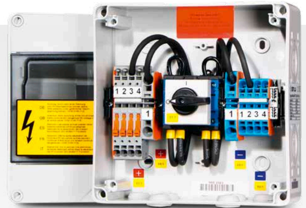
Generator Junction Box
