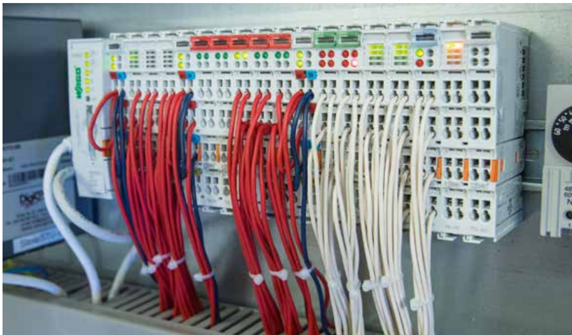
The WAGO PFC200 Control-ler links the heat transfer station to the control center of the district heating network.
