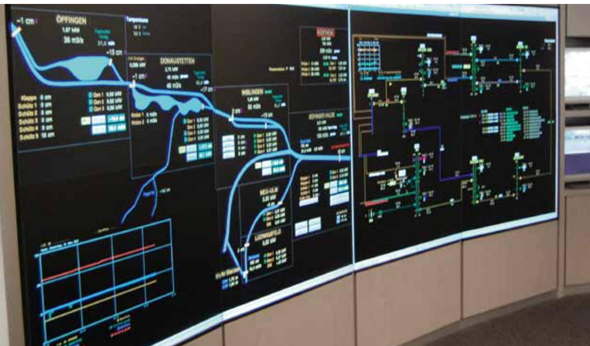
In the control center: due to the increased use of renewables, electrical flows are more complex and controlling the network has become more expensive. Therefore, the utility in Ulm/Neu Ulm invested in telecontrol technology.
