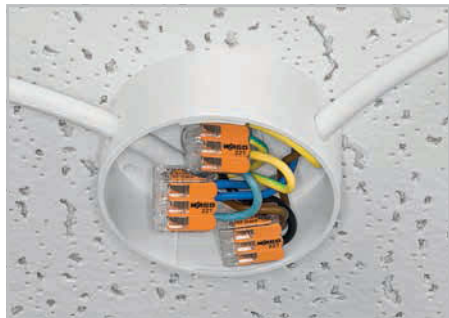
Lighting distribution in ceiling canopy
