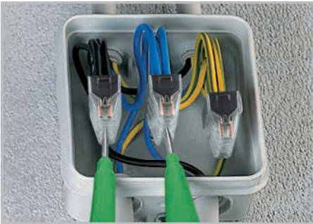
Voltage testing via separate test ports.
