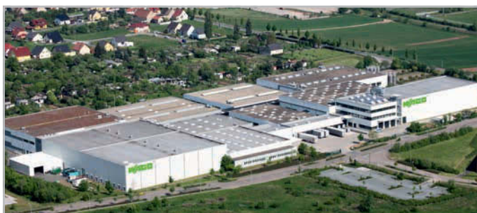
WAGO Sondershausen, Germany
