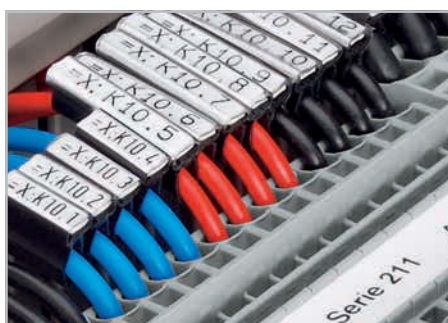
Marking conductors via marking sleeves.
