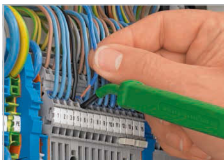
Open the clamping unit using an operating tool.
