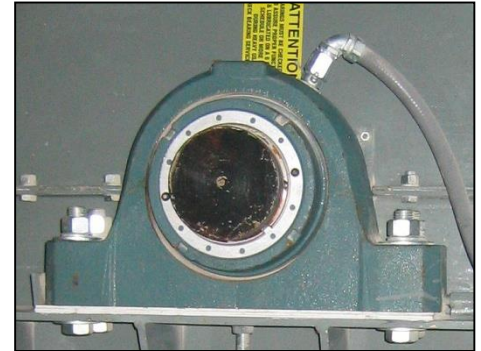
Sensor Installed on Conveyor Bearing
