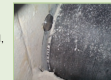
Touchswitch on Enclosed Conveyor
