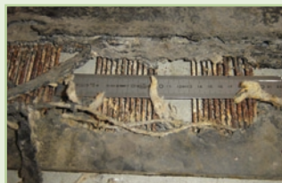
Traditional Belt - Cables Exposed
