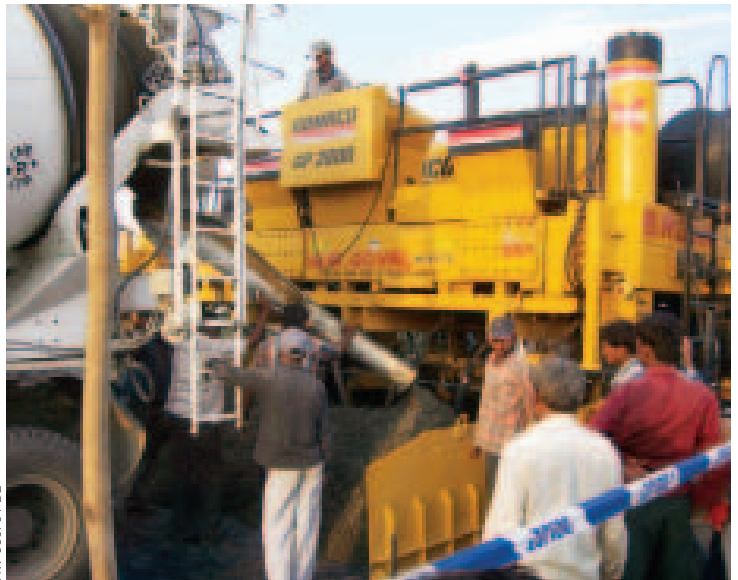
B.R. Goyal slipforms a new highway near Madhya Pradesh, India, with their two-track GP-2600 paver.
