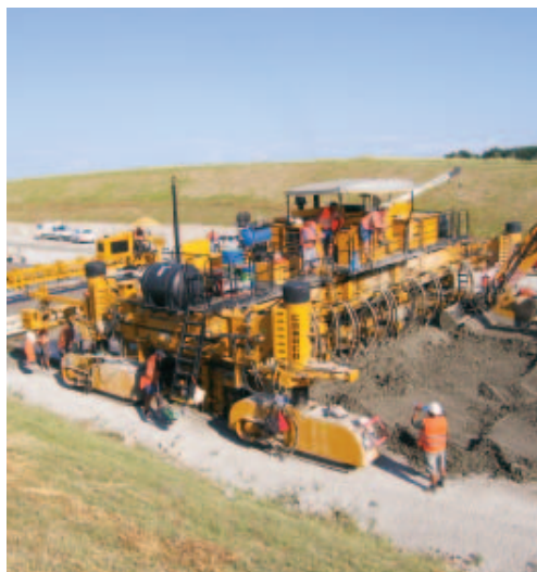
Skanska and their GP-4000 with IDBI is currently at work slipforming 42 km (26 mi) of Highway D11 connecting Hradec Králové to Podúbrady in the Czech Republic.
