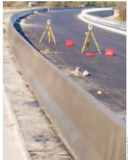
Two Total Stations track the GT-3600 as it slipforms barrier wall through a radius.
