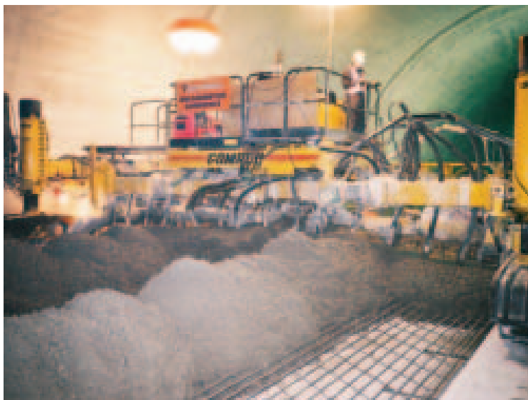
A Commander III slipforms the new roadway through Japan's Suzuka Tunnel project.
