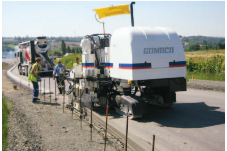
Eurovia's operator uses the GT-3400's remote control and operates the machine from ground level as they slipform curb and gutter on a project near Villedieu les Poeles, France.
