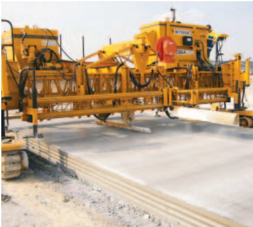
The T/C-600 texture/cure machine, equipped with a transverse curing mechanism, tines and cures in a single pass.
