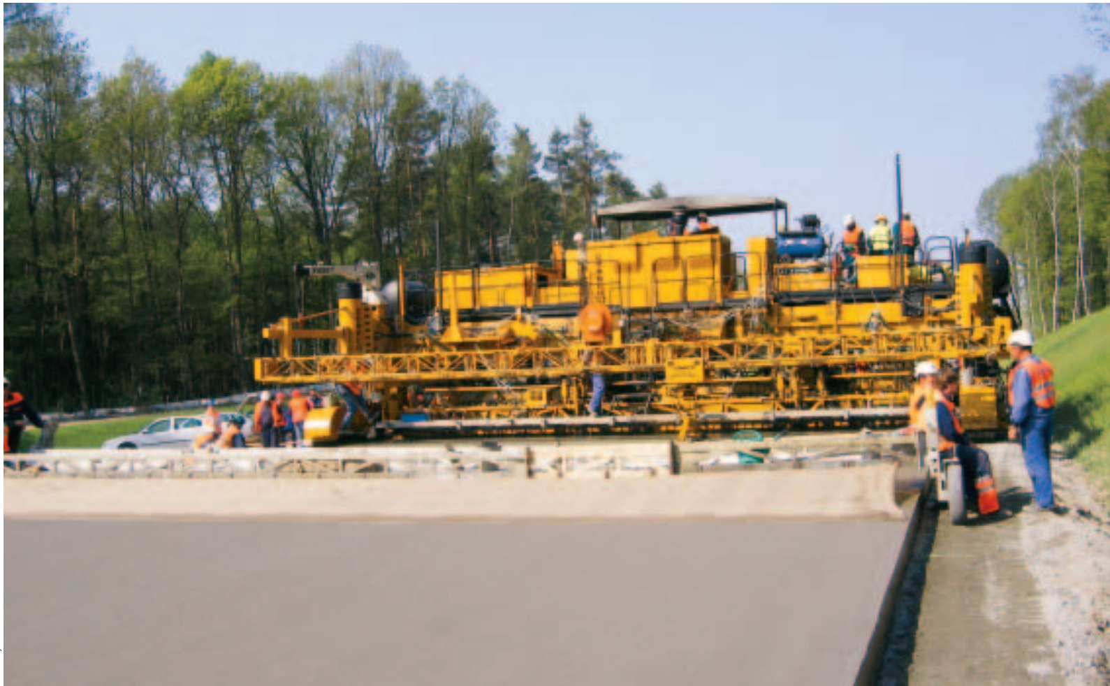
Skanska's GP-4000 with two-lift paving system, IDBI and stringless control system slipforms a new highway in the Czech Republic.
