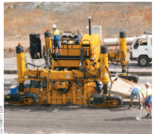
South East Concreting Pty. Ltd. slipforms half-width roadway with their four-track Commander III on a new roadway in Sydney, Australia.
