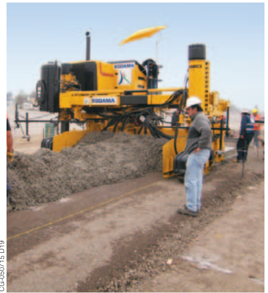
Kodama slipforms 3.5 meter (11.5 ft) wide pavement with their Commander III three-track on a project in Santiago, Chile.
