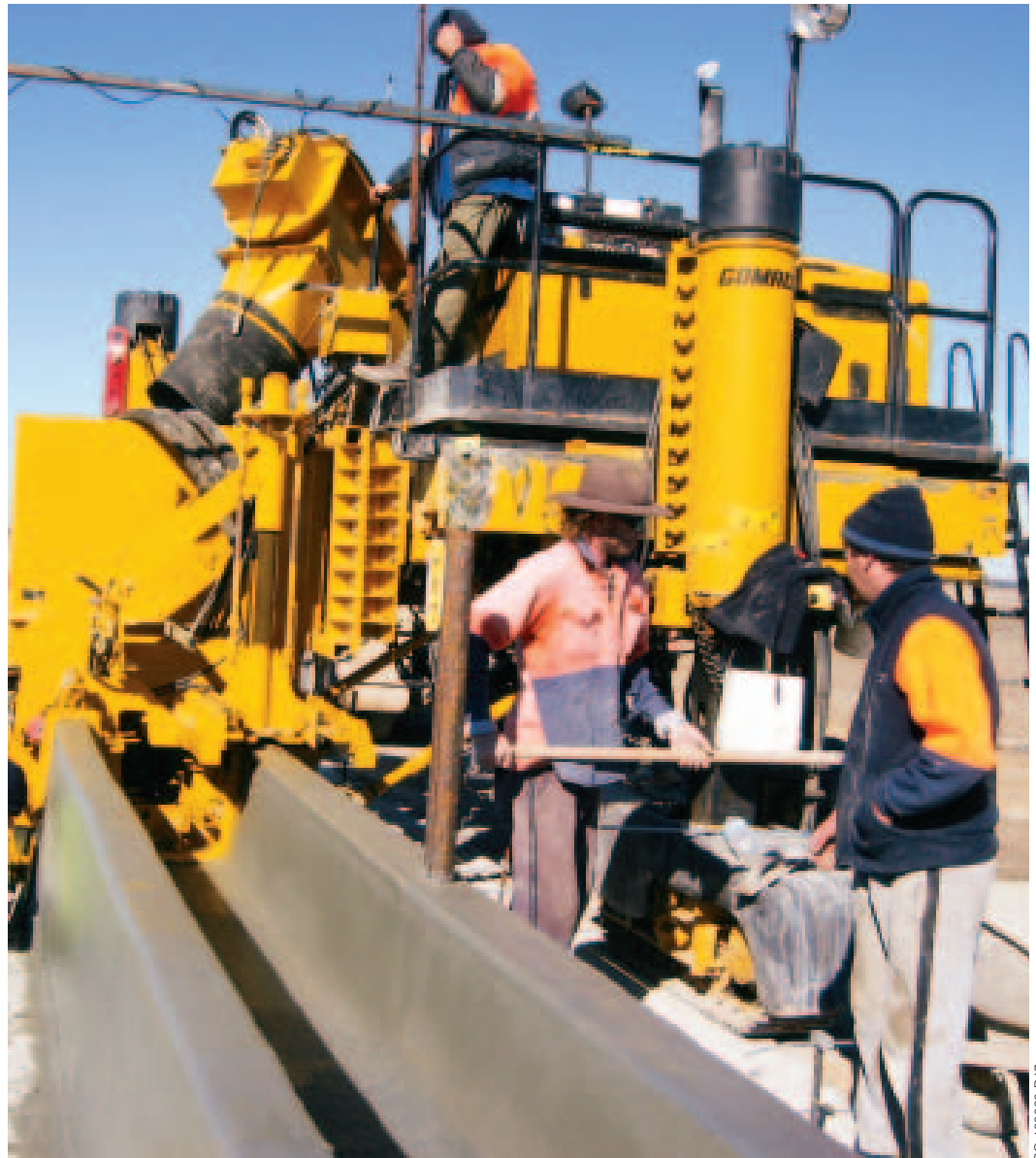
The feed bunk mold has a hydraulic pole inserter mechanism that allows finishers to insert 1.3 meter (4.3 ft) long poles into the sidewall of the new feed bunk on-the-go while slipforming.
