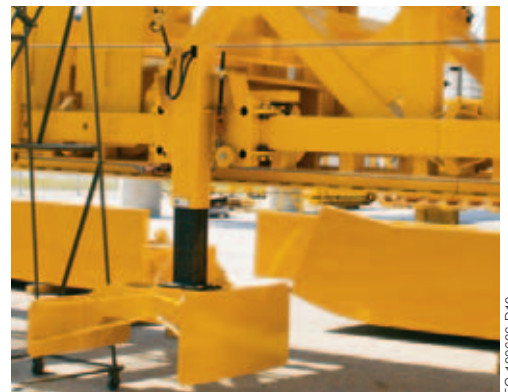
The spreader-plow moves the concrete across the bottom section of the canal floor.
