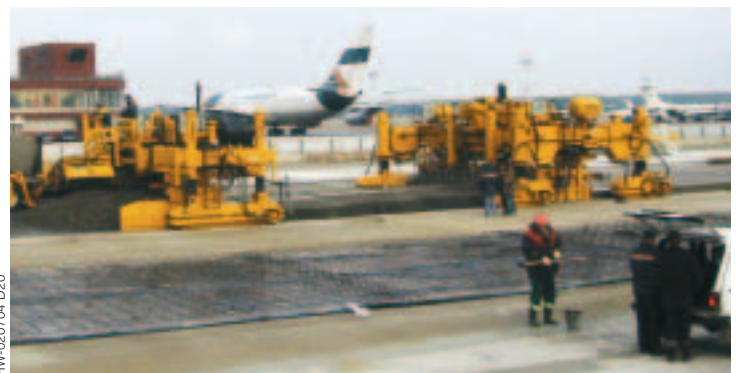
Centrodorstroy is at work with their PS-2600 placer/spreader and four-track GHP-2800 paver on a project at the Domodedovo International Airport in Moscow, Russia.
