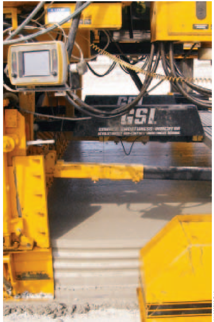
The GHP-2800 paver-mounted GSI provides Betonac with a constant indication of pavement quality.
