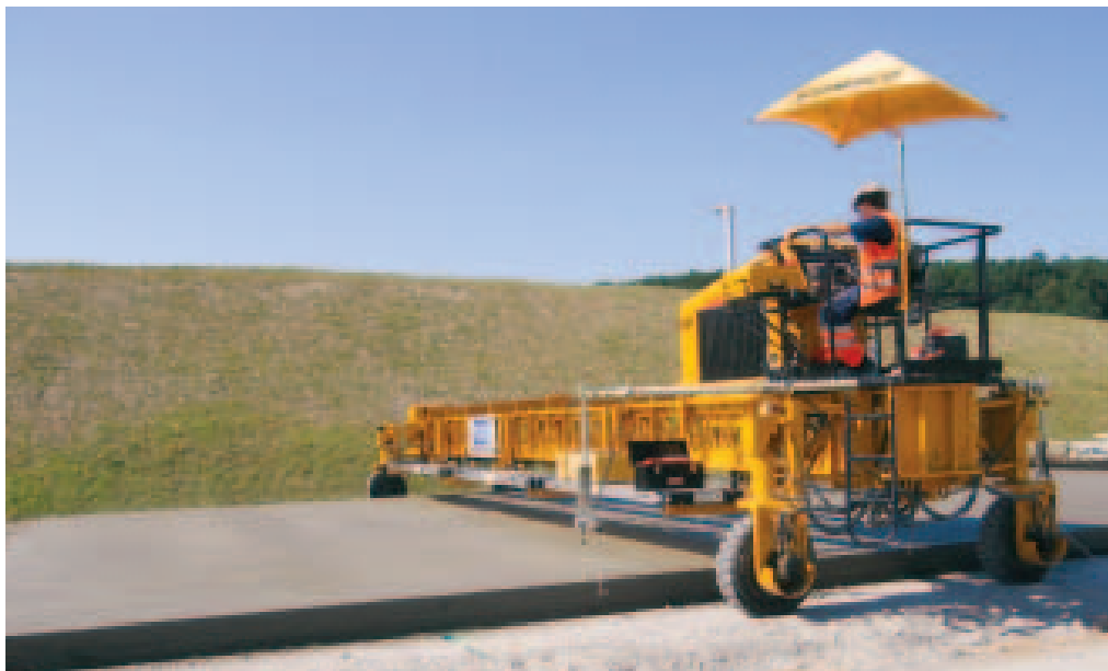
The GOMACO GSI follows the paver and measures the smoothness of the new roadway.
