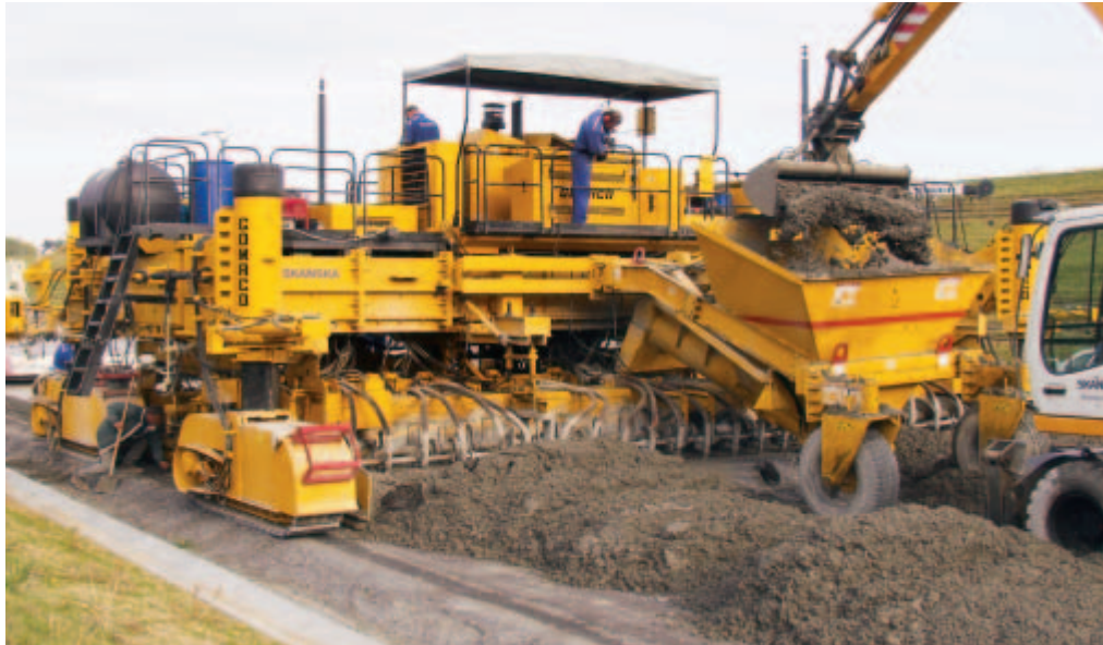
An excavator was used to place the top layer concrete mix design into the paver's hopper. The bottom layer's concrete was dumped directly on the ground, in front of the GP-4000.
