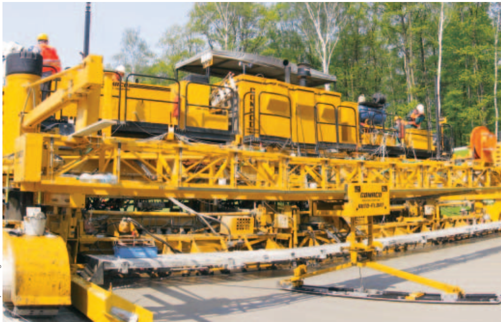
Paving production averaged 400 meters (1312 ft) per day while paving the two-lift project.
