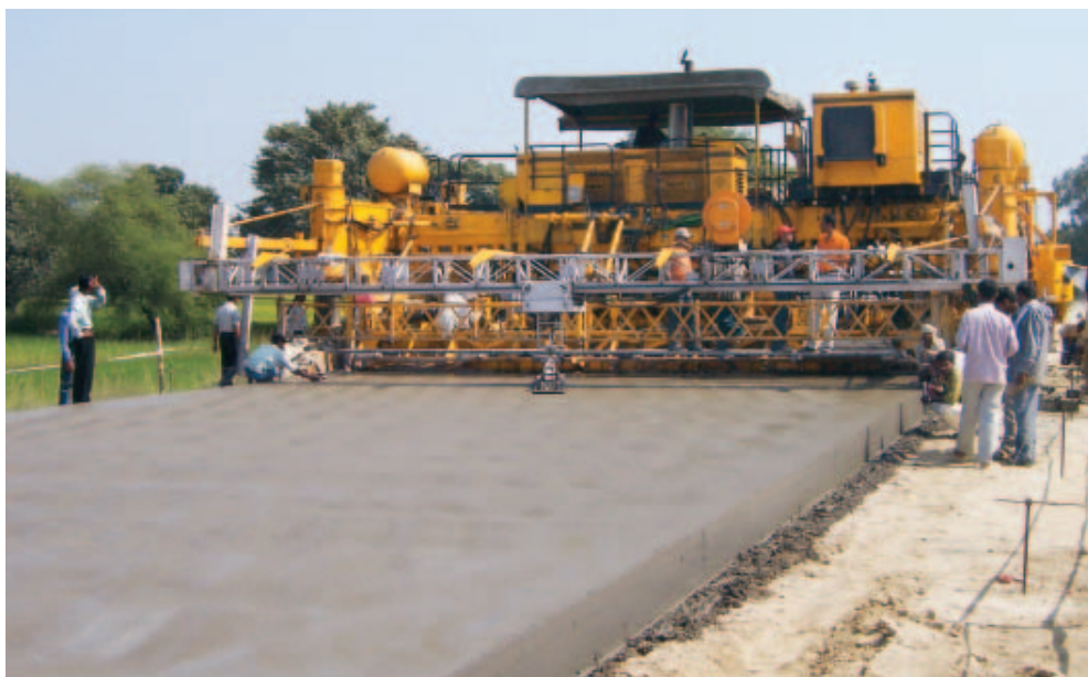
The joint venture team of CDS and Mukand are using a four-track GHP-2800 with IDBI to slipform the new National Highway 2 between the cities of Kanpur and Allahabad in Uttar Pradesh, India.
