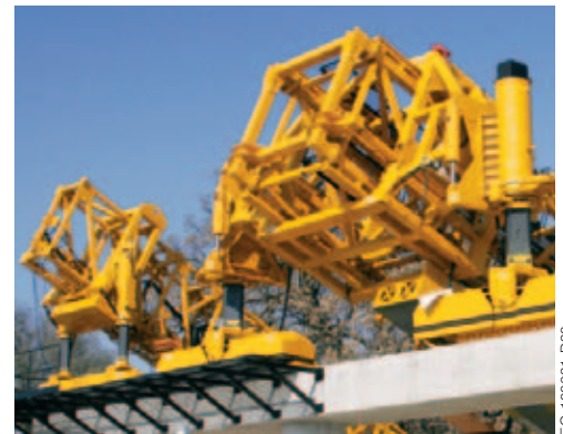
Adjustable end cars on the machines hydraulically slide for width changes.
