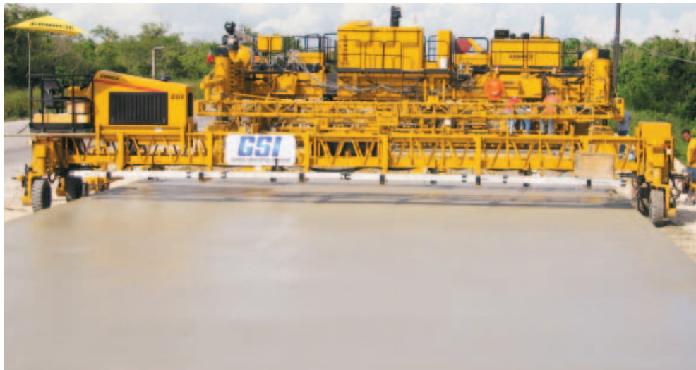
CEMEX slipforms a new roadway south of Cancun, Mexico, with their new GP-4000 with IDBI. A GSI® follows behind the paver measuring the smoothness of the new roadway.
