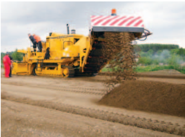
Russian contractor Nur trims base with their 9500 trimmer on a new roadway project near Kazan, Russia.
