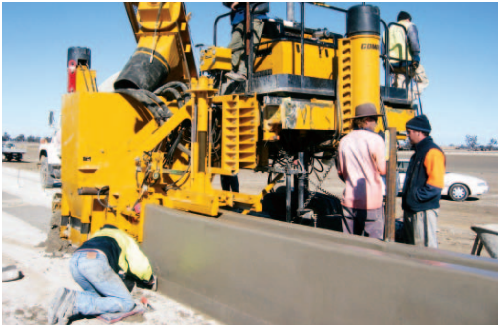
The Commander III slipforms feed bunk at the Yambinya Feedlot in New South Wales.
