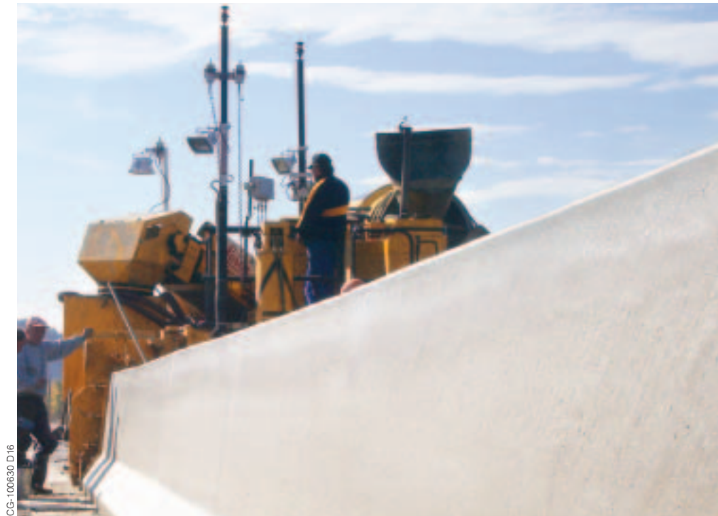
The barrier wall has a 685 mm (27 in) wide base and is 1100 mm (43.3 in) tall.
