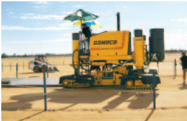
The flat slab has a roller dimple finish to help the cattle create traction and grip on the concrete.
