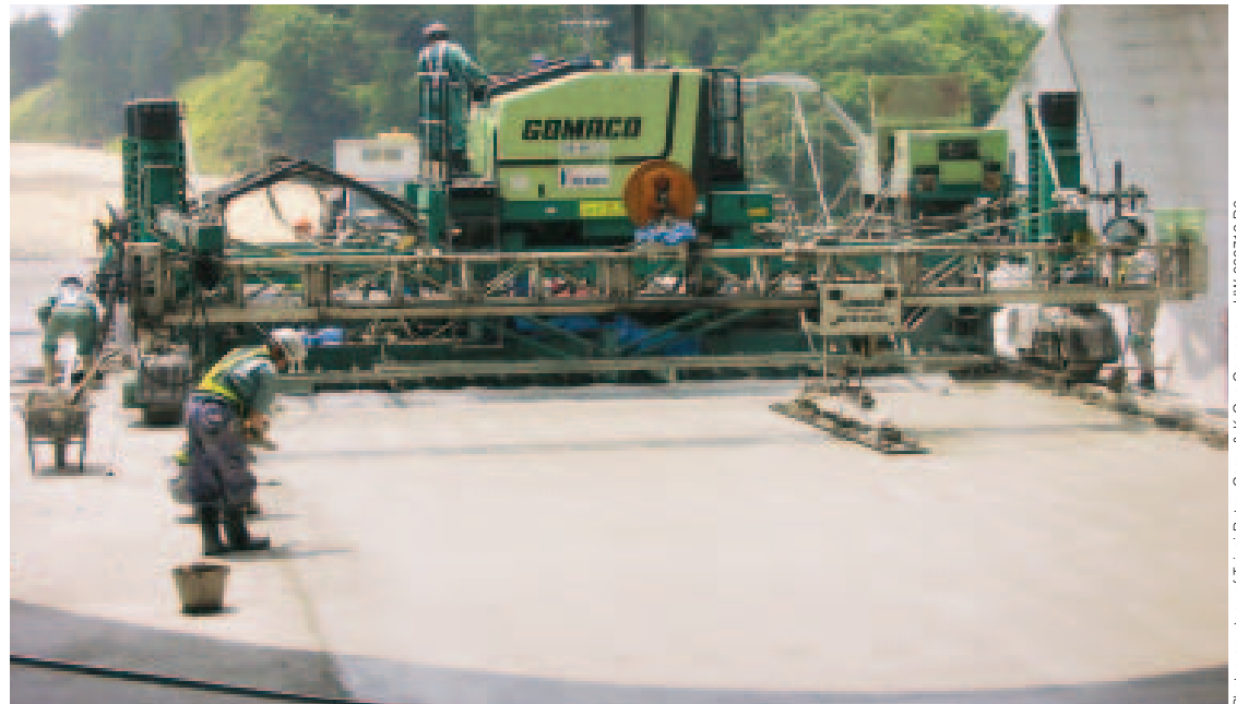
A Commander III slipforms roadway out of the Rittou Tunnel on Meishin Highway Road in Japan.
