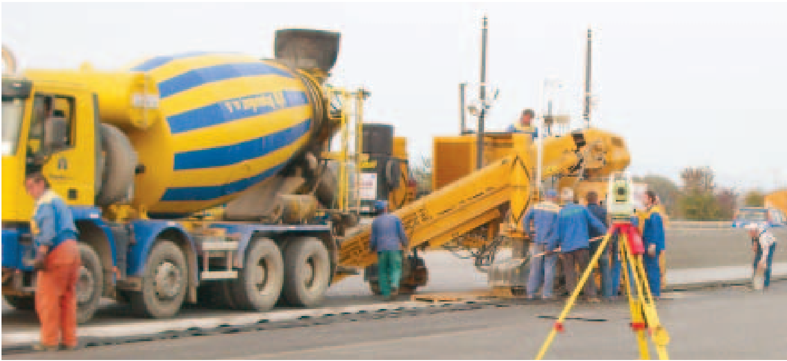
Doprastav is slipforming a 4 km (2.5 mi) long section of barrier wall on Slovakia's Motorway D1 without the use of stringlines.
