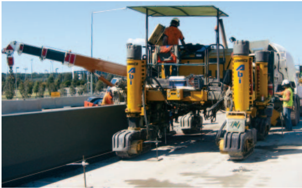
Abi Group Limited slipforms barrier wall with their four-track Commander III on the M7 Motorway near Sydney, New South Wales, Australia.
