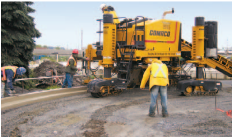
Imperial Paving Limited slipforms curb and gutter with their three-track Commander III on a parking lot project in New Westminster, British Columbia, Canada.
