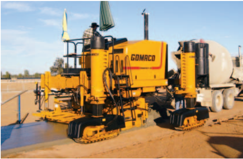
The Commander III is performing triple duties... flat slab, feed bunk and roadway on a cattle feedlot project in Australia. It's slipforming the flat slab in the above photo.
