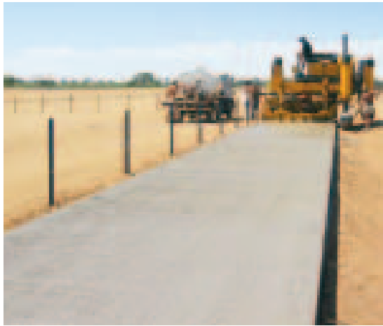
The flat slab has a roller dimple finish to help the cattle create traction and grip on the concrete.
