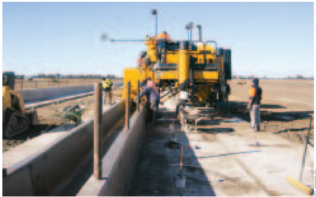
Once the project is complete, they'll have slipformed 15 km (9.3 mi) of flat slab and feed bunk with the Commander III.
