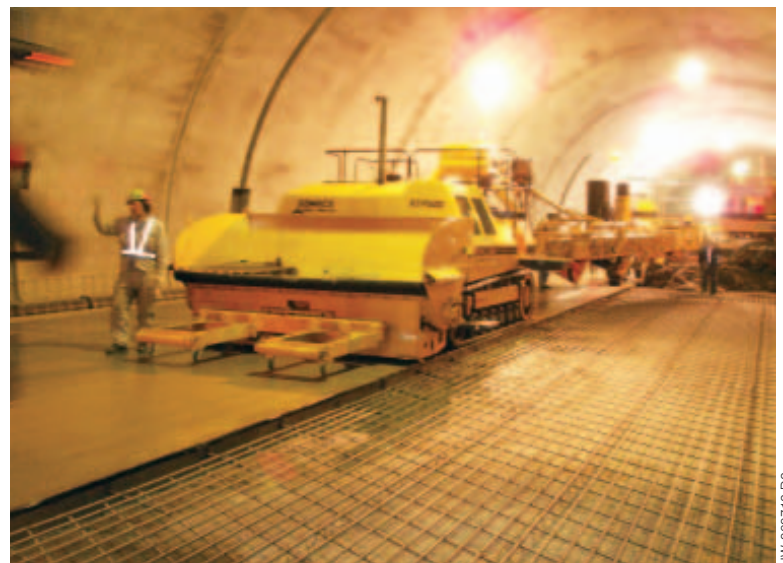
The RTP-500 has an extended truck pusher to accommodate the specially-designed concrete trucks working in the tunnel.
