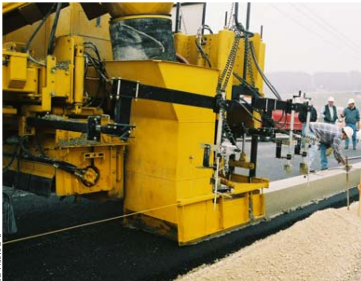
Twehous sideshifts and lifts the GT-3600's trimmerhead up out of the way as they slipform directly on the asphalt road.
