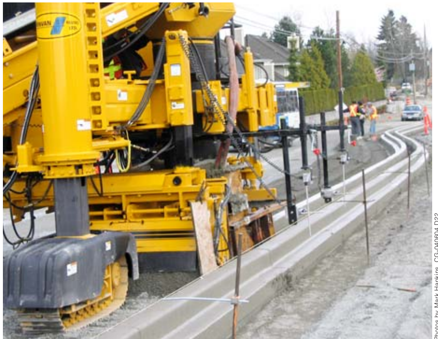
16 Side-by-side curb and gutter divides two streets on a subdivision project. The gap is later filled-in with concrete and hand-finished.
