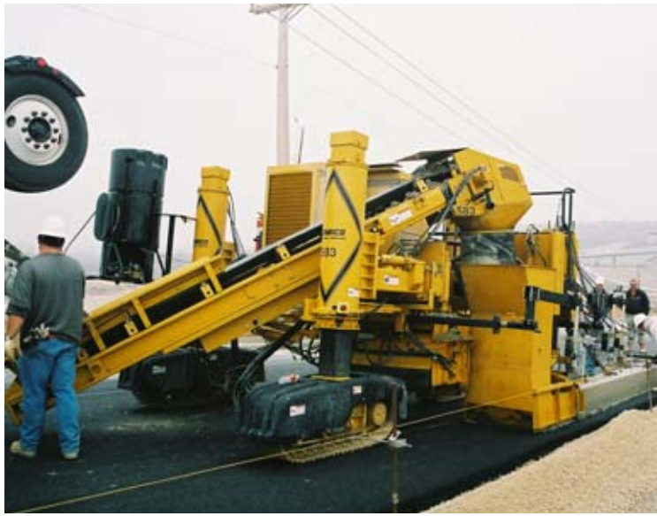
Twehous slipformed curb and gutter on the 12 percent incline on their first day on the project in Jefferson City.
