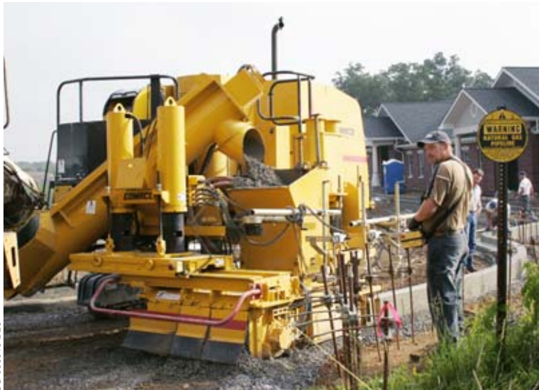
The charging hopper and large capacity hopper helped slipform through several radii on a parking lot in Murray, Kentucky.
