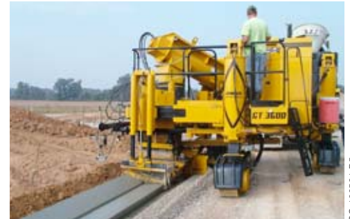
The company slipformed 11,000 feet (3353 m) of rollover curb on a new subdivision project.
