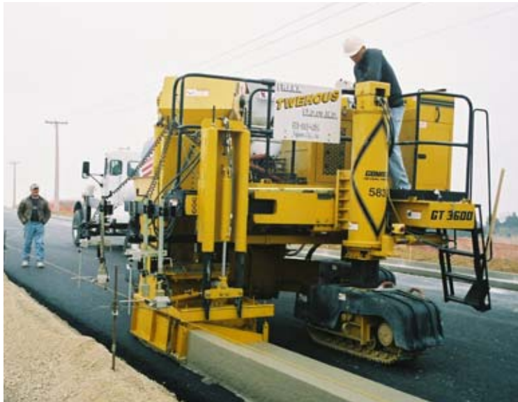
The GT-3600 is equipped with the new Hook-and-Go mold mount, which makes changing molds fast and easy.
