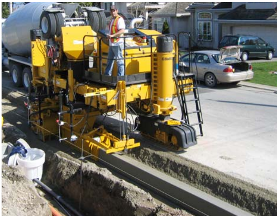
Rehab projects often times leave Winvan pouring curb and gutter in a trench.
