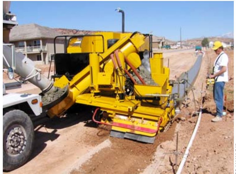
The GT-3400's powerful direct-drive trimmerhead cut through tough grade conditions on a project in Utah.
