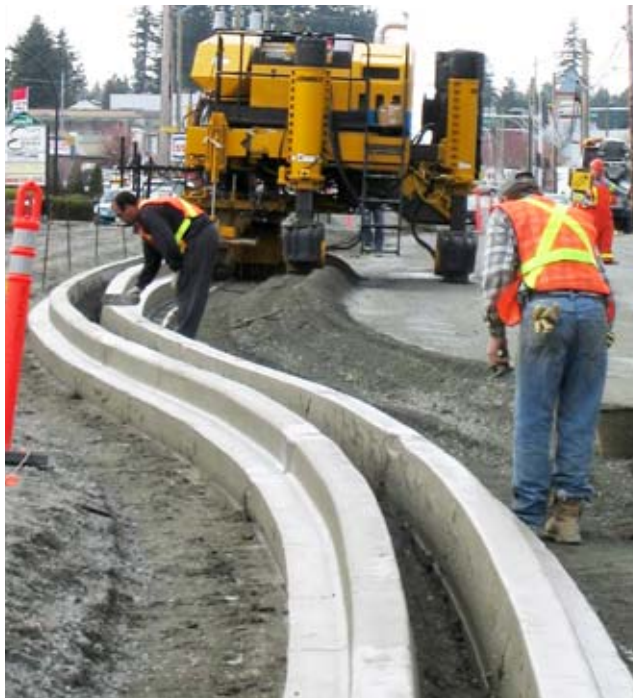
16 Side-by-side curb and gutter divides two streets on a subdivision project. The gap is later filled-in with concrete and hand-finished.
