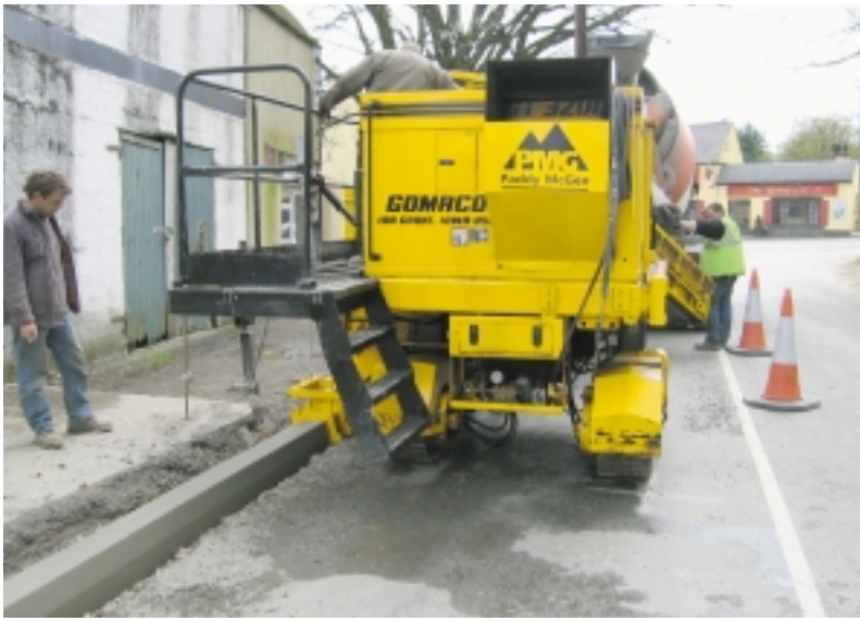
Paddy McGee uses their GT-3200 to slipform a stand-up curb profile in Wexford, Ireland.
