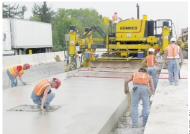
Finishers work behind the Commander III digging out electrical boxes in the pavement that are every 250 feet (76 m).
