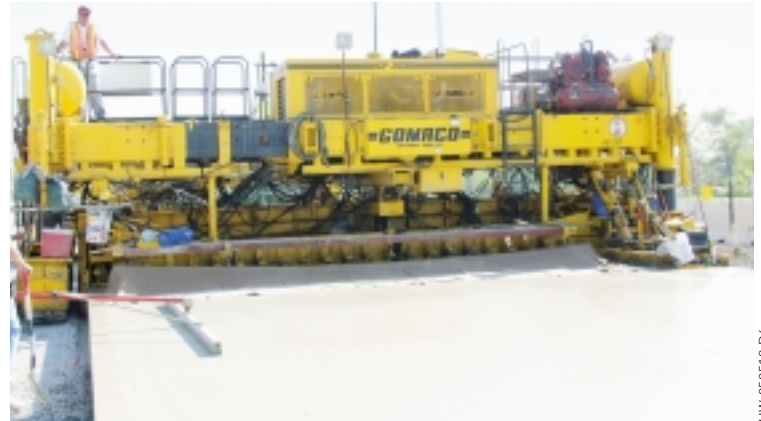
The Fort Wayne roadway requires a two percent crown in the 12 foot (3.7 m) lane, while the 14 foot (4.3 m) lane has a four percent crown.
