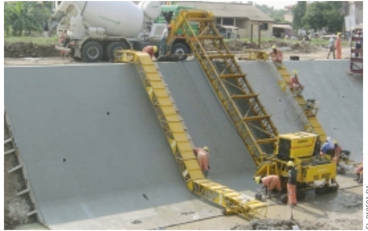
Interbeton bv of the Netherlands finishes a fill-in section of canal on the Odaw River near Accra, Ghana. They are reshaping and relining a 1.7 mile (2.75 km) section of the canal with an SL-450. The bottom width is 42.7 feet (13 m) with a top width of 75.5 feet (23 m). The slope is 1:1.
