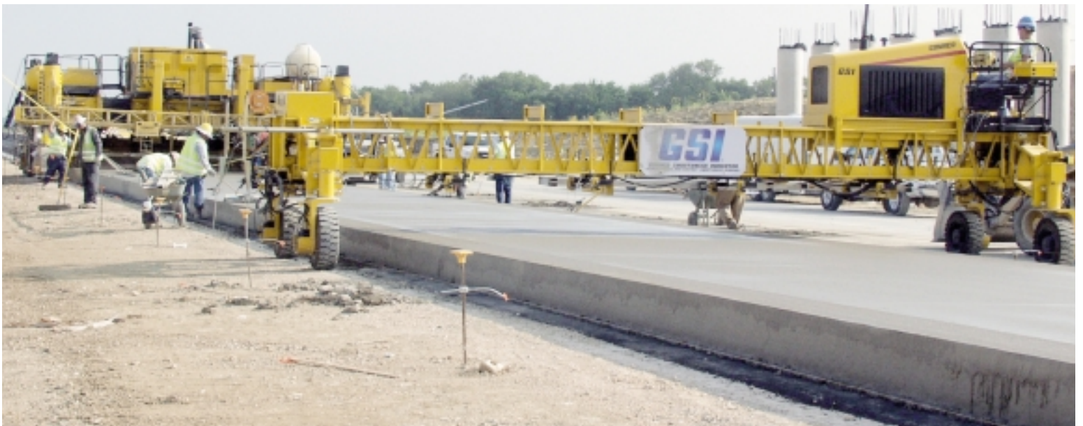
Rideability of the new concrete roadway is constantly being monitored by the GOMACO Smoothness Indicator (GSI).
