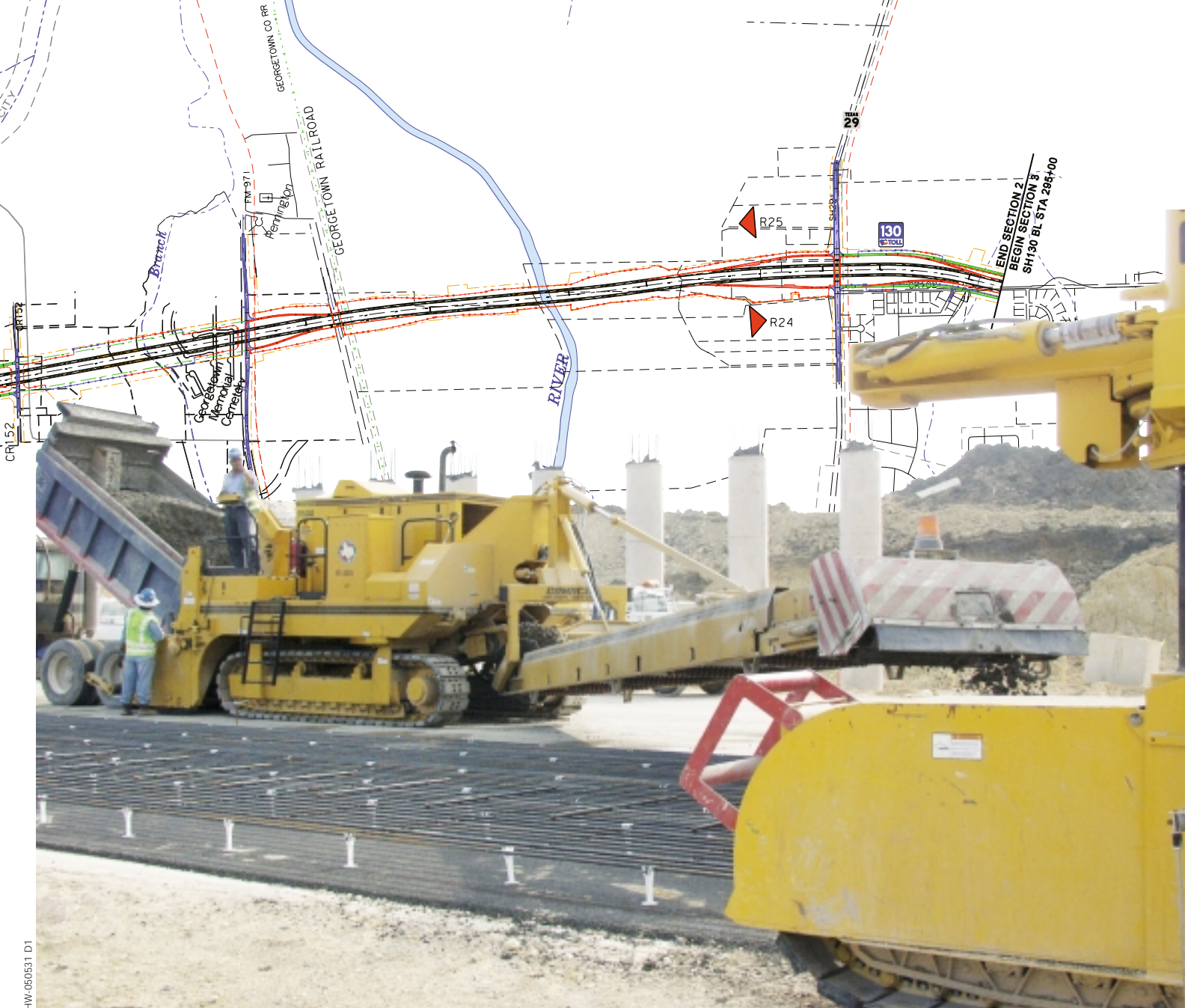
The 9500 places concrete over the continuous steel reinforcing in front of the GP-4000 four-track paver.
