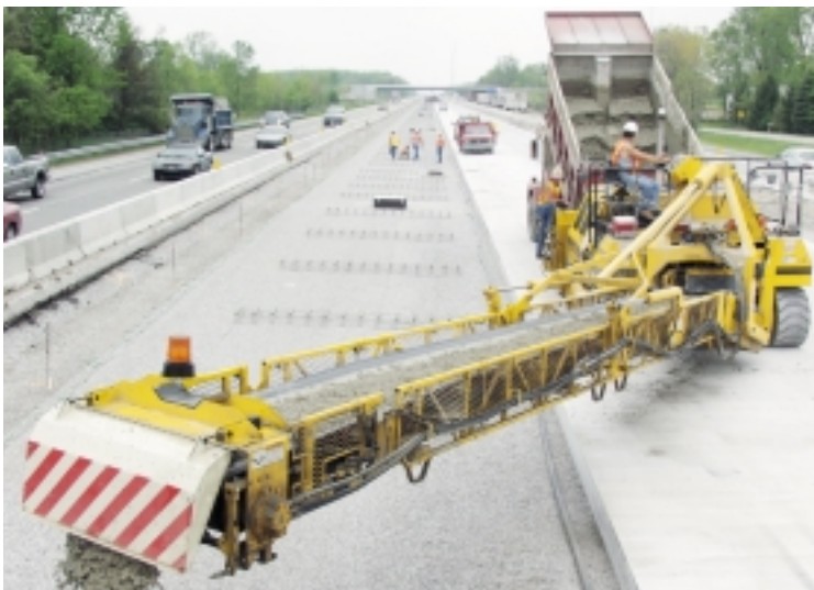
The RTP-500 runs on the new pavement, off to the side of the grade, placing concrete in front of the Commander III.
