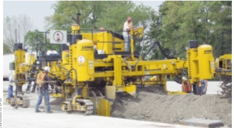
The Commander III with the V2 dual mold system allows E&B to make a two foot (0.6 m) width change in a matter of minutes.
