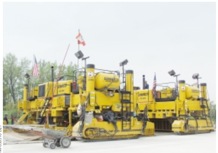
The new Borman Expressway is being built for a life expectancy of 25 years, carrying over 160,000 vehicles per day.
