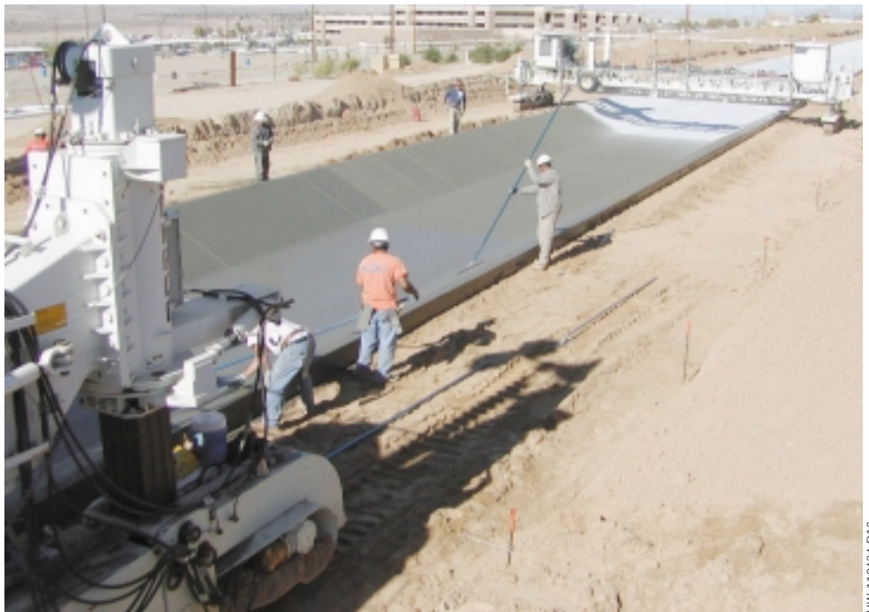
Baldi Brothers' GP-4000 paver was equipped with a chain-type trimmer to trim the final profile of the canal. They trimmed and poured simultaneously with their GP-4000 and achieved excellent production results.
