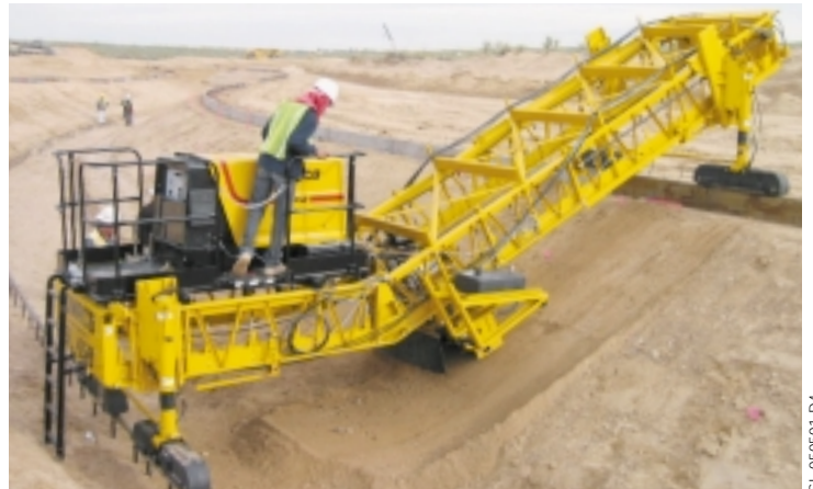
Salls Brothers Construction use their new SL-450 with trimmer attachment in Rio Rancho, New Mexico. They were trimming approximately 2.5 to three inches (64 to 76 mm) of sandy soil. The canal will have a shotcrete finish.
