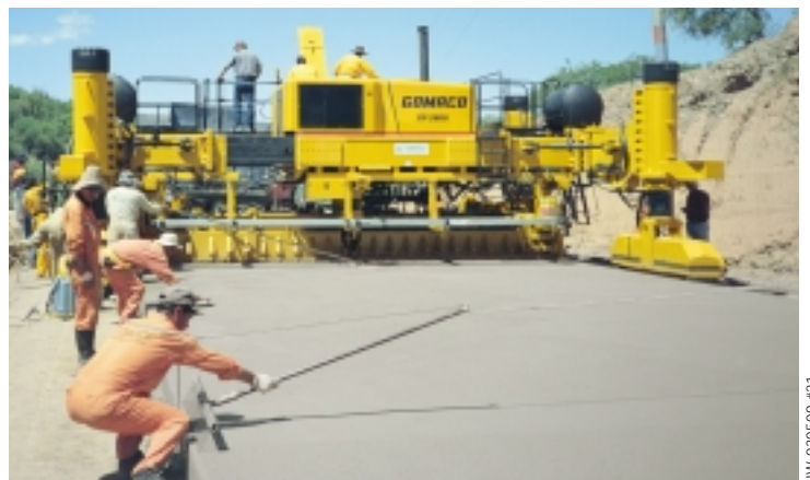
Coboce Ltda. slipforms a concrete roadway with their new GP-2600 near Cochabamba, Bolivia.
