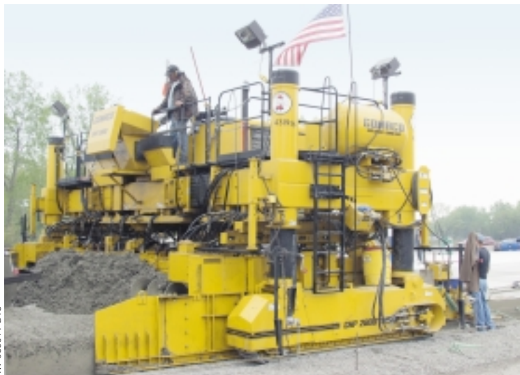
The two-track GHP-2800 paver is helping E&B earn 97 percent bonus incentive on their new mainline paving.
