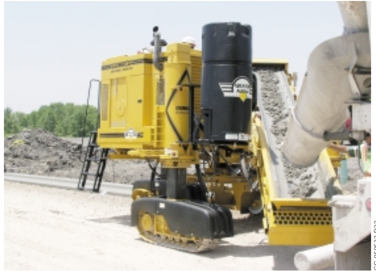
Concrete slump will average between 1.5 to two inches (38 to 51 mm), depending on base material and temperature.
