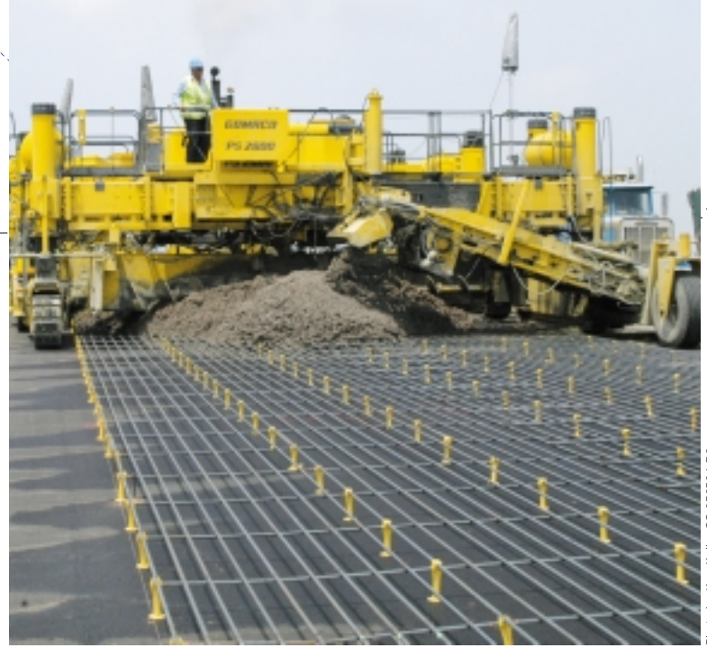
A PS-2600 placer/spreader is also being used on the project for placing and spreading concrete at the wider paving widths.
