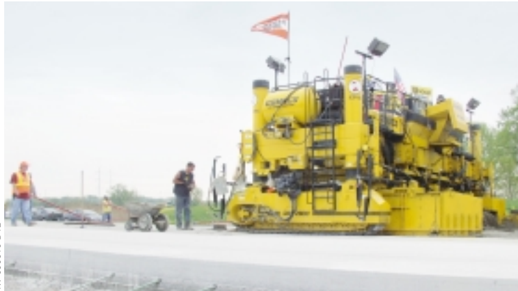
The new GHP-2800 is paving 24 feet (7.3 m) wide, 15 inches (381 mm) deep on the project in Gary.
