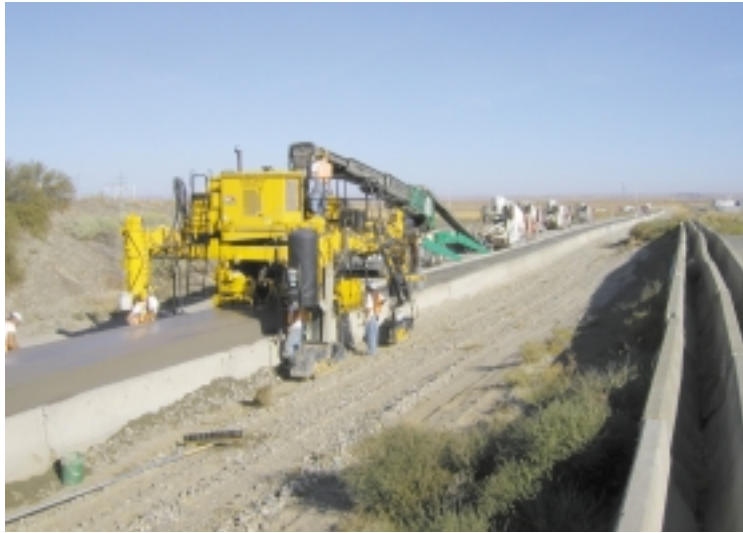
The old barrier wall varied in height from one section to the next so the GT-6300 was used to blend the differences smoothly.
