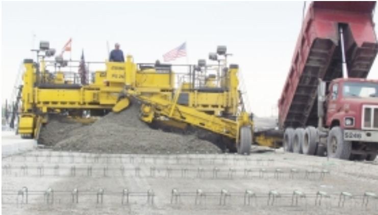
A new PS-2600 placer/spreader leads the GOMACO paving train on the project in Gary, Indiana.
