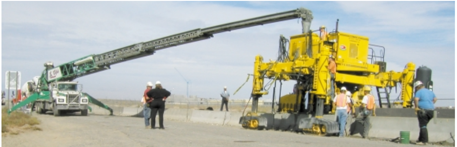
A Telebelt® placer was brought in to feed concrete to the GT-6300. Production averaged just under 1300 feet (396 m) per day.
