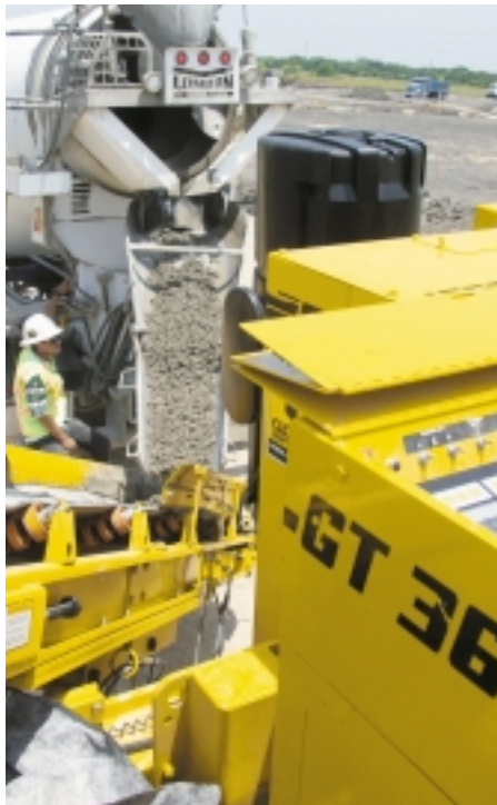
The operator has a clear view of the conveyor, concrete truck and chute man.
