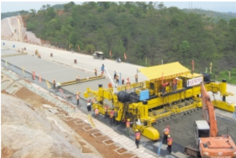
Guangdong Changda uses their GP-4000 paver with In-The-Pan Dowel Bar Insertter (IDBI) to mainline pave in the Guangdong province of China.
