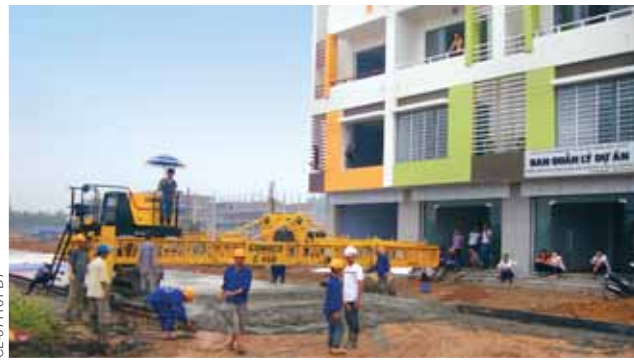
A C-450 finishes a residential road 7.6 meters (24.9 ft) wide by 250 millimeters (9.8 in) thick for contractor Bao Quan in Vihn Yen City, Vietnam.
