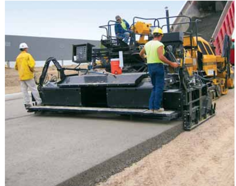
A worker makes adjustments on-the-go from the RCC screed's work bridge.
