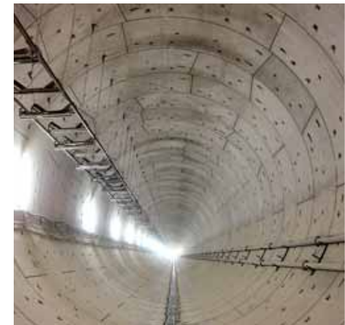
The inside of the tunnel before the installation of the concrete floor...
