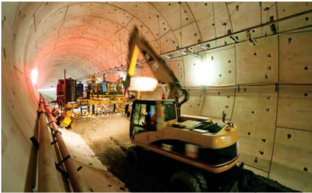
An excavator worked in front of the Commander III, spreading the concrete across the width of the tunnel.
