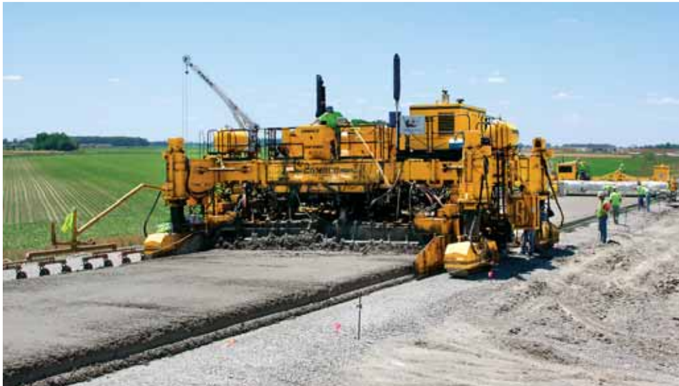
Shelly & Sands uses a placer/spreader to keep a consistent amount of concrete in front of the GHP-2800 paver, which helps them achieve smooth rideability numbers.
