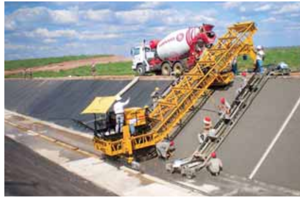
Camter finishes a portion of the São Francisco Canal with their SL-450 cylinder finisher in Floresta, Brazil.
