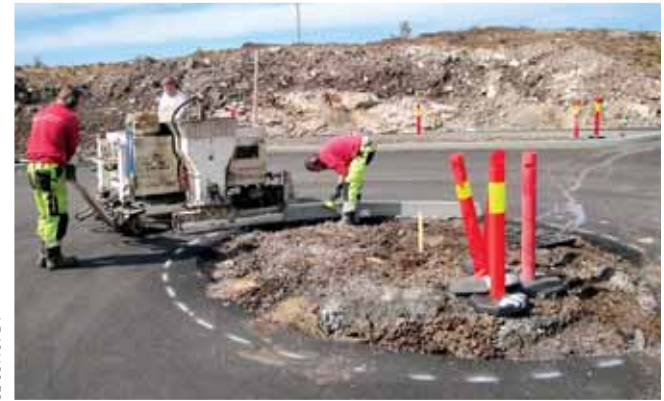
A Curb Cadet extrudes curb around a radii for Asphalt og Maskin A/S in Bergen, Norway.
