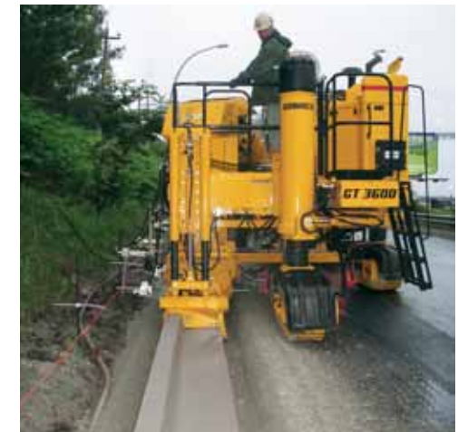
Brycon Construction Ltd. slipforms curb and gutter with their GT-3600 on a rehab project in Halifax, Nova Scotia, Canada.
