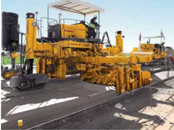
Tarcutta Hume Alliance reversed the tracks on their four-track Commander III so the machine could travel backwards while keeping the controls in forward. The side-mounted shoulder is paved two meters (6.6 ft) wide and 240 millimeters (9.4 in) thick in Tarcutta, New South Wales, Australia.
