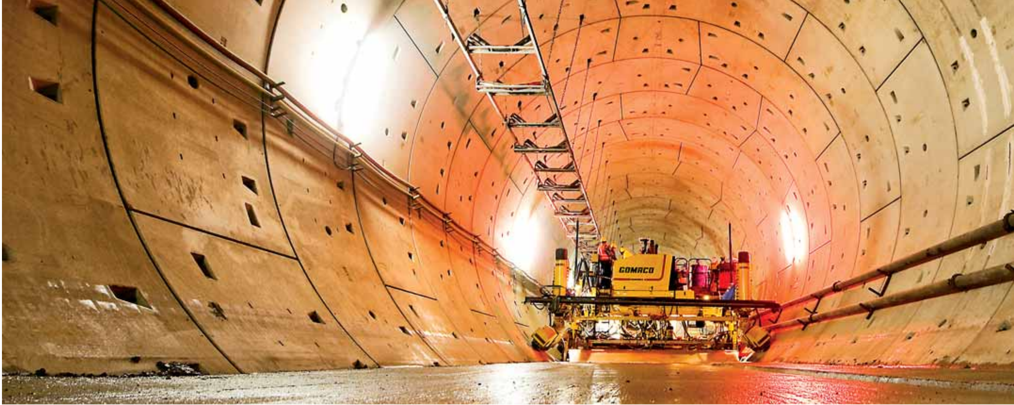
A GOMACO Commander III slipforms inside one of two seven kilometer (4.3 mi) long tunnels that are part of the Finne Tunnel project between Leipzig and Erfurt, Germany.
