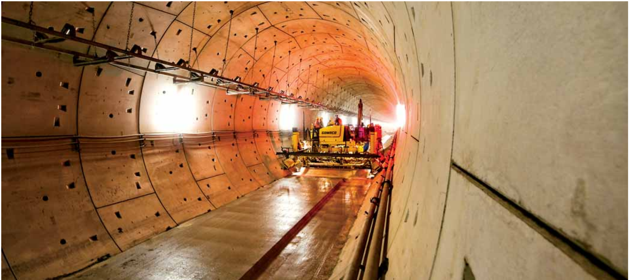
The Commander III's tracks were turned at 35 degree angles to pave inside the circular tunnel. The floor's profile was slipformed with a 720 millimeter (28.3 in) wide drainage channel.
