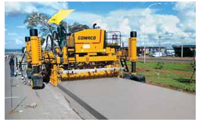
EPC Paving Brasilia slipforms a new bus route with their four-track Commander III in Brasilia, Brazil.
