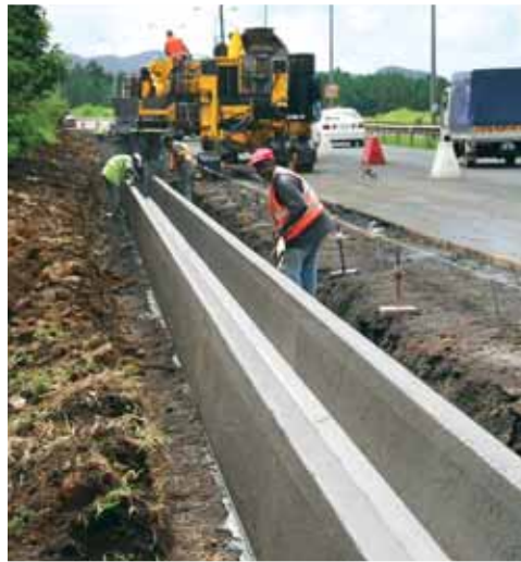
The 4400 slipforms left-side pour U-channel, 500 millimeters (19.7 in) tall, below grade next to an existing roadway.
