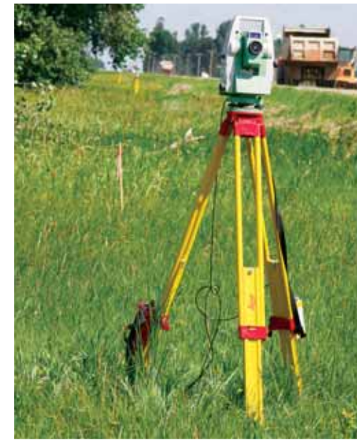
Total stations set up on a 3D project.
