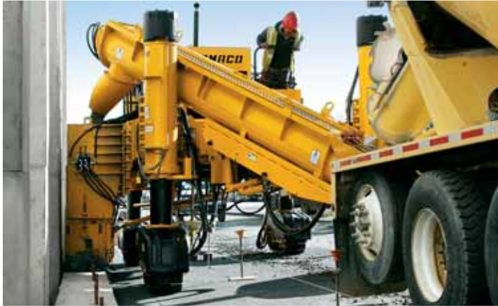
The right-side pour barrier wall is slipformed on top of a footer, right next to a new sound wall along the Capital Beltway.
