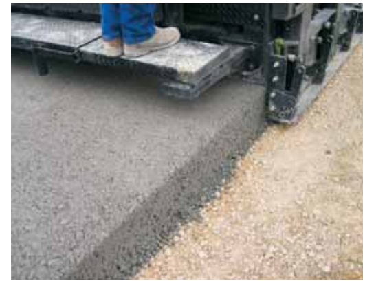
GOMACO's RCC screed produces a sharp edge on the new roadway.
