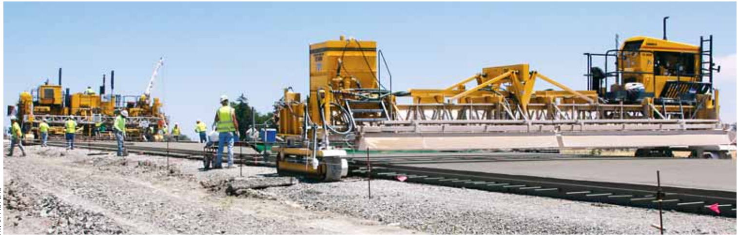
Shelly & Sands Inc. is paving Ohio's U.S. Route 24 with their GOMACO paving train, which includes a GHP-2800 with IDBI. The project uses the IRI to measure smoothness and Shelly & Sands has achieved some outstanding results and earning incentive.
