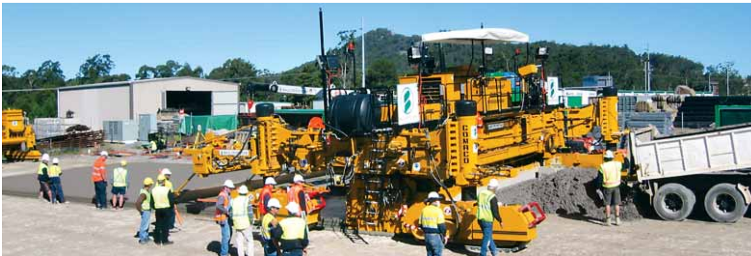
A test pour with the GP-4000 paver and Leica Geosystems stringless controls went well for Baulderstone Hornibrook Pty Ltd in Bulahdelah, New South Wales, Australia. They are now slipforming on the Pacific Highway upgrade project by Bulahdelah.
