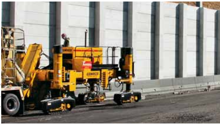
The new 4400 is slipforming barrier wall flawlessly on Tavares Concrete’s projects around the Washington, D.C., area.
