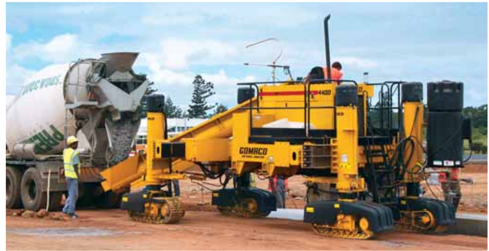
Colas Maurice introduced slipform paving to the island of Mauritius last year with a GOMACO Commander III. This year they purchased a new 4400 to slipform various applications from the right-side and left-side of the paver.
