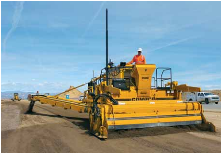
A GOMACO 9500 trims with 3D on a new highway project near Reno, Nevada.
