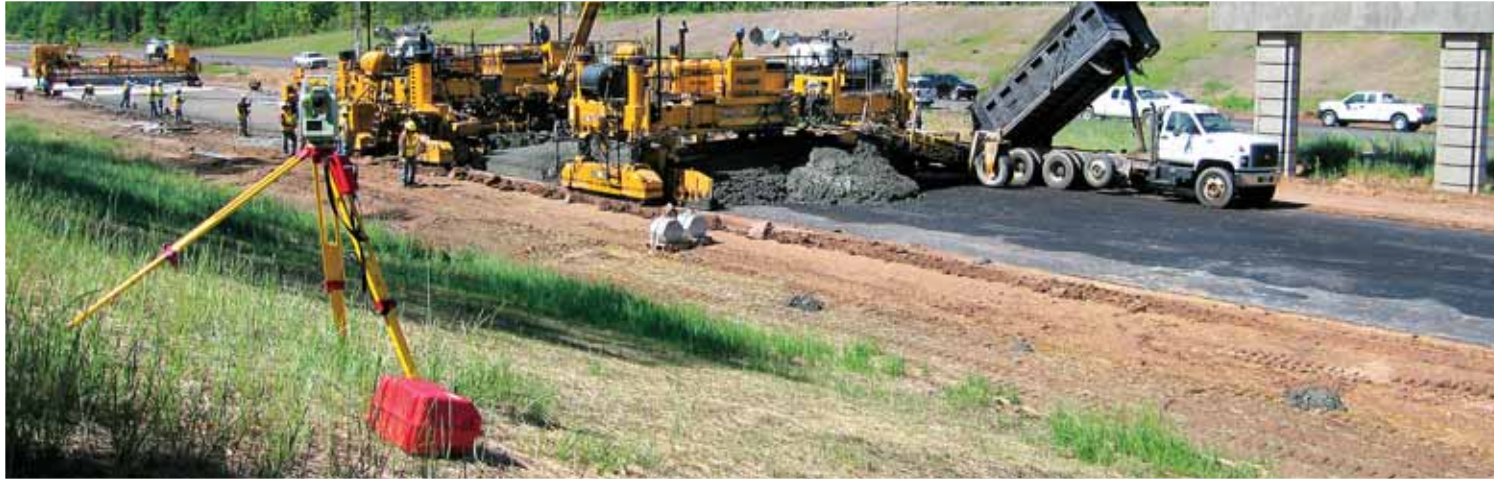
A GOMACO paving train with 3D controls on both the PS-2600 placer/spreader and GHP-2800 at work near Cary, North Carolina.
