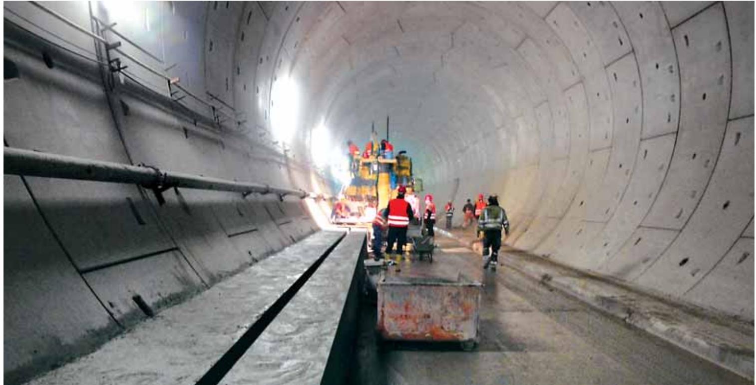
The walkway mold's telescoping ability allowed it to compensate for changes in the tunnel's alignment. The walkway mold could telescope up to 700 millimeters (27.6 in) in width and up to 350 millimeters (13.8 in) in height.
