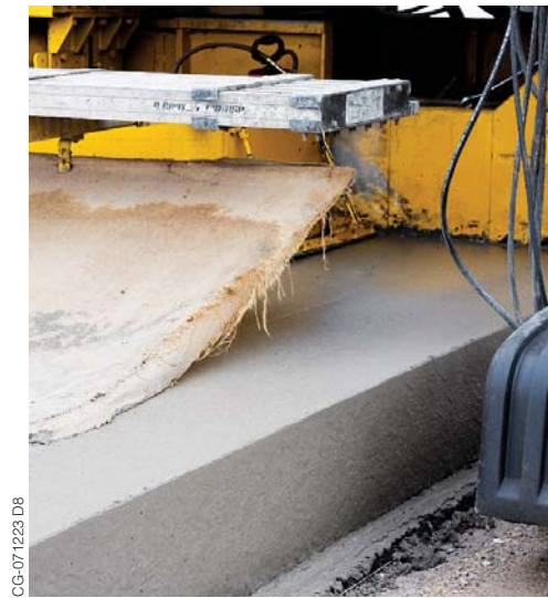
The Commander III with V2 mold produces the sharp GOMACO edge.
