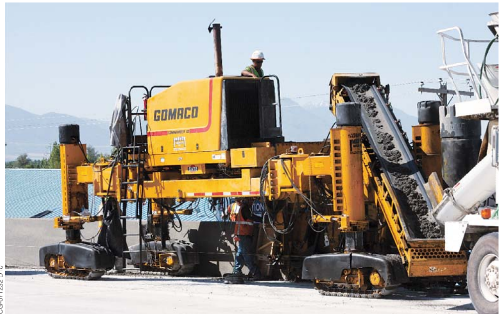
Harper Concrete is using both a three-track and a four-track Commander III to slipform their portion of barrier wall along the new stretch of interstate.
