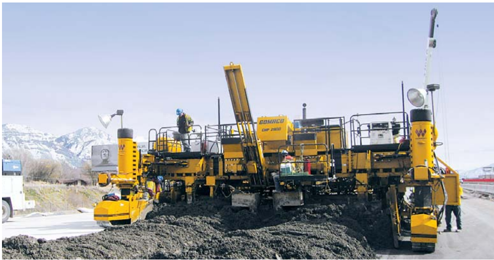
A frame-mounted bar inserter on the front of the GHP-2800 and a sidemounted bar inserter on the rear of the paver inserted bars every 30 inches (762 mm) into the new roadway.
