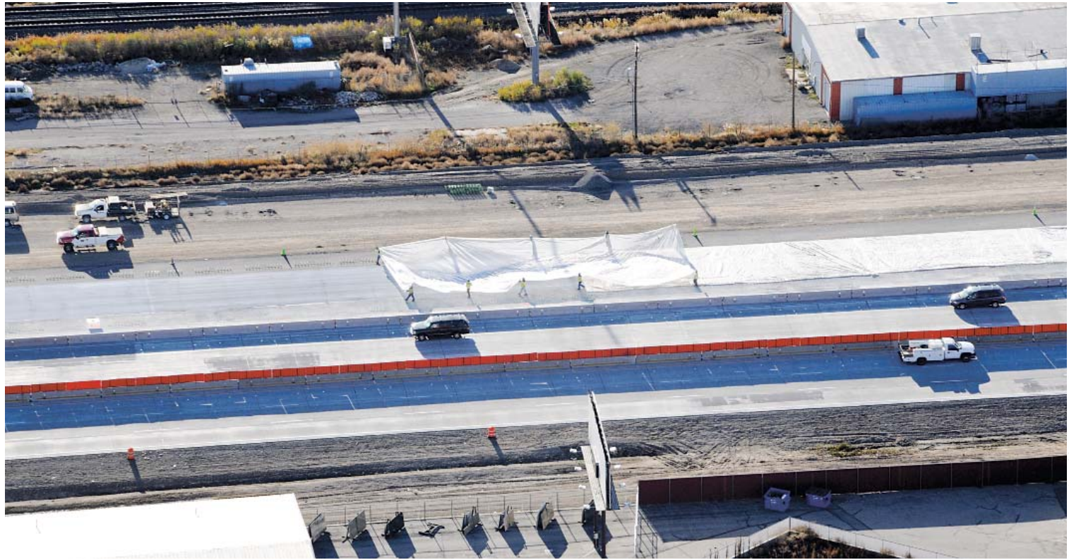
Paving through Utah's below-freezing winter temperatures was necessary to complete the enormous project on time. PRC worked together with UDOT to reinvent cold weather paving protocols and establish new standards for winter paving.
