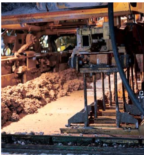
The IDBI's forks wait in stand-by position for the next insertion process to begin.
