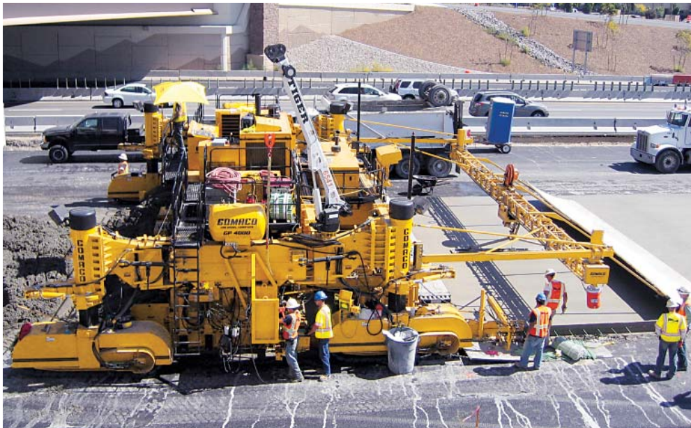
The GOMACO GP-4000 with IDBI attachment slipforms 39 feet (11.9 m) wide on the northern portion of the I-15 CORE project.
