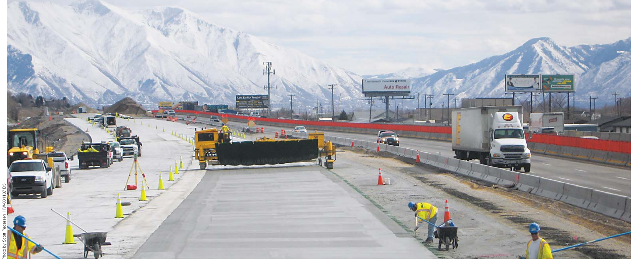
Miles of temporary barrier wall separates live traffic from the construction work as just one part of the detailed and comprehensive management of traffic plan in place on the project.
