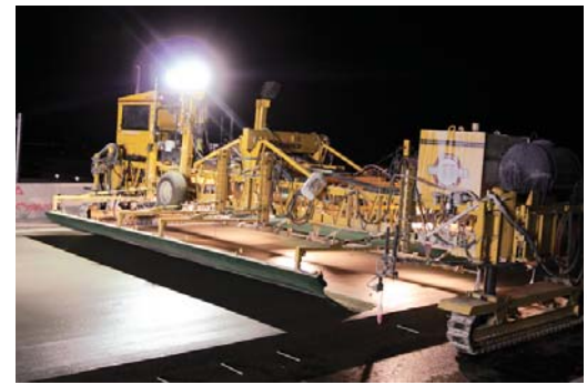
A GOMACO T/C-600 applies an Astroturf drag finish behind the two-track GHP-2800.
