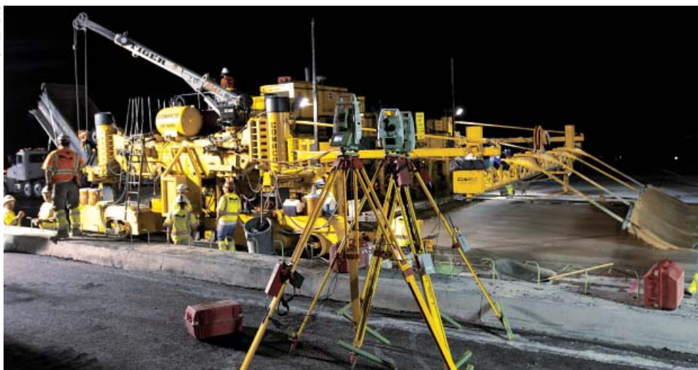
Paving would often times take place 24 hours a day, seven days a week. The GP-4000 paving crew slipformed 26 feet (7.9 m) wide during this night pour.
