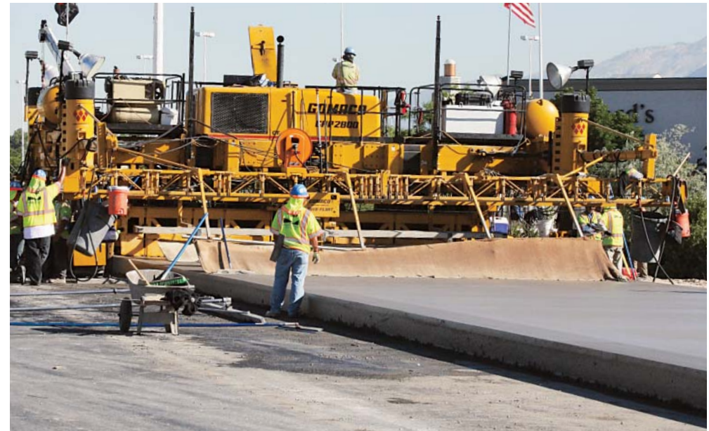
Three GOMACO GHP-2800s are at work on the project. Two of them are four-track pavers with IDBI attachments, and one is a two-track machine.
