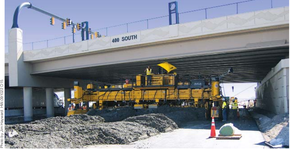
The GP-4000 with IDBI attachment paves underneath the 400 South interchange.
