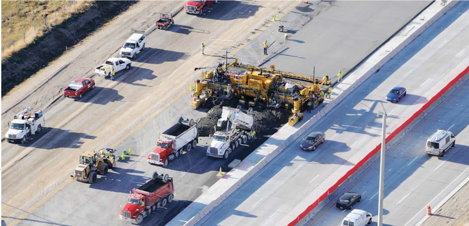
The northern section of the project is six travel lanes wide northbound and southbound for 12 lanes of concrete pavement.
