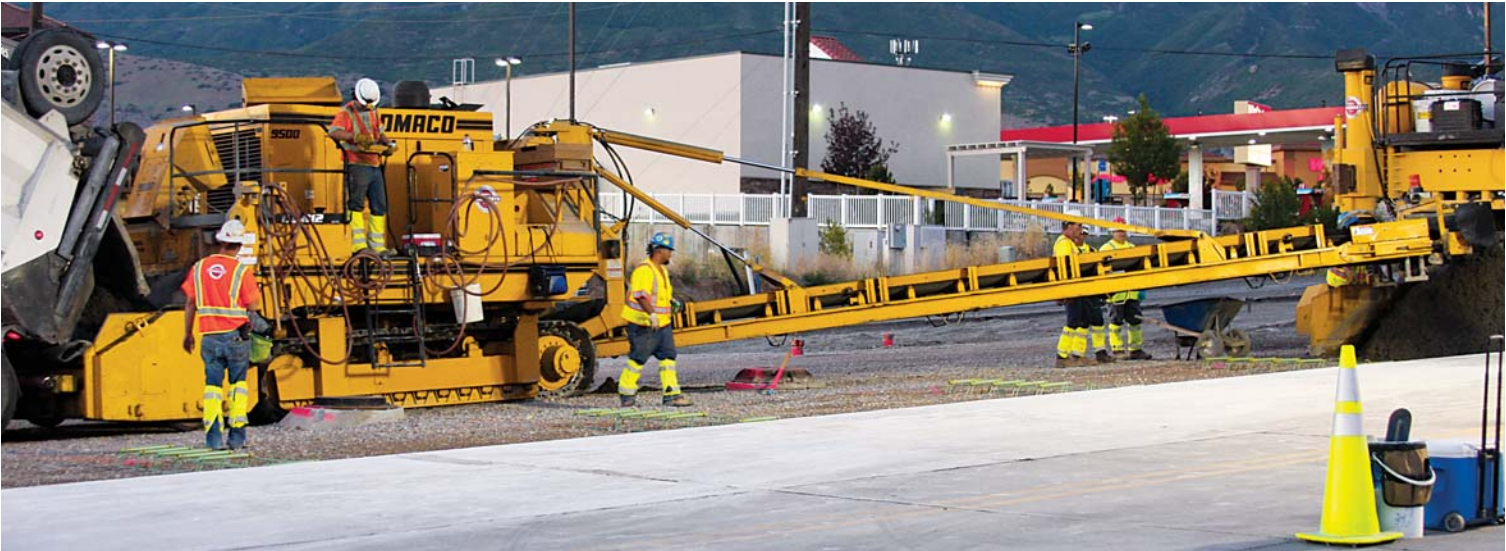
The operator on the 9500 works with the placer's remote control and can move along the operator's platform to get the ultimate view of both the concrete truck dumping into the hopper and the belt placing in front of the GHP-2800 paver.
