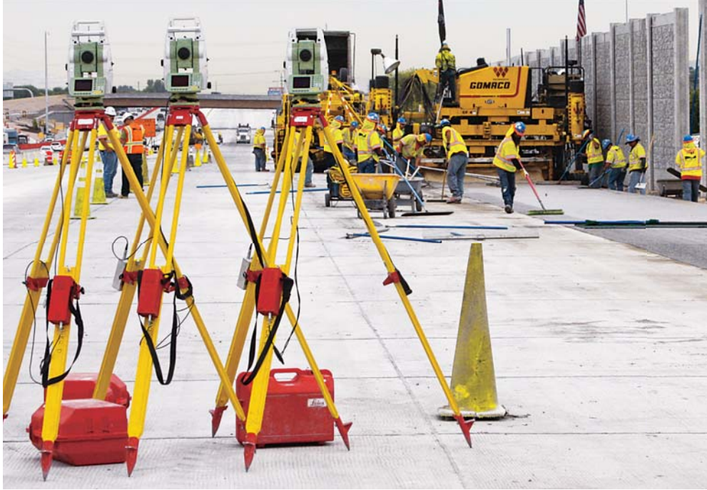
Five total stations are used on each pour. Three work with the paver, set up at 200 foot (61 m) intervals and the other two are used for grade checks.
