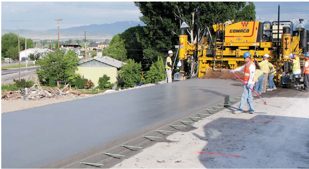
The GOMACO Commander IIIs on the project are slipforming a variety of applications, including ramps, shoulders, and zero-clearance median.
