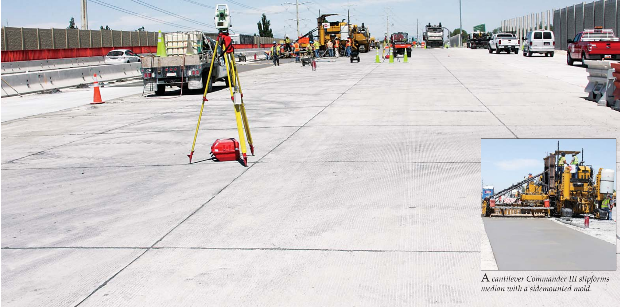
A 13 foot (4 m) paving mold remains mounted underneath the Commander III as it slipforms with its sidemounted mold. This allows for quick paving application changes.
