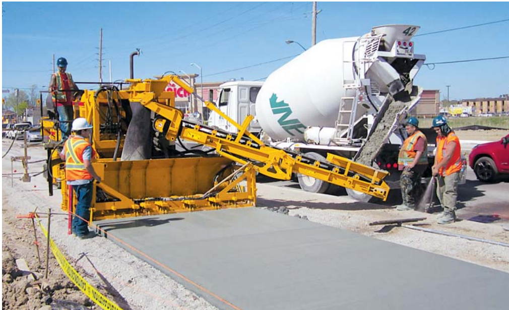
The GT-3200 sidewalk paver is specifically designed for sidewalks and minimum clearance projects. The GT-3200 is slipforming a three meter (10 ft) wide sidewalk.
