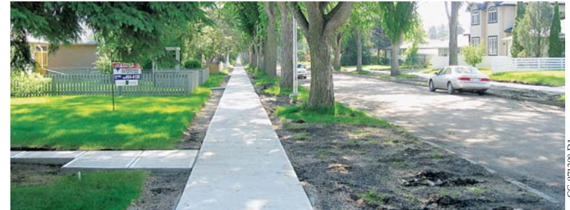
This sidewalk was slipformed by a GT-3200 sidewalk paver within an existing residential area. The paver's minimum clearance allowed for high production on this sidewalk replacement project.
