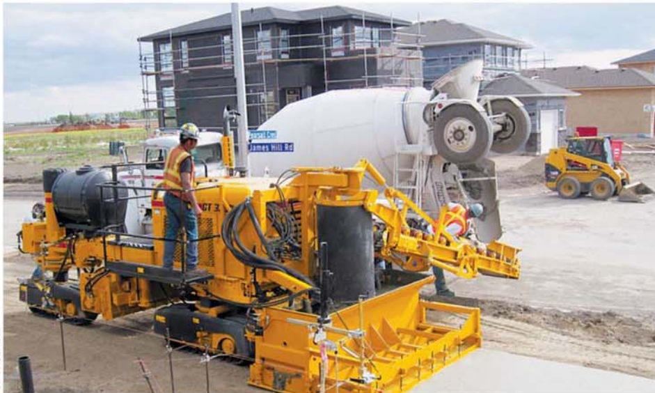
The GT-3200 sidewalk paver can slipform widths up to 3.66 meters (12 ft) with a well-prepared grade.
