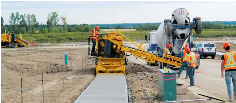
The GT-3200 sidewalk paver slipforms a 1.5 meter (5 ft) wide sidewalk through a future housing development.
