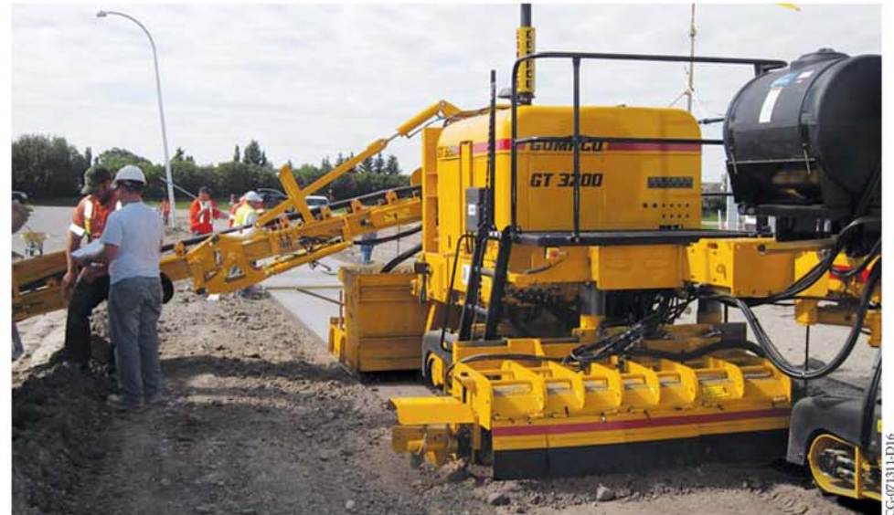
The GT-3200 sidewalk paver can be equipped with a trimmerhead for fine grade trimming. The GT-3200 above is simultaneously trimming the grade and slipforming the sidewalk for a future residential area.
