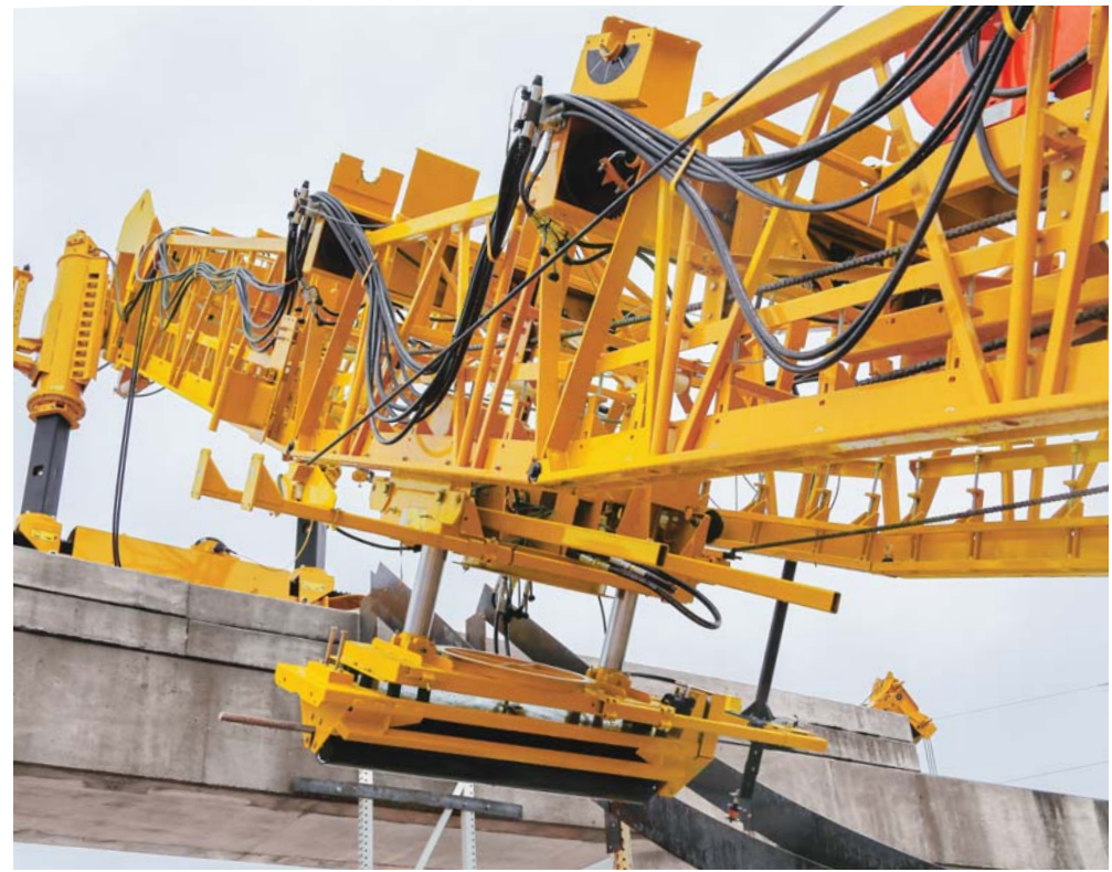
The SL-750 features an undercarriage with hydraulic vertical adjustment controlled by 3D guidance. “Smart” cylinders on the undercarriage allow it to move up and down for precision paving of the test track’s changing slope.
