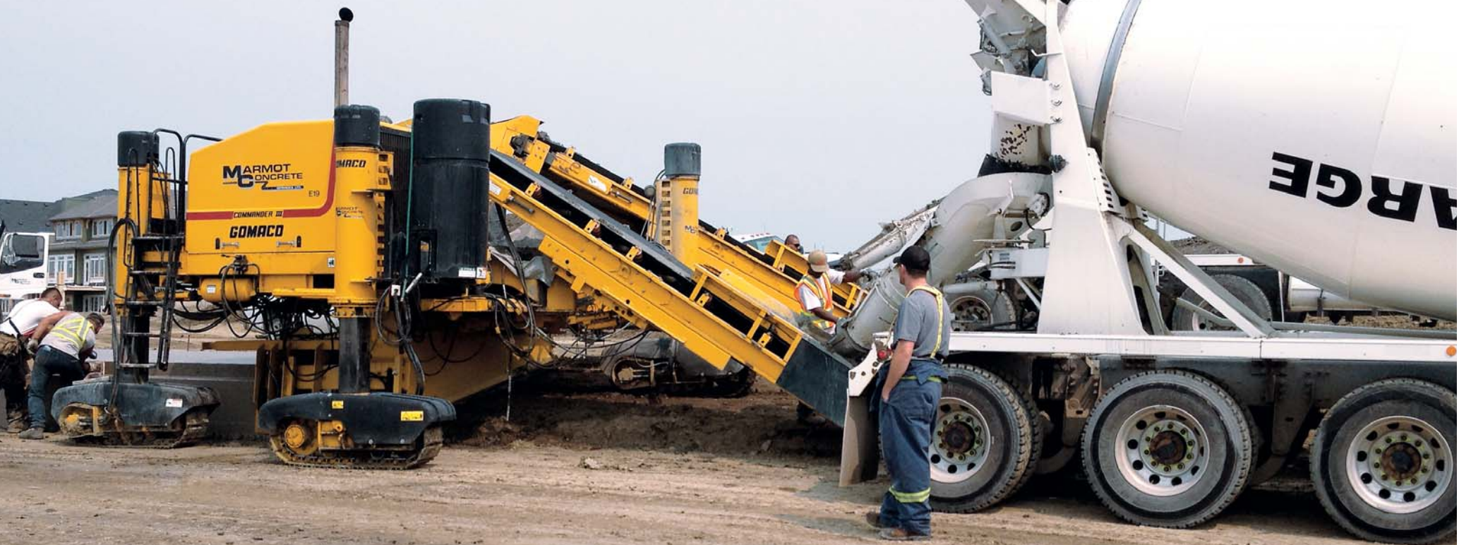
Two conveyor belts mounted to the Commander III were needed to supply enough concrete to the mold for the unique profile around the lake's edge at the Mahogany Central Beach site.
