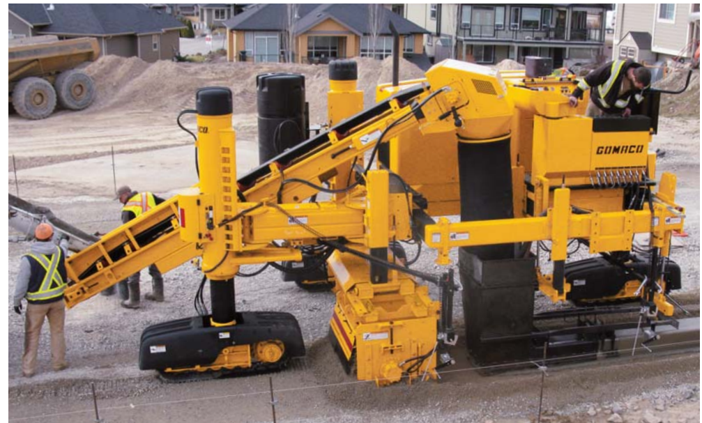
First days production rates reached as high as seven lineal meters per minute (23 ft/min) with Valley Curbing emptying a six cubic meter (7.8 yd 3 ) ready-mix truck in under eight minutes.
