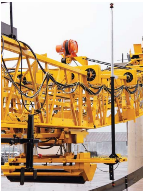
A mast with a Leica Geosystems 3D prism and a slope sensor are used to control the rear “smart” cylinder’s vertical adjustments.
