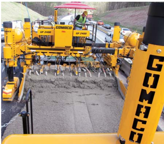
A GOMACO GP-2400 with 5400 series bar inserter follows a PS-2600 placer/spreader on a project in Hamburg, Pennsylvania.
