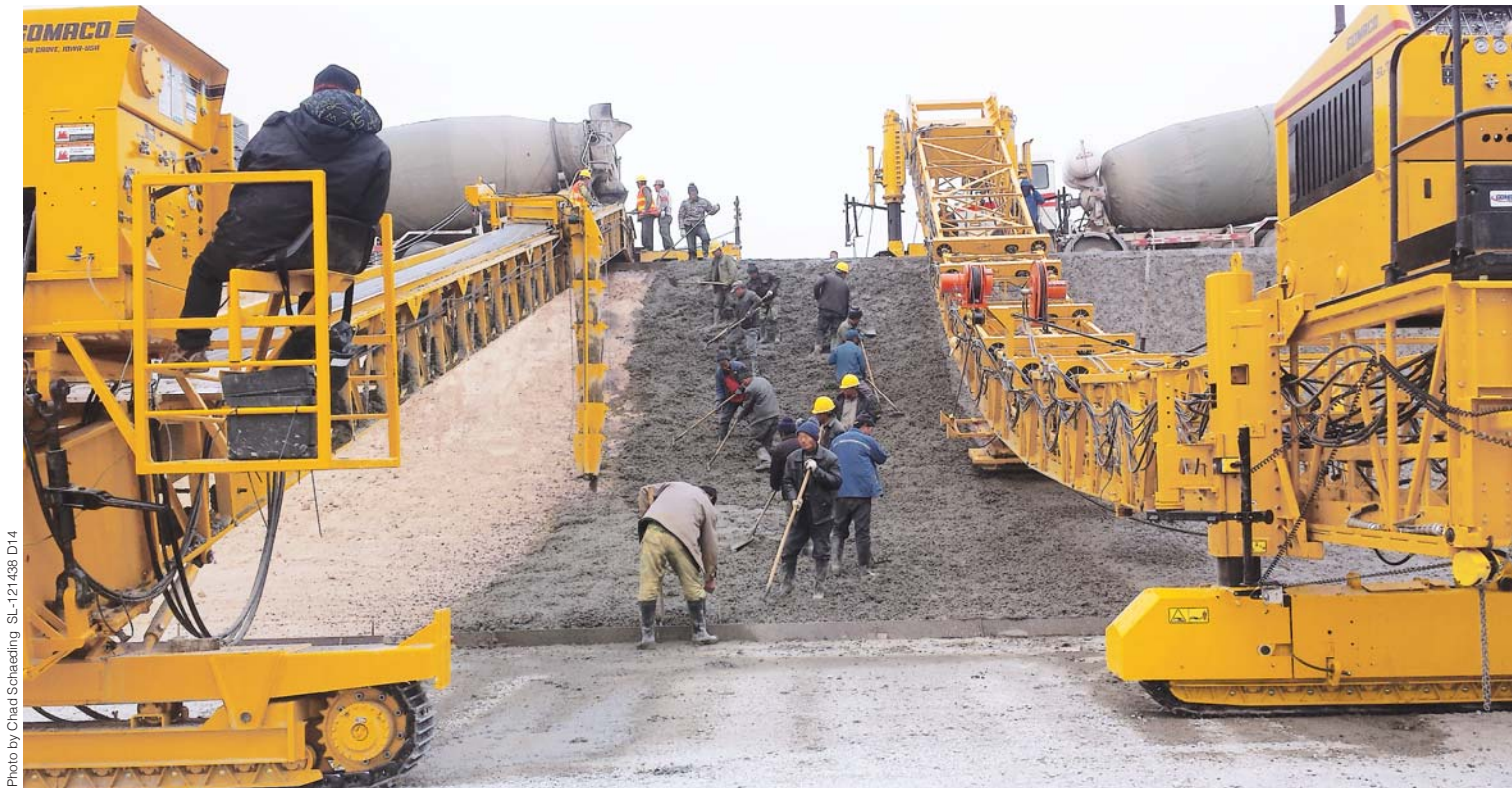
The GOMACO RC Conveyor with telescoping tremie places the lean base material onto the slope of the test track. To prepare the lean base, the SL-750's undercarriage is equipped with an auger that helps level the material. The auger is switched out to a cylinder to finish the concrete layer of the track.
