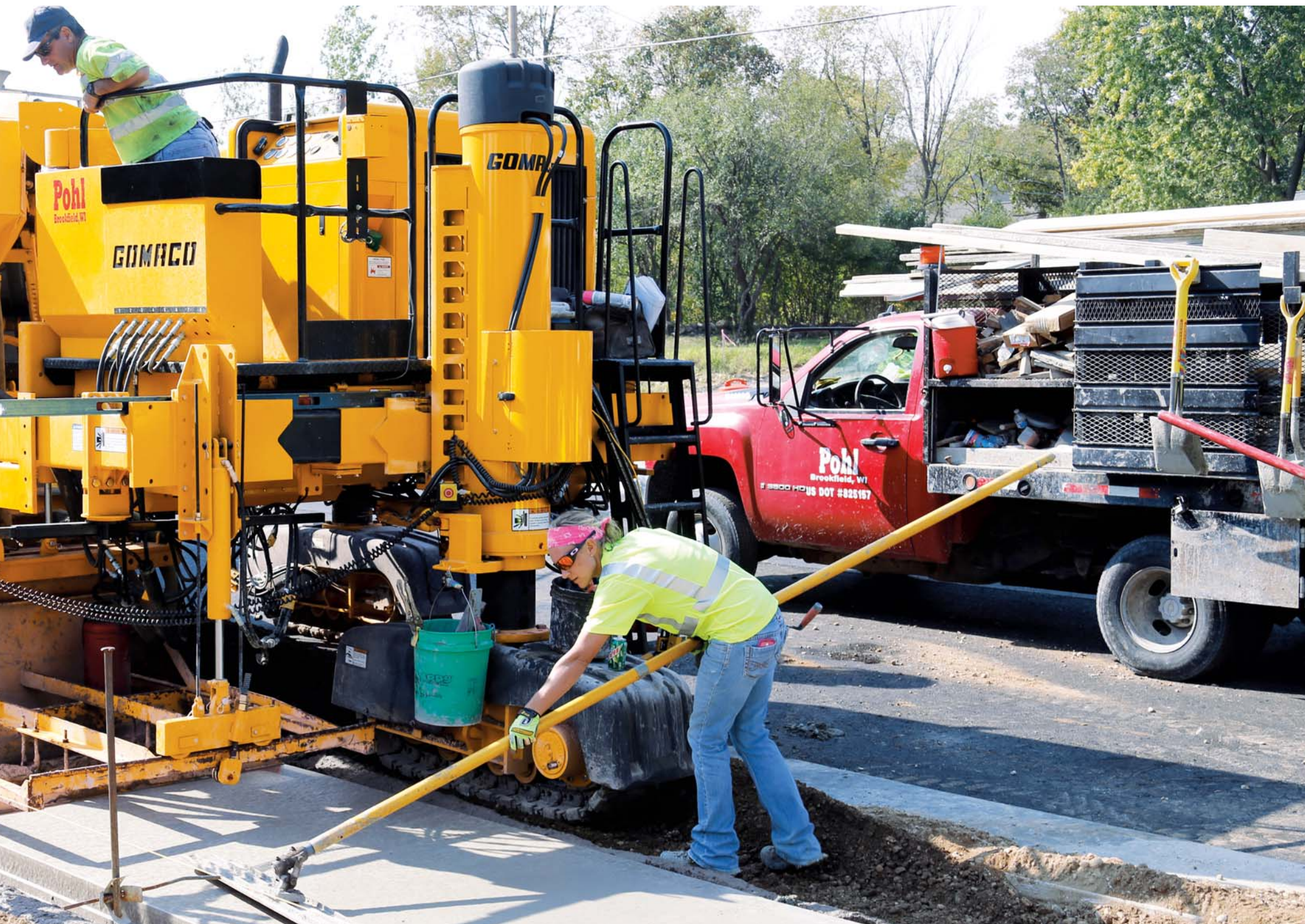
operation with the redesigned operator's platform with a pivoting console, relocated vibrator circuits control panel, isolated platform and more.
