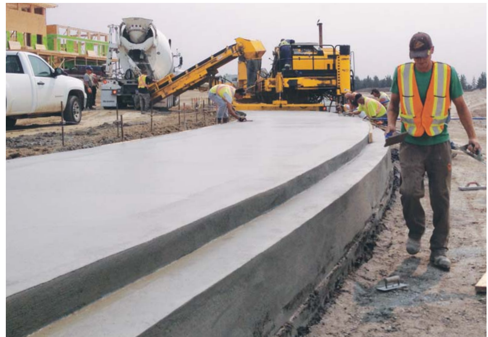
The profile is a 2.5 meter (8.2 ft) wide sidewalk with an 800 millimeter (31.5 in) face that prevents the sand from blowing into the grass at the new development.
