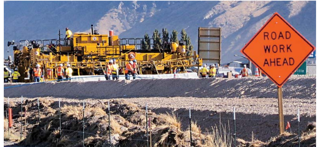
Concrete was the material of choice for the state of Utah’s I-15 Corridor Expansion Project that replaced 24 miles (38.6 km) of Interstate 15 between Lehi and Spanish Fork.
