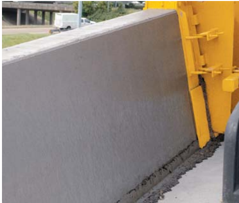
WMC Contracting slipformed 4642 feet (1415 m) of 36 inch (914 mm) tall single slope parapet on the flyover.
