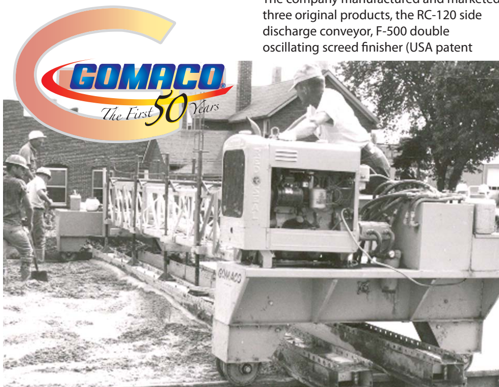
A prototype double oscillating screed bridge deck finisher was first used on a bridge deck in Denison, Iowa, in October 1962.
