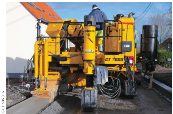
A GOMACO GT-3600 slipforms curb and gutter for a new street in Zingem, East Flanders, Belgium.
