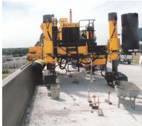
WMC Contracting will be slipforming over 40,000 feet (12,192 m) of four different wall profiles on the Memphis I-40/240 project.
