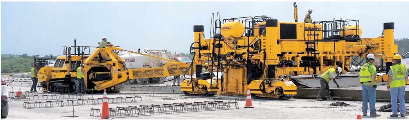
A GOMACO RTP-500 places concrete in front of a GHP-2800 paver at work on the Baltimore/Washington International Thurgood Marshall Airport in Baltimore, Maryland. A complete listing of airports that GOMACO equipment has been on can be found at www.gomaco.com/airports .
