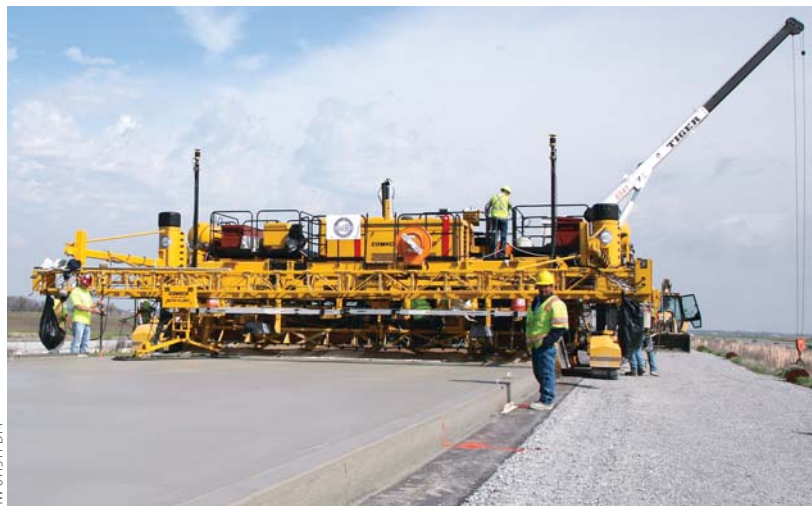
A GOMACO GHP-2800 with IDBI and two paver-mounted GSI® units slipforms Highway 67 with a Topcon 3D guidance system between Cash and Walnut Ridge, Arkansas.
