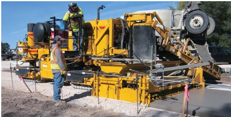
Ten foot (3 m) wide sidewalk is slipformed with the GOMACO GT-3200 sidewalk paver in a new development in St. Peter, Minnesota.
