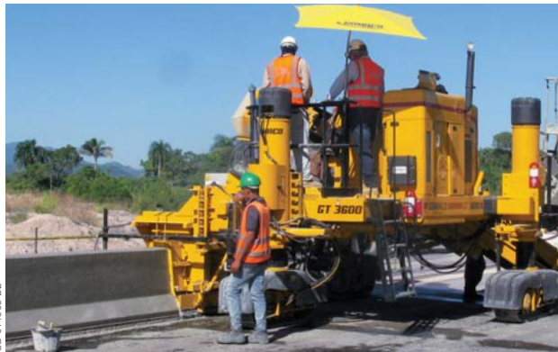
A GOMACO GT-3600 slipforms 810 millimeter (31.9 in) tall barrier wall on a project in Santo Domingo, Dominican Republic.
