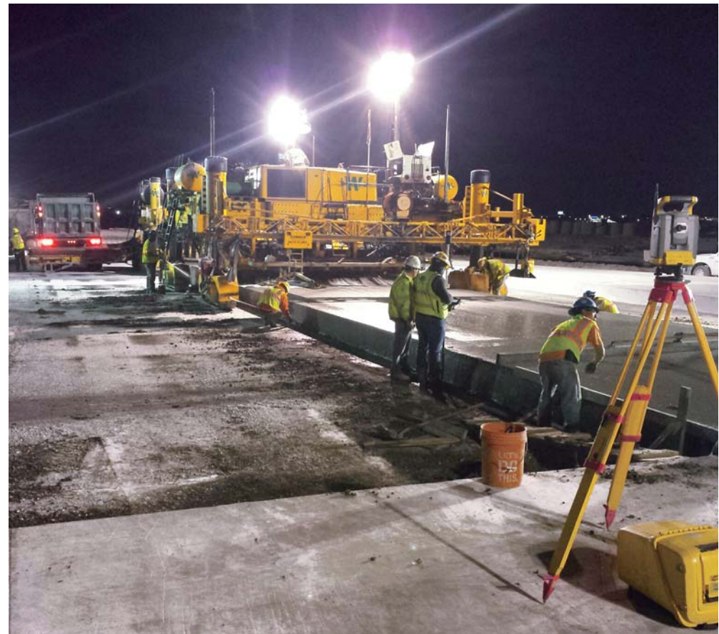
The GHP-2800, using a Leica Geosystems 3D guidance system, comes off the evening’s header and paves down ramps off the new 16.5 inch (419 mm) thick section of runway.
