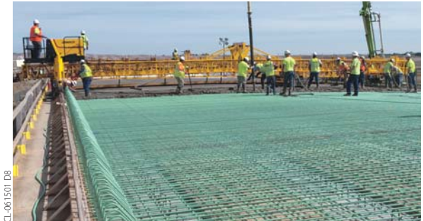
A GOMACO C-450 with a power transition adjuster (PTA) finishes a bridge deck 64 feet (19.5 m) wide in Dickinson, North Dakota.
