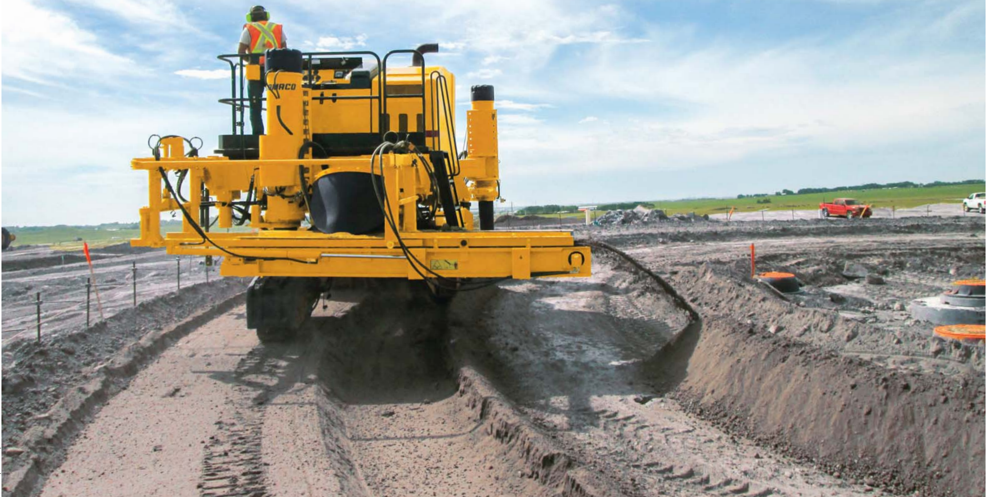
Marmot Concrete's three-track Commander III high-production trimmer features a powerful trimmer to cut through the clay-based and rocky soil found in Calgary, Alberta, Canada, for monolithic sidewalk profiles.
