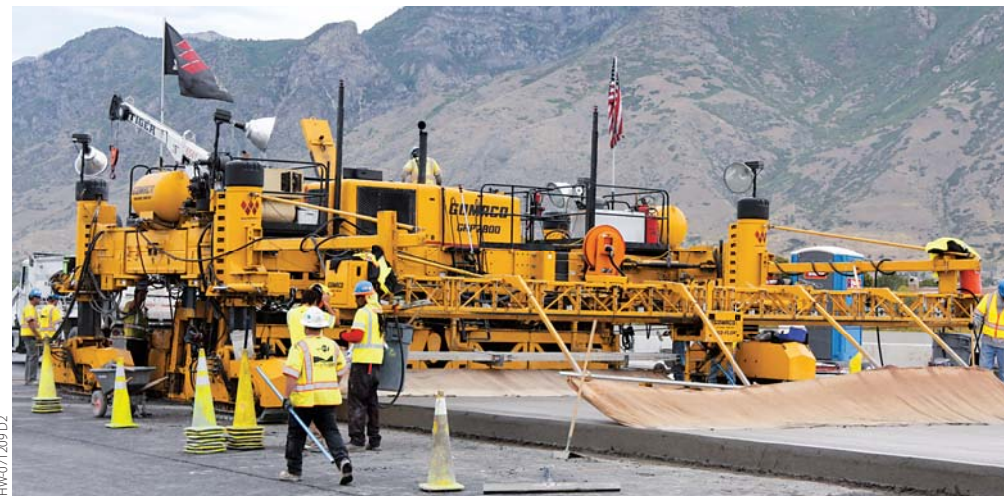
The concrete used to pave I-15 CORE project has a 40-year pavement design. It's a 6.5 sack mix design, 60 coarse, 40 fine, with a typical air entrainment of five to seven percent.
