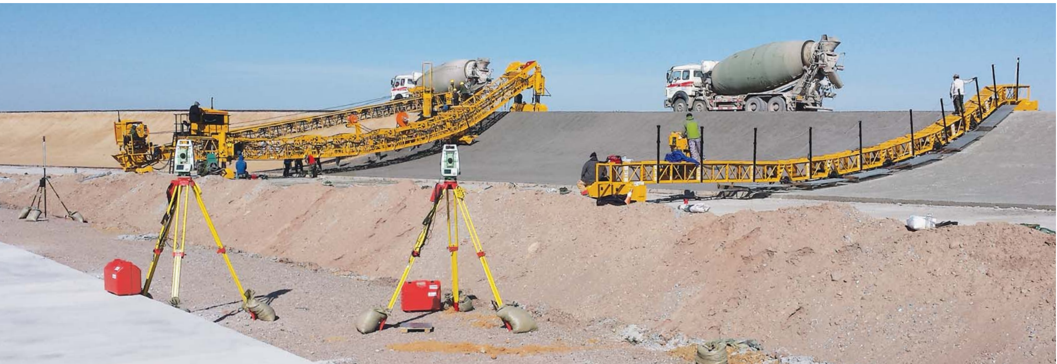
A GOMACO SL-750 cylinder finisher working on a Hyundai test track for their vehicles manufactured in China became the first finisher to be controlled with a 3D guidance system.
