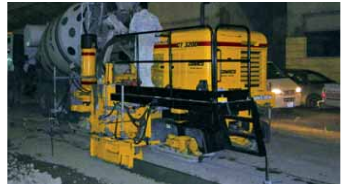
Al Musban slipforms stand-up curb with their new GT-3200 curb and gutter machine in Jeddah, Saudi Arabia.
