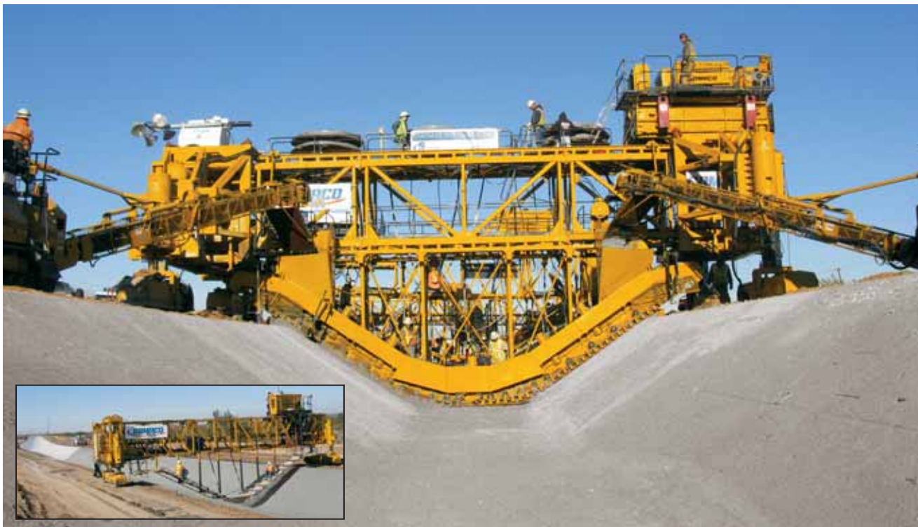
Coffman Specialties has reconfigured their All-American Canal paver into a full-prism paver and is slipforming a new canal project in Sacaton, Arizona. The water stop machine and work bridge are also being used on the canal. For more information on the All-American Canal project and equipment, please refer to GOMACO World, Volume 36, Number 2.
