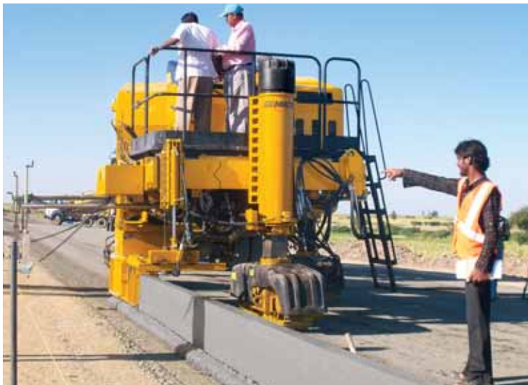
KNR Construction Ltd. uses their Commander III to slipform a stand-up curb along a new roadway in Bijapur, a city in the state of Karnataka, south of Mumbai, India.
