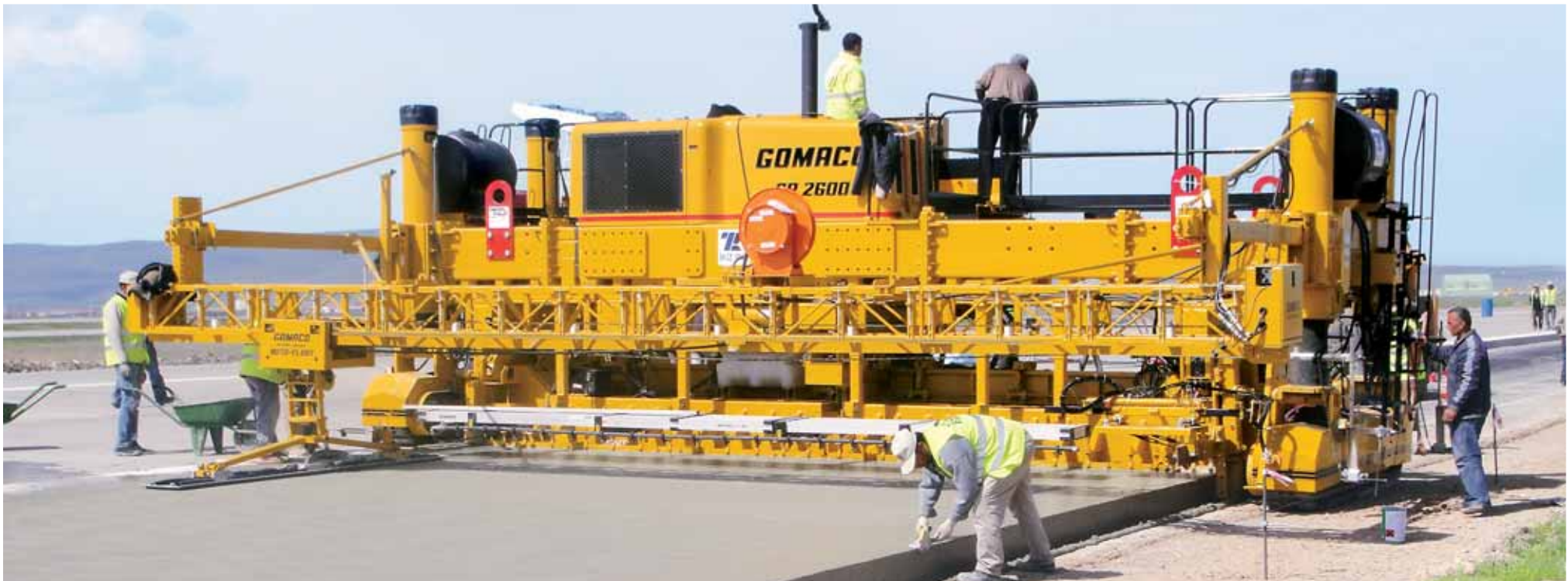
İkiz İnfaat Turizm Ve Tic. Ltd. Sti slipforms a scab-on lane with their four-track GP-2600 paver on an airport project near Ankara, Turkey.
