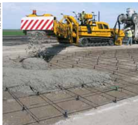
An RTP-500 rubber-tracked placer works in front of the GP-2600 paver.
