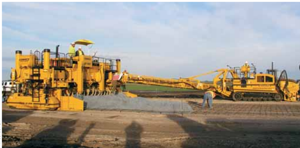
Opp Construction’s GOMACO RTP-500 rubber-tracked placer and two-track GP-2600 paver slipforms sugar beet pads.
