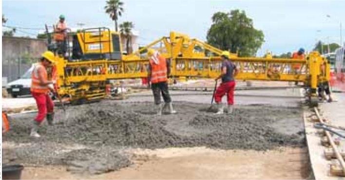
Stiler S.A. finishes a fill-in lane with an 80 to 120 millimeter (3.1 to 4.7 in) crown with their C-450 on a street project in Montevideo, Uruguay.
