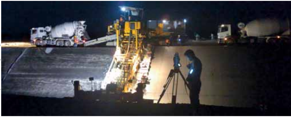
A surveyor checks the Total Station working across the canal from Eren's GOMACO four-track GP-2600 paver on the stringless project in Turkey.
