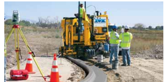
Marcon Concrete LLC slipforms stringless curb and gutter with their GOMACO GT-3600 in Meridian, Idaho.
