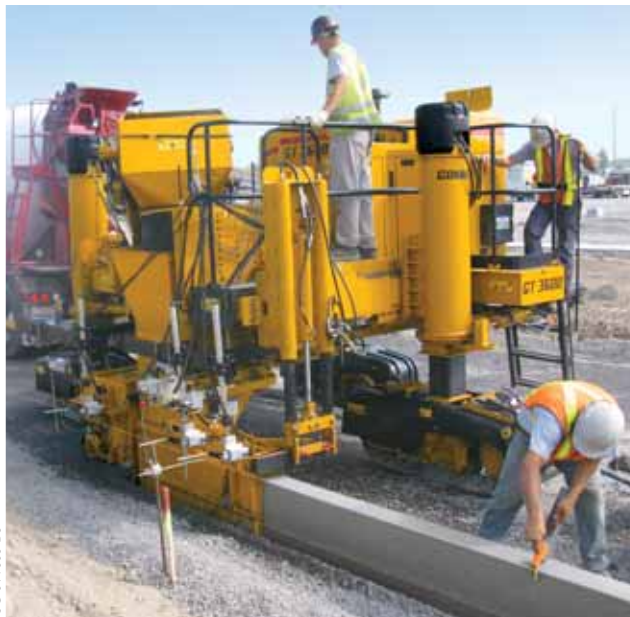
Coffrages Dunasso 2001 Inc. slipforms stand-up curb on a new development project in Cowansville, Quebec, Canada.
