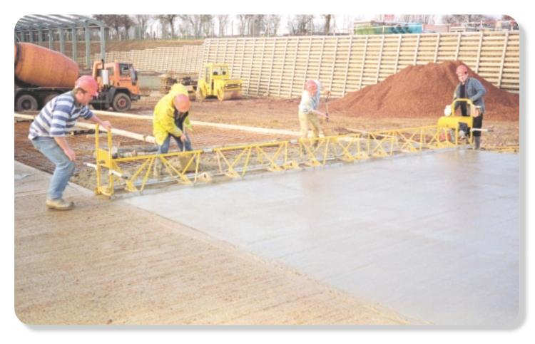
The GOMACO Hawkeye Screed is designed for finishing a variety of projects including driveways, streets, ramps, or any flat slab. The truss system on the MV-18 model is manufactured out of high tensile tubular steel in an 18 in. (457 mm) equilateral triangle. This screed is built to last in concrete job-site conditions.
