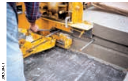
Female keyway with hydraulic side bar inserter (SBI) and vibration to the bar.
