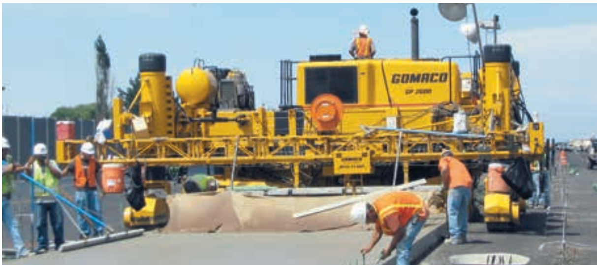
This versatile four-track GP-2600, equipped with the GOMACO Auto-Float®, slipforms mainline paving in Salt Lake City, Utah.
