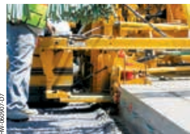
Trailing form with air-powered bar insertion.
