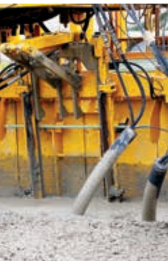
Male keyway with side bar inserter (SBI).
