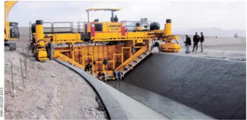
The sectional mold and front hopper feature different inserts to change the slope length and the depth. A sliding berm cap allows an extra 300 millimeters (11.8 in) of slope length adjustment on this canal in Turkey.
