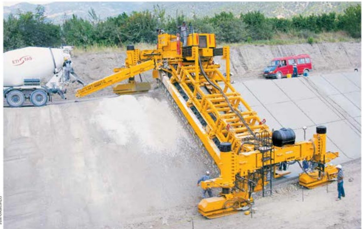
A paver with a front-mounted chain trimmer slipforms a new canal between Amasya and Tasova in northern Turkey in a three-pass process.
