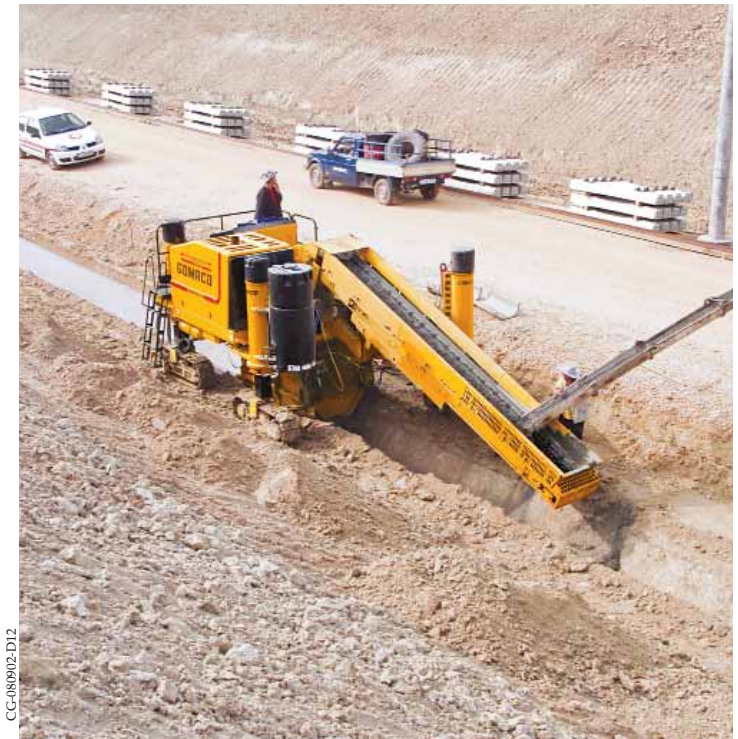
The Commander III uses the conveyor for fast delivery of concrete to the hopper, as it paves a waterway in Bulgaria.
