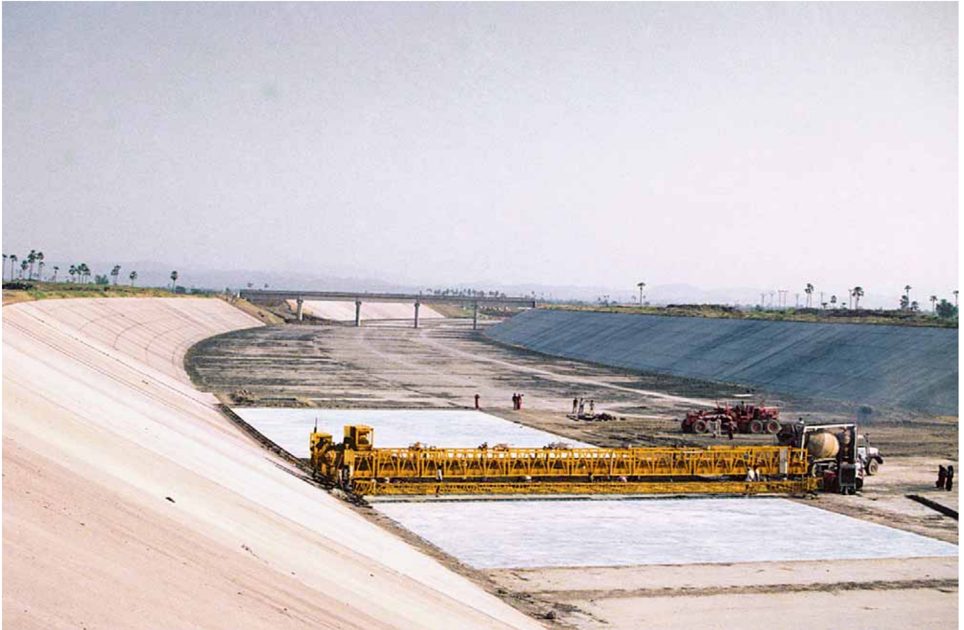
An overview of the Narmada Canal with the GOMACO 700 series as it paved the bottom portions of the canal.
