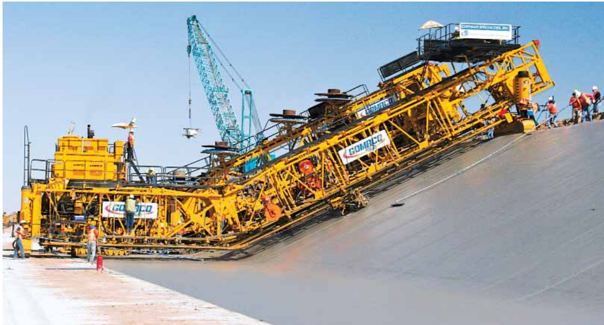
Portions of the All-American Canal were slipformed at 21.9 meters (72 ft) wide in a single pass.
