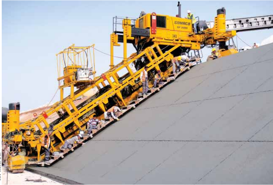
A work bridge has been attached to the back of the paver allowing the crew to finish the concrete around the joints being scored into the side of the slope.
