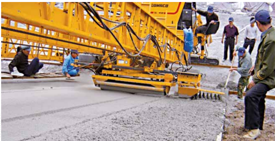
A vibrating finishing cylinder is available to enhance the finish of the concrete on a slope.
