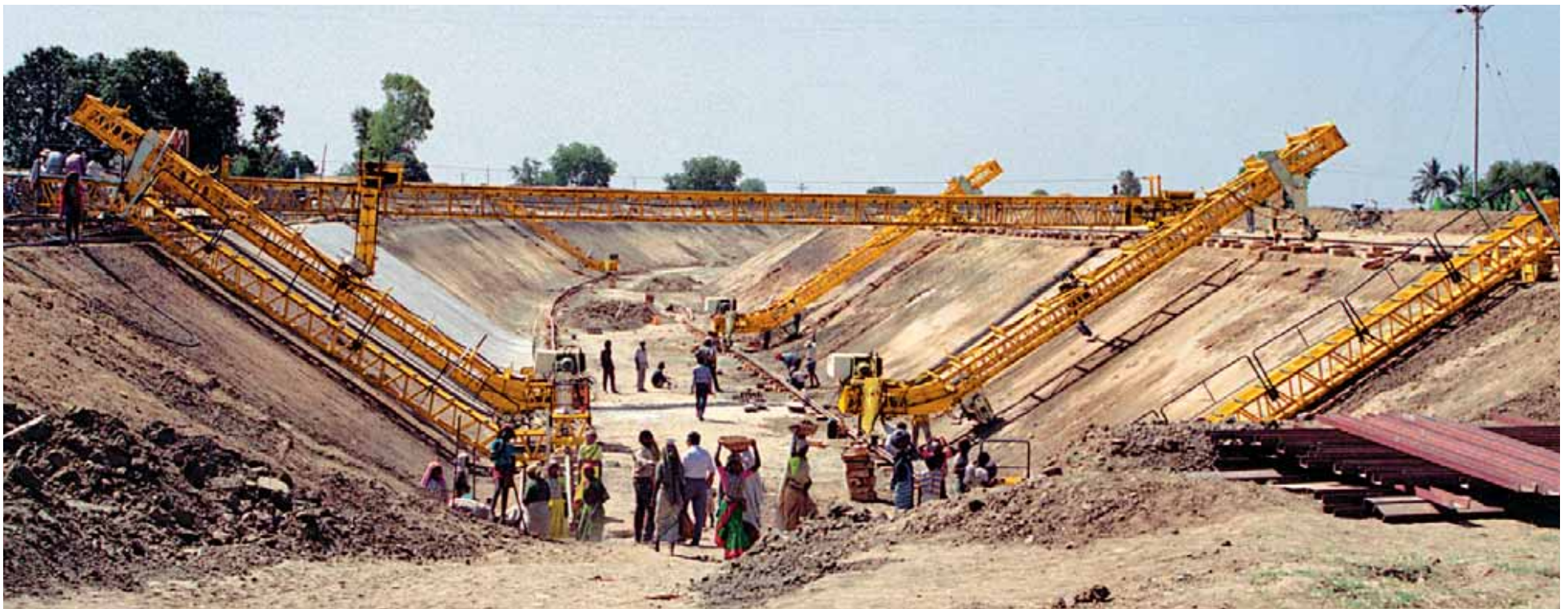
An overview of the canal with the GOMACO slope trimmers and finishers, RC Conveyors, and work bridges.
