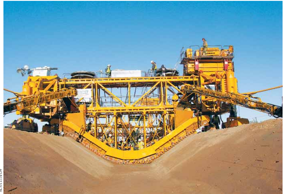
The All-American Canal paver was reconfigured into a full-prism paver and is slipforming a new canal project in the southwestern United States.
