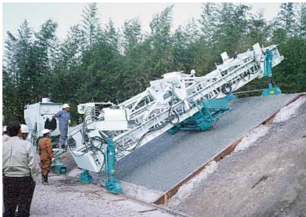
An SL-450 in Japan tests a patented concrete mix, called Permeacon, for ecologically friendly flood control slopes.
