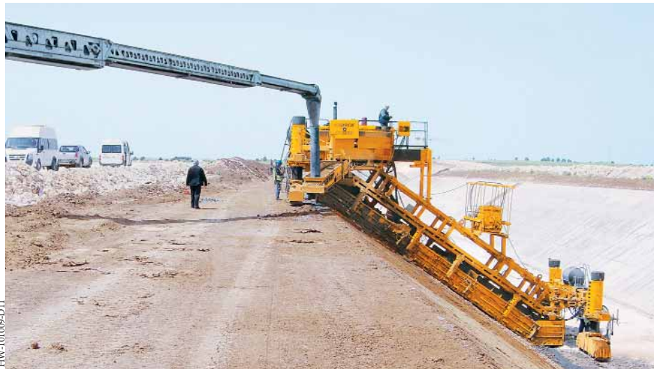
Concrete is metered down the slope by an auger. A system of baffles controls the concrete and keeps it from sliding down to the bottom of the canal.
