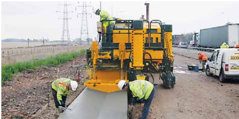
A Commander III paves a drainage channel in England.
