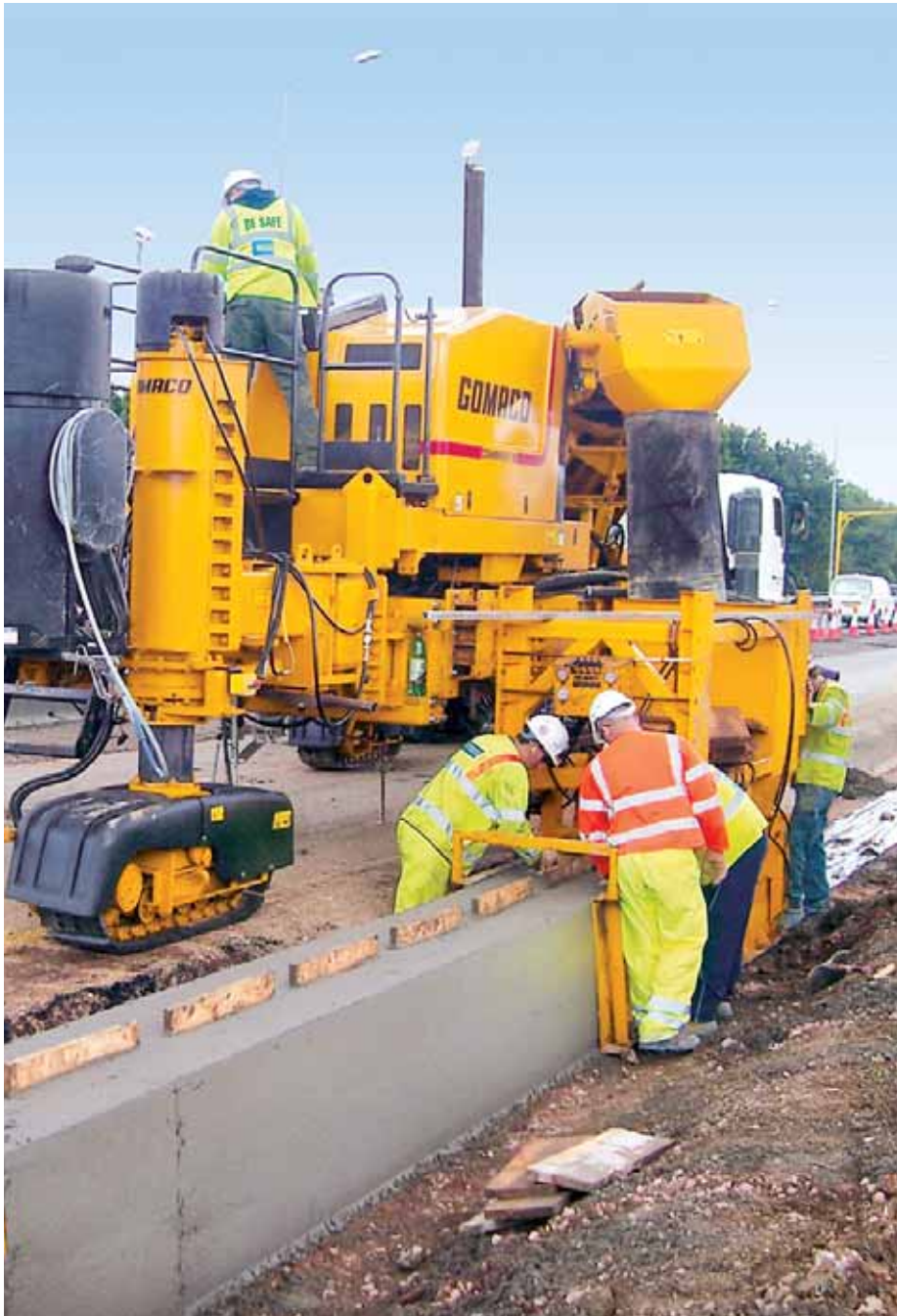
The Commander III three-track slipforms a slotted drain in England.
