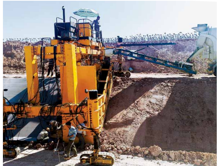
A Commander III four-track is equipped with a half-width mold and is paving an eight meter (26.25 ft) slope with a 500 millimeter (19.7 in) base and top cap, on a 1.5:1 slope in Turkey.
