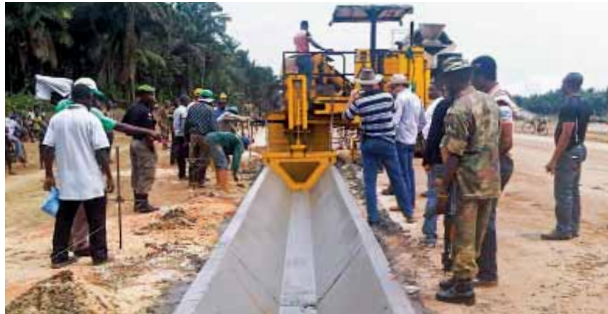
A GT-3600 slipforms a water drainage channel.
