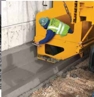
A GT-360 slipforms a drainage channel for water to run off the bridge in the United States. The stringline holders have been mounted to the wall, so the GT-360 will follow the wall profile.
