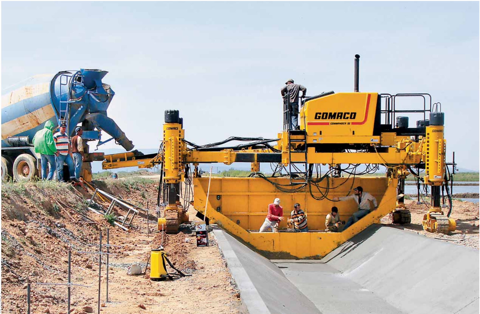
The trapezoidal canal mold has the ability to pave a deeper and wider canal by adjusting the berm caps.
