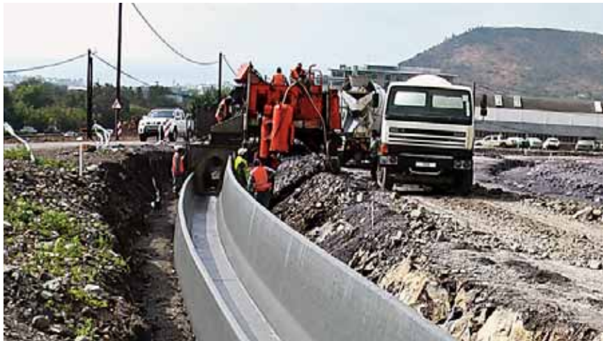
GOMACO's C-750 on a pivot-point finishes the concrete base for water waste treatment tanks in the Netherlands.
