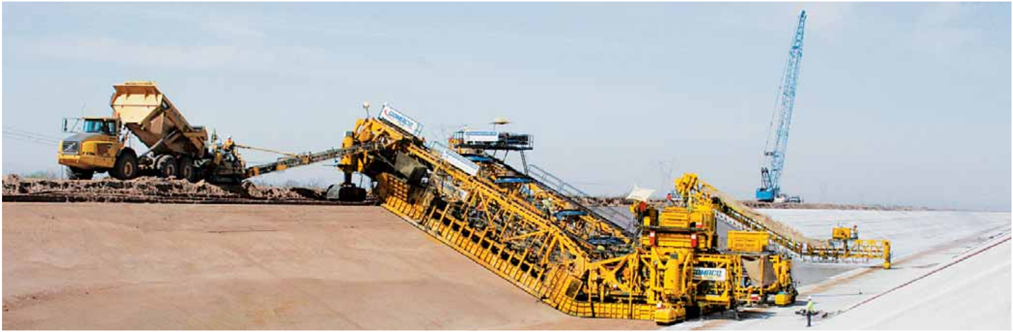
A GOMACO RTP-500 placer fed all of the concrete to the All-American Canal paver for this project.
