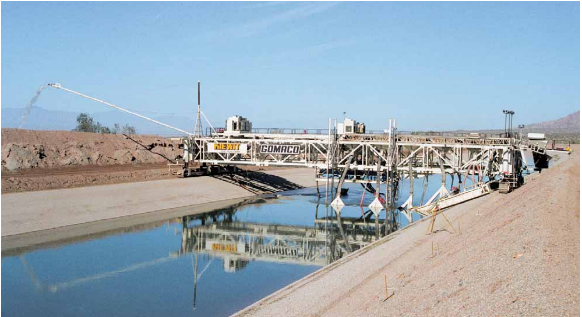
The trimming of the slopes and bottom of the Coachella Canal was required to be done underwater, while doing one slope and half of the bottom with each pass. The trimming and slipforming of the canal were done in two passes to avoid the interruption of the water flow. GOMACO equipment could have slipformed this project in a single pass if the water was not in the canal.
