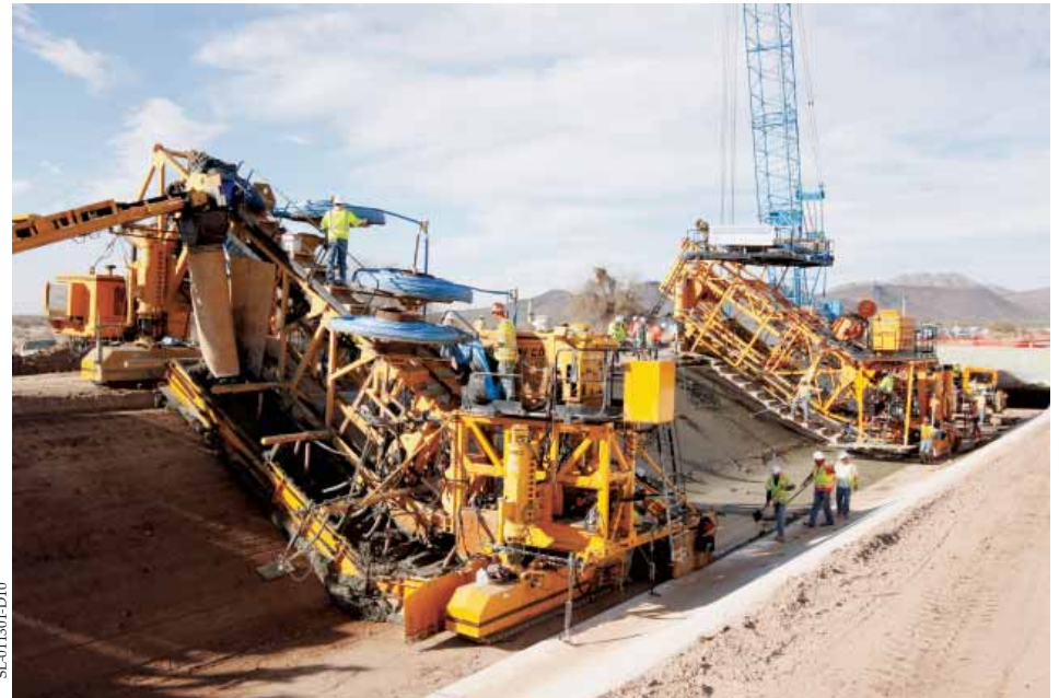
The reconfigured All-American Canal work bridge doubles as a paver on a canal in the southwestern parts of the United States. The paving train consists of the canal work bridge (as a paver), water stop insertion machine, and a T/C-600 texture/cure machine.
