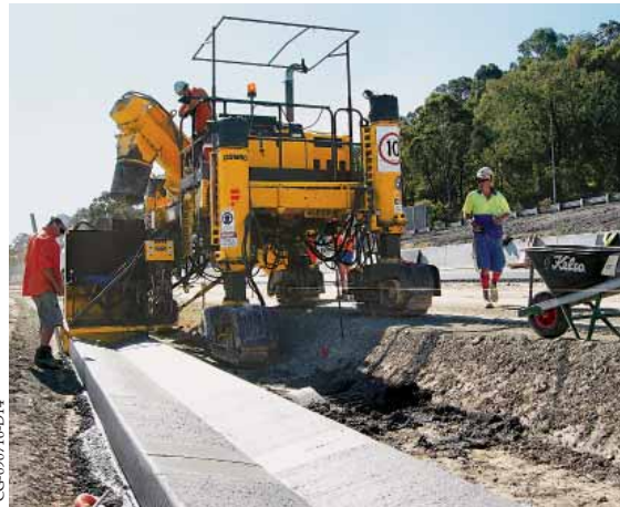
A Commander III uses the versatility of the track placement to slipform a drainage canal in Australia.
