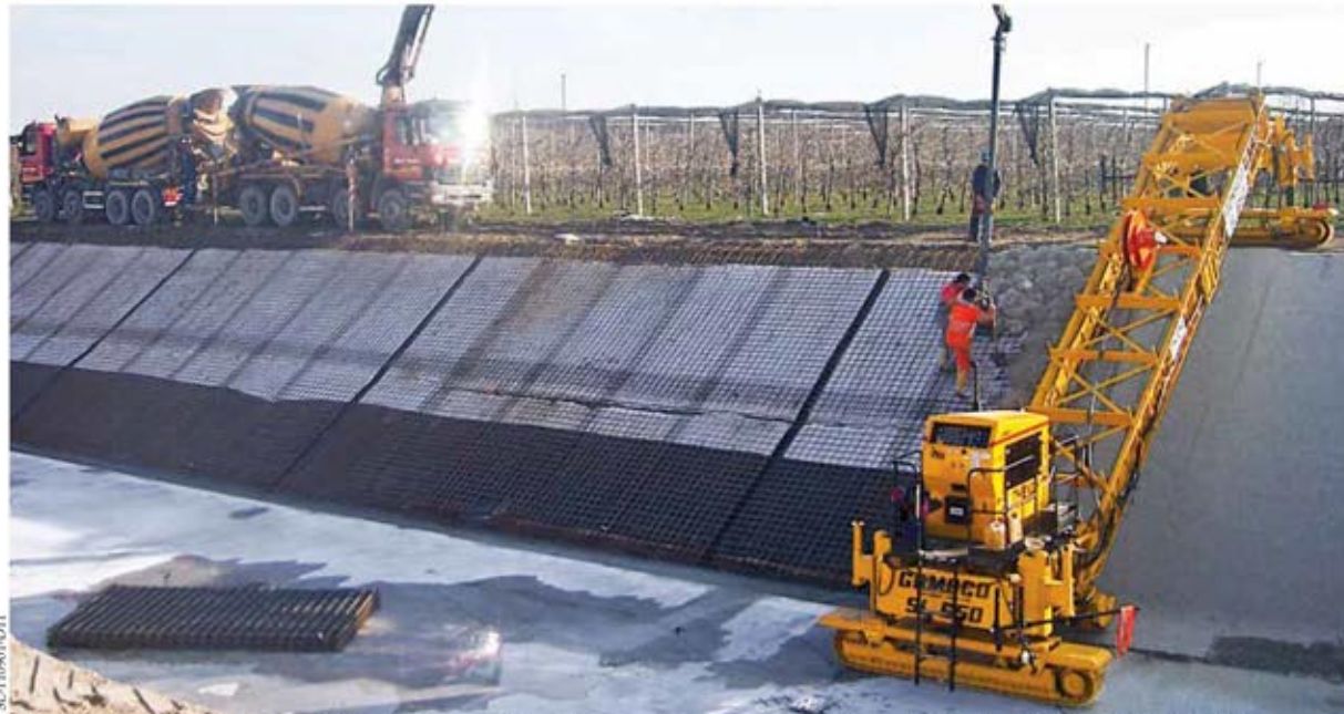
The SL-650-S has a possible frame width of up to 17 meters (56 ft) and the finishing width is 1.5 meters (5 ft) less than the frame width.
