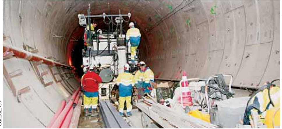
The Commander III three-track paves a slotted drain through the Perthus Tunnel between France and Spain.
