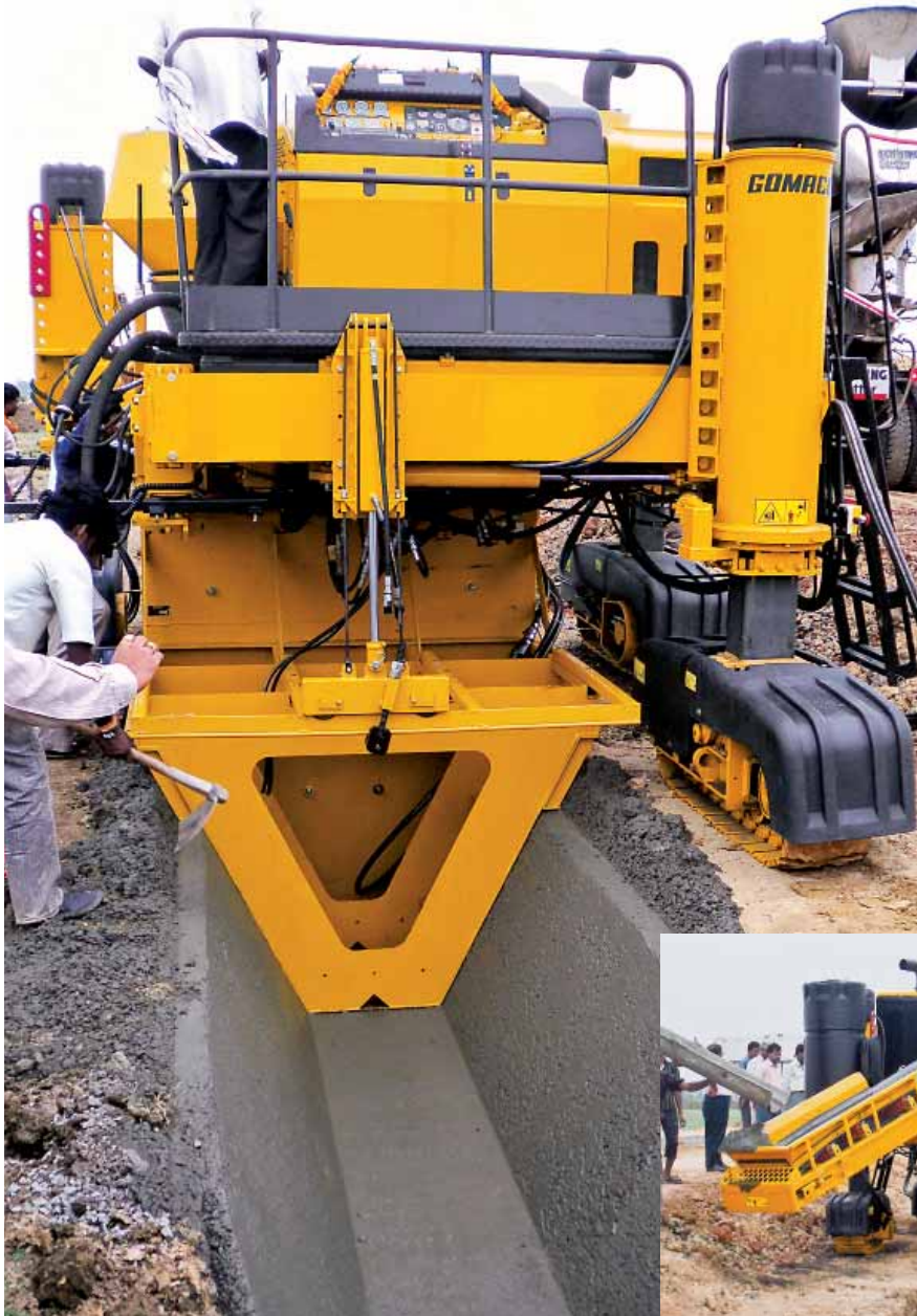
The Commander III three-track slipforms a V-ditch in India.
