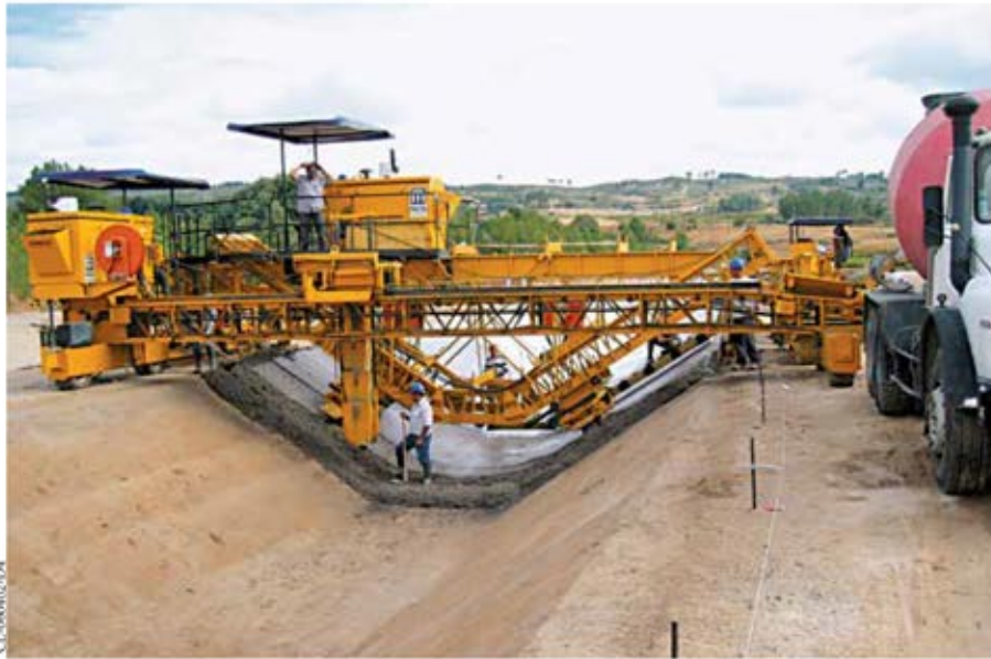
The CP-650 paves a canal with a trapezoidal profile in one pass in Portugal.
