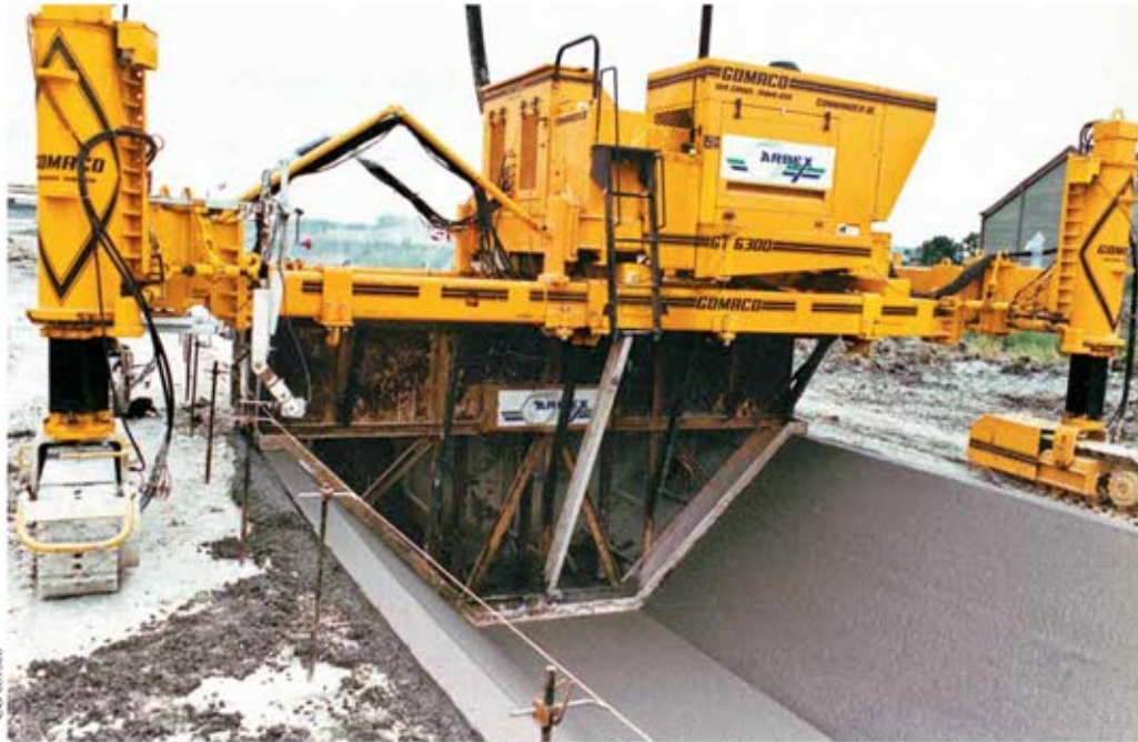
The GOMACO paver is referencing stringline from inside the track line for the trapezoidal canal.
