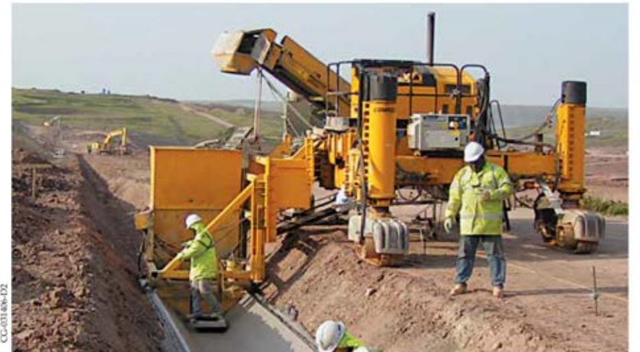
This four-track GOMACO machine slipforms a water drainage channel below grade, around natural liquid gas storage tanks in South Wales.
