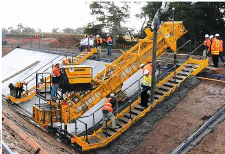
This is a two-pass paving process for a canal in Australia.
