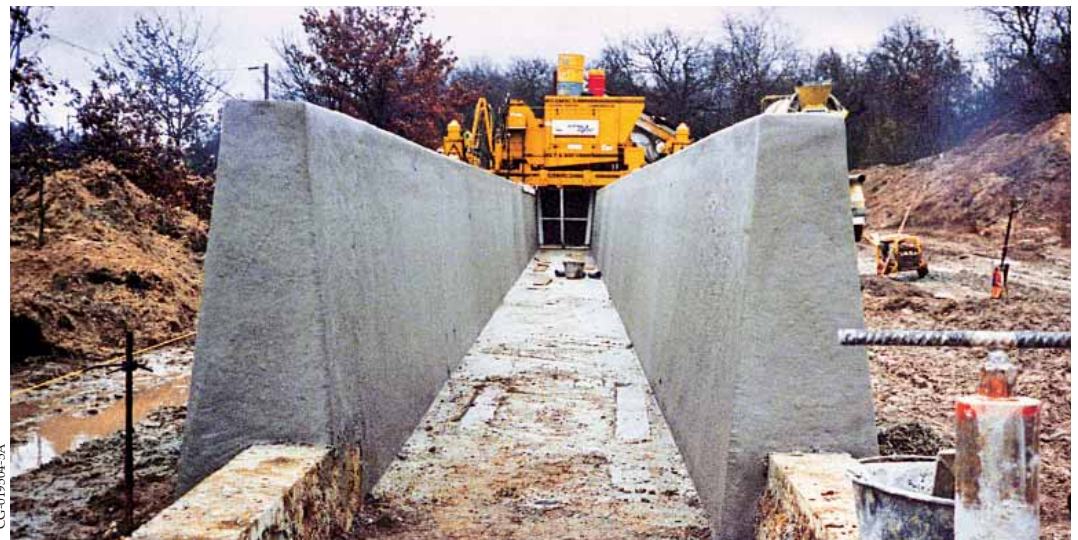
This four-track GOMACO paver slipforms a U-Channel in France.
