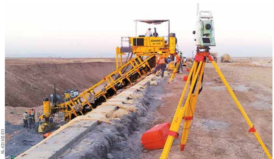
This paver is using 3D machine guidance for slipforming the concrete canal lining.
