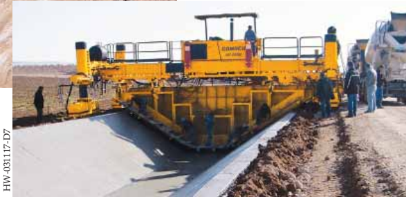
A chain trimmer on the front of the paver fine trims the grade as the canal is simultaneously poured allowing canal paving efficiency.
