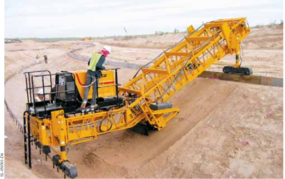
The trimmer attachment is used to trim approximately 76 millimeters (3 in) of sandy soil in New Mexico, U.S.A., before paving the canal.
