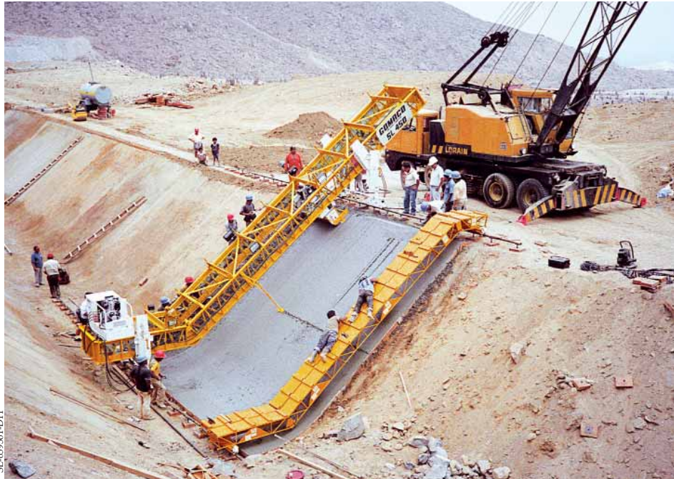
The GOMACO finisher is followed by a double work bridge and the center joint is cut on-the-go on this canal in Peru.
