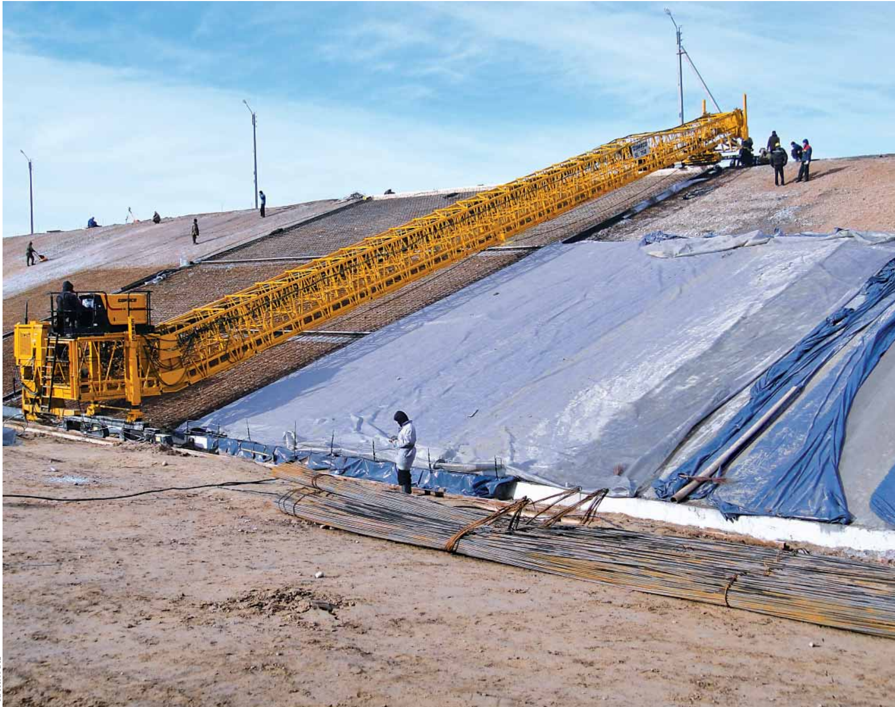
The SL-750 with a 45.1 meter (148 ft) frame is ready to finish the concrete lining on a reservoir in Kazakhstan.
