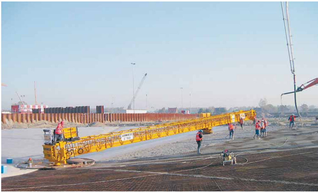
GOMACO's C-750 on a pivot-point finishes the concrete base for water waste treatment tanks in the Netherlands.
