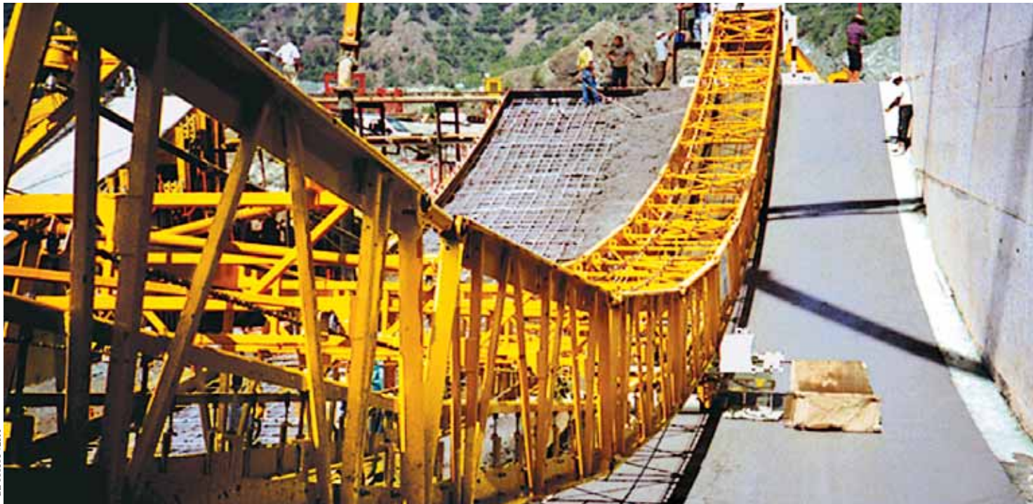
This GOMACO machine paves a spillway on the San Roque Dam in San Roque, Philippines
