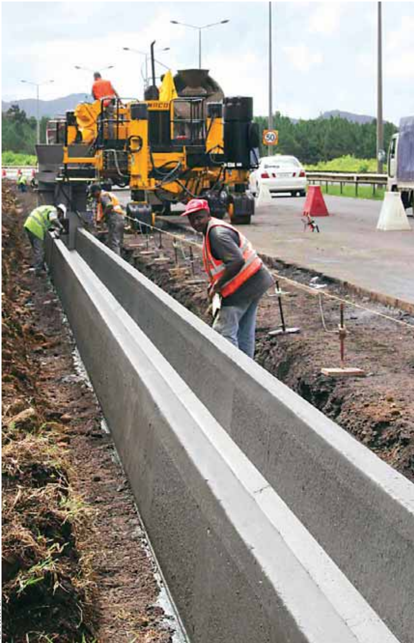
The GOMACO 4400 slipforms a left-side pour U-Channel 508 millimeters (20 in) tall, below grade, and next to an existing road in Mauritius.
