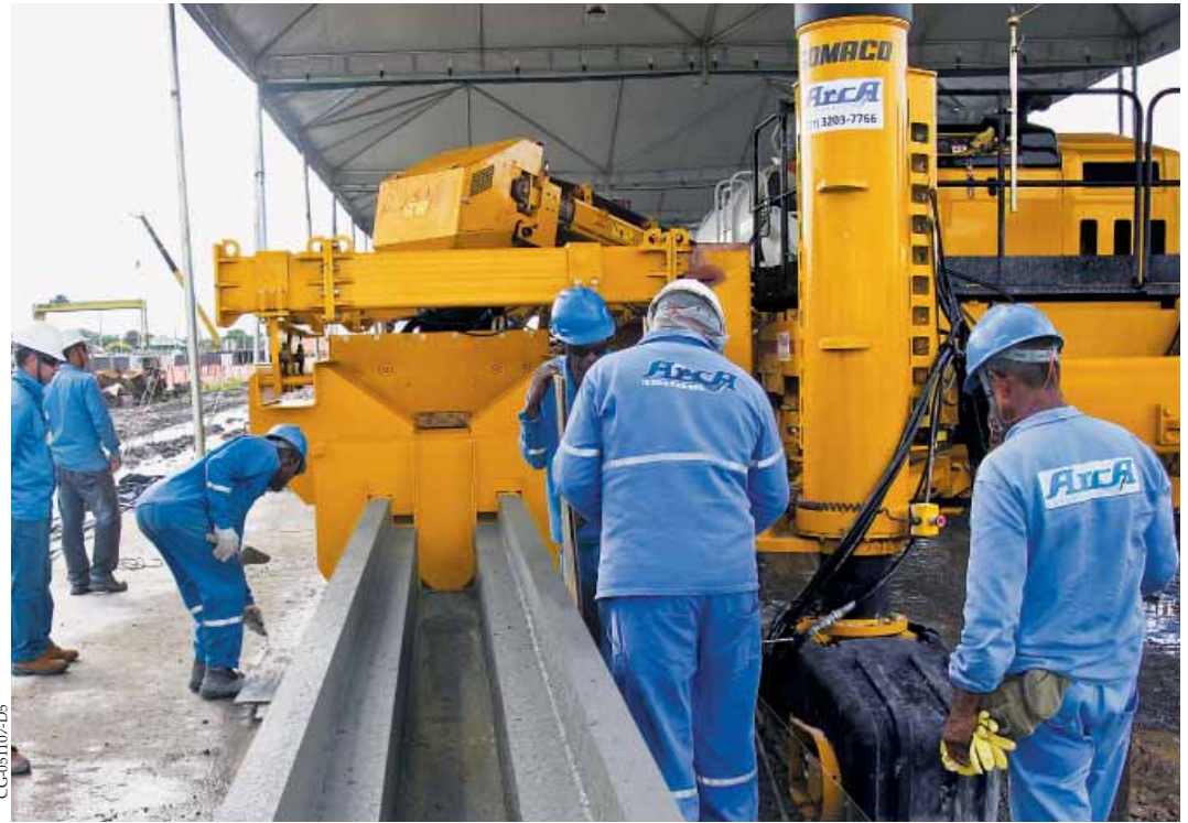
The Commander III with a sidemounted mold paves a U-Channel in Brazil.
