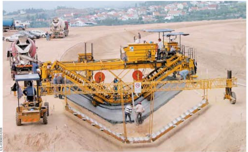
The CP-650 finishes a canal that has a slope of 1.5:1 with a bottom width of two meters (6.6 ft).
