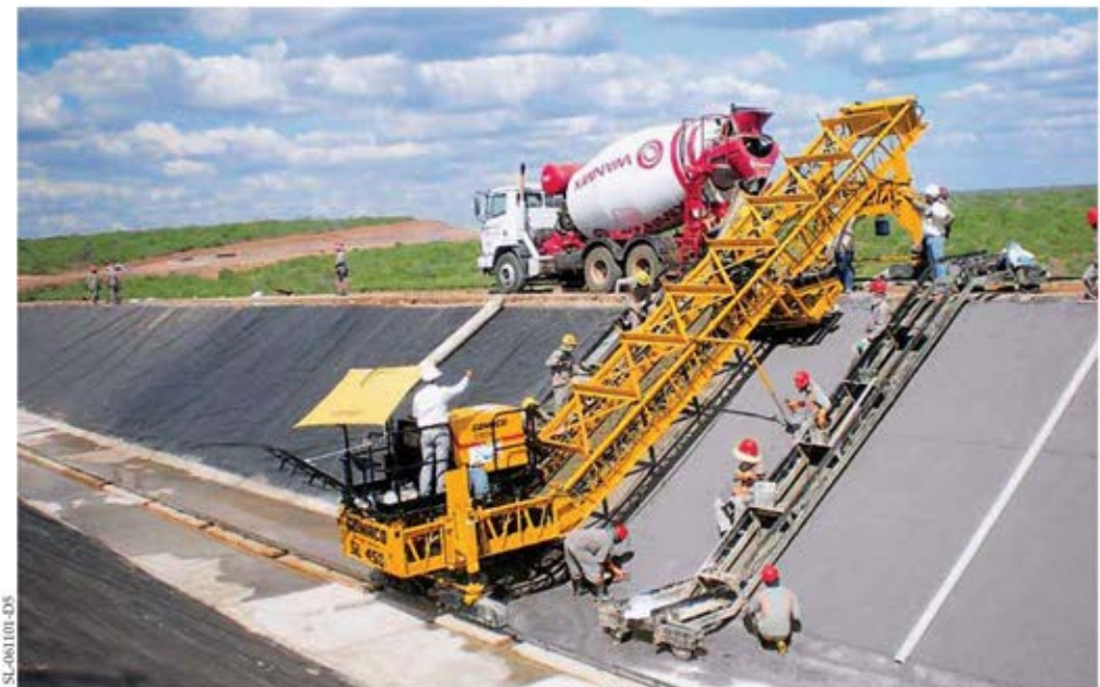
This is a three-pass paving process on a canal in Brazil.
