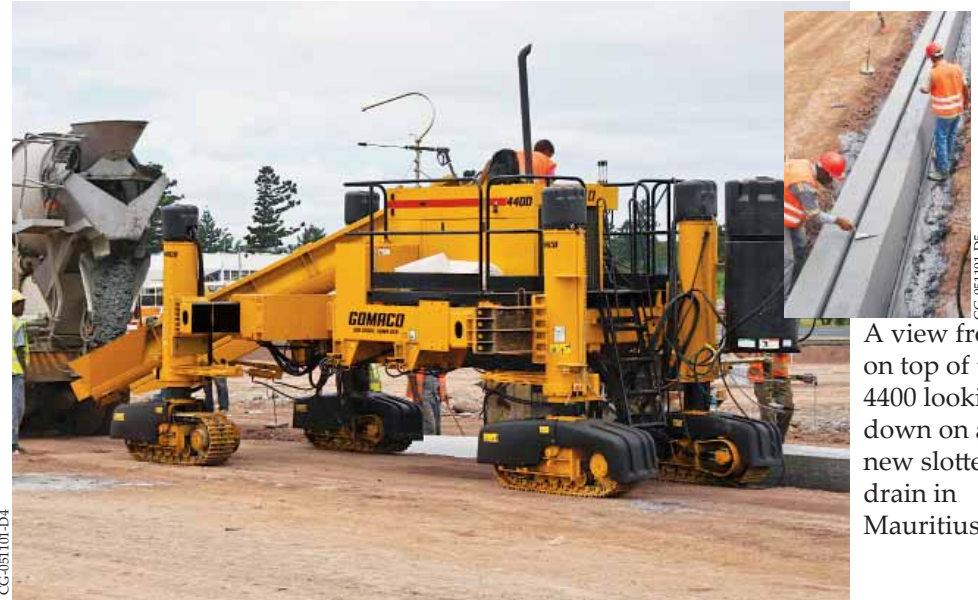
A four-track 4400 paves a 500 millimeter (19.7 in) slotted drain in Mauritius.
