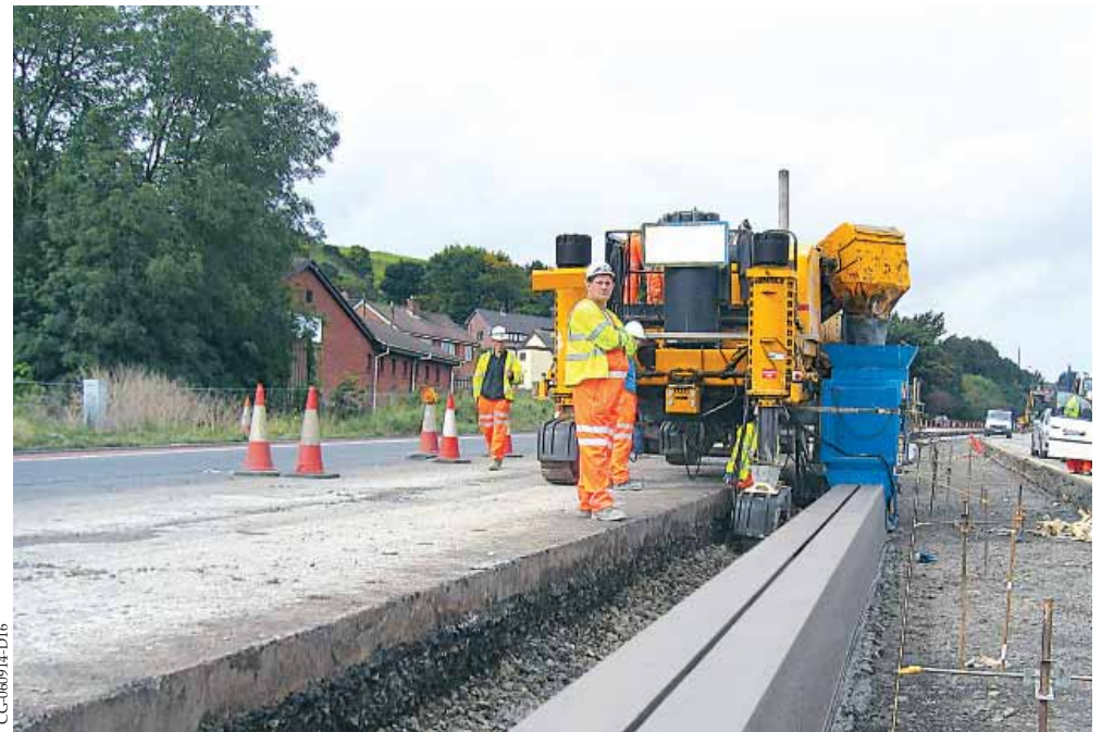
The Commander III paves a slotted drain and drainage channel in Northern Ireland.
