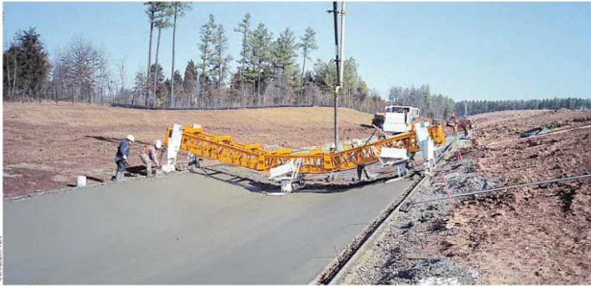
The SL-450 paves a drainage channel next to an airport.
