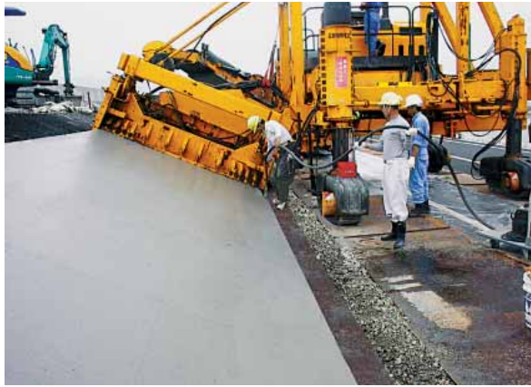
This slipformed three meter (9.8 ft) wide slab at a 1:2.4 slope is part of a breakwater system in Japan.
