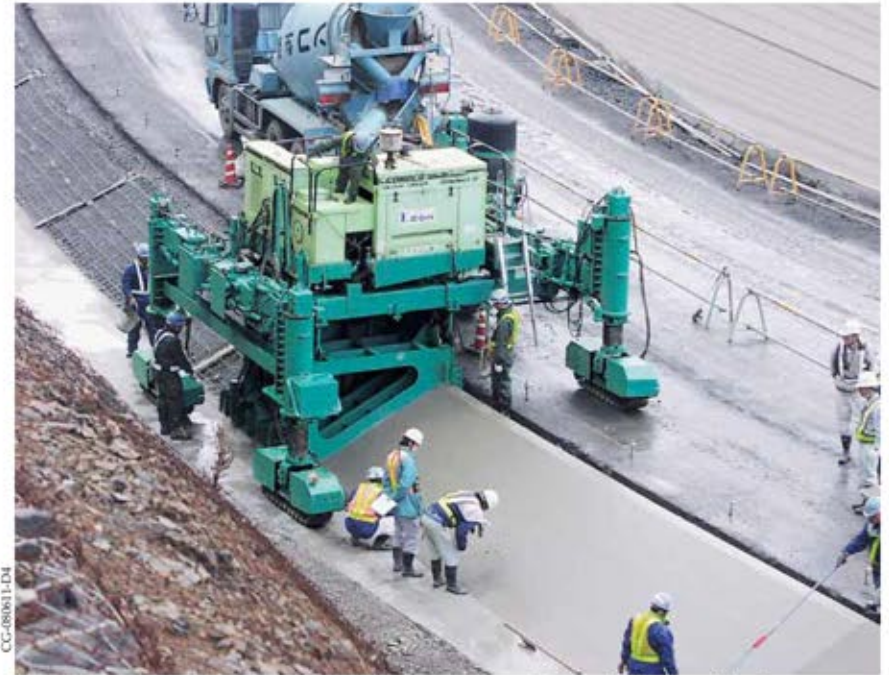
This four meter (13 ft) wide, 200 millimeter (8 in) thick canal in Japan was slipformed in two paving passes.
