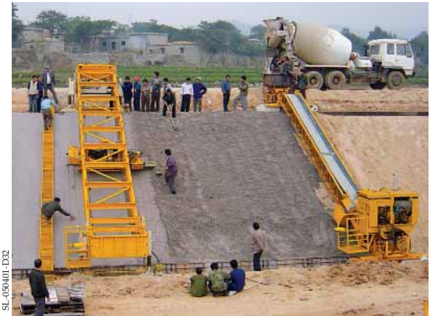
An SL-450 lines a canal project in China with concrete.
