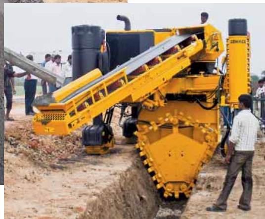
The Commander III three-track uses the simultaneous trim/pour method to slipform the V-ditch.
