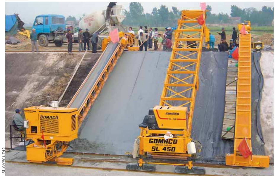
An RC Conveyor places concrete the width of the pour and a Spanit® work bridge follows the finisher.
