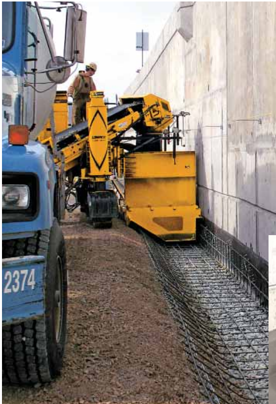
A GT-360 slipforms a drainage channel for water to run off the bridge in the United States. The stringline holders have been mounted to the wall, so the GT-360 will follow the wall profile.
