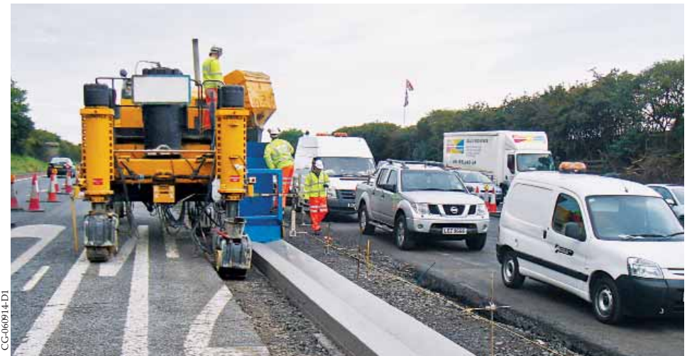
A Commander III slipforms a drainage channel in Northern Ireland.
