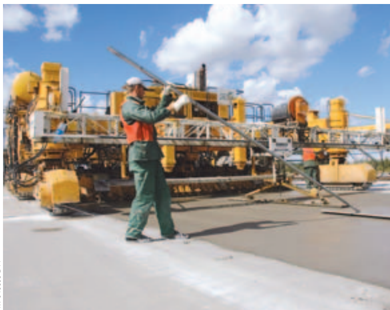
A four-track GHP-2800 slipformed the new runway in 24.6 feet (7.5 m) wide paving passes.
