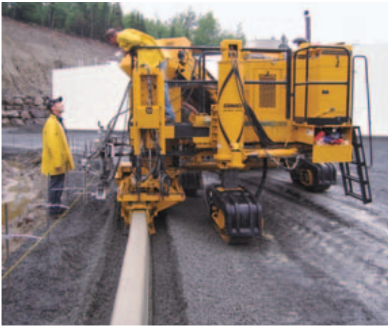
Maska Paving slipforms 16 inch (406 mm) tall ribbon curb with their GT-3600 in Montreal, Quebec, Canada.
