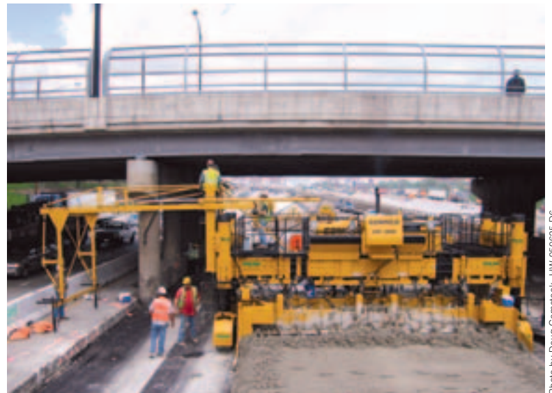
The gantry system is hydraulically extended, and normal paving continues once the paver is clear of the bridge piers.
