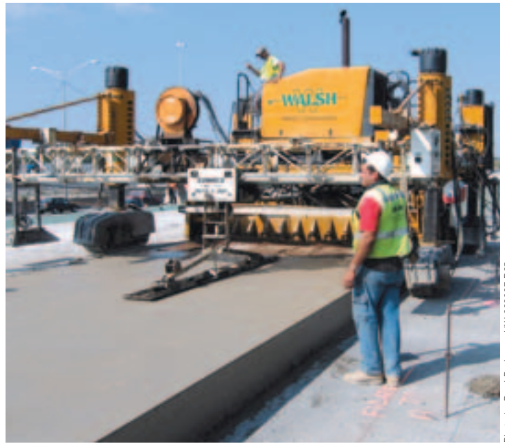
A Commander III four-track with Auto-Float® attachment slipforms exterior shoulders on the Dan Ryan Expressway.
