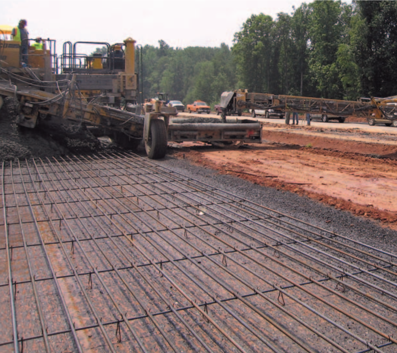
An RTP-500 transfers concrete across the median onto the belt of the PS-2600 in some areas of the project because shoulder conditions were
