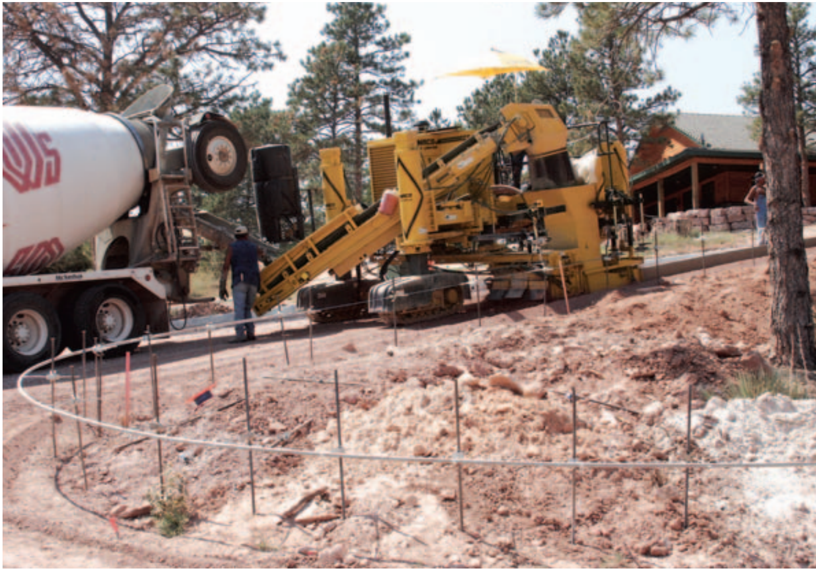
The GT-3600's auto-transition system automatically adjusts the curb flow line from a catch to a spill during the length of the radius.
