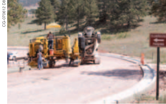
Tru-Form's GT-3600 at work on the Southern Hills Golf course in Hot Springs, South Dakota.
