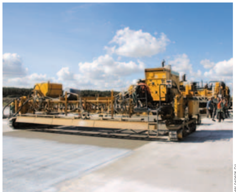
A GOMACO T/C-600 texture/cure machine followed the paver applying a tine finish and curing compound.
