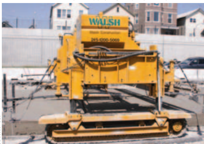
A T/C-600 with the new skewed tining option tines the slab on a 6:1 skew before applying a spray cure finish.
