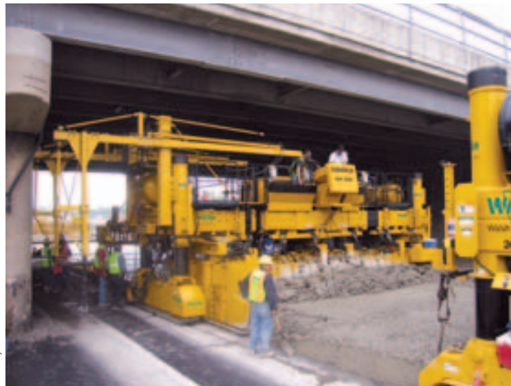
A front view of the GHP-2800 as it paves under the bridge structure with the paver locked in on cross slope.
