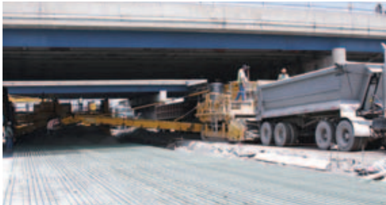
The 9500, with its long belt, places concrete in front of the PS-2600 underneath a bridge structure on the Expressway.
