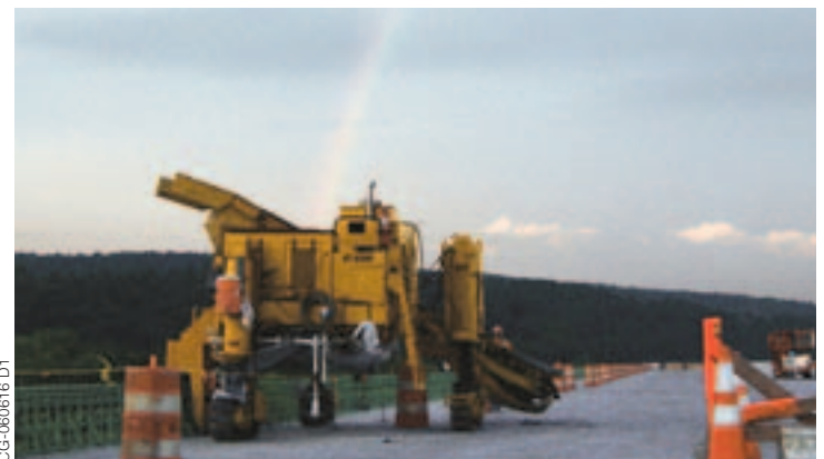
David Leith at Syrstone Inc. took this photo of his company's GT-6300 ready to slipform parapet early one morning on the Pennsylvania Susquehanna River Bridge project. "We know where our pot of gold is," Leith said.
