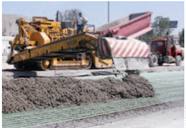
The 9500's 80 degrees of hydraulic side swing gives Walsh maximum placing capabilities on the project.
