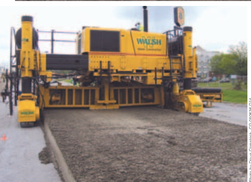
A PS-2600 placer/spreader places concrete over continuous steel reinforcing on one of the project's single lane exit ramps.
