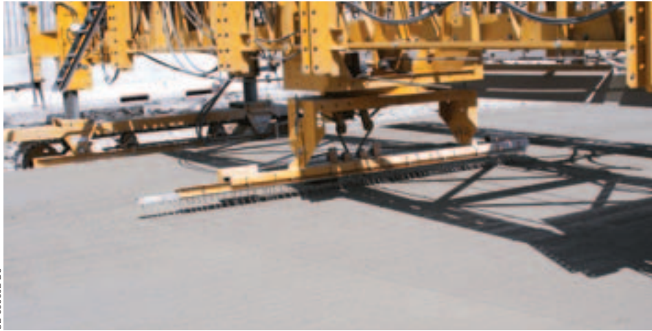
The T/C-600's new skewed tining option allows Walsh to finish on a 6:1 skew without adding any additional pieces to the framework.
