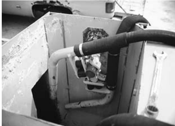
Photo #1 – Placing your vibrators
