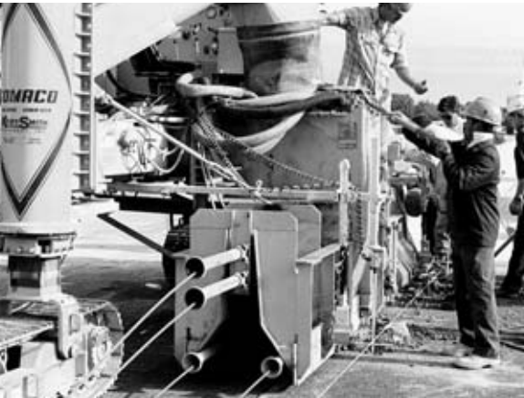
Photo #5 – Continuous reinforcing steel
