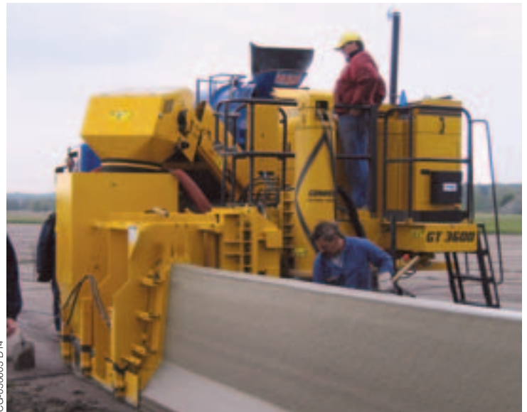
Doprastav A.S. slipforms two 472 foot (144 m) long walls with their GT-3600 on a project in Prague, Czech Republic.
