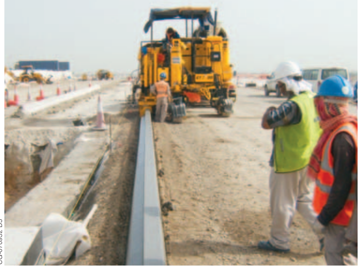
Orascom slipforms a unique profile of curb and gutter on a project in Abu Dhabi, United Arab Emirates.
