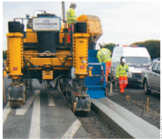
The first step of the project required slipforming a drainage system, with either a v-channel or slot drain.
