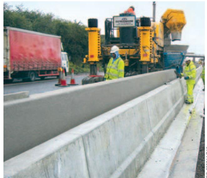
Extrudakerb poured off the right-side with their four-track Commander III on all of the different profiles on the project.
