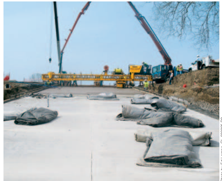
The ramps were finished in two pours, each 55 feet (16.8 m) long and 40 feet (12.2 m) wide.
