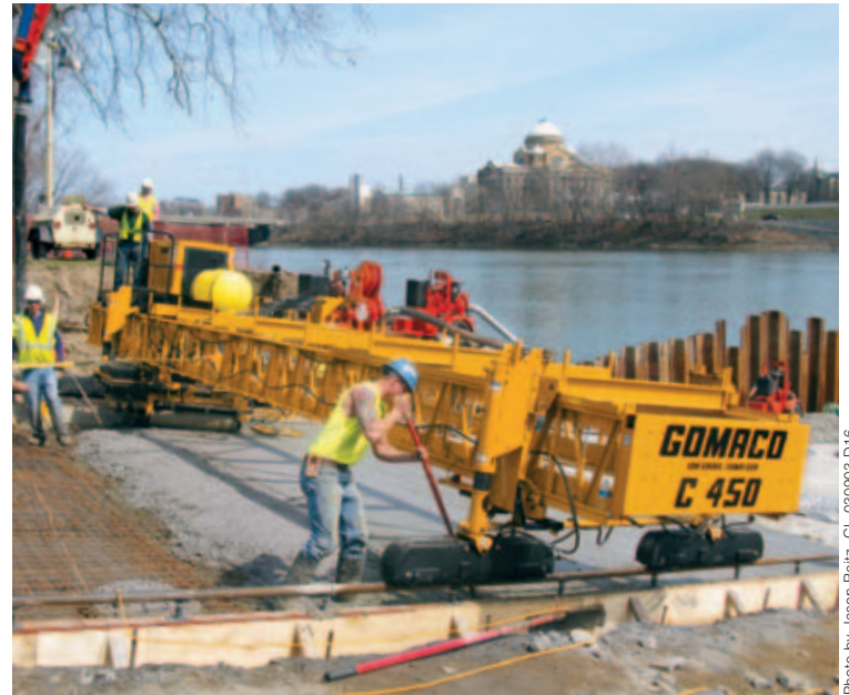
Kruger’s C-450 has an all-wheel drive system with cupped wheels to help deal with the ramp’s steep 10 percent slope.
