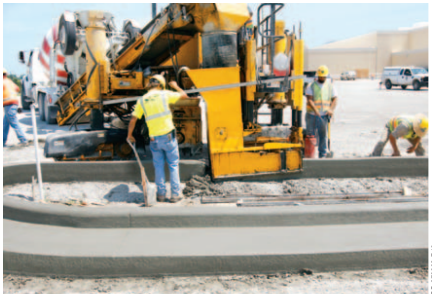
The operator sideshifts the trimmerhead out of the way so the mold can slipform up to the point where the island’s curb and gutter was started.
