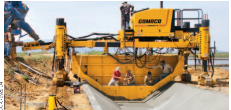
Aktek slipforms a new water canal, with their four-track Commander III, to irrigate rice fields in Kesan, Turkey.
