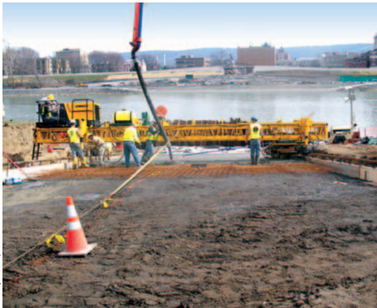
The C-450 was attached to a winch and a dozer as a safety precaution. The extra precaution was not needed on the pours.
