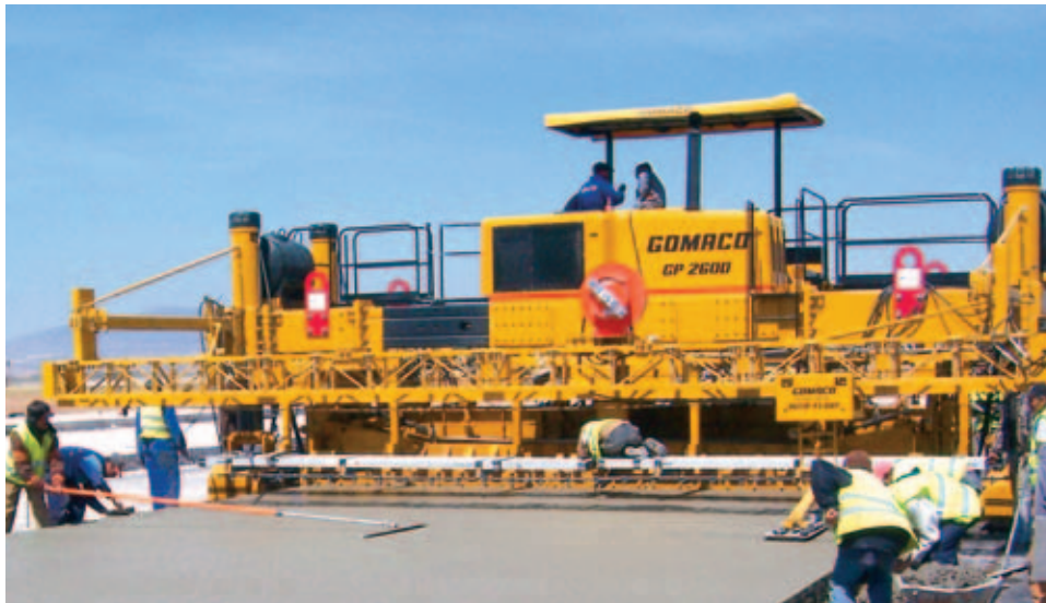
STAIP Ltd. slipforms an airport project with their two-track GP-2600 paver in Oujda, Morocco. The paving passes were 7.5 meters (24.6 ft) wide and 330 millimeters (13 in) thick.
