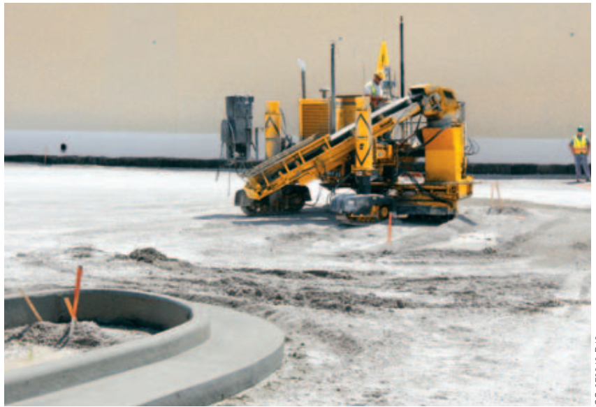
The operator chooses the island he wants to slipform next on a map in the stringless computer. Stringline no longer dictates the project phasing.
