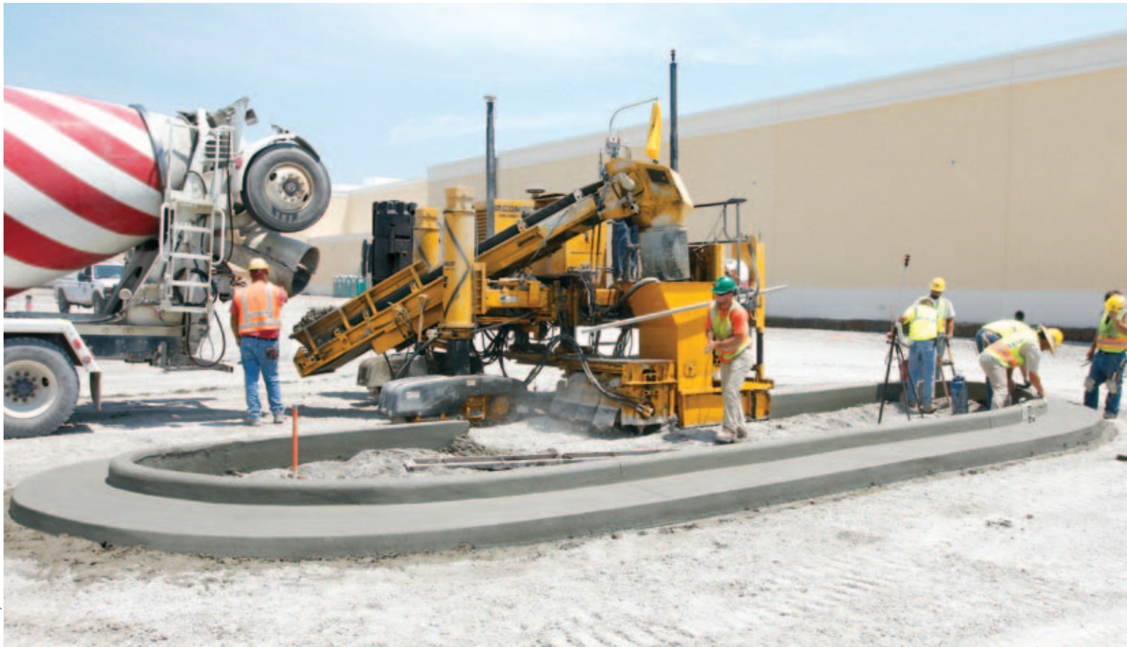
Fred Weber slipforms parking lot radii with a stringless system on their GOMACO GT-3600 on a project in St. Louis, Missouri.
