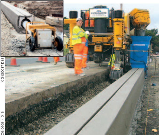
The slot drain had a diameter of 300 millimeters (11.8 in) and was slipformed over a plastic, inflated tube.
