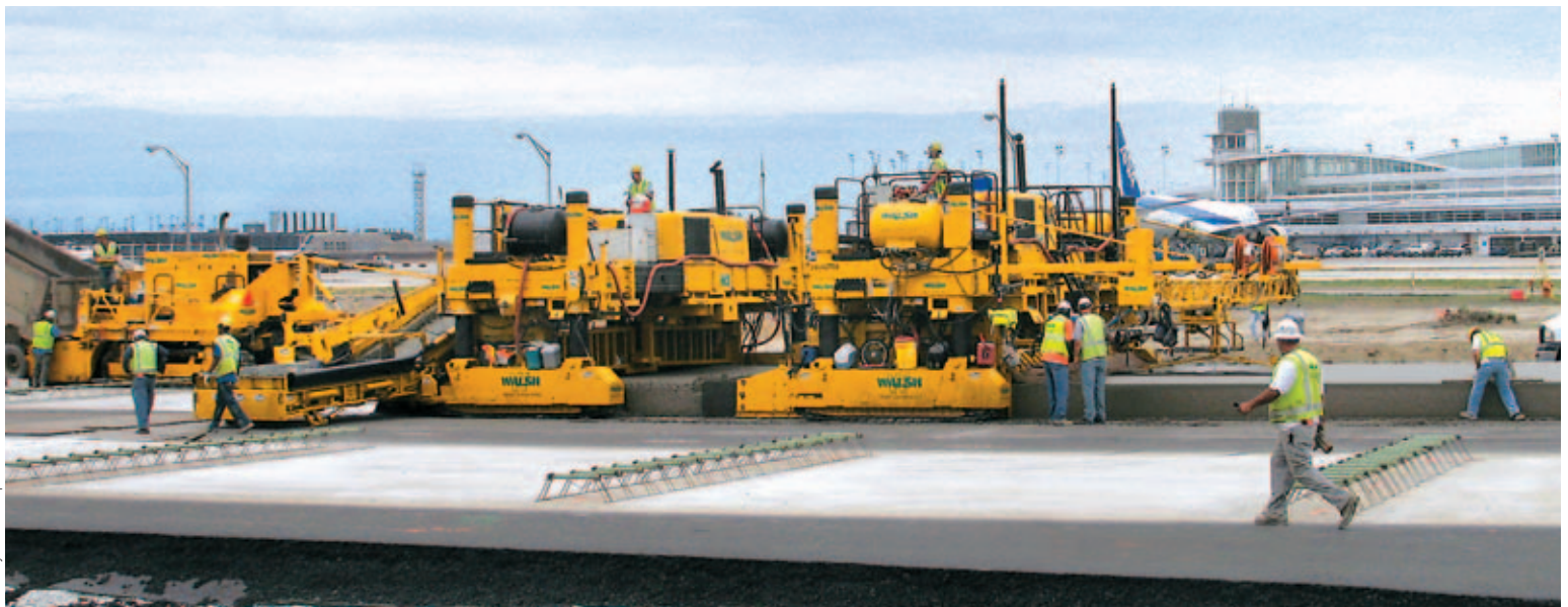
Photo by Tom Phillips HW-080907 D5 Walsh slipformed 7728 cubic yards (5908 m 3 ) of concrete in a 12.5-hour day at the O'Hare International Airport in Chicago.
