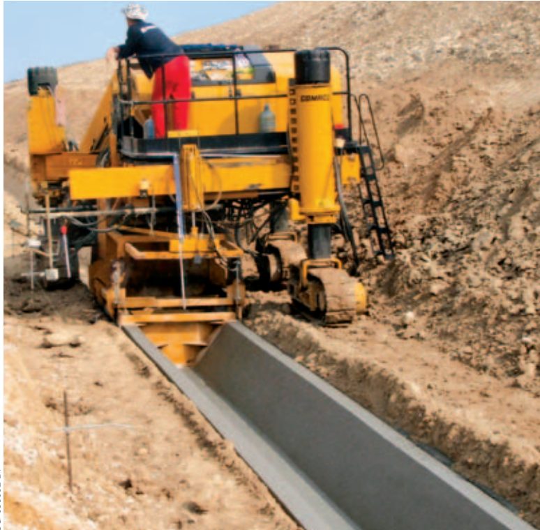
Patstroy Ead Lovetch slipforms water canal with their three-track Commander III in the countryside near Lovetch, Bulgaria.
