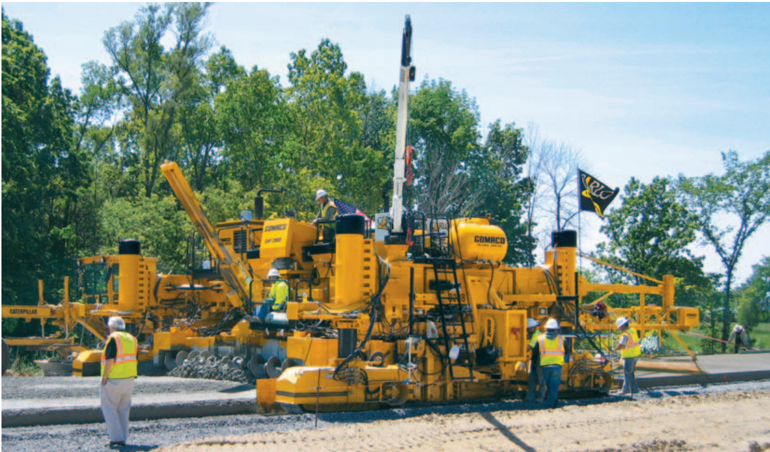
The westbound lanes of I-94 were slipformed with the GHP-2800 with IDBI placing the transverse joint, 24 bars every 14 feet (4.3 m).
