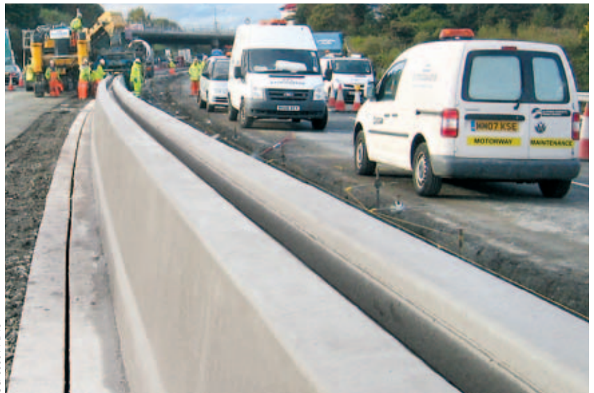
Extrudakerb slipformed the wide step barrier when the differences in roadway heights was less than 300 millimeters (11.8 in).
