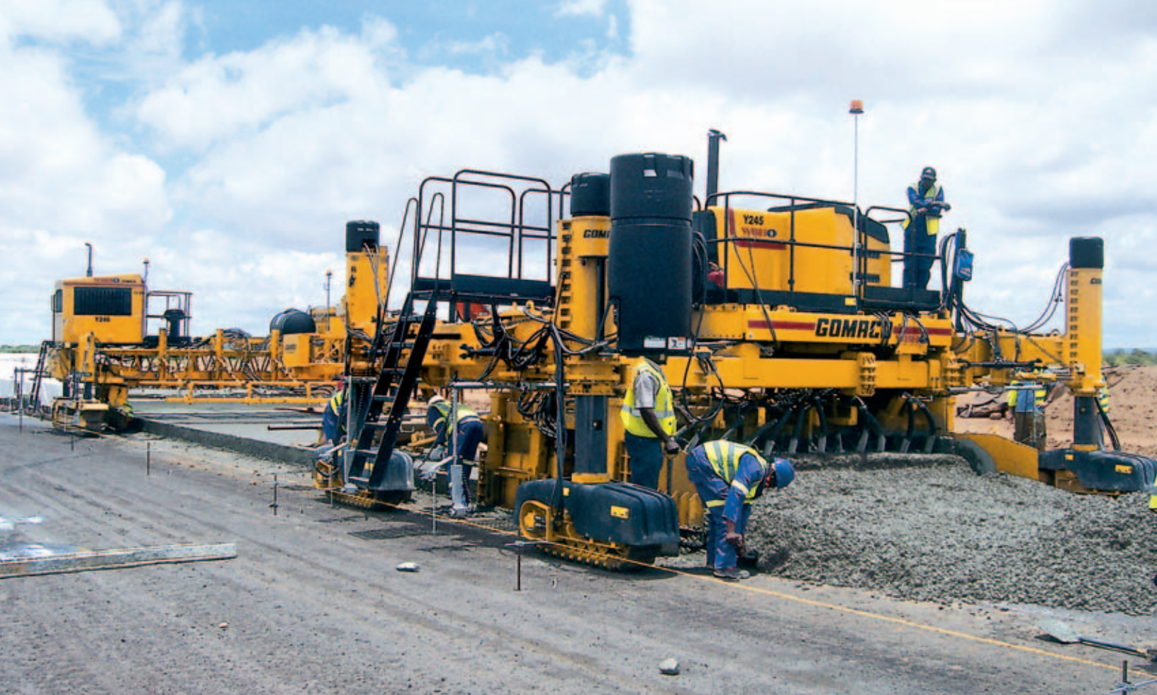
A Commander III four-track slipforms a new one kilometer (0.6 mi) long runway extension on the international airport in Botswana.
