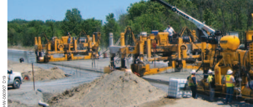
Two placer/spreaders work in front of the paver. Carlo never wants th
