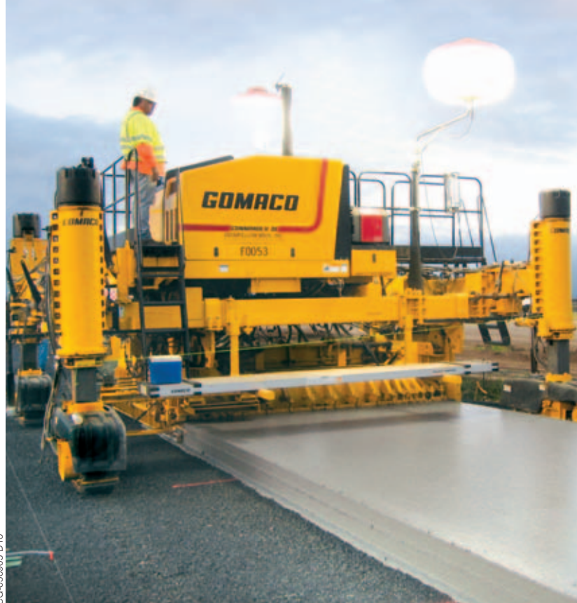
The Commander III paves each of the four lanes of the new roadway 12 feet (3.7 m) wide and 10 inches (254 mm) thick.
