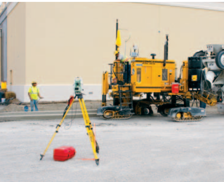
The GT-3600 holds line and level on the curb and gutter in the straight sections of the project.
