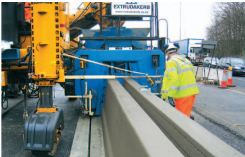
The wide step barrier required 0.7 cubic meters (0.9 yd 3 ) of concrete to slipform just one meter (3.3 ft). The sheer size and dimensions of the wall are illustrated in the drawing.
