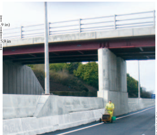
The finished wall shows the hand-formed concrete support for the street lamps and bridge pier approaches.
