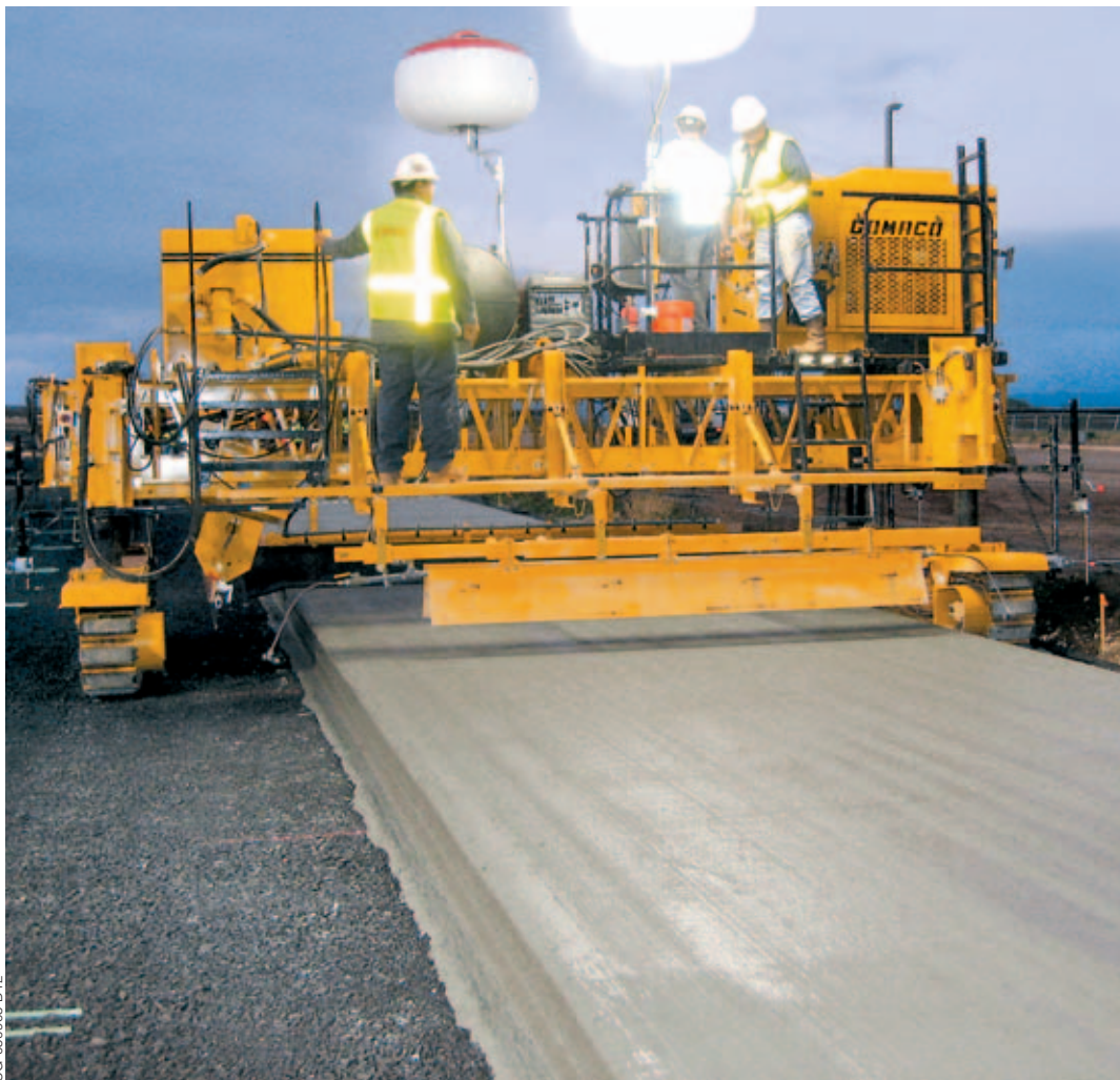
A T/C-600 texture/cure machine, set at 16 feet (4.9 m) wide between the tracks, follows the paver pulling an AstroTurf drag, and applies a spray cure and a transverse tine.
