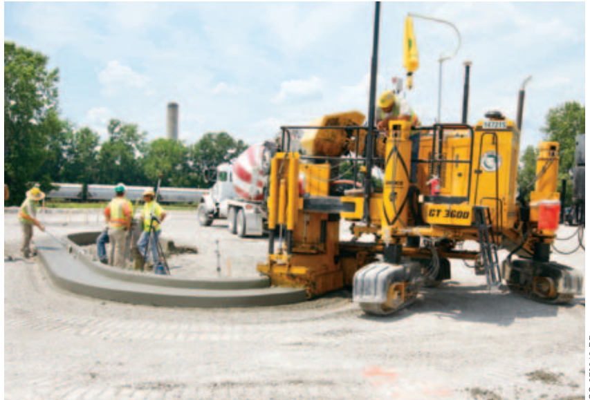
The G21 controller on the GT-3600 works with the Leica computer and its tracking system to slipform the project’s tight radii.
