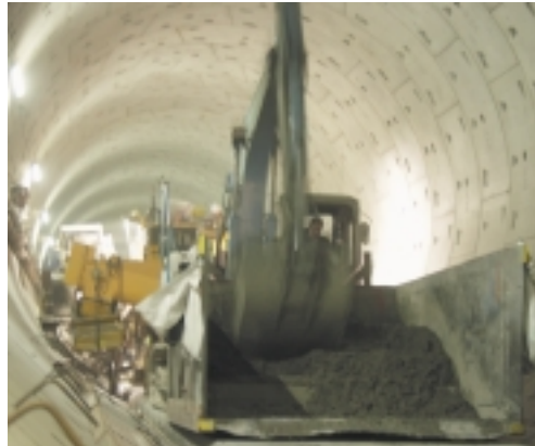
Concrete is dumped into a skid and an excavator places the concrete into the hopper.
