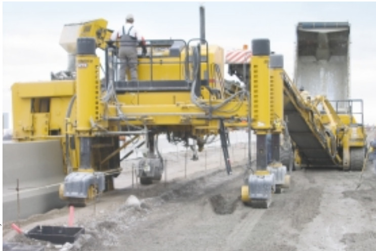
An RTP-500 or 9500 fed concrete into the Commander III.
