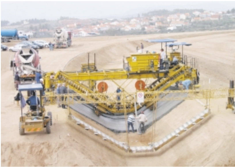
The CP-650 finishes the three-sided canal in one pass. The canal had a slope of 1.5:1 with a bottom width of 6.6 feet (2 m).
