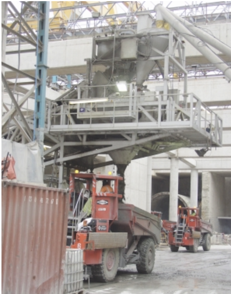
Davidson's Compactor batch plant is located down in the Stratford box, just outside the two tunnel openings.
