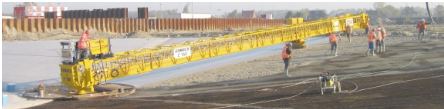
Van Burgt in Zoetermeer, Netherlands, are finishing concrete bases for wastewater treatment tanks. The C-750 works on a pivot point and is set up at 105 feet (32 m) wide to finish half of the 210 foot (64 m) slab during each pour.
