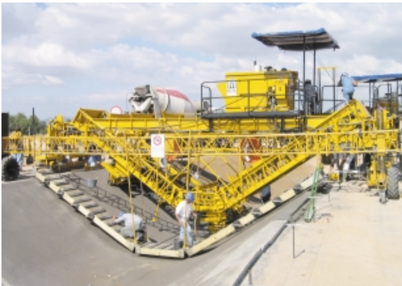
Mota has an RC Conveyor placing concrete on the grade in front of the CP-650 and a Spanit work bridge follows the finisher.
