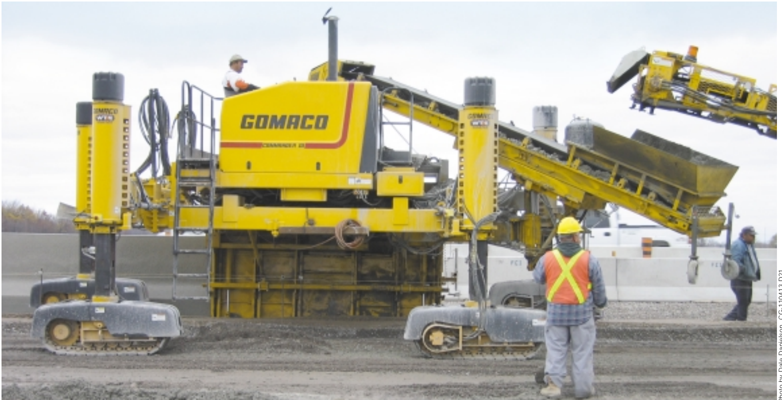
A four-track Commander III slipformed variable barrier as tall as six feet (1.8 m) high on the project.
