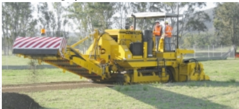
Boulderstone Hornibrook Pty. Ltd. test trim an area with their 9500 with Leica stringless control in Sydney, Australia.
