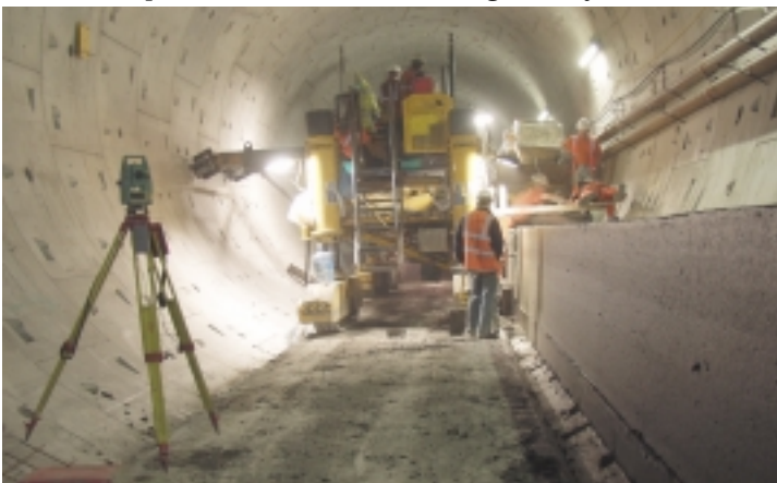
Tunnel conditions didn't allow room for the setting of stringline, so Davidson equipped his paver with the Leica stringless system.
