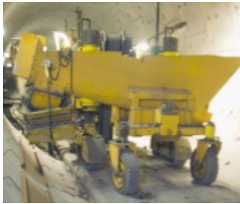
The Commander III has an extra-large hopper to receive concrete from the excavator.
