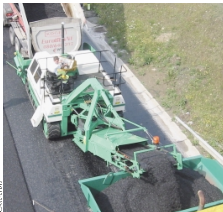
Hoogmartens N.V.'s RTP-500 was equipped with heat resistant belts to place asphalt on a project in Belgium.
