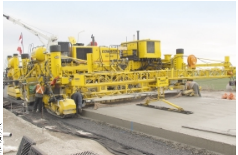
An AutoFloat® works behind the GHP-2800 IDBI paver.
