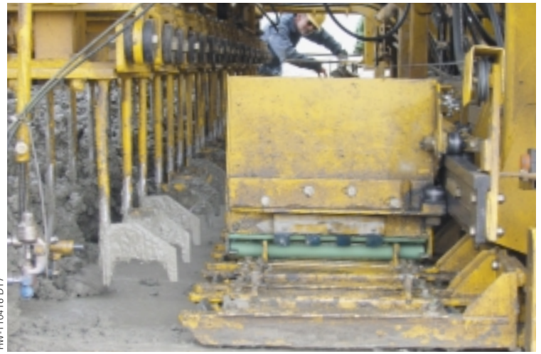
The IDBI, paving 23.8 feet (7.25 m) wide, inserted 23 bars across the slab, 11.8 inches (300 mm) apart.
