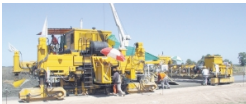
Esuco S.A. is slipforming 24.6 feet (7.5 m) wide on the new Route 6 with their GP-2600 paver with IDBI near San Vicente, Argentina.
