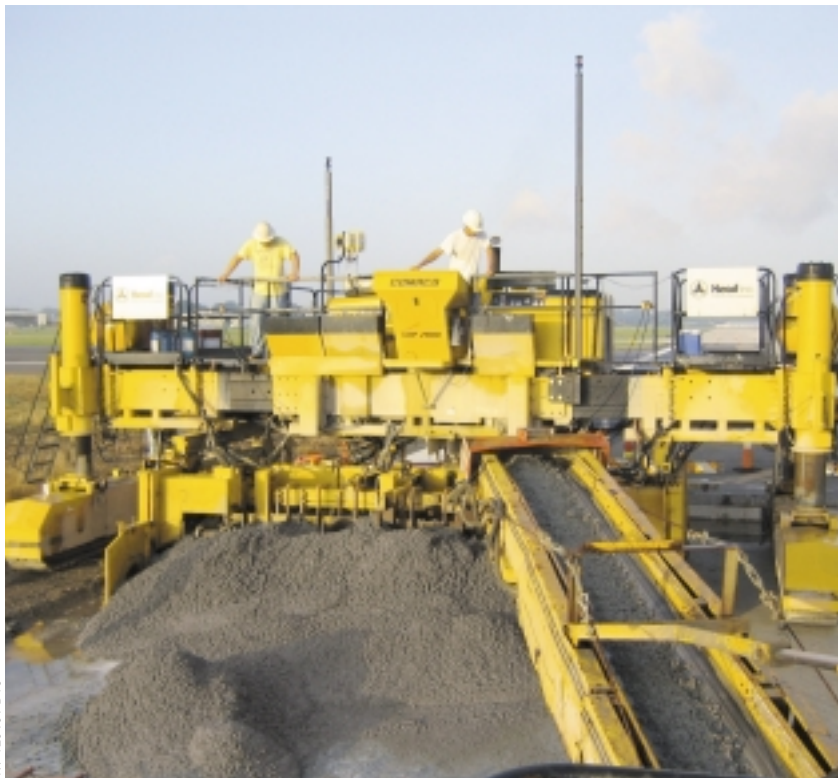
The GHP-2800 paver is slipforming 18.75 feet (5.7 m) wide and 15 inches (381 mm) thick.
