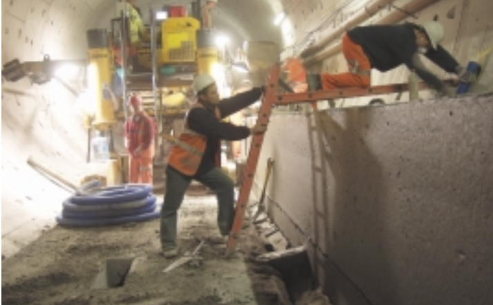
The Commander III paves over the ductwork in the wall and finishers expose and finish around it right away.
