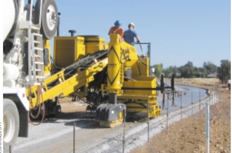
Muse slipformed 5500 feet (1676 m) of five foot (1.5 m) wide, four inch (102 mm) thick sidewalk on the project.
