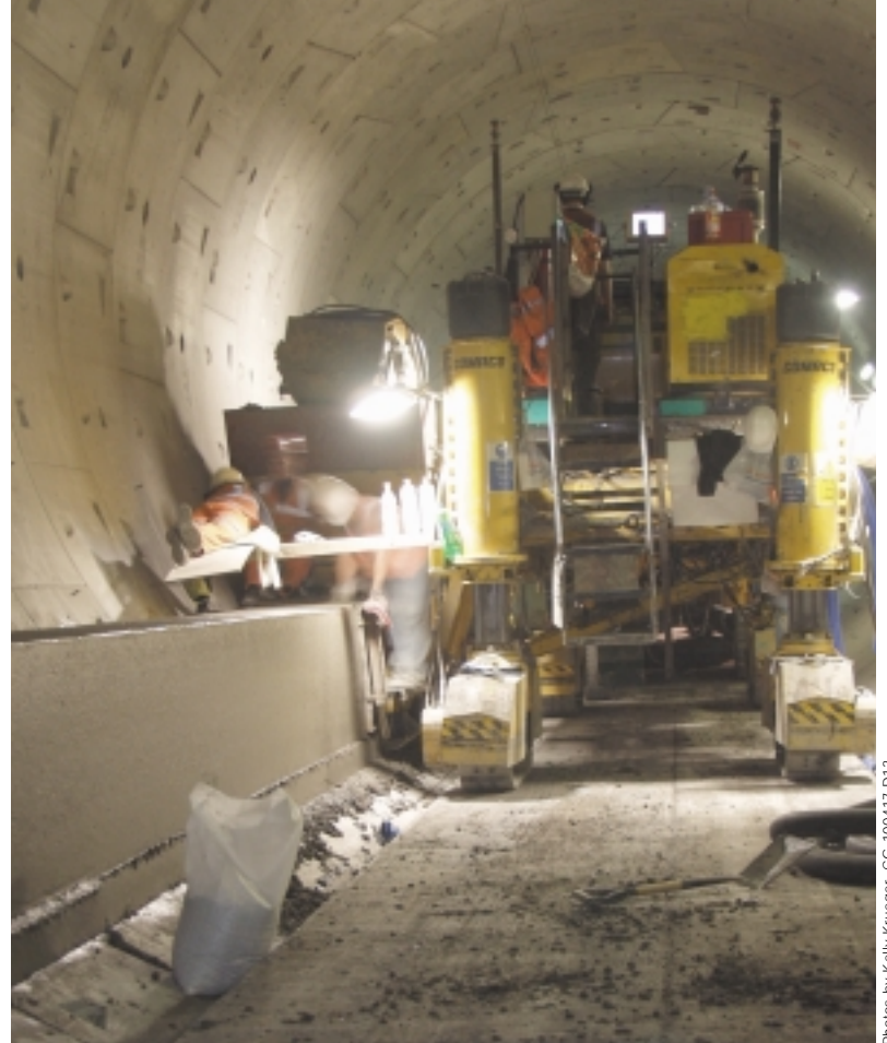
Tunnel conditions didn't allow room for the setting of stringline, so Davidson equipped his paver with the Leica stringless system.
