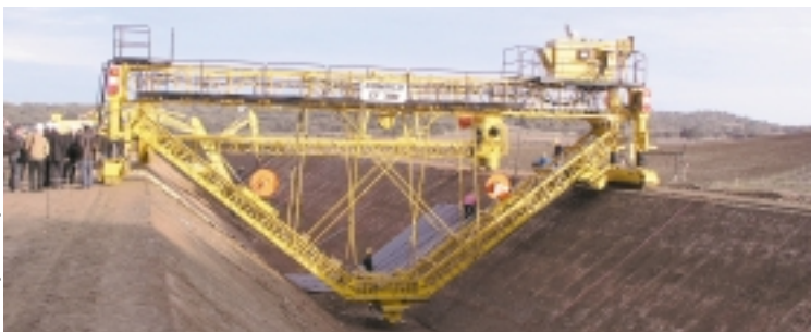
The CF-790 successfully completes a dry run in Portugal.
