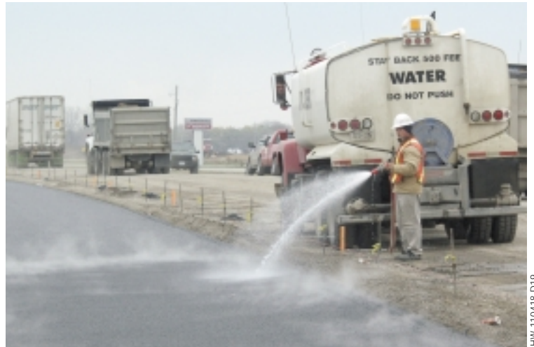
The asphalt drainage layer was laid directly in front of the paver and had to be cooled down to meet temperature requirements.
