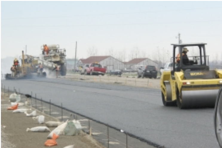
The subgrade on the project was an open-graded drainage layer (OGDL) made up of an asphalt drainage layer.
