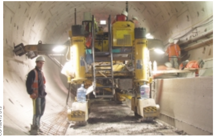
A hydraulic jack system keeps the paver from being pushed off line throughout the tunnels' many curves.
