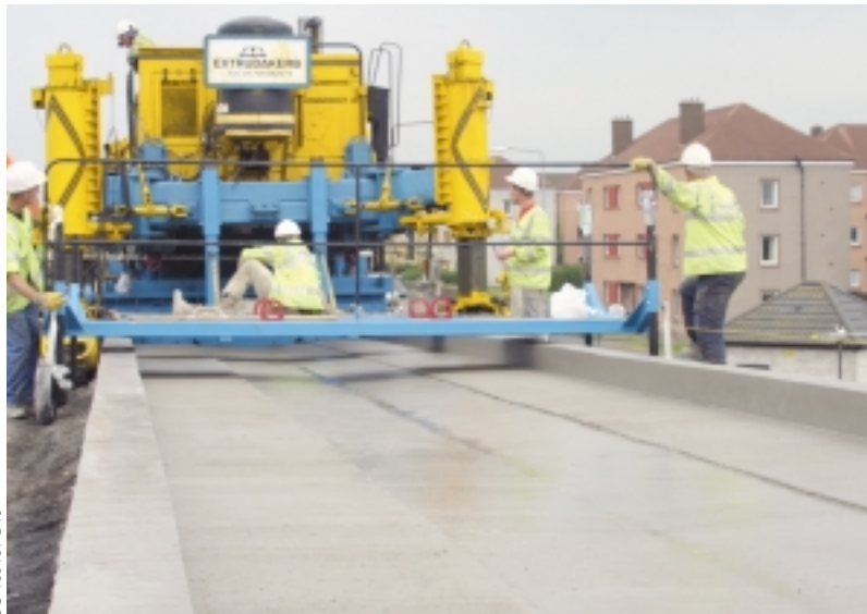
Extrudakerb slipformed busways for the city of West Edinburgh, Scotland. The special profile is for the city's buses, which have steering mechanisms on the wheels that sense off the curbs for automatic steering capabilities.
