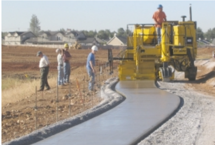
The meandering sidewalk is a city of Redding, California, specification with radii up to 100 feet (30.5 m) long.
