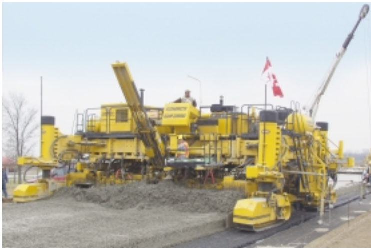
A front-mounted bar inserter for longitudinal joints is controlled by the IDBI's computer which inserts the bars at the proper spacing.
