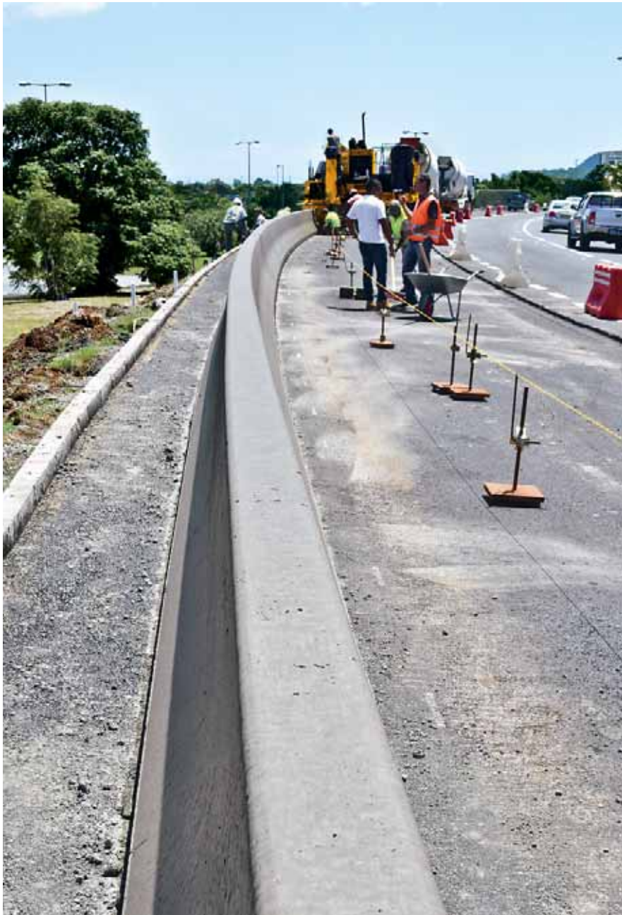
The 4400 slipforms left-side mount barrier wall next to traffic.
