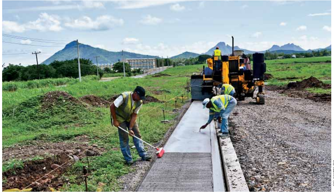
The 4400 paves a sidewalk with finishers applying a hand-broomed texture behind the machine.
