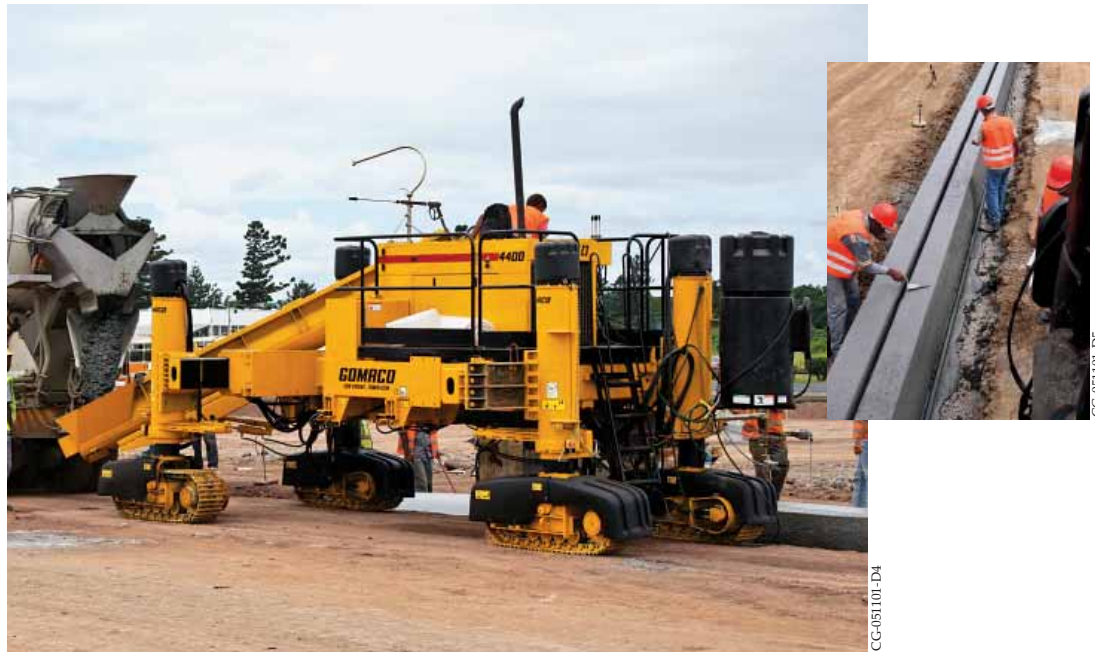
The 4400 slipforms a 19.7 inch (500 mm) slot drain. The photo to the right shows the view from the top of the 4400 looking down on the new slot drain.
