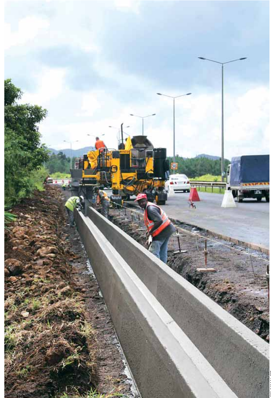
The 4400 barrier paver slipforms a 19.7 inch (500 mm) tall U-channel, below grade, and next to an existing road.
