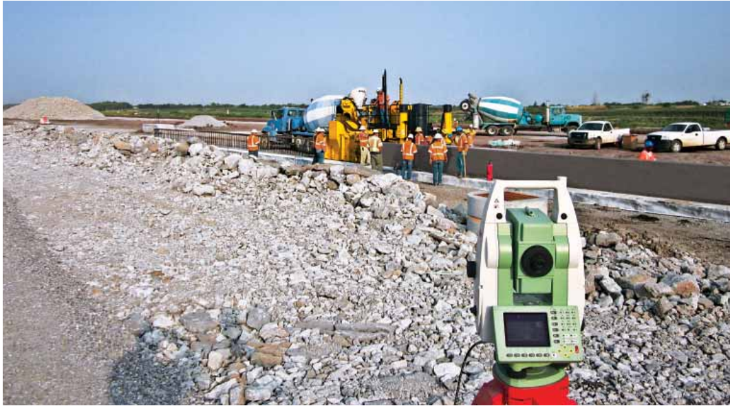
The 4400 uses 3D stringless technology to slipform a barrier.
