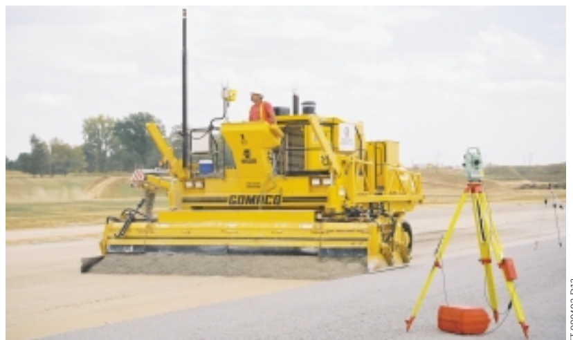
A total station tracks the progress of a 9500 trimmer as it works on a project in St. Louis, Missouri.
