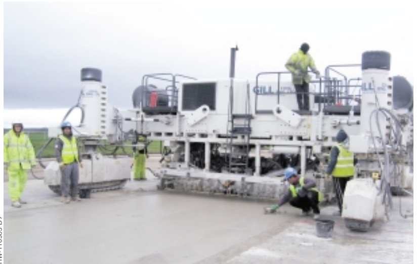
The airport project, with only 16,744 square yards (14,000 m 2 ) of concrete paving, was a small one for Gill Civil Engineering.
