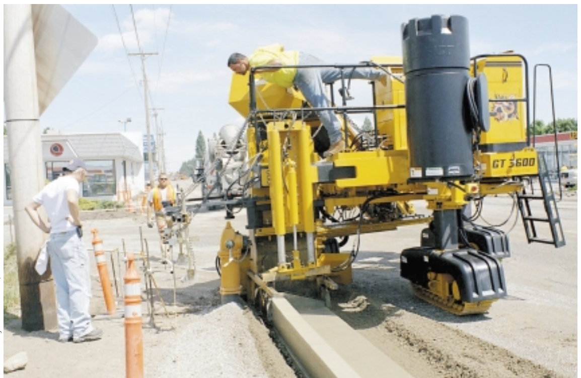
The GT-3600 does some tight-clearance paving to get by a fire hydrant on the project.
