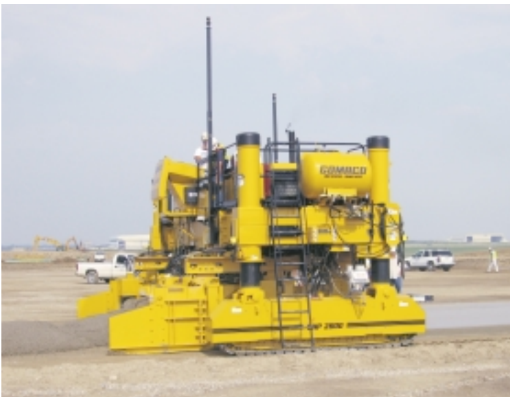
A GHP-2800 paver slipforms an econcrete subbase on this project at the Indianapolis International Airport.
