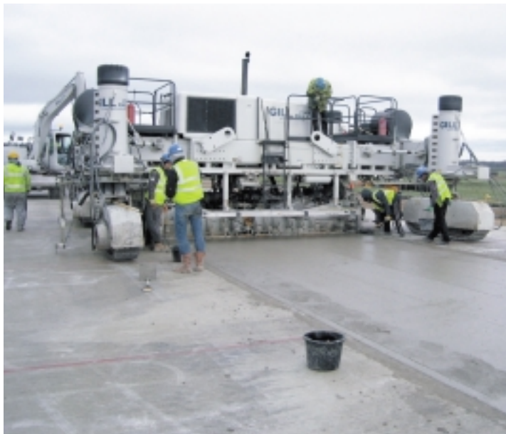
Joints had to be wet saw cut every 16.4 feet (5 m) and crews were cutting up to 105 joints per day into the new concrete.
