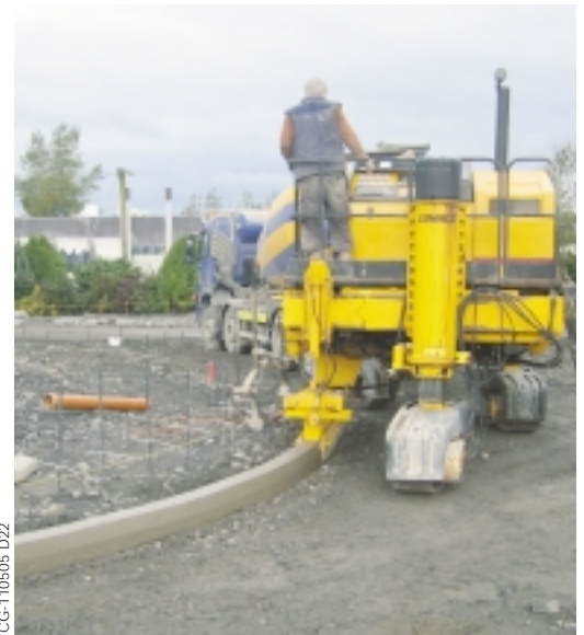
Liam Maher uses a Commander III to slipform curb around a new car dealership in Cashel in County Tipperary, Eire, Ireland.
