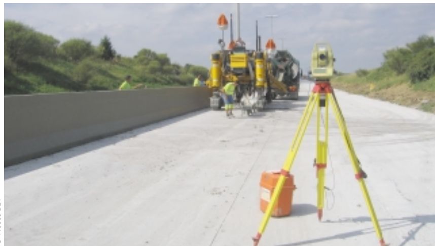
Barrier wall on Highway E411 in Belgium was slipformed with the Leica 3D stringless guidance system.
