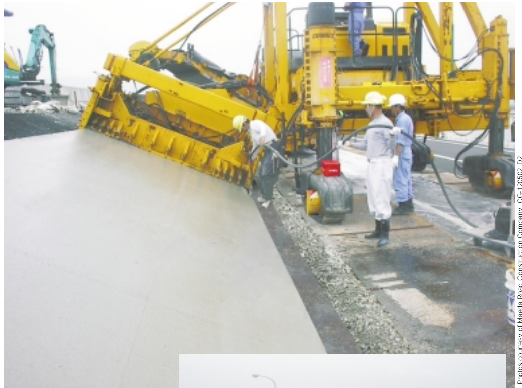
Photos courtesy of Maeda Road Construction Company CG-120502 B2
