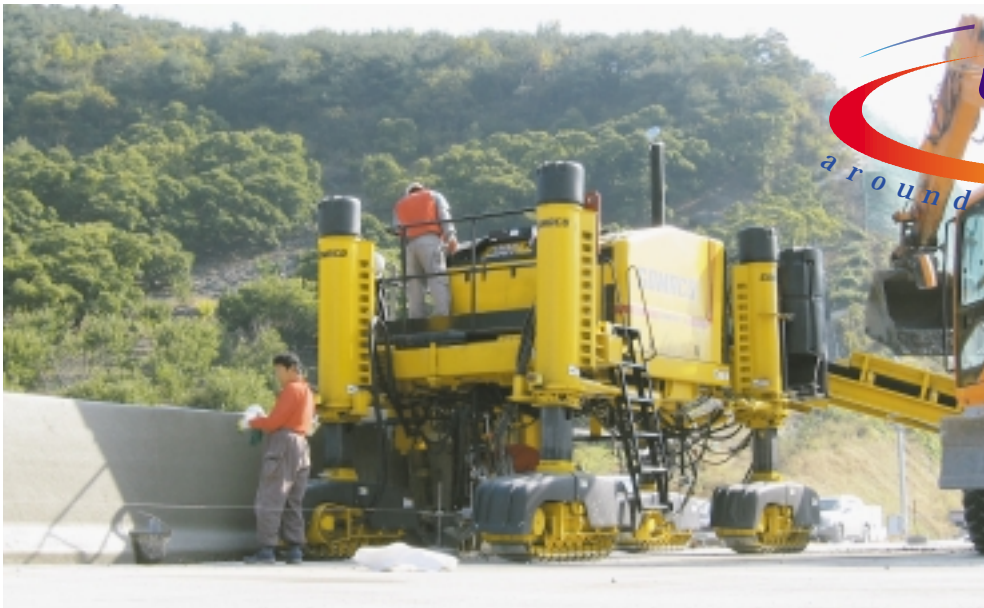
Machang Construction Equipment slipformed barrier wall with their new Commander III on a project in Korea.
