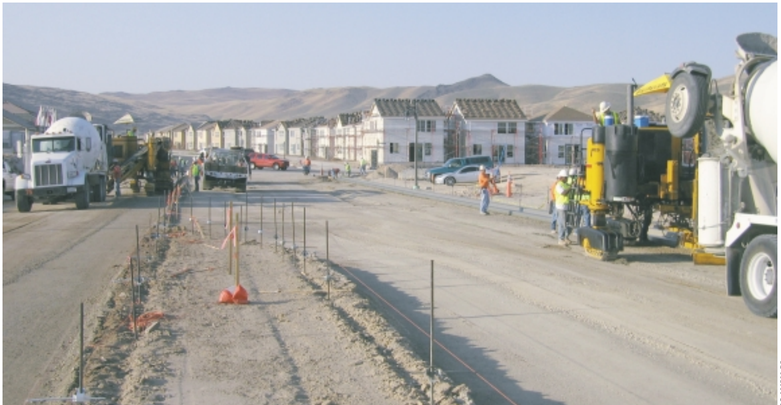
Two curb machines with operators, 16 ready-mix trucks and 26 workers slipformed 550 cubic yards (421 m 3 ) of curb and gutter in 9.5 hours.
