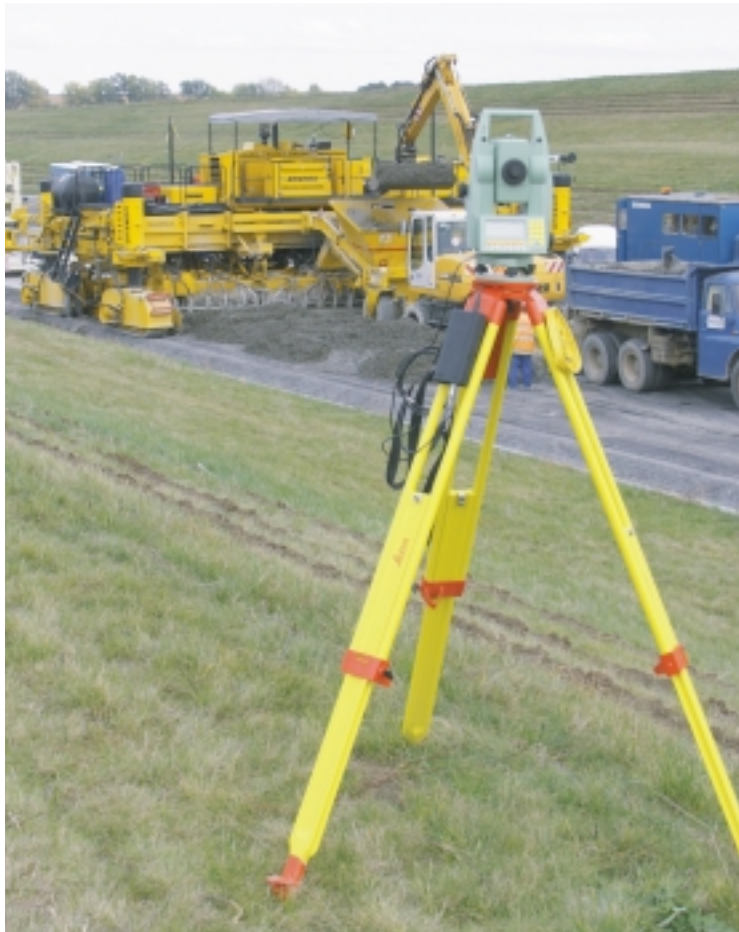
A Leica total station tracks the progress of the GOMACO GP-4000 paver on a highway project in the Czech Republic.
