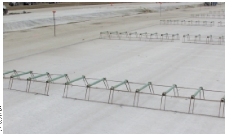
The econocrete subbase has to be sprayed with a bond-breaker before paving.
