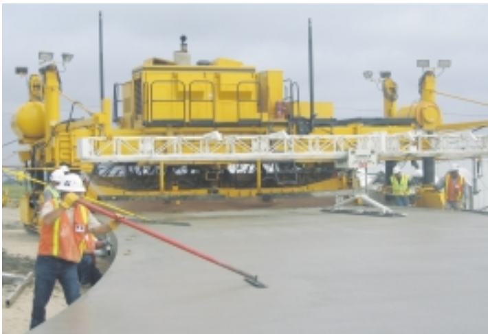
A stringless GP-4000 slipformed a 24 inch (610mm) thick slab at the Atlanta Hartsfield Airport in Atlanta, Georgia.
