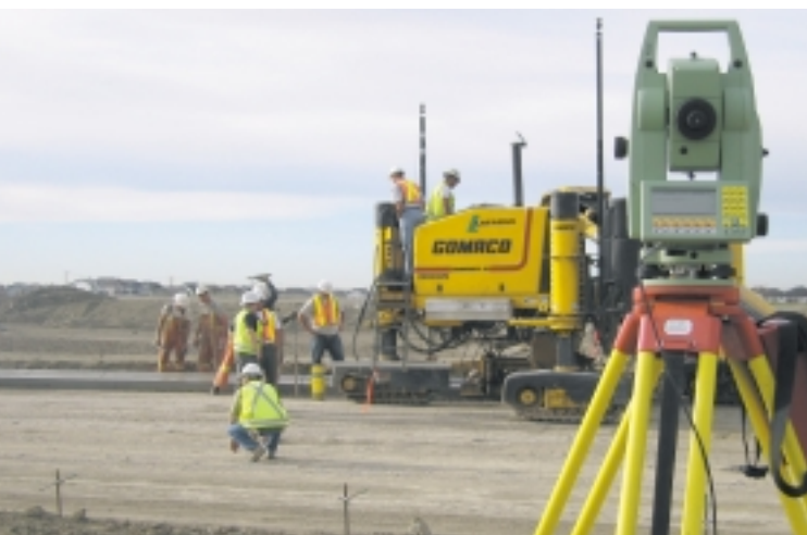
A Commander III slipforms curb and gutter with the 3D system on a project in Calgary, Alberta, Canada.
