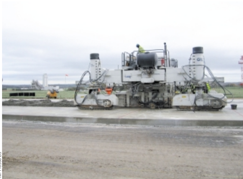
Gill Civil Engineering's next projects will be on the Birmingham, East Midlands and Manchester airports in England.
