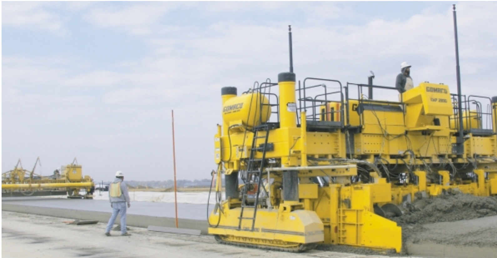
Edge slump on the airport paving project is very important, and according to Keys, the GHP-2800 is doing very well with it.
