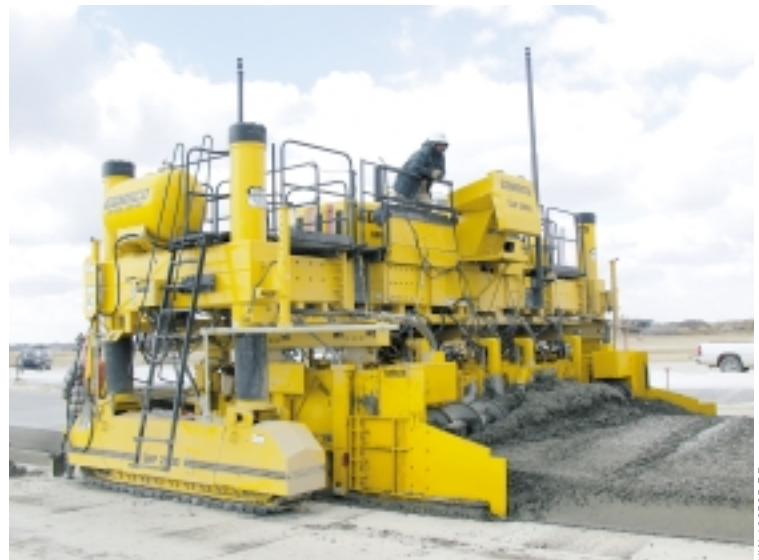
P aving passes with the two-track GHP-2800 are 20 feet (6.1 m) wide and 16 inches (406 mm) thick.
