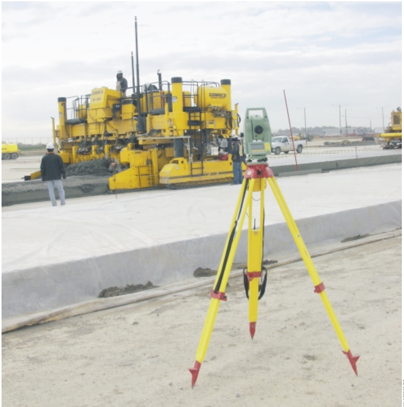
One of the three Leica total stations on the project tracks the GHP-2800 paver as it slipforms the new apron.
