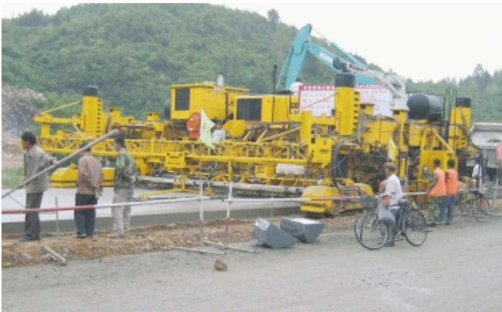
Jiangcheng Highway and Bridge Company use their new four-track GHP-2800 with In-the-Pan Dowel Bar Inserter (IDBI) to slipform a new highway in the Yanbian Autonomous Region, China.
