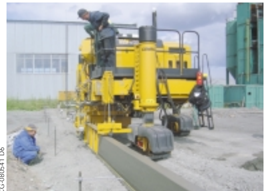
Kosmos slipforms stand up curb with their Commander III in Perm, Russia.
