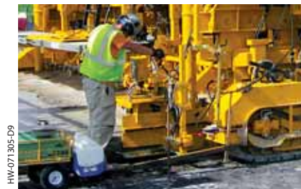
Trailing form with manual bar insertion. The trailing form with manual or air-powered bar insertion is designed to trail the track on two-track pavers. This system will accommodate most types of bars.
