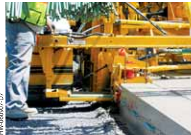
Trailing form with air-powered bar insertion.
