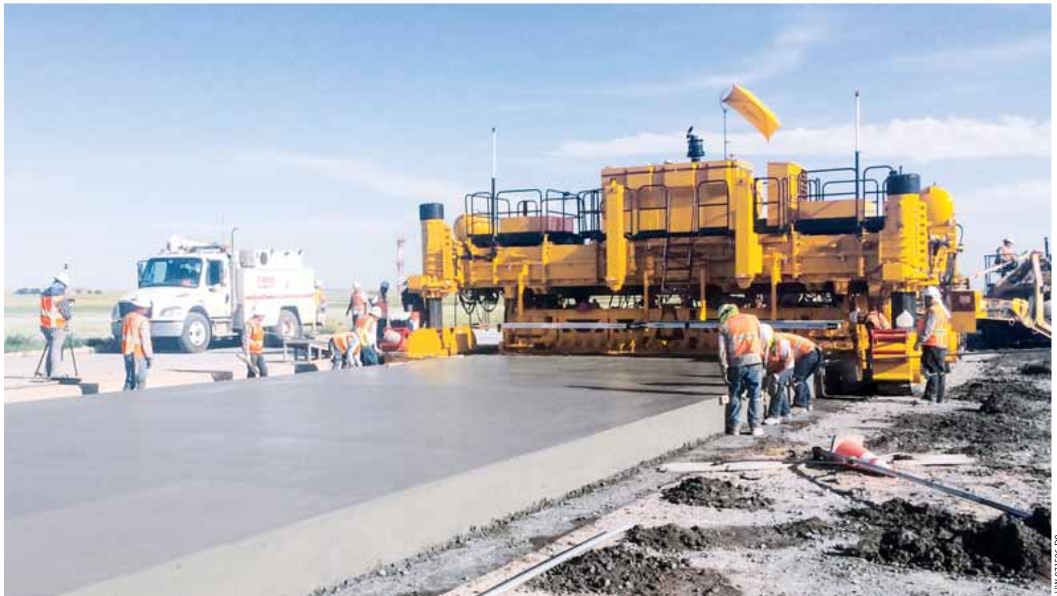
The GOMACO GP-4000 slipform paver features the exclusive G+ control system and is at work on the Denver International Airport in Denver, Colorado. The four-track GP-4000 is slipforming paving passes 25 feet (7.6 m) wide and 18 inches (457 mm) thick on the new runway. It is equipped with a 3D stringless guidance system.
