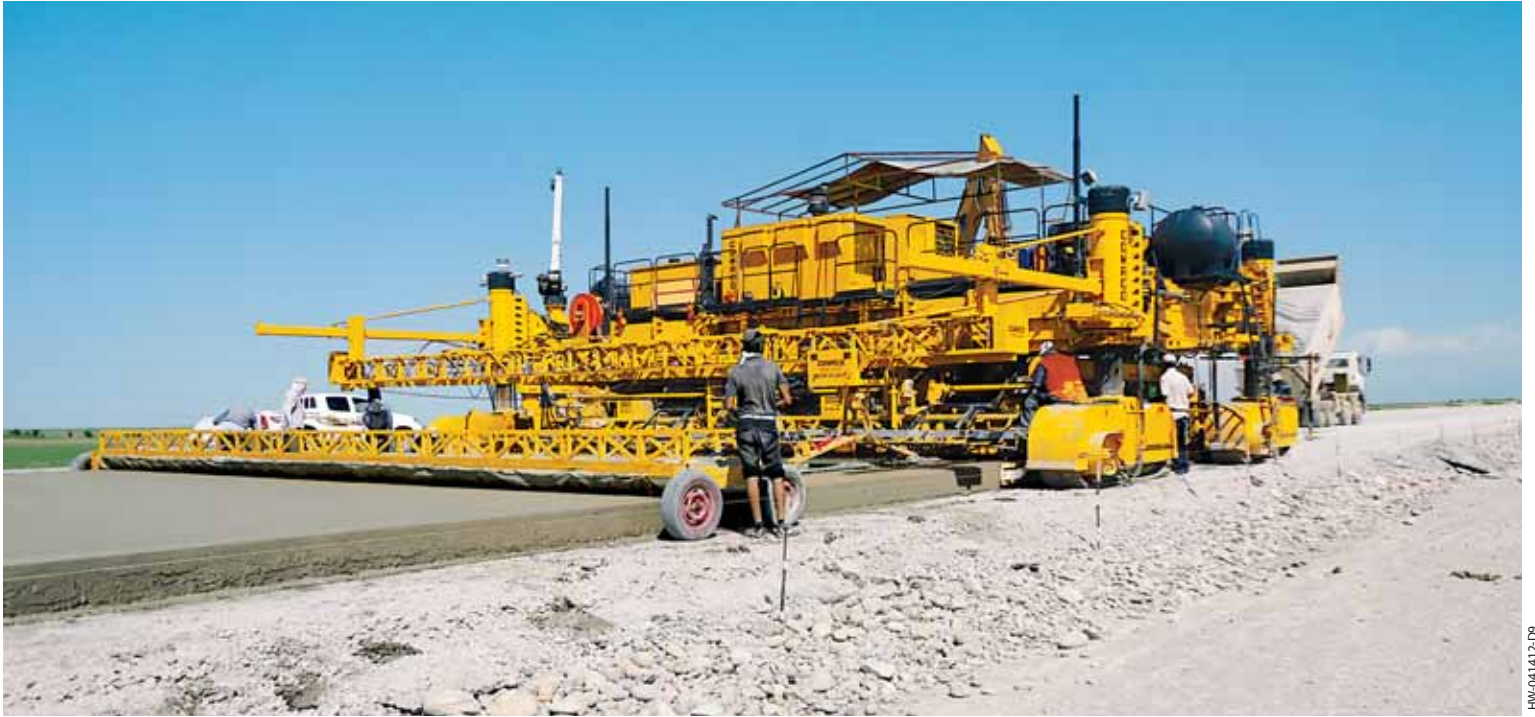
GOMACO's four-track GP-4000 is equipped with an IDBI for accurate dowel bar placement while slipforming the "New Silk Road" in Kazakhstan.
