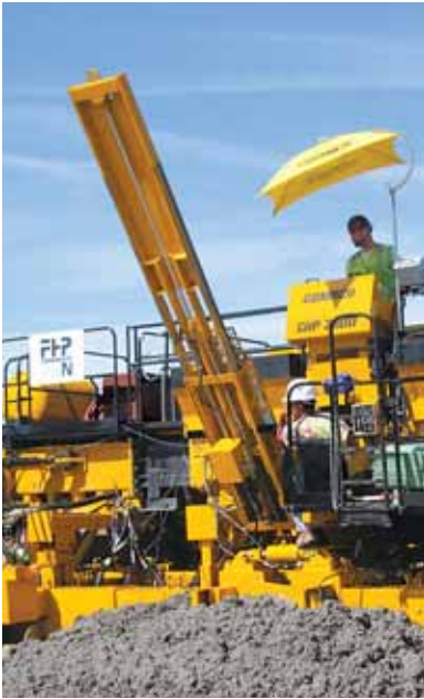
The frame-mounted tie bar inserter (TBI) accurately places the transverse bars for the longitudinal joint by placing the bars behind the vibrators.
