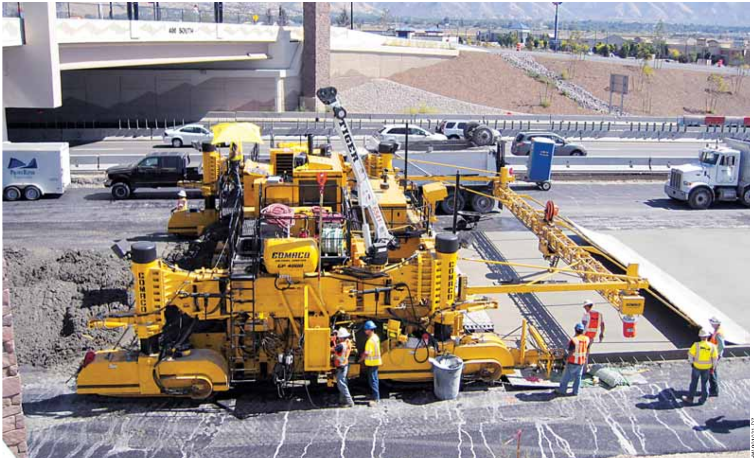
The GOMACO four track GP-4000 with IDBI attachment slipforms 39 feet (11.9 m) wide on the northern portion of the Interstate 15 CORE project in Utah. The northern section of the project is six travel lanes wide northbound and southbound for 12 lanes of concrete pavement.
