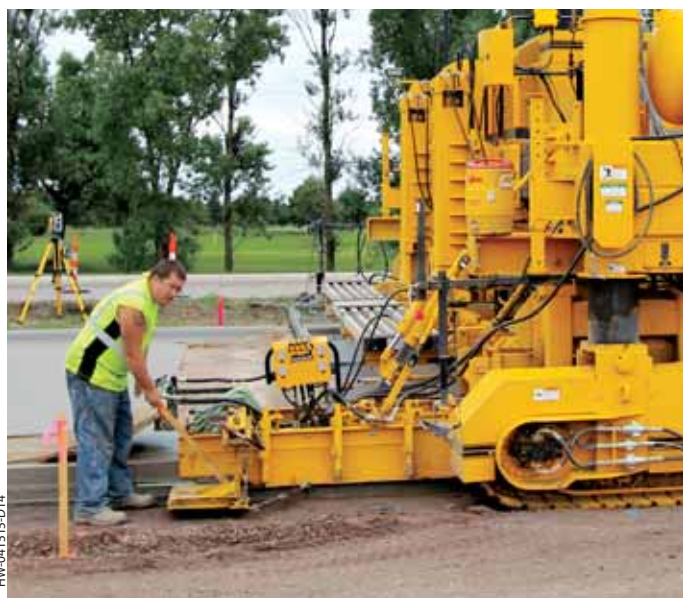
Trailing form with manual bar insertion. The trailing form with manual or air-powered bar insertion is designed to trail the track on two-track pavers. This system will accommodate most types of bars.
