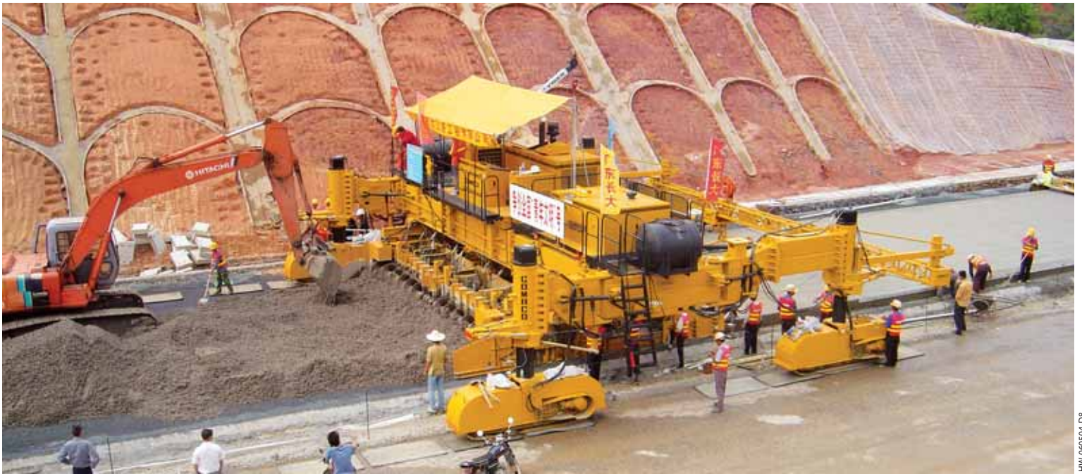
The GP-4000 four-track, equipped with the IDBI dowel bar inserter, is slipforming the Meihe Highway in the Guangdong province of China. This mainline highway project is being slipformed at 29 feet (8.84 m) wide and 11 inches (279 mm) deep.
