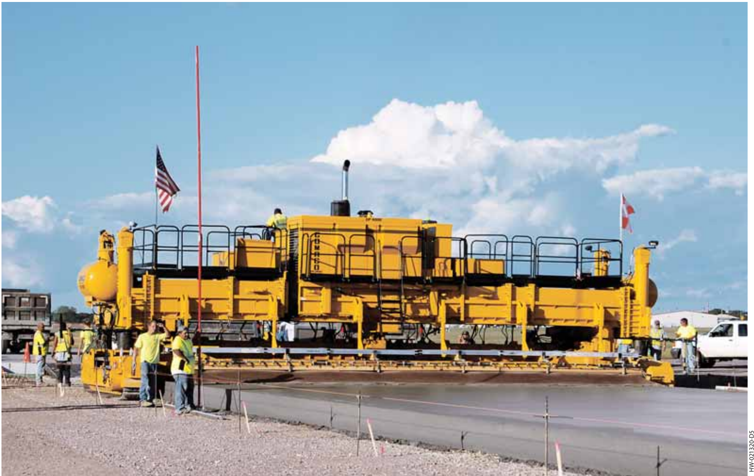
The intersection between the two major runways at the Sioux Falls Airport in Sioux Falls, South Dakota, was removed and replaced in just two weekends. Paving production with the GOMACO GP-4000 averaged 400 cubic yards (305.8 m 3 ) per hour. A second batch plant had to be utilized to keep up with the paver's production while slipforming 37.5 feet (11.4 m) wide.
