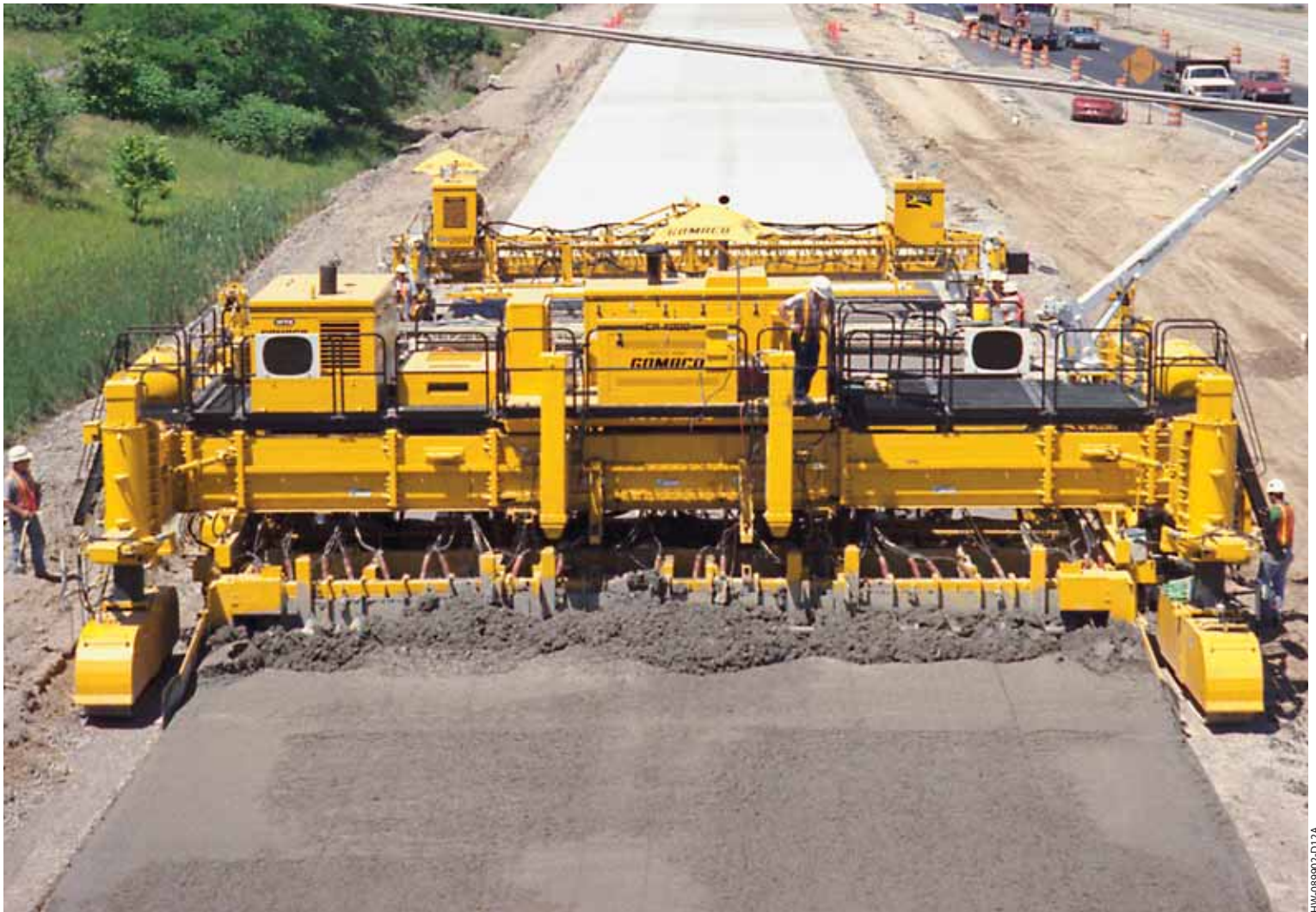
The GOMACO paving train provided high-production on this mainline paving project in Detroit, Michigan. The company used their GOMACO placer/spreader for accurate placing and spreading of concrete in front of the GP-4000 paver, and following the paver was the GOMACOT/C-600, used for texturing and curing the slab. The versatile GP-4000 has a telescoping modular frame. Depending on the paving width, various vibrator packages provide from 16 to 48 vibrator circuits.
