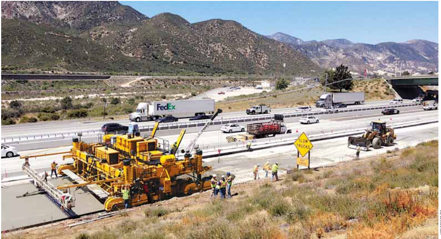
The four-track GP-4000 is slipforming a 34 foot (10.36 m) wide section of the Interstate 15 in Ontario, California. The slipform paver is equipped with GOMACO's exclusive G+® operating system and an IDBI to place the transverse dowel bars.
