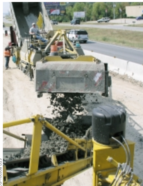
The front of Weaver Bailey’s mold is hydraulic and can be opened or closed depending on what type of reinforcement the wall specification requires.
