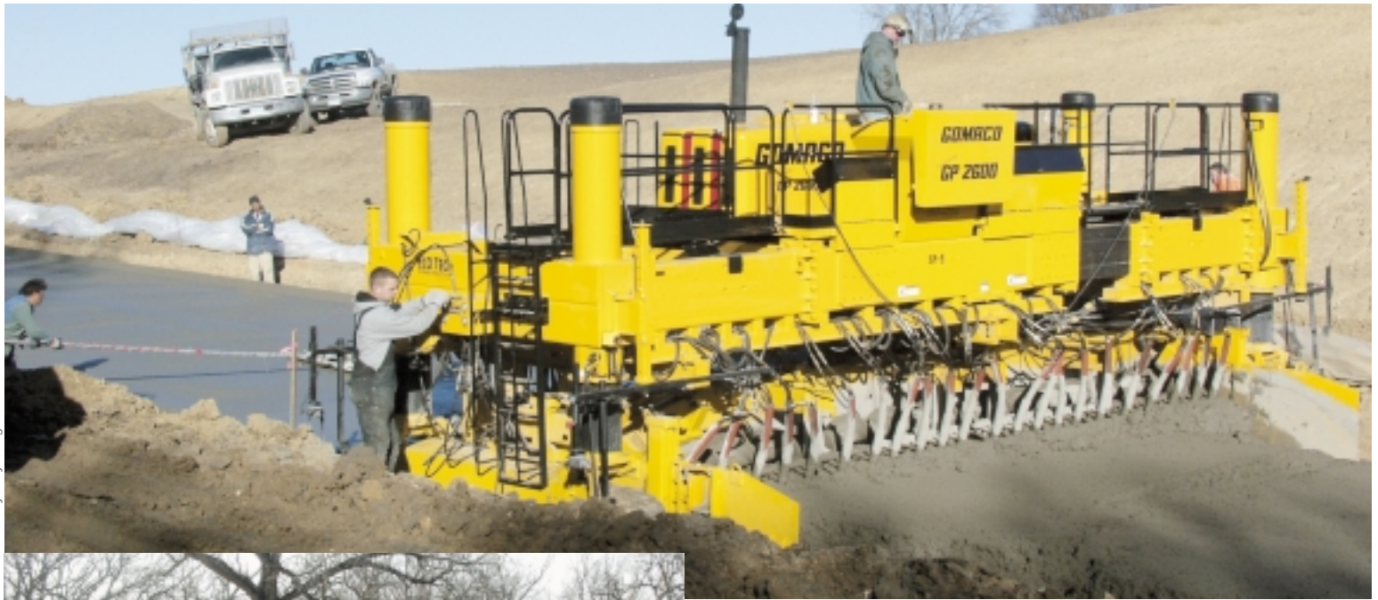
Eco Tech works on a new roadway with their new generation GP-2600. The full-width paving is slipformed with integral curb on both sides.
