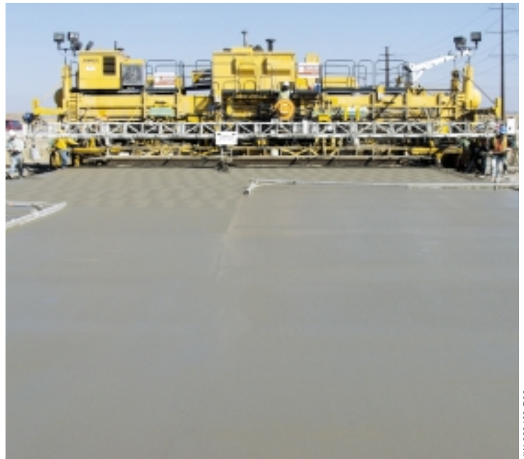
CDOT utilizes the one-tenth blanking band on their projects and readings under 15 inches per mile (287 mm/km) earn bonus. On this section of pavement, Lawson's best reading was 9.4 inches (148 mm).
