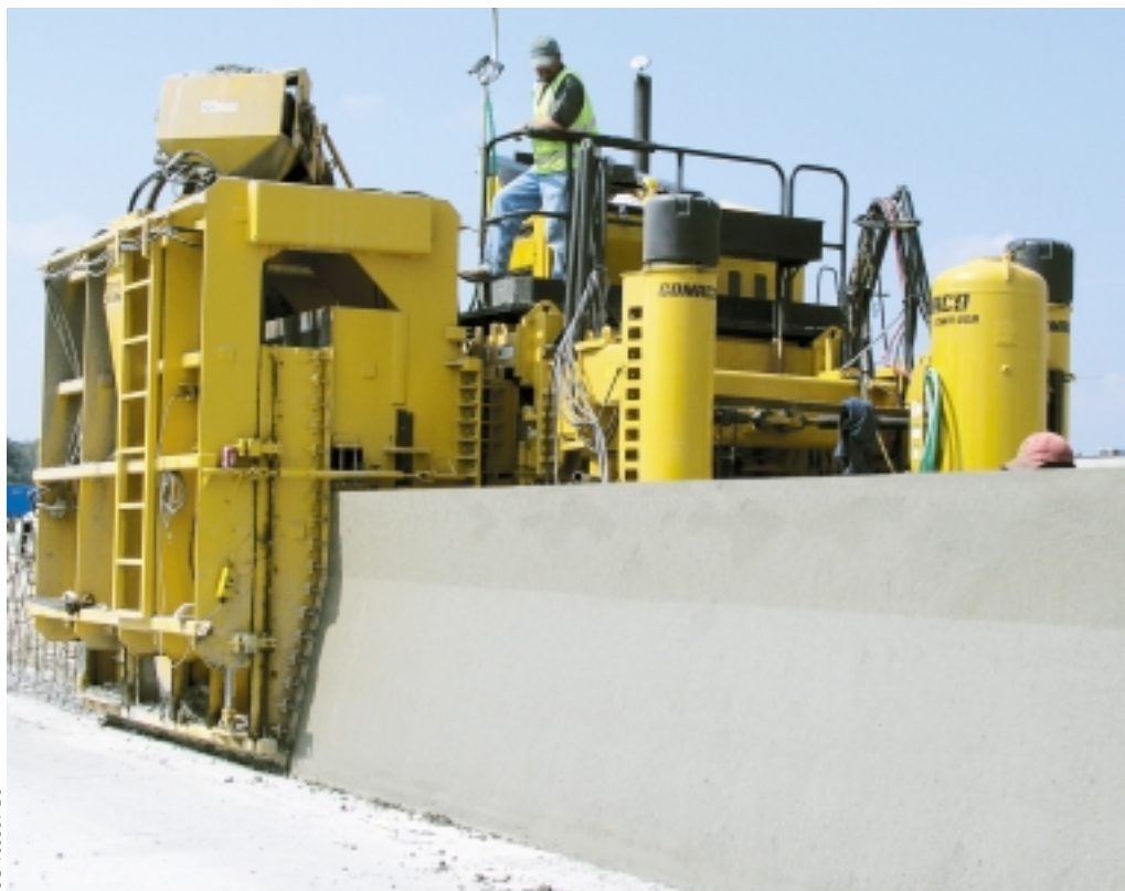
A high volume of concrete was needed to slipform the wall. Weaver Bailey used end-dump trucks and an RTP-500 to keep the Commander III supplied.
