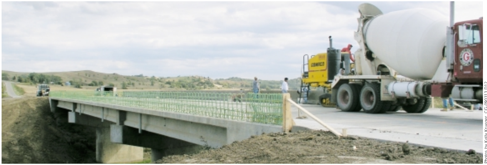
Dormark Construction slipforms 34 inch (864 mm) tall parapet wall with their Commander III on two bridges near Holly Springs, Iowa.
