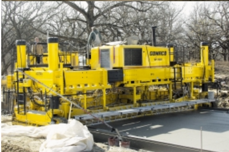
Eco Tech works on a new roadway with their new generation GP-2600. The full-width paving is slipformed with integral curb on both sides.
