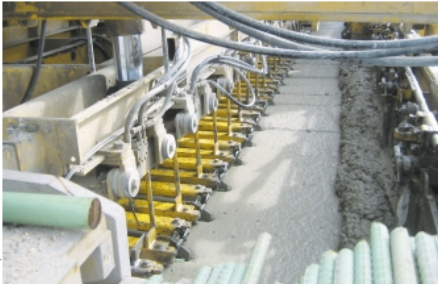
Concrete slump averages 1.5 inch (38 mm). Lawson feels it’s the ideal slump when working with an IDBI and inserting bars.
