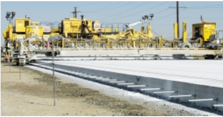
Lawson is paving 40.5 feet (12.3 m) wide, 13 inches (330 mm) thick with their GP-4000.
