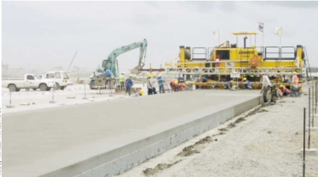
The width of the new slabs varies between 16.4, 18 and 19.7 feet (5, 5.5 and 6 m) wide. All of the slabs are 17.7 inches (450 mm) thick.
