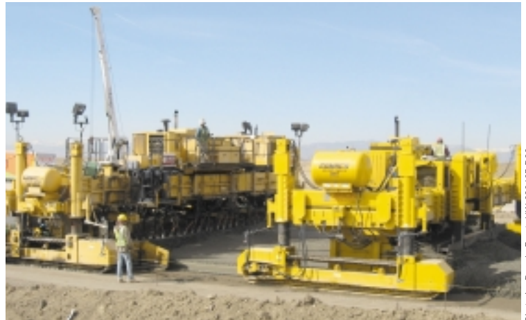
A GP-3500 with a strike-off blade attached to the outrigger works in front of the GP-4000 paver spreading the concrete.
