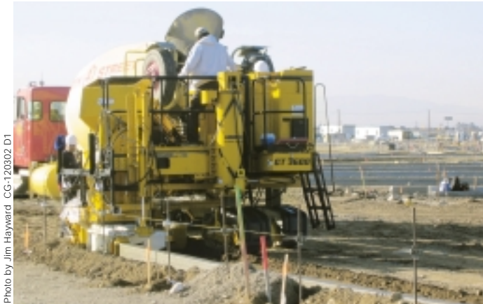
The GT-3600 will be slipforming approximately 60,000 feet (18,288 m) of curb and gutter for the new shopping center.
