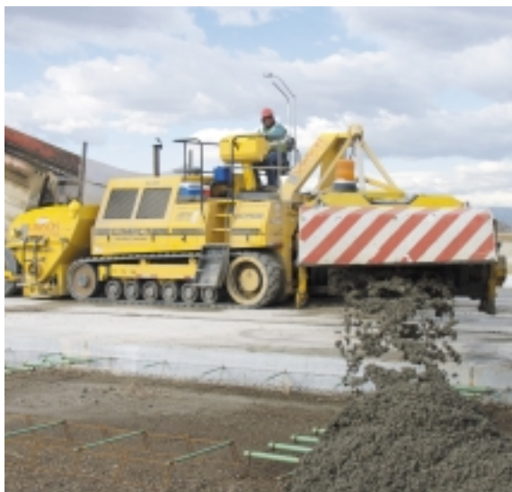
An RTP-500 places concrete in front of the GP-2500.
