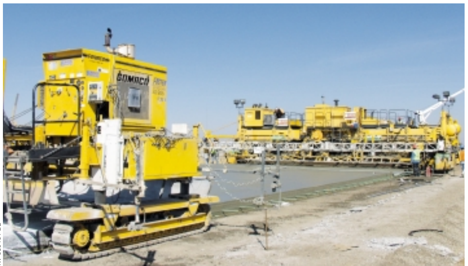
A T/C-600 applies a longitudinal tining to the new interstate.
