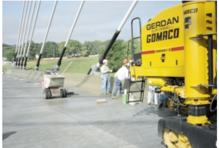
The Commander III is putting such a smooth finish on the wall, the finishers have very little work to do behind the machine.
