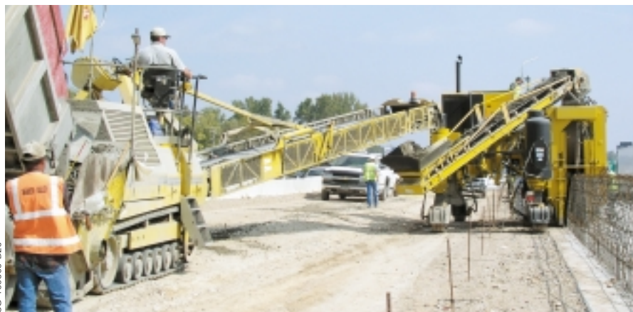
The steel reinforcement was one of the most challenging aspects of the project and Weaver Bailey worked closely with GOMACO engineers to develop a barrier mold that could accommodate it.
