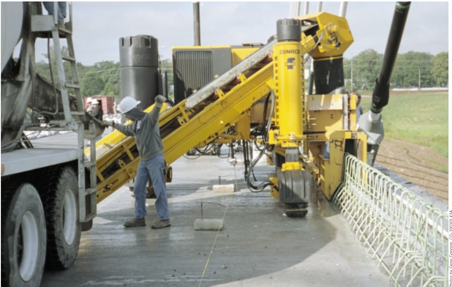
Production averaged 1100 feet (335 m) of 18 inch (457 mm) wide median barrier per day.
