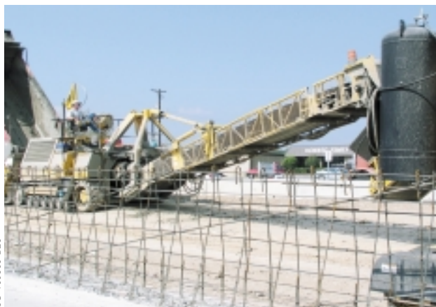
A high volume of concrete was needed to slipform the wall. Weaver Bailey used end-dump trucks and an RTP-500 to keep the Commander III supplied.
