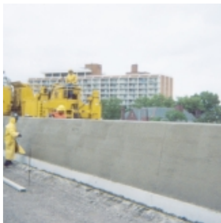
Complete General slipformed what could be the tallest section of barrier wall without steel reinforcement. The wall is 93 inches (2362 mm) tall.
