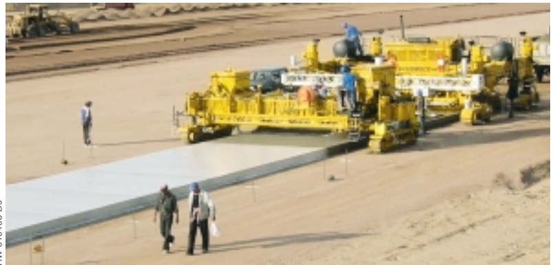
Condotti slipforms a runway (above) for a new airport in Aqaba, Jordan. They're using a four-track GP-2600 with Auto-Float® and a T/C-600 texture/cure machine.
