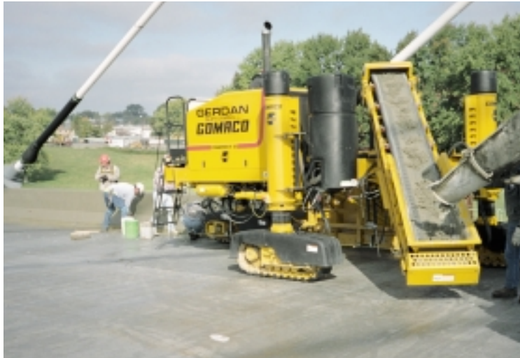
Gerdan is slipforming three different types and approximately 14,500 feet (4420 m) of wall on the new bridge.
