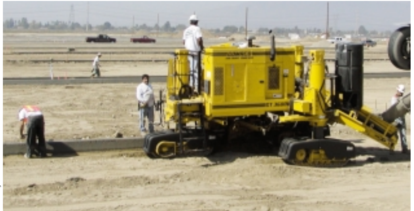
Michael Anthony was trimming through some very rocky ground while slipforming the A-style curb.
