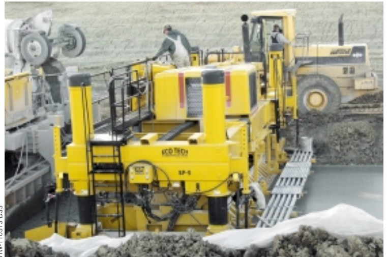
Eco Tech works on a new roadway with their new generation GP-2600. The full-width paving is slipformed with integral curb on both sides.
