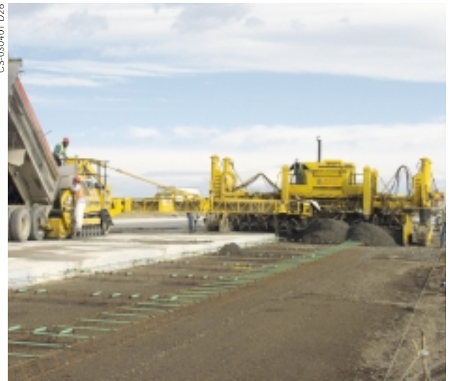
A GP-2500 is used for various paving widths on the projects entrance/exit ramps.
