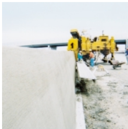
Complete General slipformed what could be the tallest section of barrier wall without steel reinforcement. The wall is 93 inches (2362 mm) tall.
