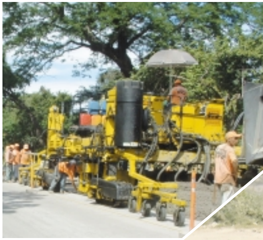
Astaldi S.P.A. (left) is at work in El Salvador on a whitetopping project with their GT-6300.
