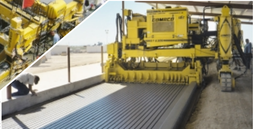
Miller Brothers dealt with some tight clearances while working on a cattle barn floor in Casa Grande, Arizona. The company used their GT-6300 to slipform the floor while applying a longitudinal groove.
