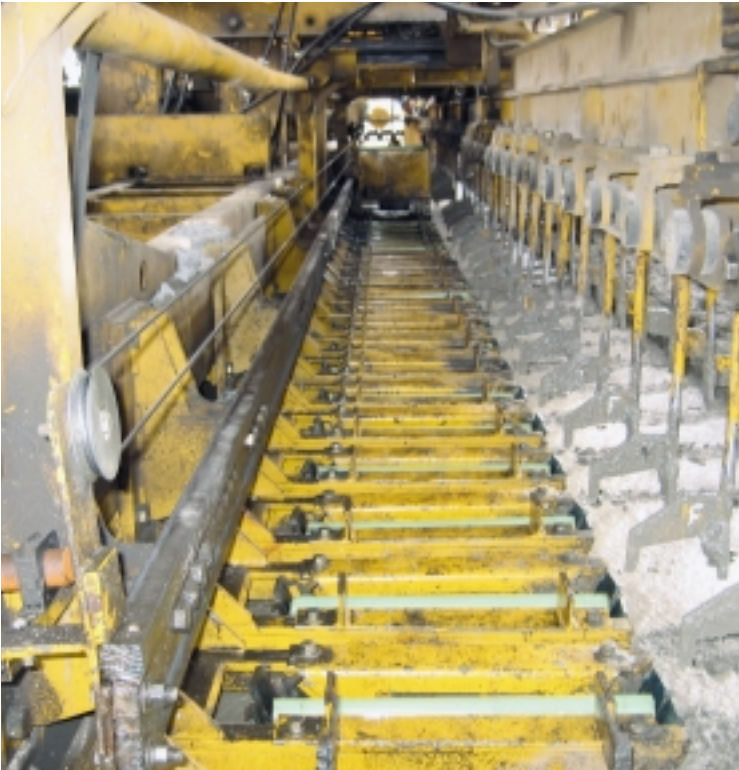
The IDBI inserts 36 bars across the width of the slab. The bars are 1.5 inch (38 mm) in diameter.
