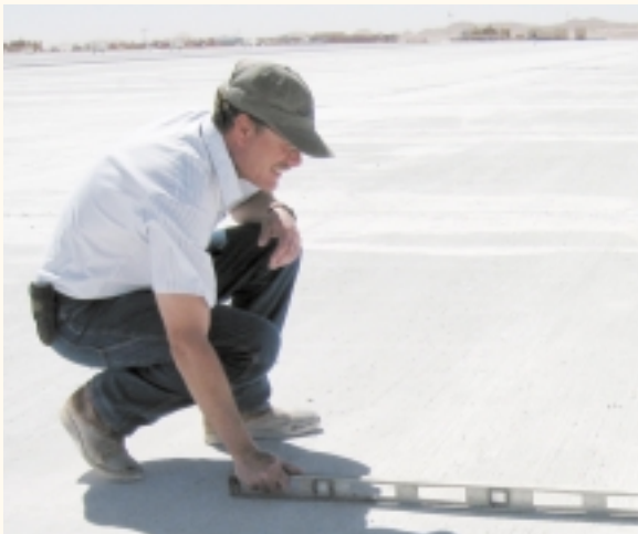
Ken Tippie checks for edge slump.
