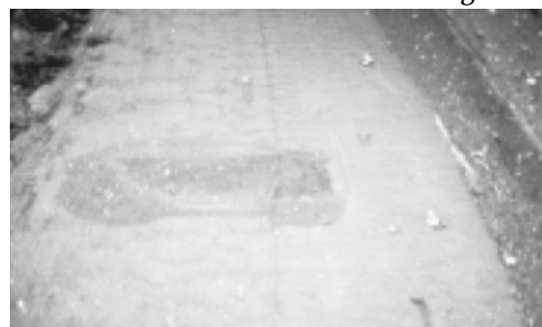
Photo #2 - excessive fine material on grade
