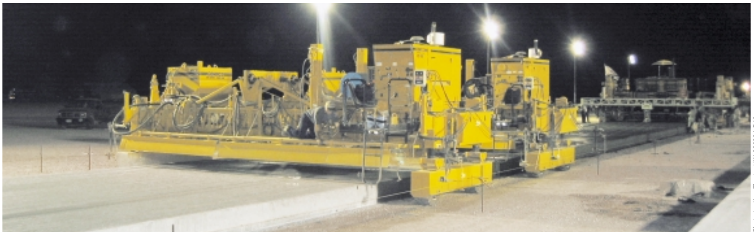
Two T/C-400s follow the paver dragging burlap and spraying the curing compound on the 16 inch (406 mm) thick slab.
