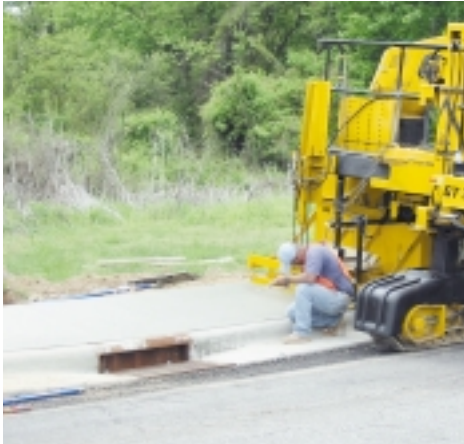
A view from the operator's platform looking down as the sensor rolls across the top of a catch basin. The photo below shows the finished sidewalk.
