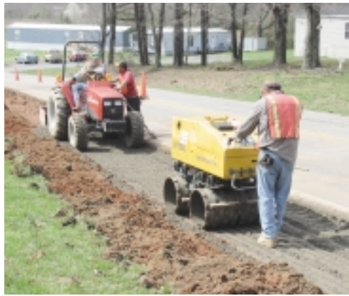
The aggregate base course is leveled out with a tractor and box blade to form the grade.
