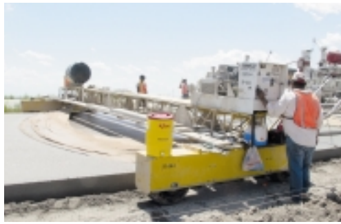
Wemhoff supervises the trimming operation. A powered Spanit® work bridge drags burlap. Spray cure is applied to the new roadway.
