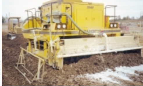
Spraying lime-stabilizing material on the grade.
