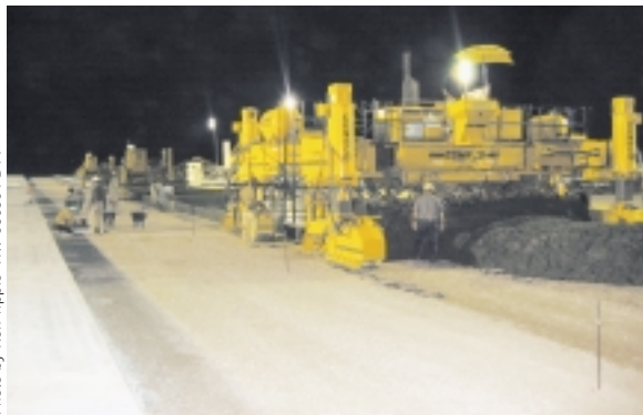
Eighty percent of the project was slipformed at night to combat the hot desert temperatures that surpassed 100° F (38° C) during the day.
