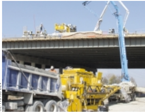
Feeding a concrete pump on a bridge deck project.
