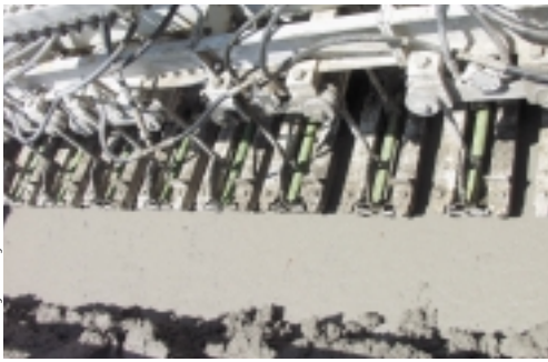
The IDBI inserts the bars into the slab.
