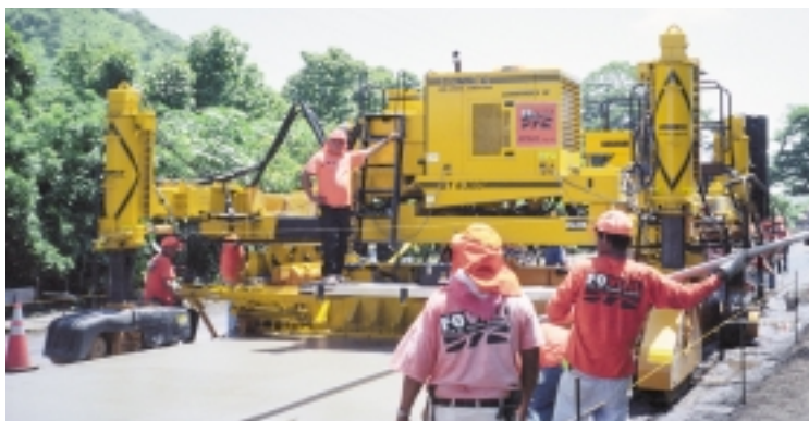
Astaldi uses their GT-6300 with high-drive track to slipform a 15.7 foot (4.8 m) pass for a new roadway near Santa Ana, El Salvador.
