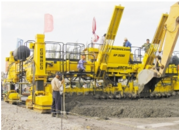
Hydropower Engineer Bureau #13 use their GP-2600 to pave a new 30 feet (9.2 m) wide, nine inch (23 mm) thick roadway connecting China to Pakistan. They are currently paving near Kashi City, in the Xinjiang province of China.
