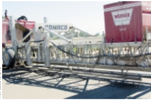
The T/C-600 applies the longitudinal tine.
