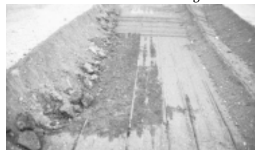
Photo #3 - chunks torn out of subgrade
