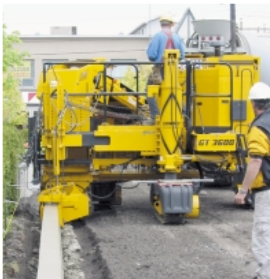
Lambert & Grenier slipform ribbon curb in tight-clearance conditions on a project in Drummondville, Quebec, Canada.
