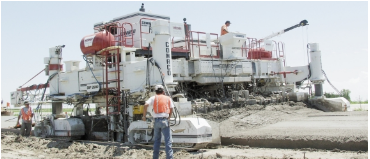
The accuracy of the IDBI was tested in several saw cut slabs. All of the bars were accurate and within the state’s specifications.
