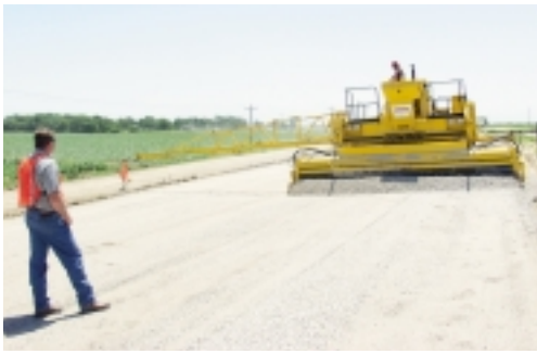
Wemhoff supervises the trimming operation. A powered Spanit® work bridge drags burlap. Spray cure is applied to the new roadway.
