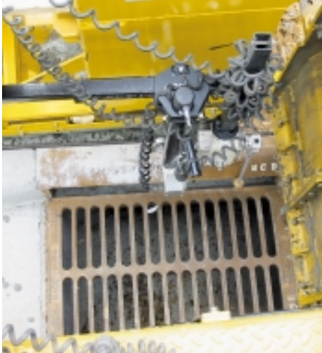
A view from the operator's platform looking down as the sensor rolls across the top of a catch basin. The photo below shows the finished sidewalk.
