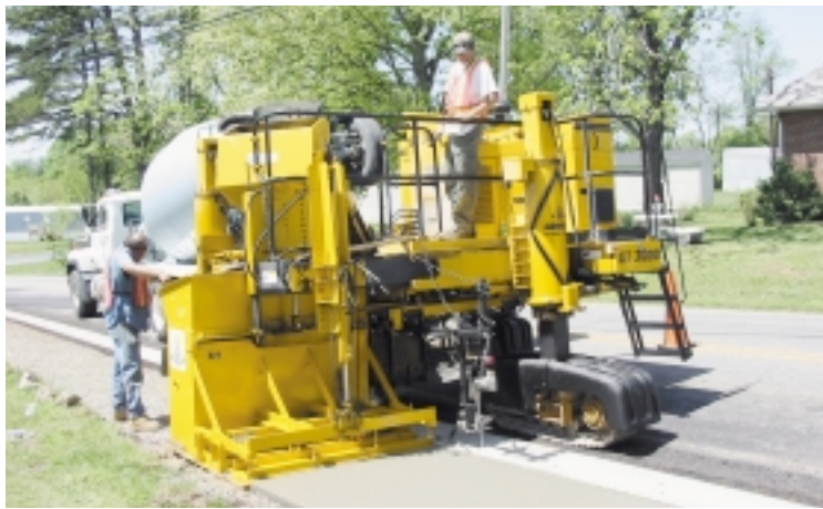
Buchanans slipformed the curb and gutter in the first phase of the project. A week after completing it, they came back with their sidewalk mold and tackled their stringless challenge.
