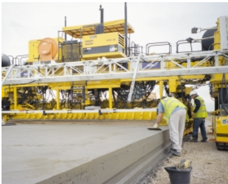
AMEC slipforms a slab 25.6 inches (650 mm) thick as part of a test pour at the Heathrow Airport in London, England.
