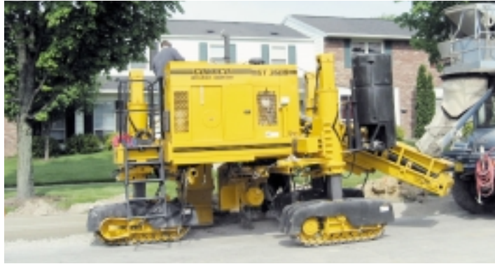
Hipskind Concrete has more than tripled their curb and gutter production since adding a GT-3600 to their operation last year.
