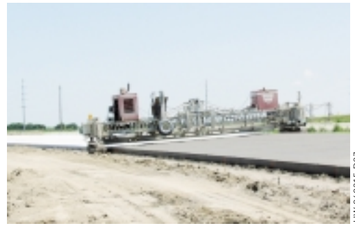
Wemhoff supervises the trimming operation. A powered Spanit® work bridge drags burlap. Spray cure is applied to the new roadway.
