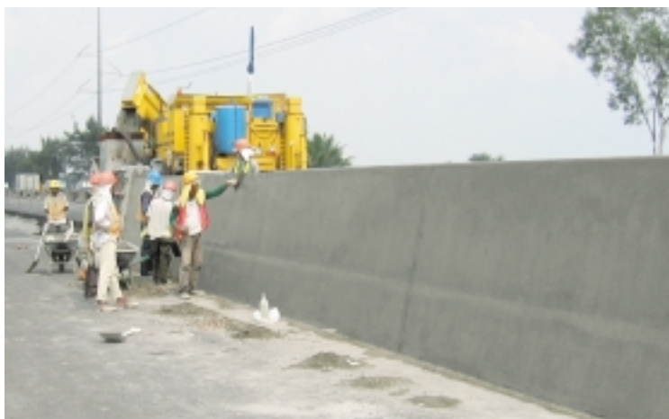
Meltreach Proprietary Ltd. is the slipform contractor on the first ever slipformed barrier in the Philippines. They are using their GT-6300 to slipform wall as tall as 6.1 feet (1.85 m). Meltreach has approximately 12.4 miles (20 km) of the Texas-type barrier to slipform on the North Luzon Tollway near Manila for the project's main contractor, Leighton Asia.
