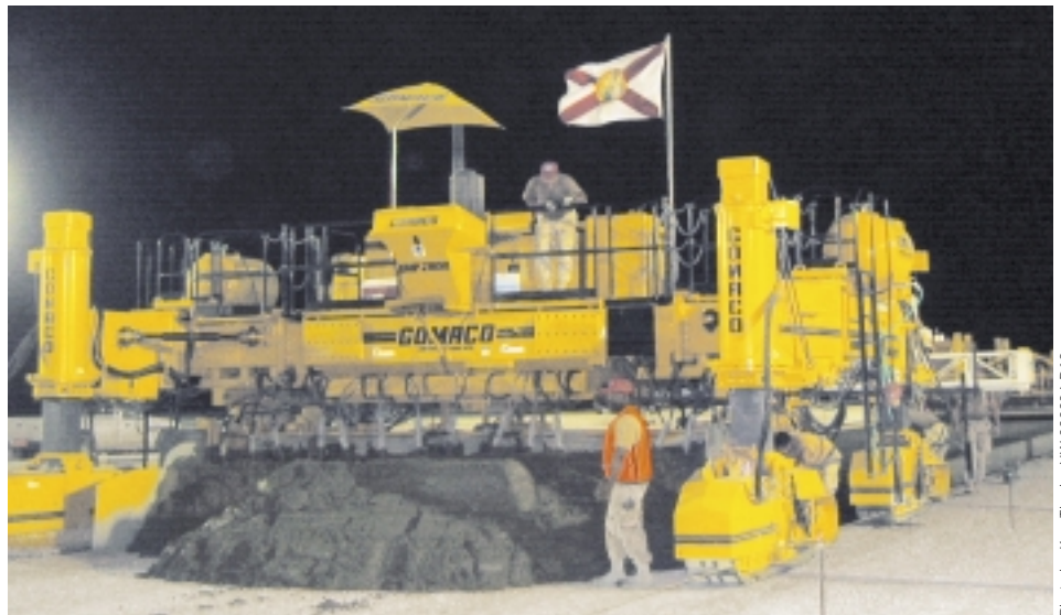
Eighty percent of the project was slipformed at night to combat the hot desert temperatures that surpassed 100° F (38° C) during the day.
