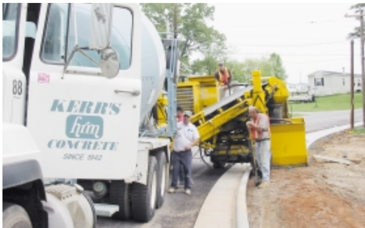
The trimmerhead was sideshifted and vertically lifted out of the way while the sidewalk was slipformed.
