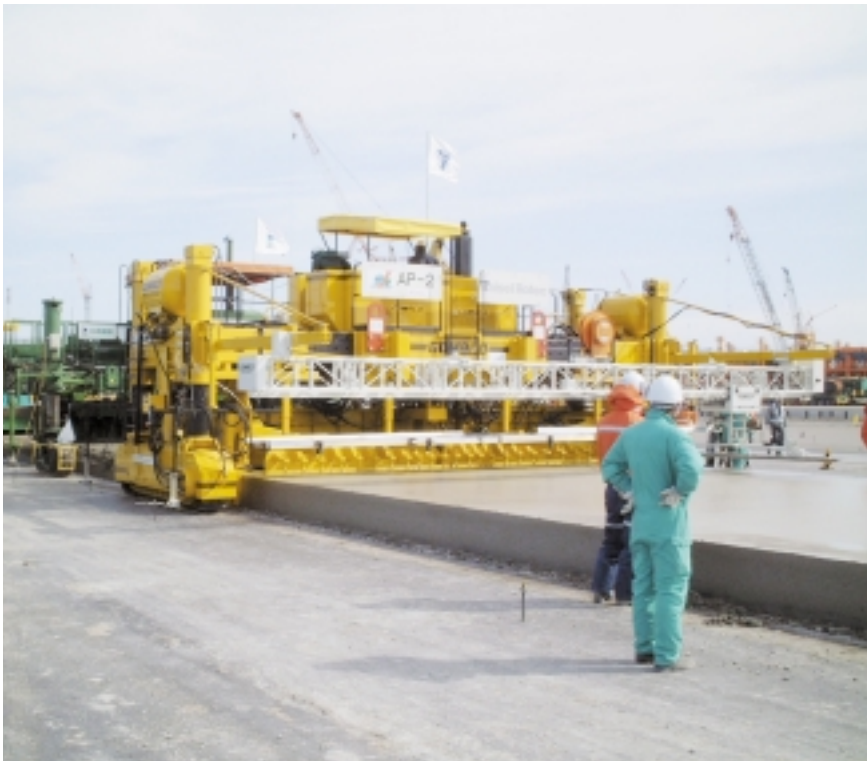
The GHP-2800 impressed Japanese officials and had no problems with edge slump on a test project for the new international Chubu airport near Nagoya, Japan. Each paving pass is 24.6 feet (7.5 m) wide and 18 inches (460 mm) thick.
