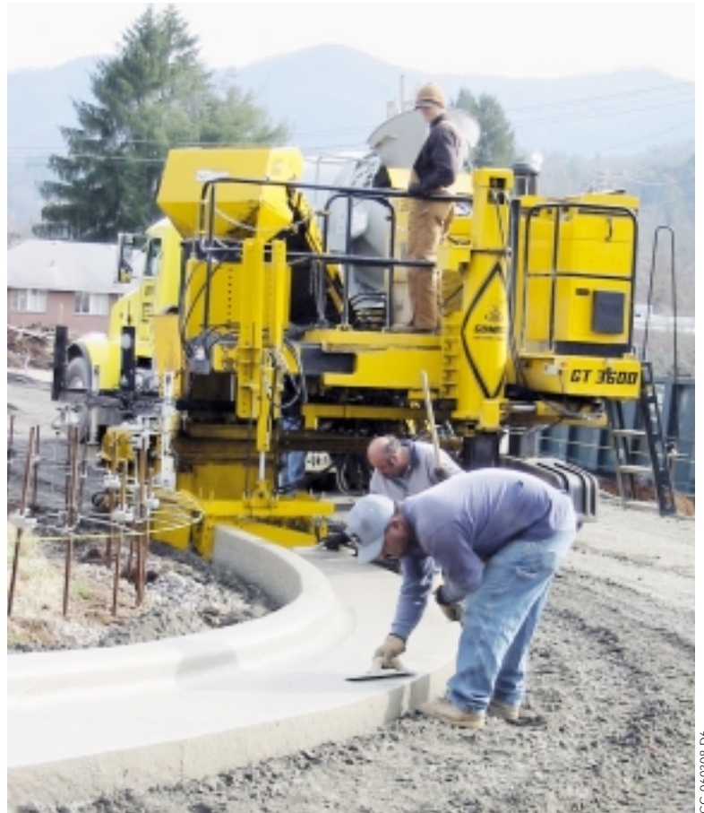
Buchanans slipformed the curb and gutter in the first phase of the project. A week after completing it, they came back with their sidewalk mold and tackled their stringless challenge.
