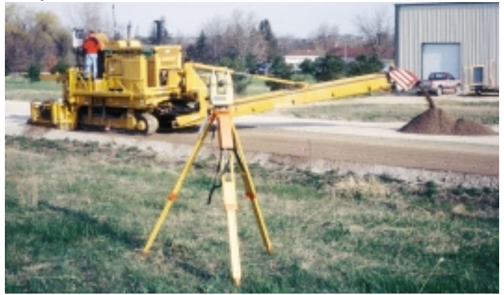
A 9000 trimmer is controlled by the Laser Alignment stringless guidance system as it trims grade on a project near Panora, Iowa.
