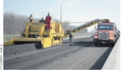
Picking up windrowed asphalt off the grade.
