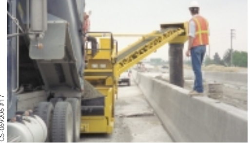
Placing rock over a barrier wall for subgrade.
