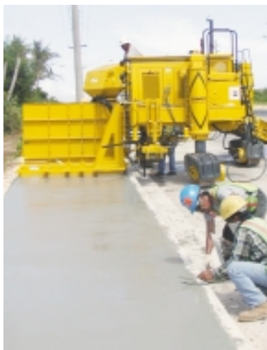
Giant Construction Guam slipforms four inch (102 mm) thick, 7.5 feet (2.3 m) wide sidewalk on a project in front of the Micronesia Mall in Guam.
