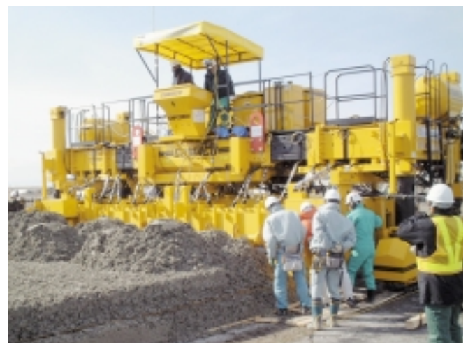
The GHP-2800 impressed Japanese officials and had no problems with edge slump on a test project for the new international Chubu airport near Nagoya, Japan. Each paving pass is 24.6 feet (7.5 m) wide and 18 inches (460 mm) thick.
