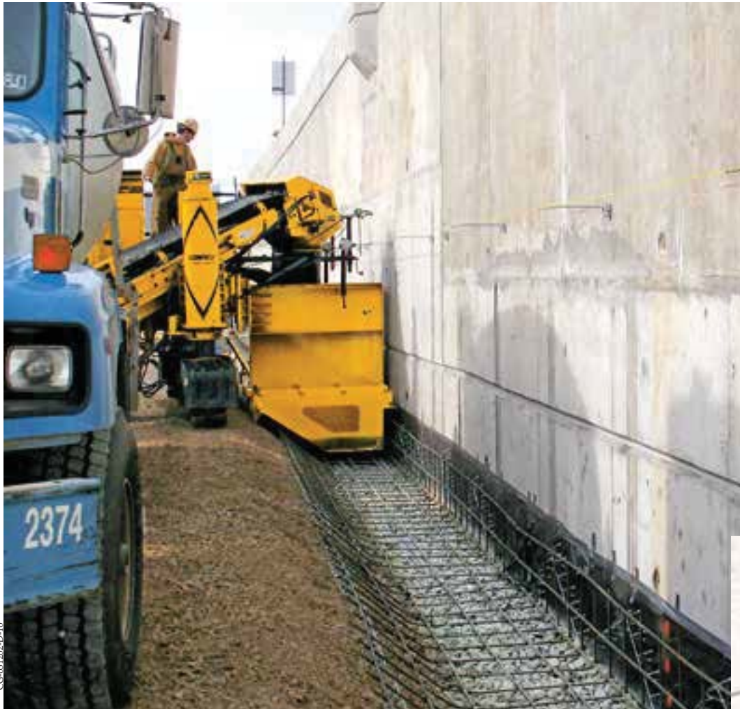
A GT-3600 slipforms a drainage channel for water to run off the bridge. The GT-3600 is slipforming up against a wall. The stringline holders have been mounted to the wall, so the GT-3600 will follow the wall profile.
