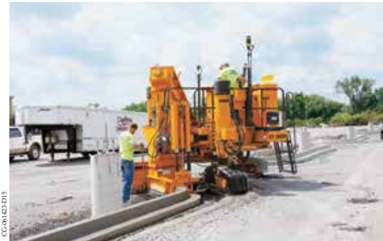
Sixteen islands and one longer island design in the center of this parking lot project were paved the first day on the job. This was also the first day the contractor paved with Topcon 3D guidance, integrated with the GOMACO G+ control system on their GOMACO GT-3600 curb and gutter machine.
