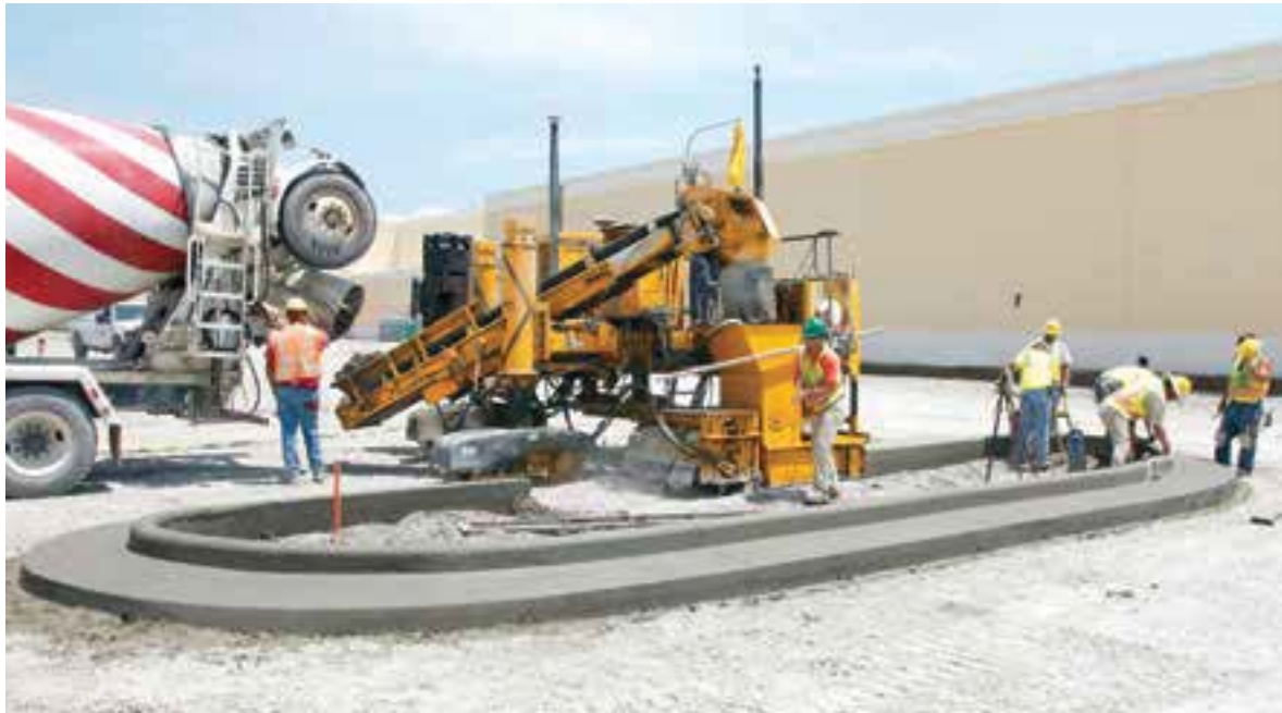
The GT-3600 equipped with the Leica Geosystems 3D guidance slipforms the tight radii of parking lot islands with ease after having loaded the hopper and charging conveyor prior to starting the island.
