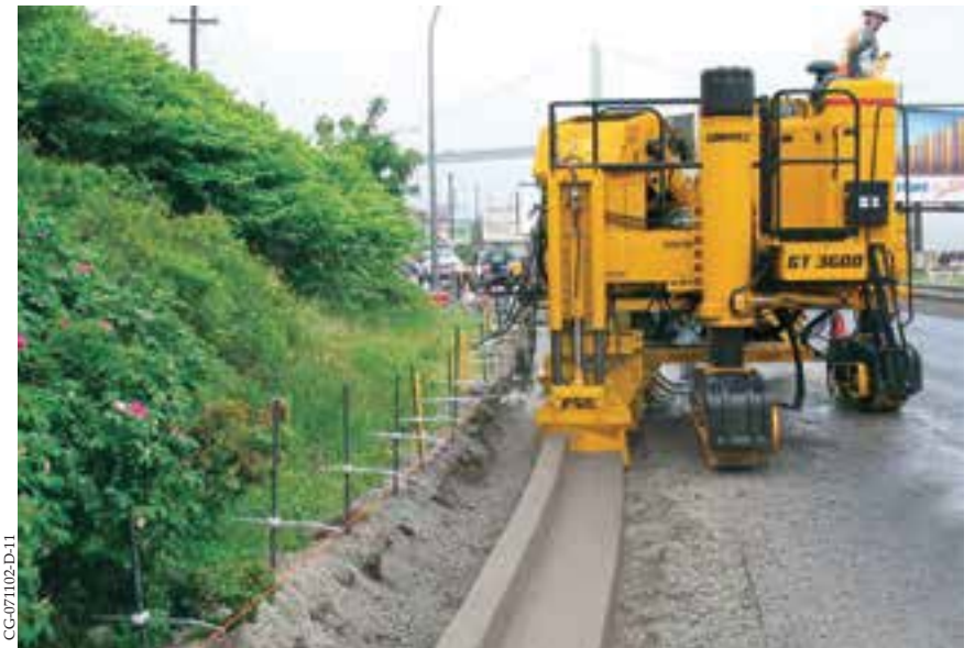
This GT-3600 slipforms curb and gutter next to traffic on a road in Canada.
