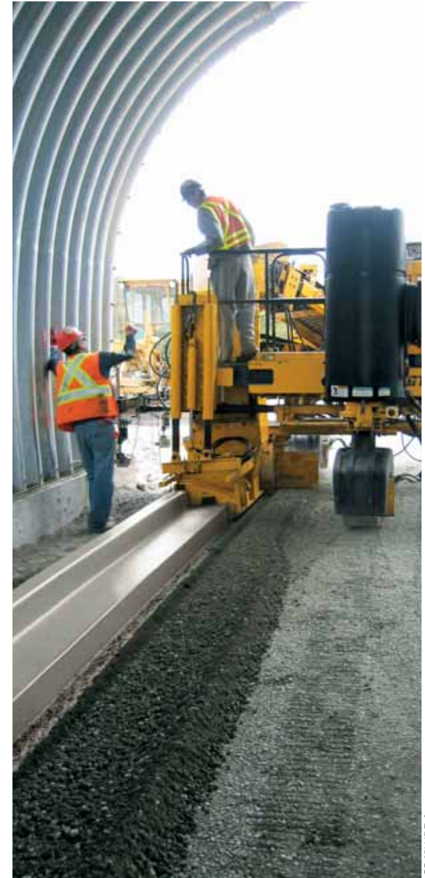
The GT-3600's compact paving width makes it an ideal machine for working within confined spaces, like this tunnel project in Canada.
