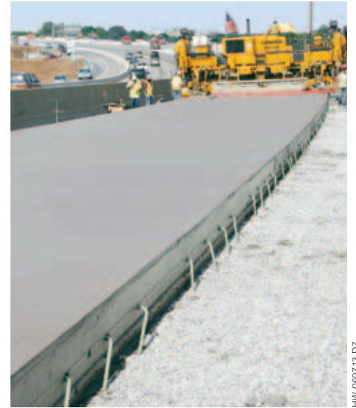
All of the concrete pavement on the project was 16 inches (406 mm) thick.
