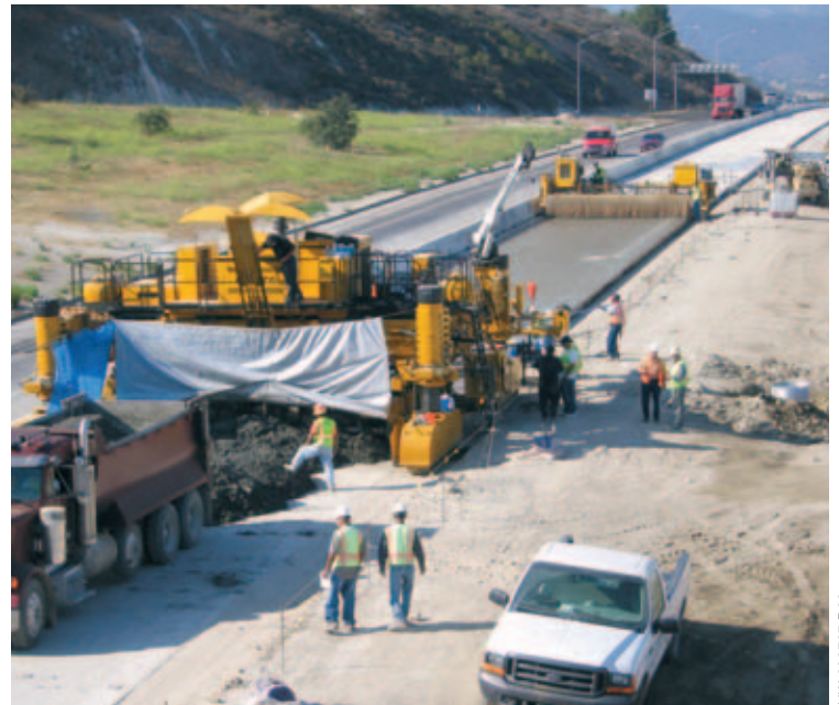
Production averaged approximately 2000 cubic yards (1529 m 3 ) per eight hour shift under live traffic.
