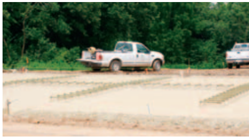
The tank crossing has extra steel reinforcing and thicker concrete.
