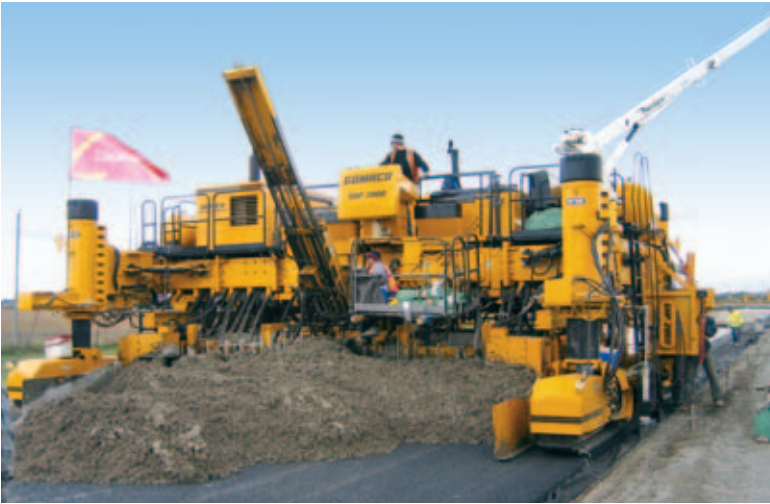
Coco Paving is slipforming a new section of Highway 401 with their four-track GHP-2800 paver equipped with an In-The-Pan-Dowel Bar Inserter (IDBI) near Windsor, Ontario, Canada.
