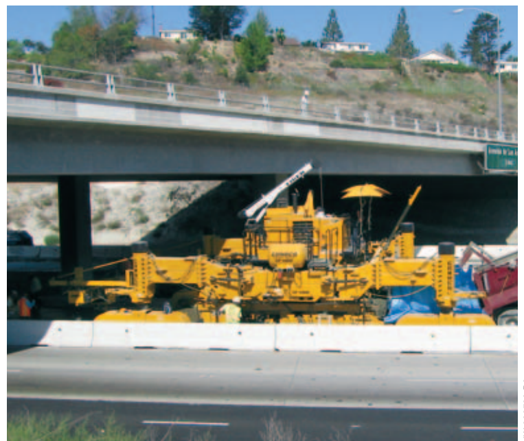
Security Paving’s GP-4000 four-track paver with IDBI slipforms underneath a bridge overpass on Highway 23.
