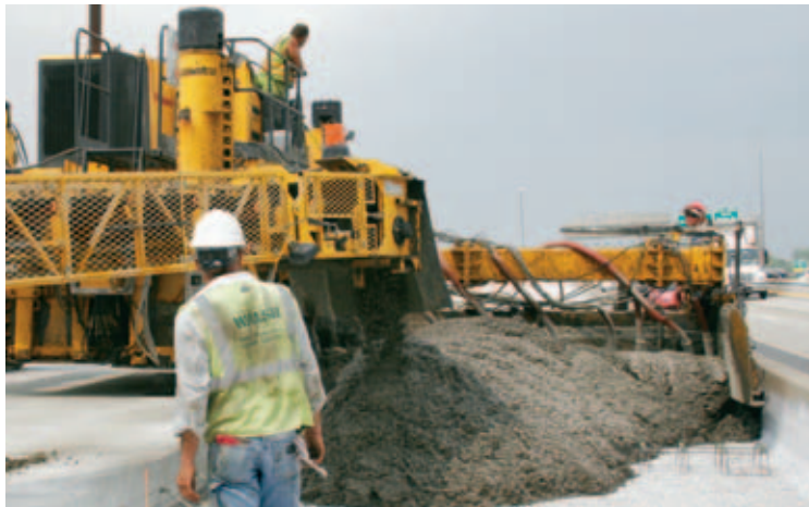
An RTP-500 placed concrete on the grade over baskets in front of the Commander III’s side-mounted mold.
