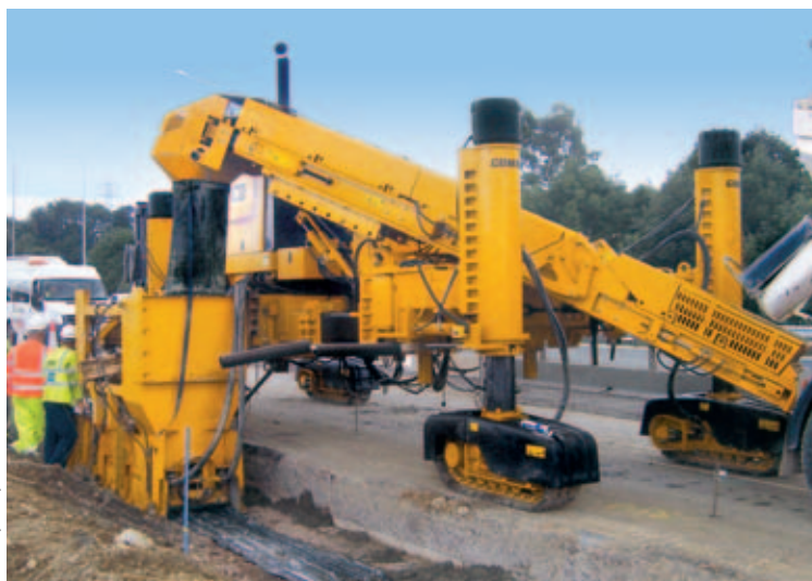
The Commander III’s hydraulically folding conveyor is positioned for slipforming right-side slot drain on the M1.
