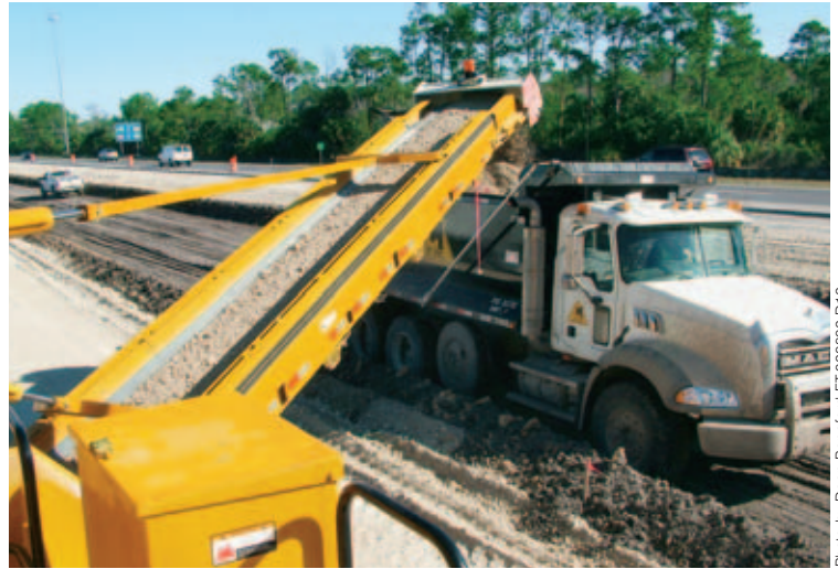
The 9500's long-reaching placing belt, over 34 feet (10.6 m) long, conveys the trimmed material into an awaiting dump truck.
