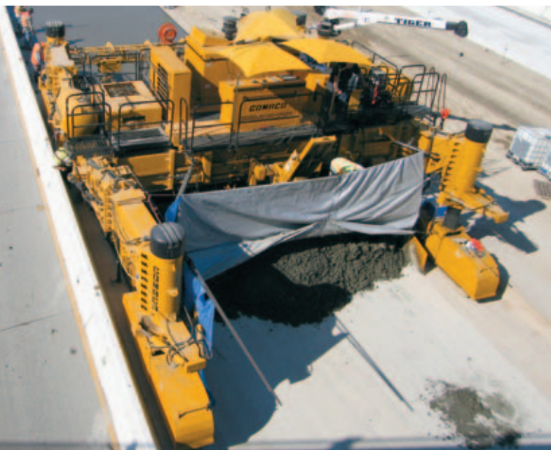
Pivoting leg extensions allowed Security to place the GP-4000’s tracks in their optimum position for the project’s tight conditions.
