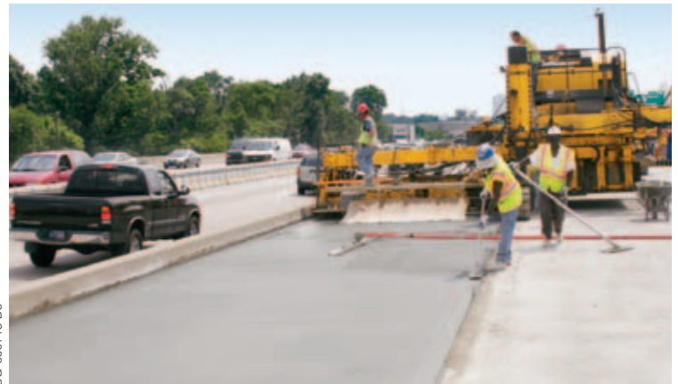
The company kept their 12 foot (3.7 m) paving package mounted underneath the Commander III while they paved with their side-mounted 14 foot (4.3 m) zero-clearance mold.
