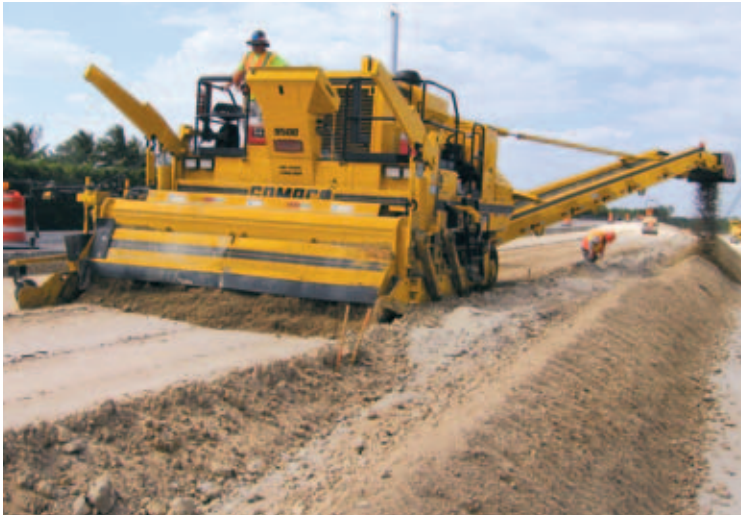
Two trimming passes, each 12 feet (3.7 m) wide, form two new lanes of traffic making Interstate 75 six lanes wide.
