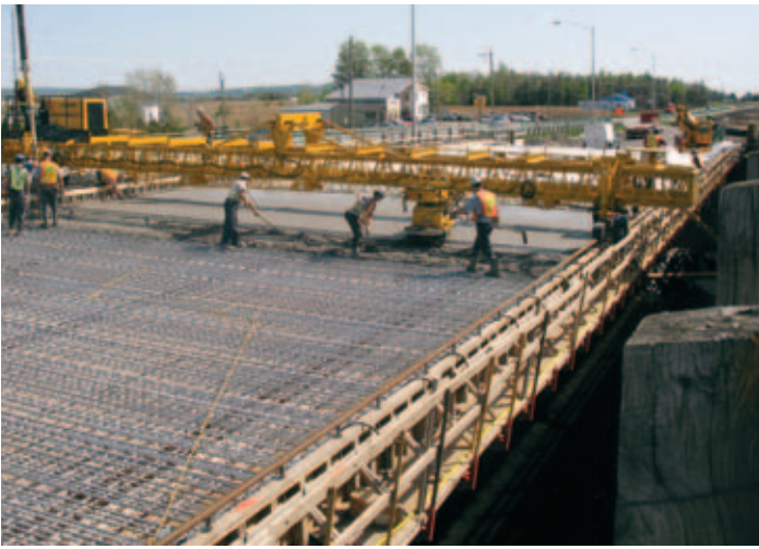
Lambert & Grenier finish a bridge deck 225 feet (68.6 m) long, 44.5 feet (13.6 m) wide with their new GOMACO C-450 in Victoriaville, Quebec, Canada.
