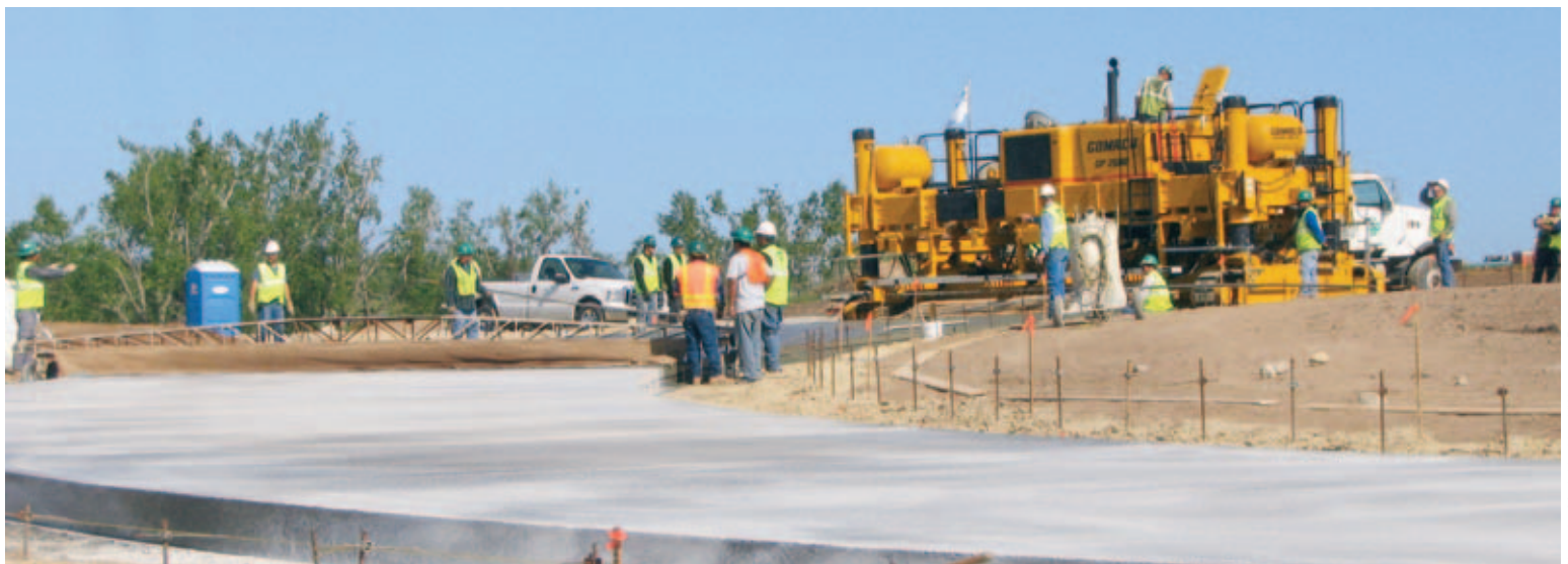
Smoky Hill’s first project with their new GP-2600 paver was slipforming a roundabout with a 100 foot (30.5 m) radius.
