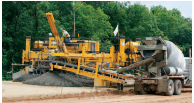
The conveyor system features a belt that can be extended for concrete placement and then retracted to allow room for the trucks to pass.
