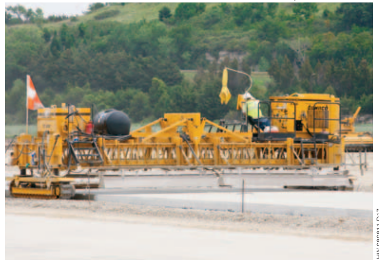
A T/C-600 followed the paver applying a white spray cure.
