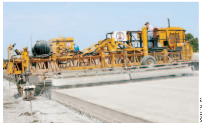
A GOMACO T/C-600 texture/cure machine applied a transverse tine and white spray cure.
