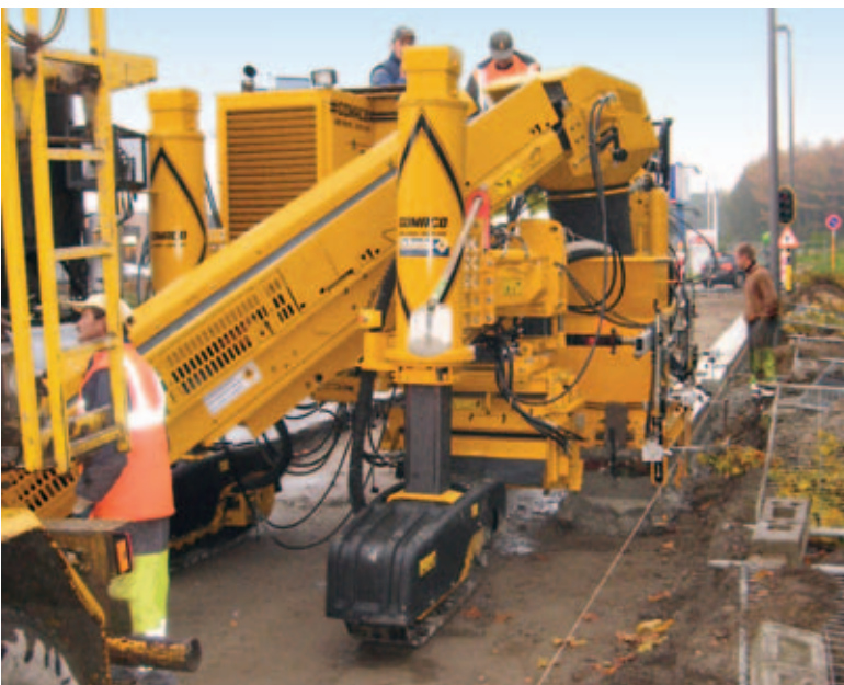
Heijmans Infras slipforms curb and gutter with their new GT-3600 on a project in Sint-Niklaas, Belgium.
