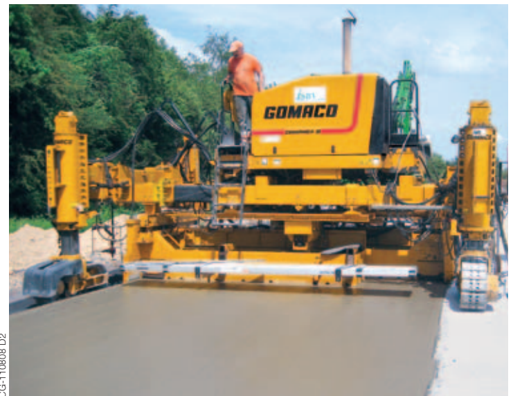
TSBV use their four-track Commander III with V2 mold on a parking lot in Soumagne, Belgium. Paving passes were five meters (16.4 ft) wide, 250 millimeters (9.8 in) thick.
