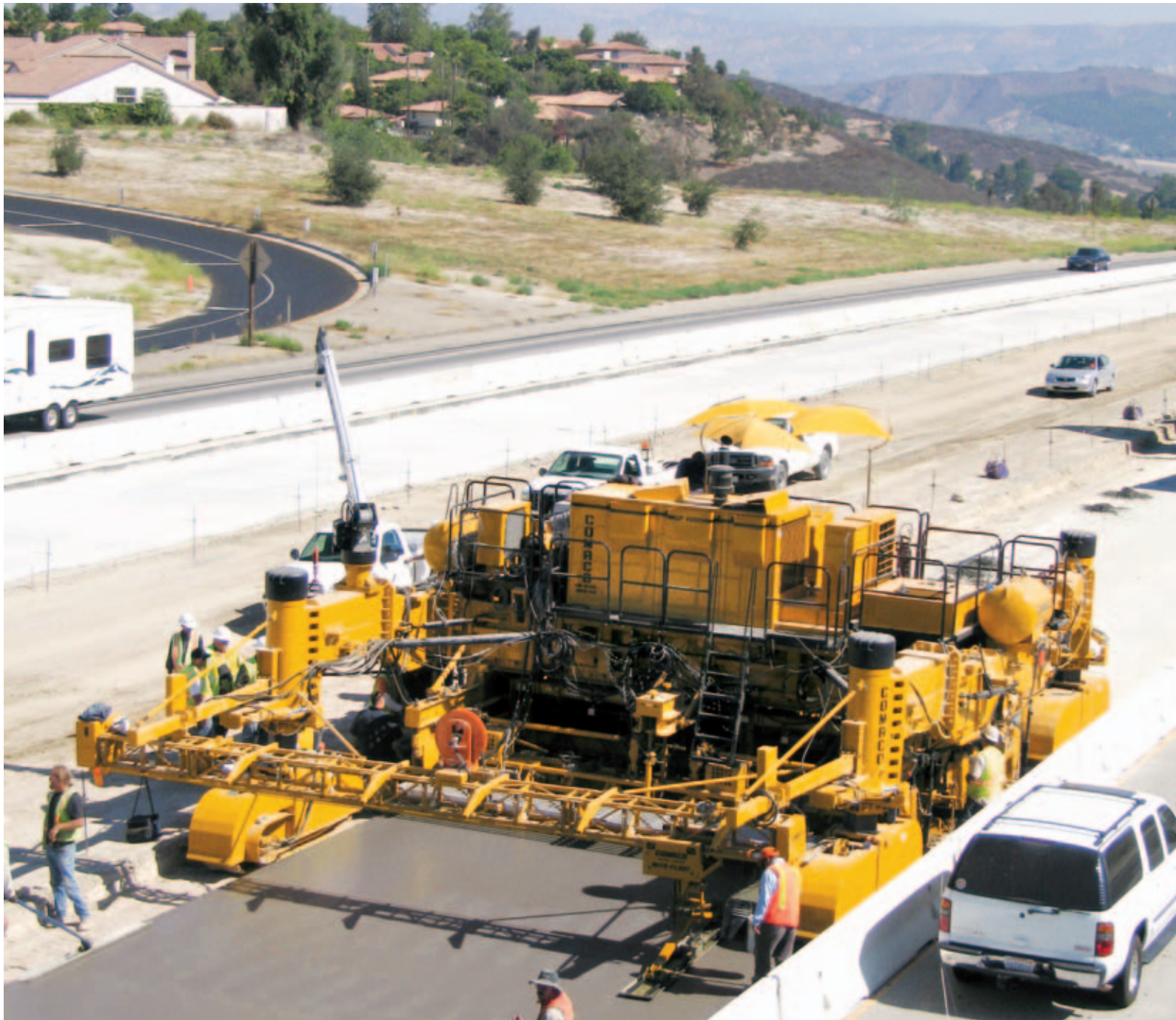
The GP-4000's right tracks had to run on the existing edge of highway and some areas were only 22 inches (559 mm) wide.
