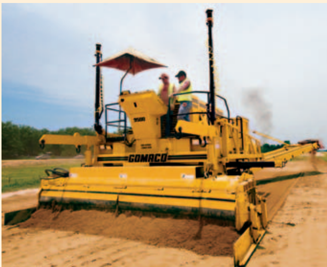
Weaver Bailey's 9500 trims stringless with the Topcon Millimeter GPS™ 3-D machine control system.
