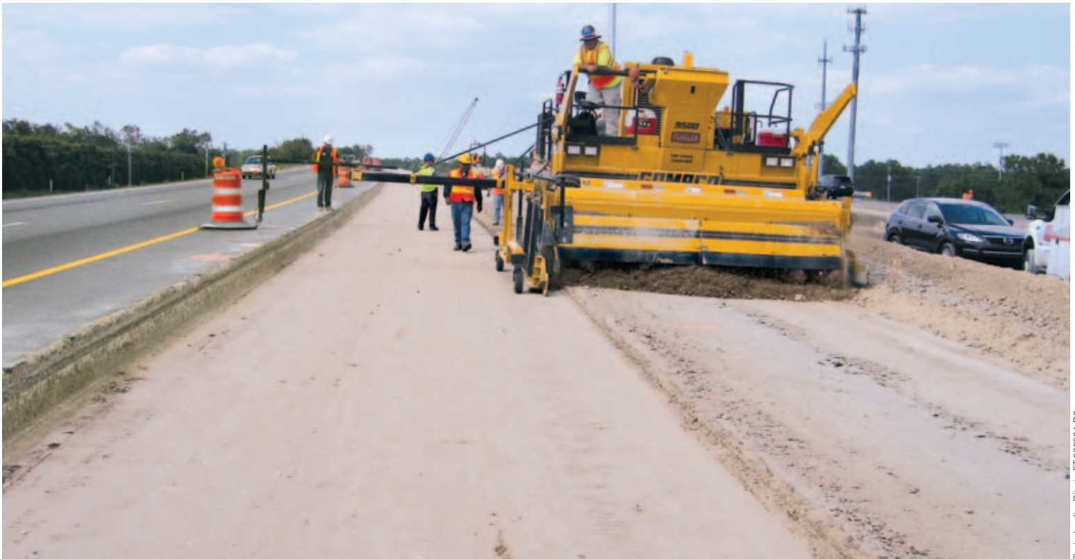
LeeMar used their 9500's built-in sensor arm boom to reference steering off the existing slab. Elevation was controlled with a rolling grade ski running on the trimmed grade.
