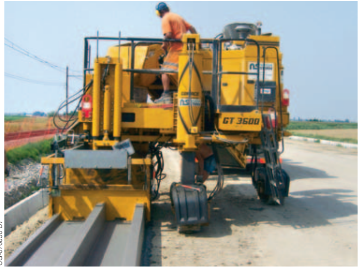
Nuove Strade Srl use their GT-3600 to slipform a unique profile for electric cables and pipes along what will be a new railway connecting Bologna to Verona, Italy.
