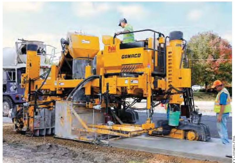
GOMACO's Next Generation Commander III, three-track, trims and paves a five foot (1.5 m) wide sidewalk.
