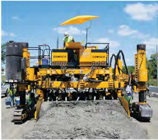
A GOMACO four-track Next Generation Commander III paves a new highway.
