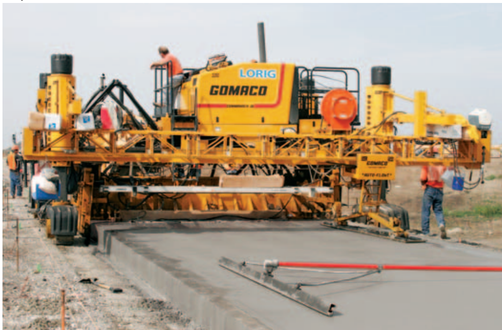
The Commander III is slipforming the new ramp 16 feet (4.9 m) wide and 12 inches (305 mm) thick.
