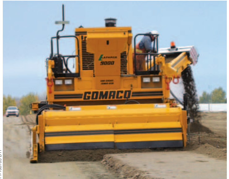
LaFarge Construction Materials trims a new roadway project to grade with their GOMACO 9000 with monolithic trimmerhead in Calgary, Alberta, Canada.
