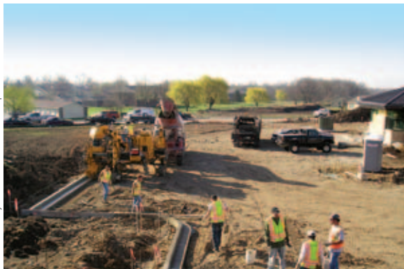
Black Diamond slipforms as much of the project as possible, even the tight radii with their GT-3600.
