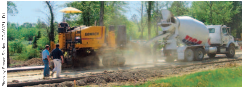
A Ready Mix USA truck feeds one of the 92 nine cubic yard (6.9 m 3 ) loads of concrete onto the belt of Shirley’s Commander III.
