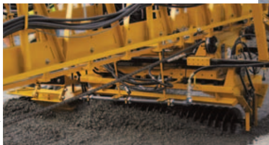
A close-up of the auger spreading the lean concrete base material.
