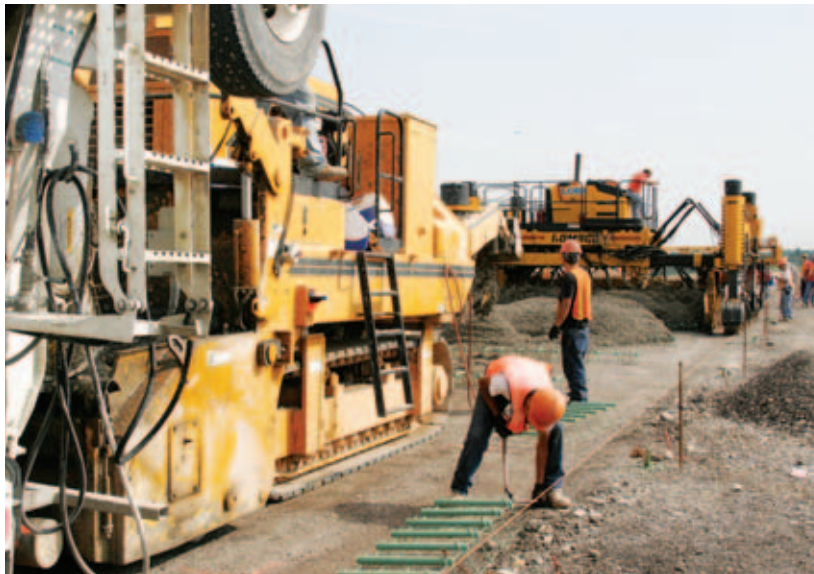
Tight conditions on the project require a 9500 placing concrete, with workers setting baskets on grade behind the 9500, directly in front of the four-track Commander III.
