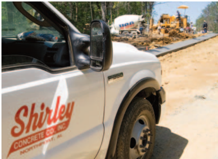
Shirley Concrete slipformed 16,357 linear feet (4986 m) of valley gutter in nine hours and 23 minutes.
