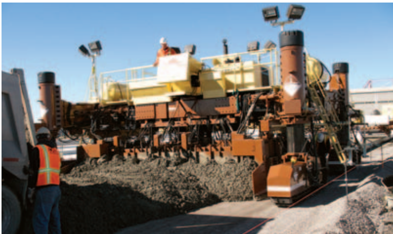
Miller Paving Ltd. slipforms a new airport parking lot in Toronto, Ontario, Canada. Their four-track GHP-2800 is slipforming 24 feet (7.3 m) wide on 2000 foot (610 m) long paving passes.
