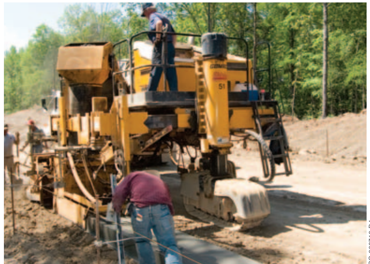
Their Commander III slipformed 828 cubic yards (633 m 3 ) of concrete during the pour.
