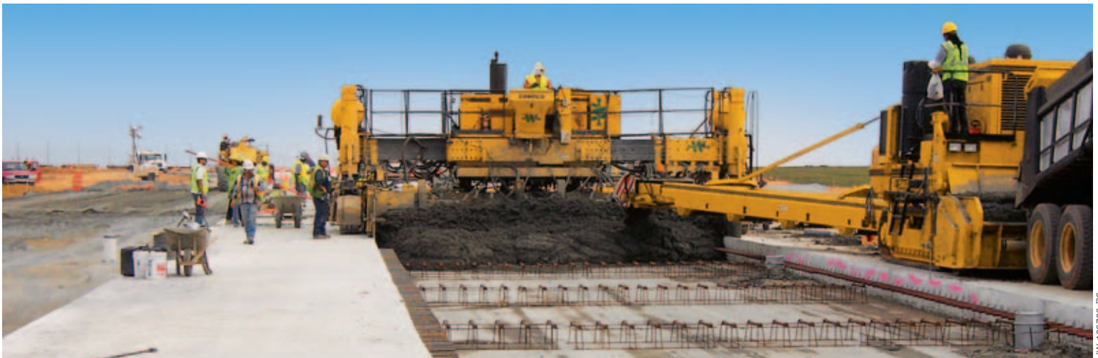
The new Taxiway V is 130 feet (39.6 m) wide, 4200 feet (1280 m) long and 20 inches (508 mm) thick.
