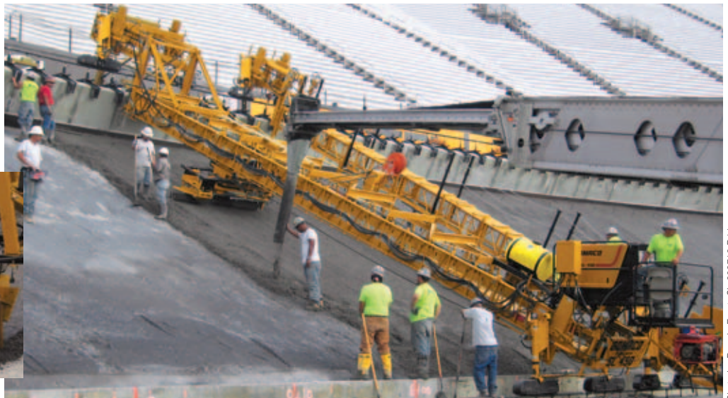
The SL-450, with a seven inch (178 mm) lowering kit on the drum, finishes the track's lean concrete base. It was also equipped with an auger to give the surface a rougher finish.
