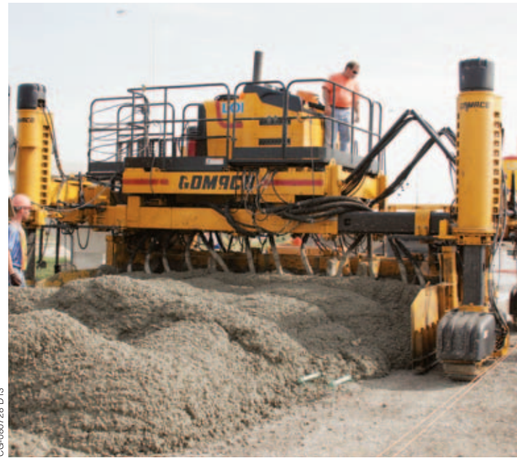
Tight conditions on the project require a 9500 placing concrete, with workers setting baskets on grade behind the 9500, directly in front of the four-track Commander III.
