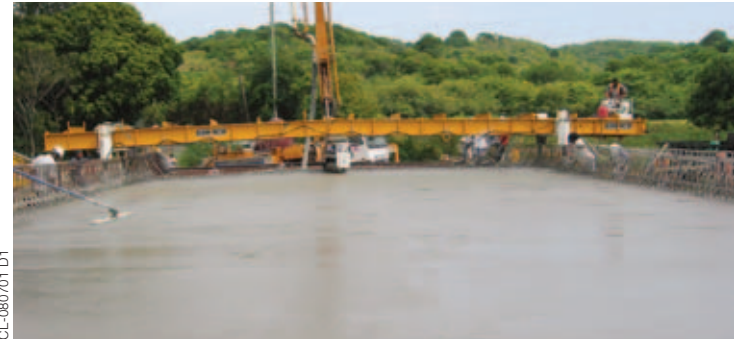
Virgin Island Paving in St. Croix, Virgin Islands, finish a new bridge deck on the island with their older style C-450.
