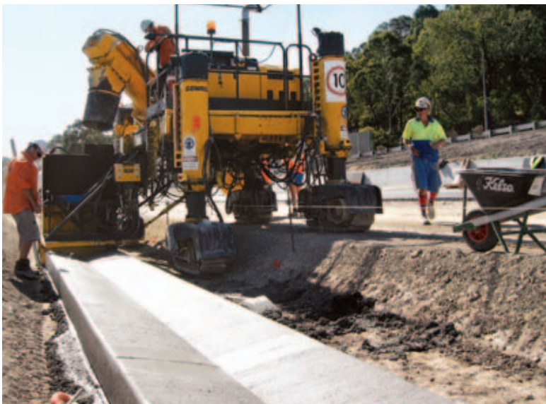
ABI Group Ltd. utilizes the versatility of their Commander III's track placement to slipform drainage canal in Australia.
