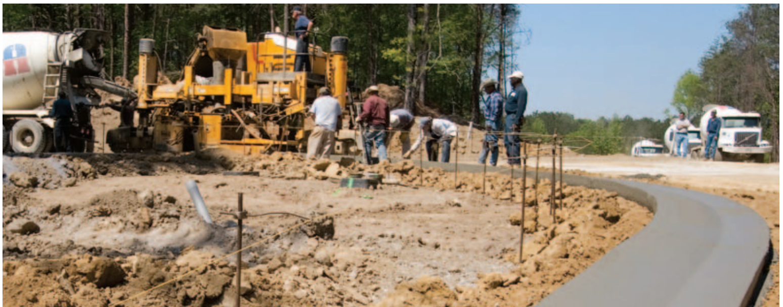
The project included seven cul de sacs, 26 radii that were 25 feet (7.6 m), and 42 inlets that all had to be dealt with during the pour.
