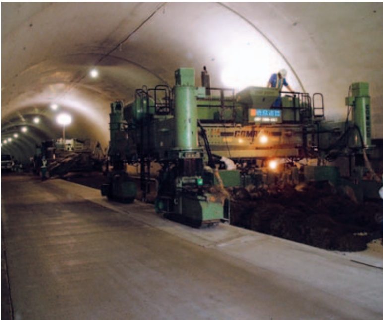
Joint partners K-Con Company and Kajima Road Company Ltd., slipform a new highway inside of the Ayabe Road Tunnel in Kyoto, Japan. They are using their four-track GHP-2800 and Commander III to complete the paving on the project.
