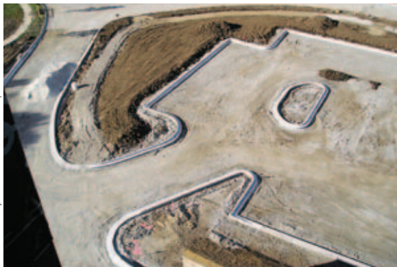
Photos from the roof of the new hospital show the challenging parking lot design.
