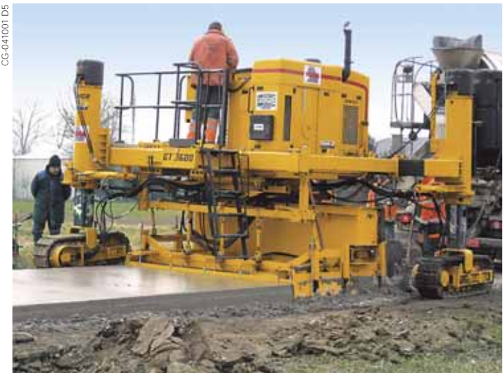
WEMA slipforms a three meter (9.8 ft) wide recreational path in Aalst, Belgium. Their GT-3600 features G22 controls with both English and Dutch languages.
