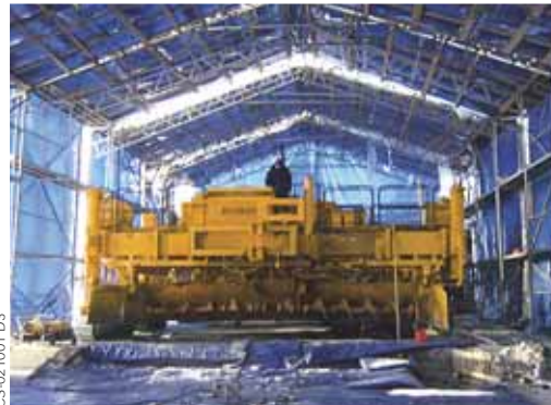
A temporary tent structure with heated mats on grade was set up at Russia's Vnukovo Airport so paving could continue throughout the cold temperatures of winter.
