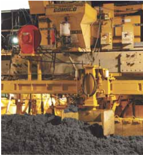
A spreader plow, mounted to the T-rail, moves the concrete across the width of the paver.
