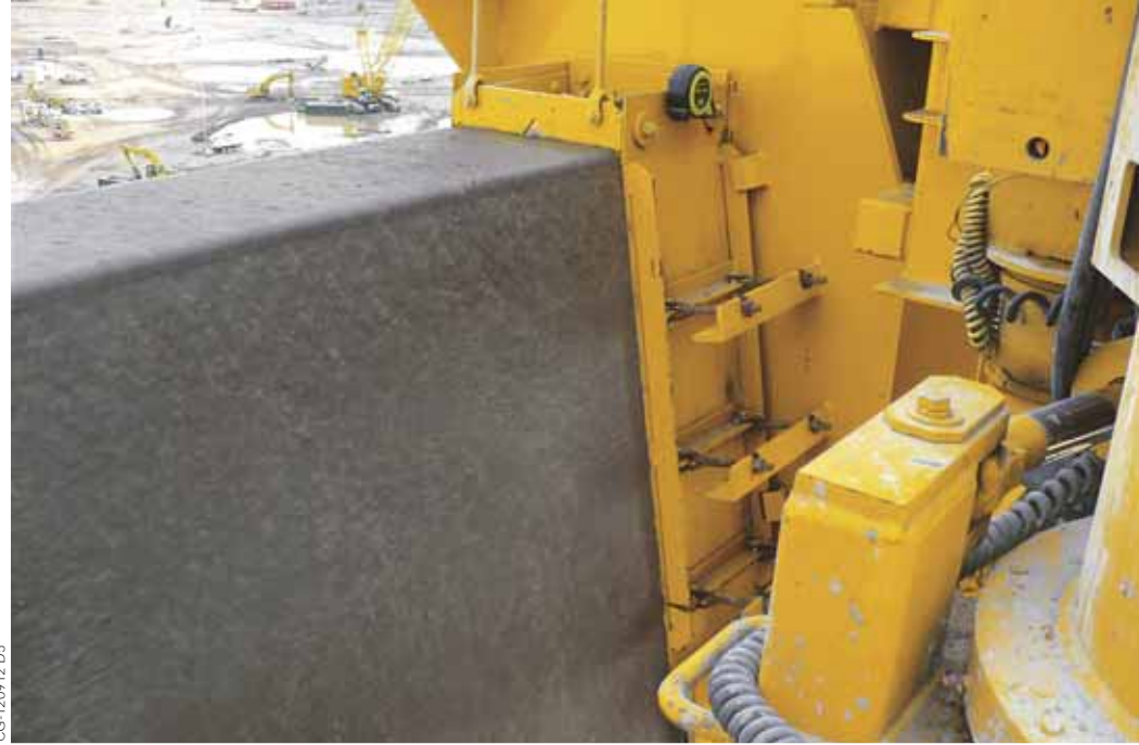
Gerdan's three-track Commander III slipformed approximately 5743 lineal feet (1750 m) of 42 inch (1067 mm) tall barrier wall on the project.
