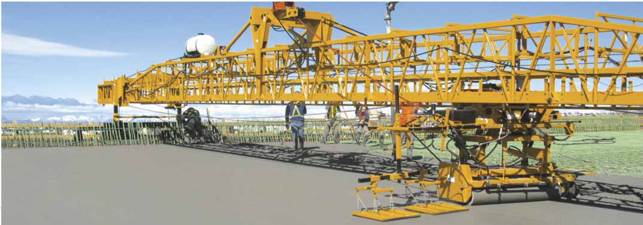
Graham finishes one of two side-by-side bridge decks on Highway 2 near Airdrie, Alberta, Canada, with their GOMACO C-450 finisher with transitional framework.
