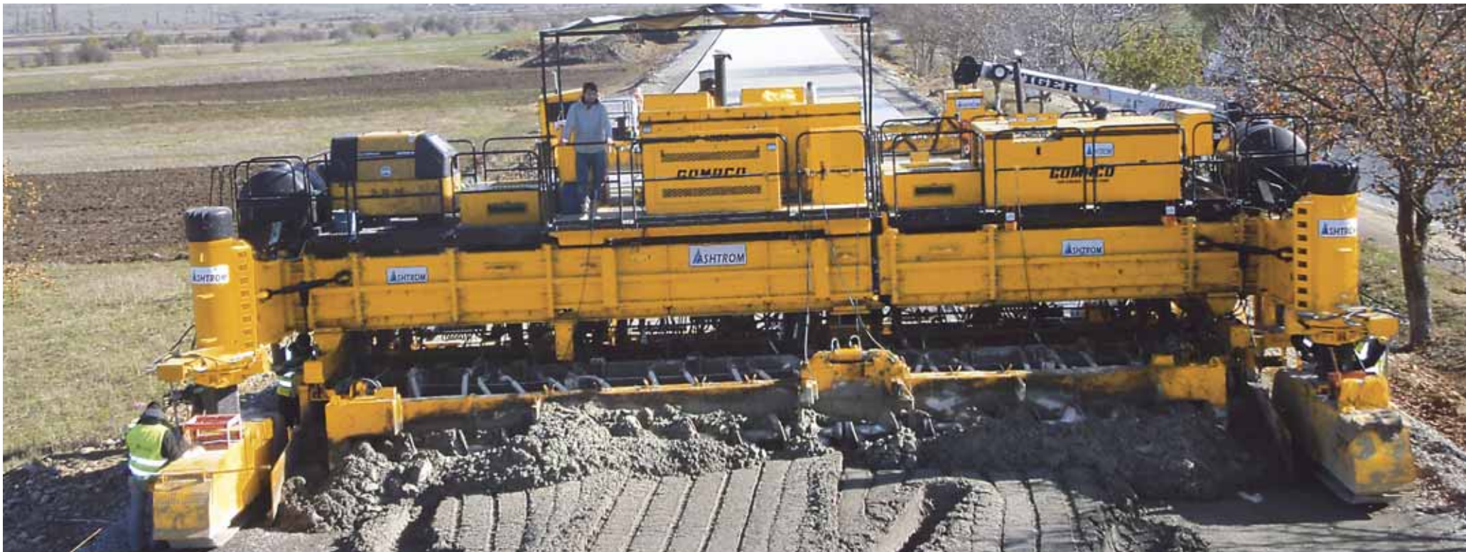
Ashtrom International slipformed a new portion of the E60 East-West Highway with their new GOMACO GP-4000 paver and T/C-600 texture/cure machine.
