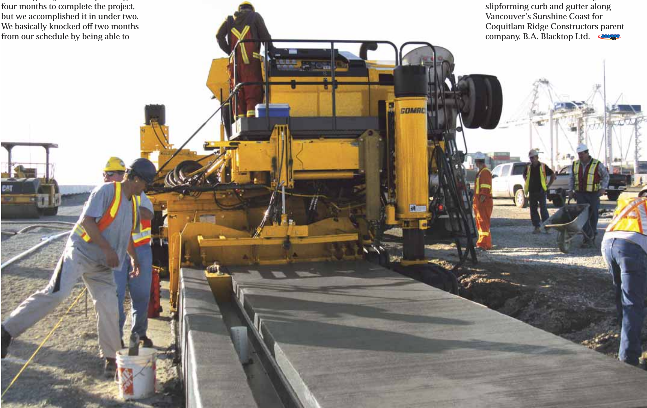
A slot drain insert with a male keyway was added to the basic rectangular mold to create an area for drainage water to run in the new concrete crane runways.
