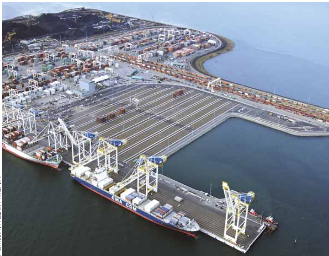
Container ships dock and wait to be unloaded at Vancouver, British Columbia, Canada's, new Deltaport third berth. A Commander III slipformed new concrete runways for the overhead gantry cranes to operate on.
