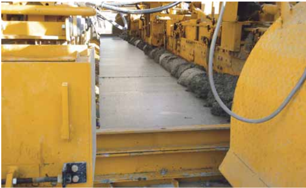
The IDBI on the GP-4000 inserted 28 bars into the slab every five meters (16.4 ft).
