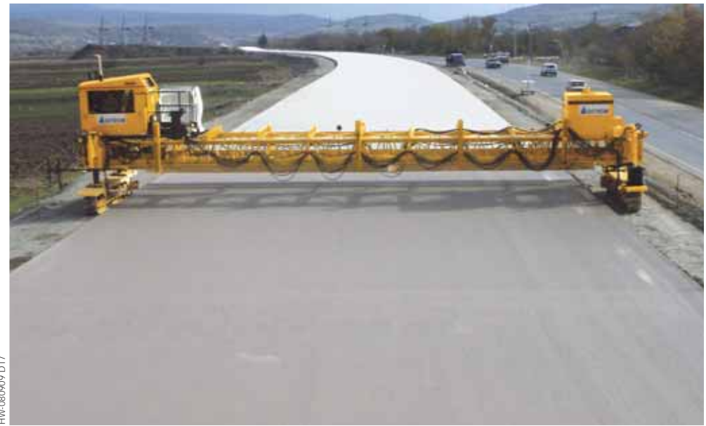
A T/C-600 texture/cure machine followed the paver applying a white curing compound.
