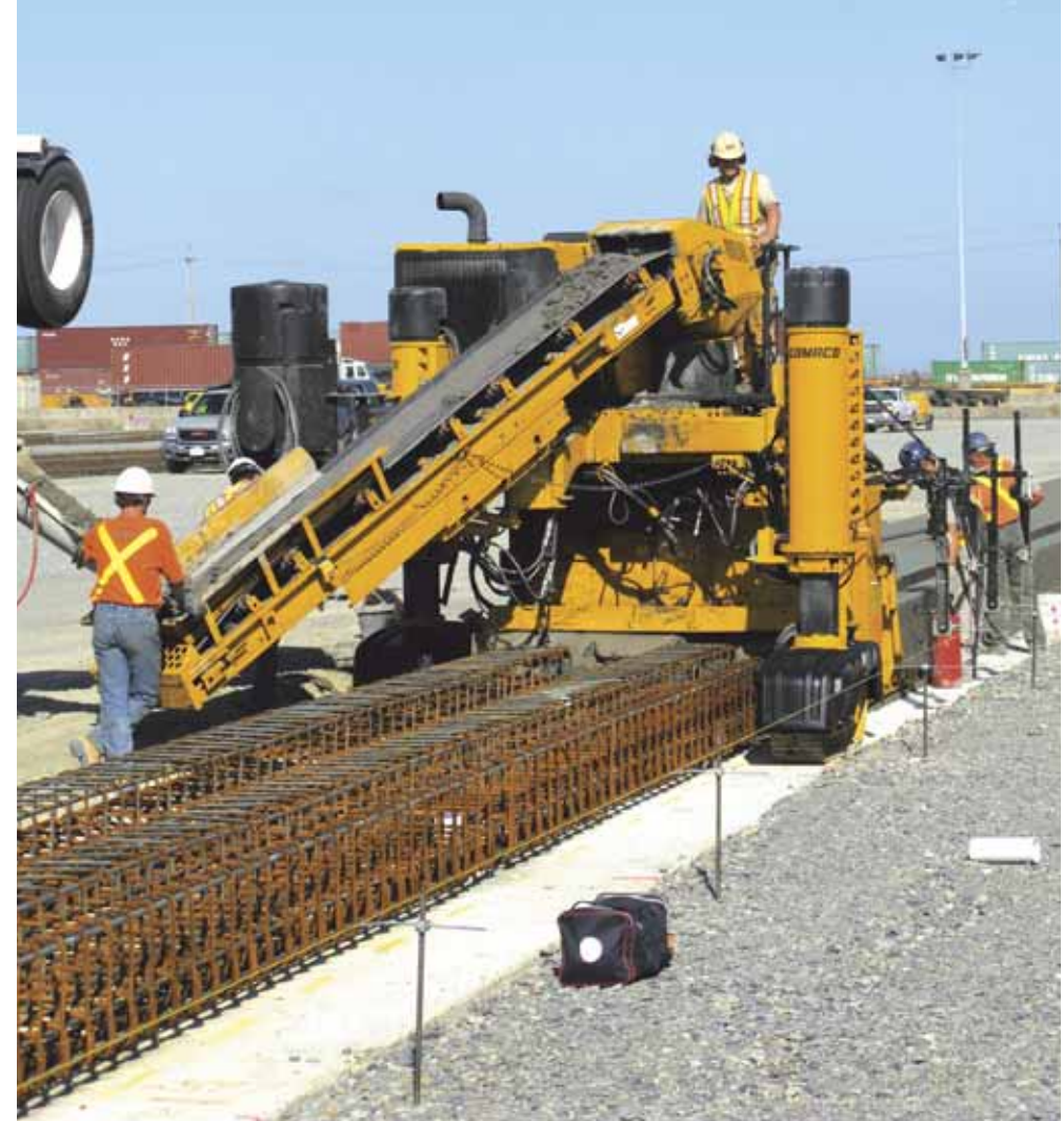
The Commander III’s mold was modified to allow the vibrators to be dropped lower than normal to help move the concrete through the steel reinforcing.
