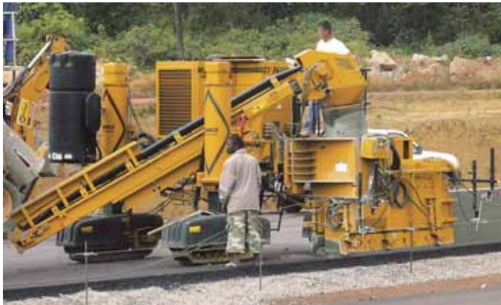
First-time slipformers, ECOCSA, work on a barrier wall project with their GT-3600 in Mongomo, Equatorial Guinea.
