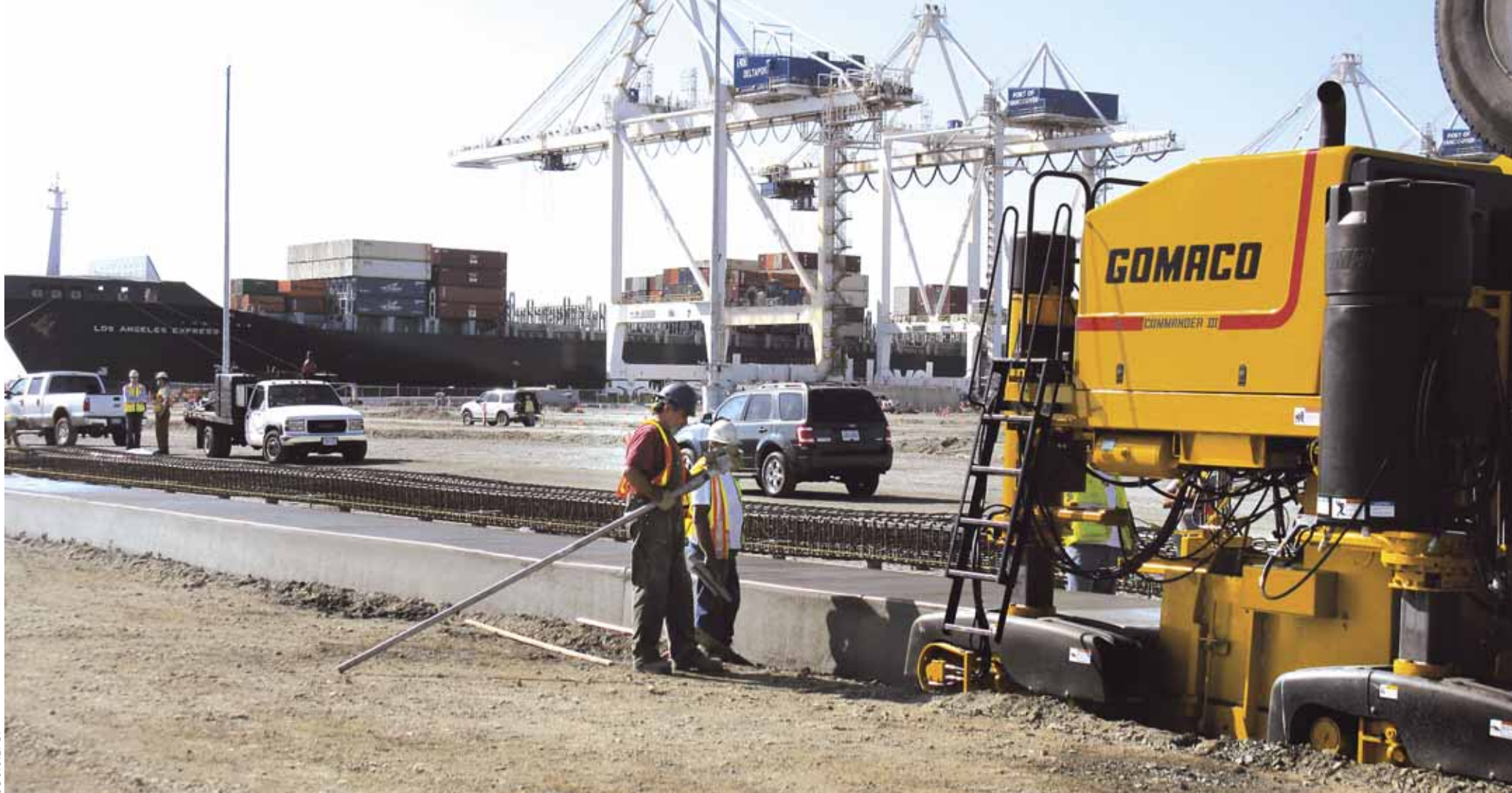
The project was the first time Coquitlam Ridge had ever slipformed. After a successful training period, they started right into production with their first pour with the Commander III.
