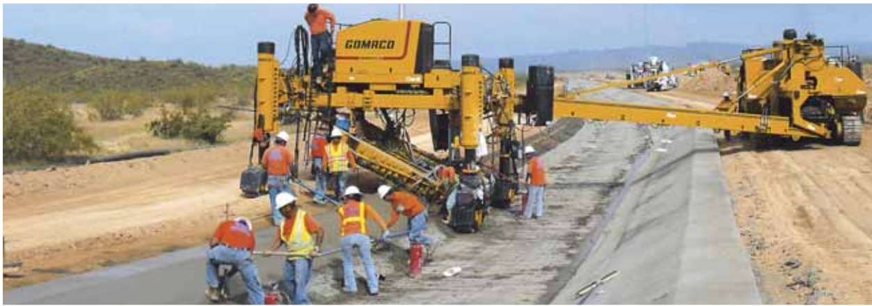
Coffman Specialties slipforms a slope for a smaller canal with their Commander III four-track and a 9500 placing concrete on a project near Phoenix, Arizona.
