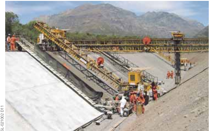
Fe Grande are at work on a large canal project in Rancagua, Chile. They are using two GOMACO CP-650s, one for concrete finishing and one equipped with a compaction roller for the grade. The RC Conveyor on the project is used for placing both the rock for the grade and the concrete for the canal.
