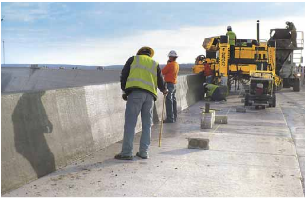
Concrete delivery for the barrier wall was a challenge. Only one ready-mix truck at a time could get to the machine, because there was not enough room for two trucks to pass on top of the reservoir.
