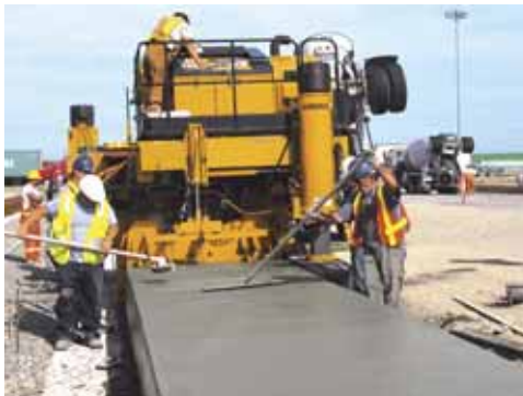
The two runway profiles were each slipformed over an intricate system of steel reinforcing.
