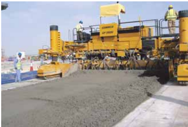
A GOMACO paving train is at work for Consolidated Contractors International Company (CCIC) on the New Doha International Airport in Doha, Qatar.
