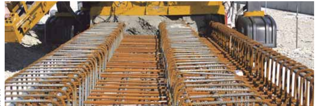
The two runway profiles were each slipformed over an intricate system of steel reinforcing.
