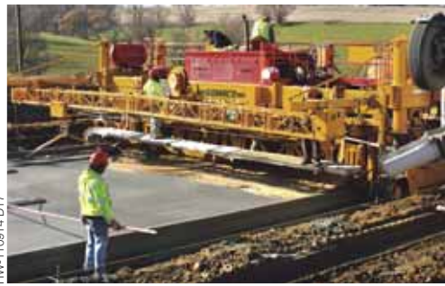
Slipforming a new roadway with integral curb on both sides of the slab.
