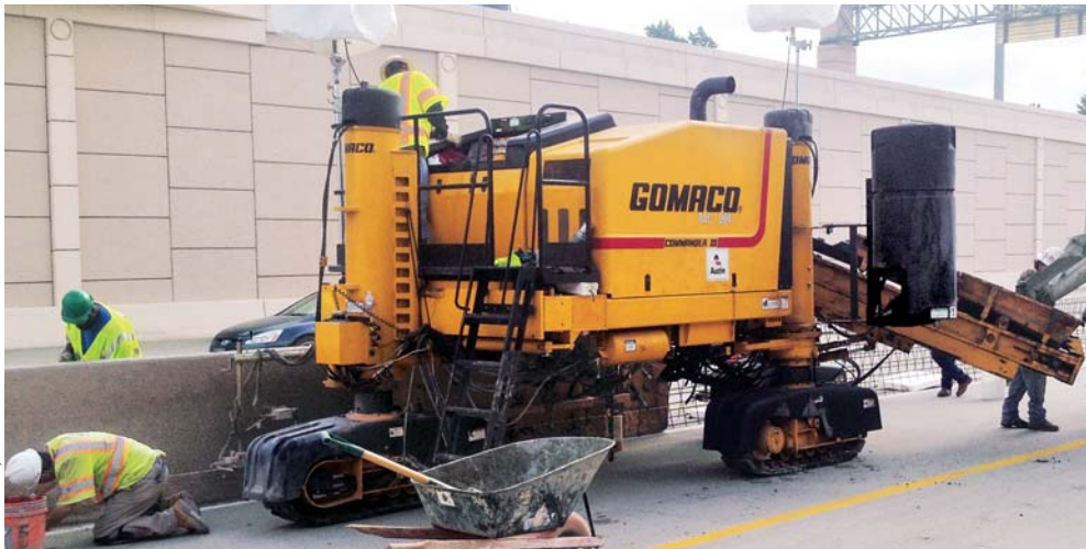
Austin Bridge & Road is slipforming over 18 miles (29 km) of barrier wall on a Texas interstate project with their GOMACO three-track Commander III.
