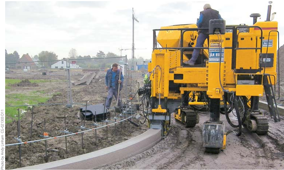
VAN HUELE slipforms a unique profile with their GT-3600 on a project in Koksijde, Belgium.
