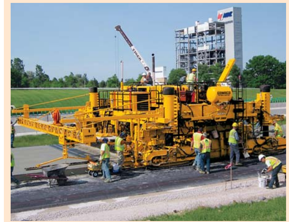
F.H. Paschen, S.N. Nielsen and Associates, LLC., is working on the I-90 westbound reconstruction and widening project in Marengo, Illinois, with their GOMACO GHP-2800 with IDBI. The four-track GHP-2800 is also equipped with a front-mounted center bar inserter, a rear-mounted side bar inserter, and an Auto-Float® attachment. On August 27, 2014, they achieved a record-setting day for their company. The details are listed below:
