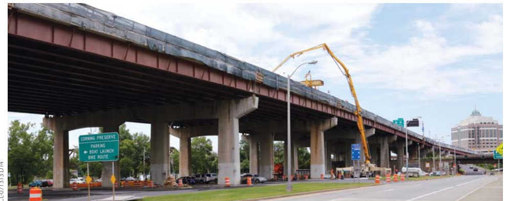
A concrete pump truck works below the bridge on Interstate 787, right next to the Hudson River, pumping the concrete with microsilica up to the GOMACO C-450 finisher.
