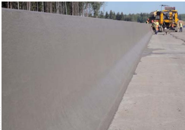
The GOMACO Commander III is at work slipforming 52 miles (83.7 m) of barrier wall along the Moscow-St. Petersburg Motorway in Russia.
