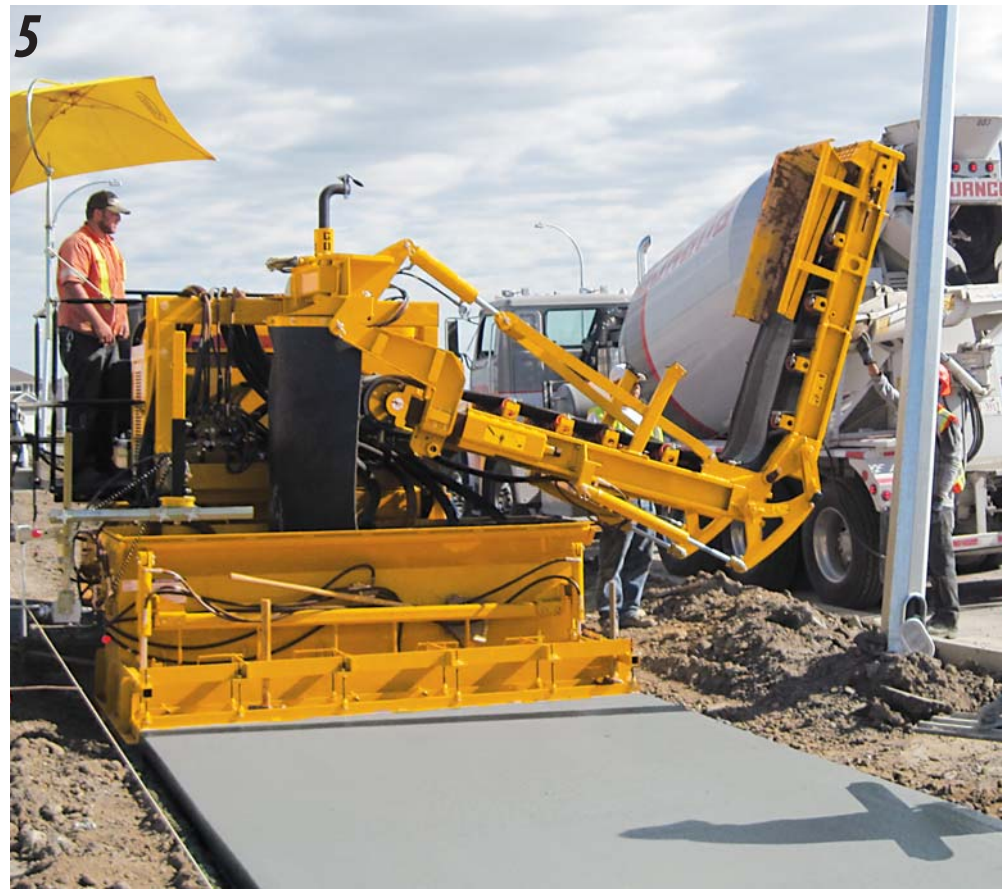
5 The GT-3200 sidewalk paver slipforms past the obstacle and then the ground person can begin to lower the conveyor.
