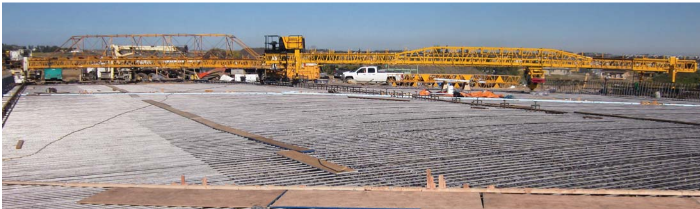
Old meets new on a 104 foot (31.7 m) wide skewed bridge deck project in Edmonton, Alberta, Canada, as an old style GOMACO C-450 finisher with overhead truss works side-by-side with a new C-450 that has transitional framework.
