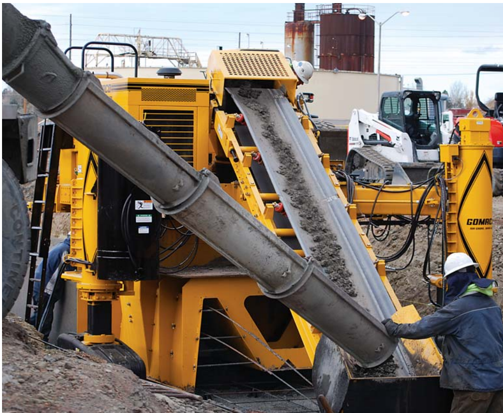
Three strands of rebar are inserted into each of the sidewalls through the front of the mold.
