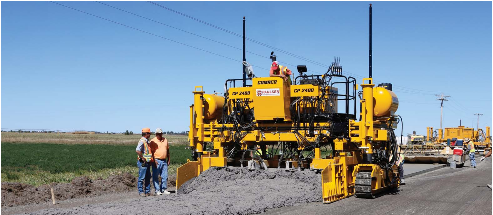
Paulsen Inc. is slipforming a half-width concrete overlay with their GOMACO two-track GP-2400 with Leica Geosystems 3D guidance system on the Darr Link near Cozad, Nebraska.
