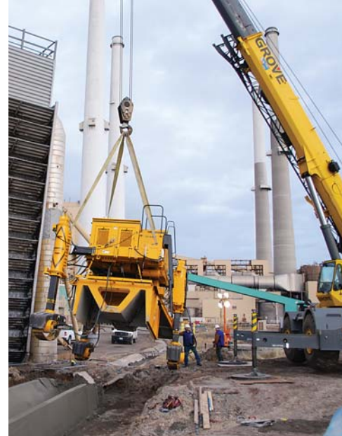
After the pour, the GT-6300 is lifted by crane out of the trench dug for the new water channel.
