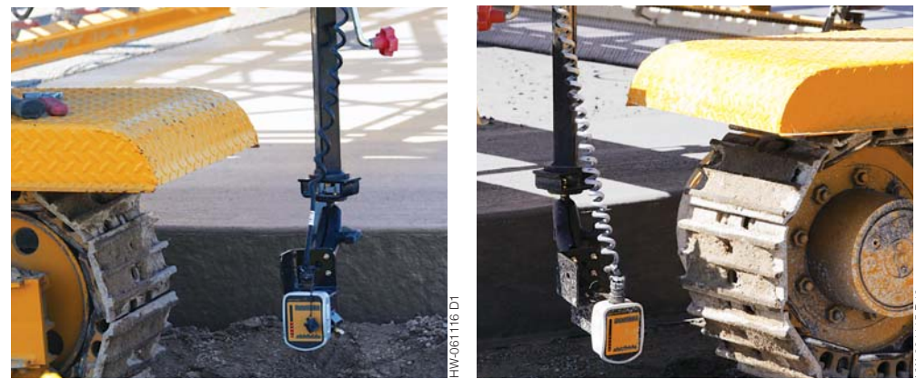
Sonic sensors placed in front and behind the track reference steering and grade for the T/C-600. According to Gehring, the system is a simple stringless solution, and has been working perfectly on the project.
