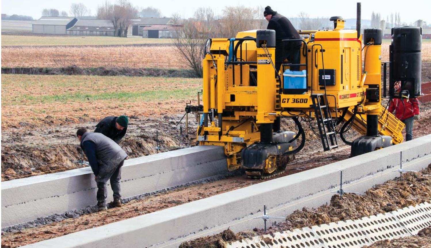
Sico slipformed the retaining wall for flood defense 500 millimeters (19.7 in) wide and 600 millimeters (23.6 in) tall using their new GOMACO GT-3600 curb and gutter machine.
