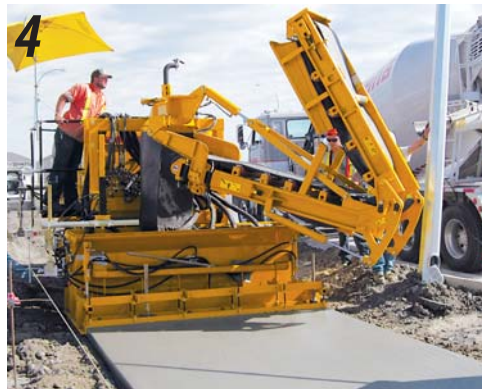
4 The hydraulic pivoting conveyor rotates 90 degrees from center to help clear obstacles.
