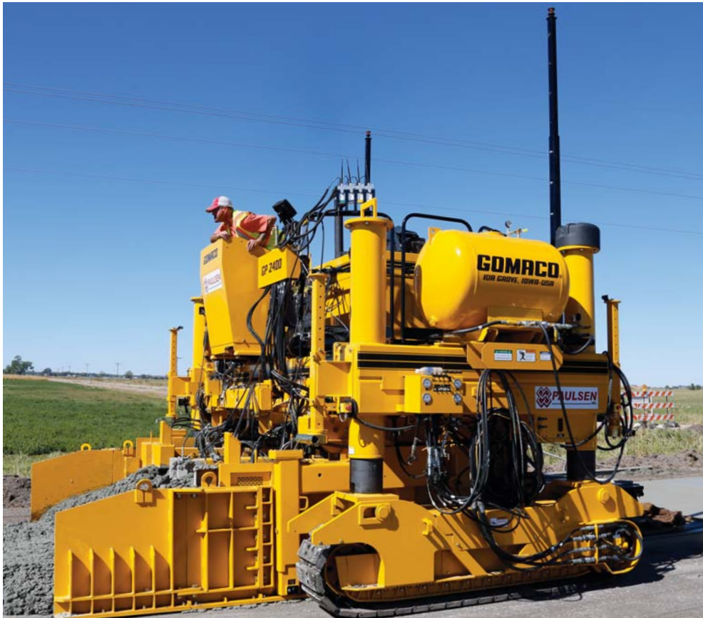
The existing asphalt surface of the road was milled off and swept clean before the GP-2400 could slipform the new five inch (127 mm) thick concrete overlay.
