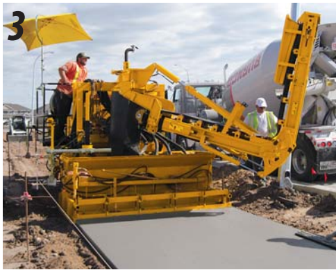
3 It only takes a matter of a few seconds to fold up the 4.3 m (14 ft) long conveyor belt.
