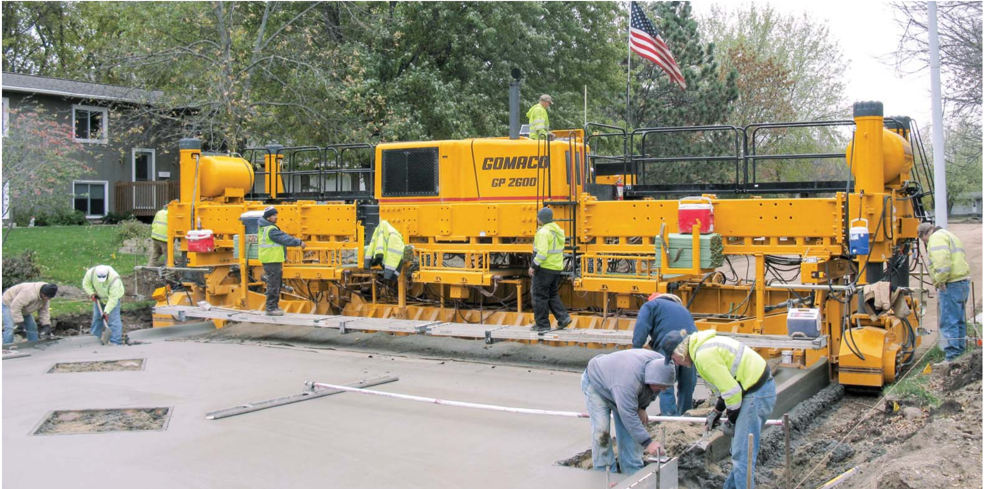
Wick's paving crew had to deal with over 150 box outs for manholes and intakes as they slipformed the 28 blocks of city street in Windom, Minnesota.
