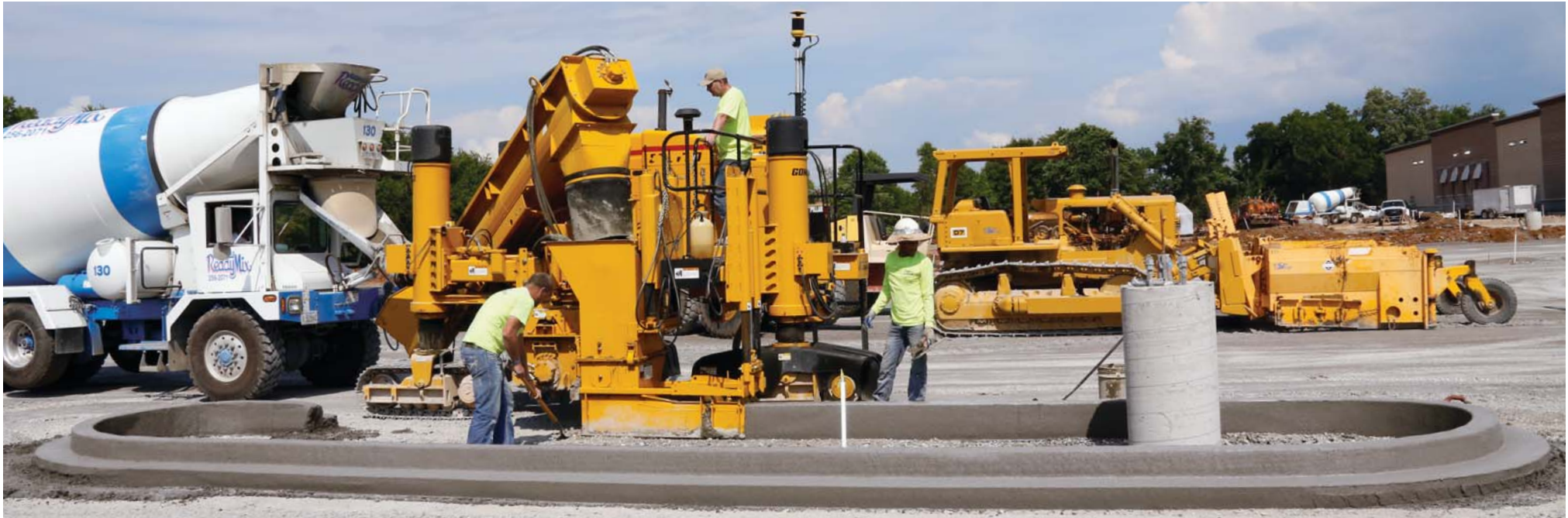
On the first day with the new 3D guidance system, England Contracting and their GT-360 slipformed 16 of the project's 43 islands. The GOMACO GT-360 is England's curb and gutter machine of choice for slipforming tight radii.
