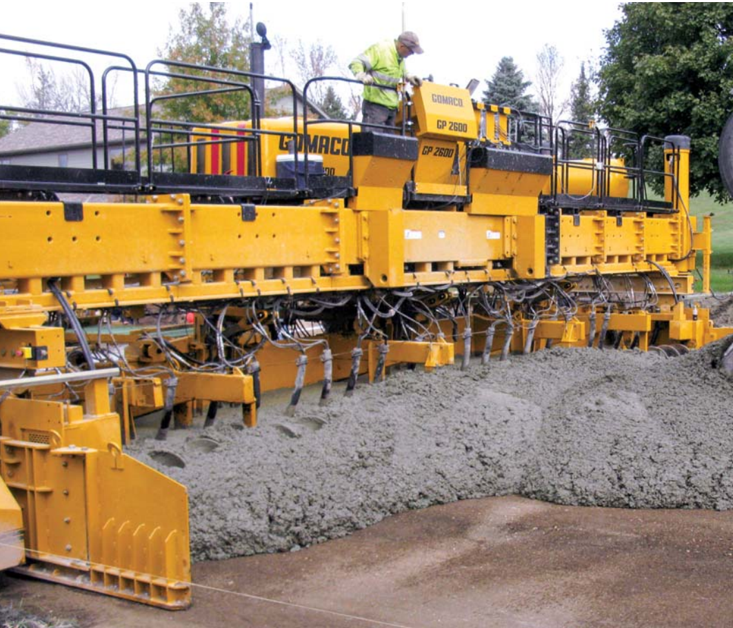
Wick's GOMACO GP-2600 paver is equipped with a 5000 series open front, auger forward mold and three 5400 series bar inserters. The bar inserters are loaded from the work bridge on the back of the paver and the bars are inserted in front of the mold. G+ control boxes manage the placement of the bars every 30 inches (762 mm) into the new city street.
