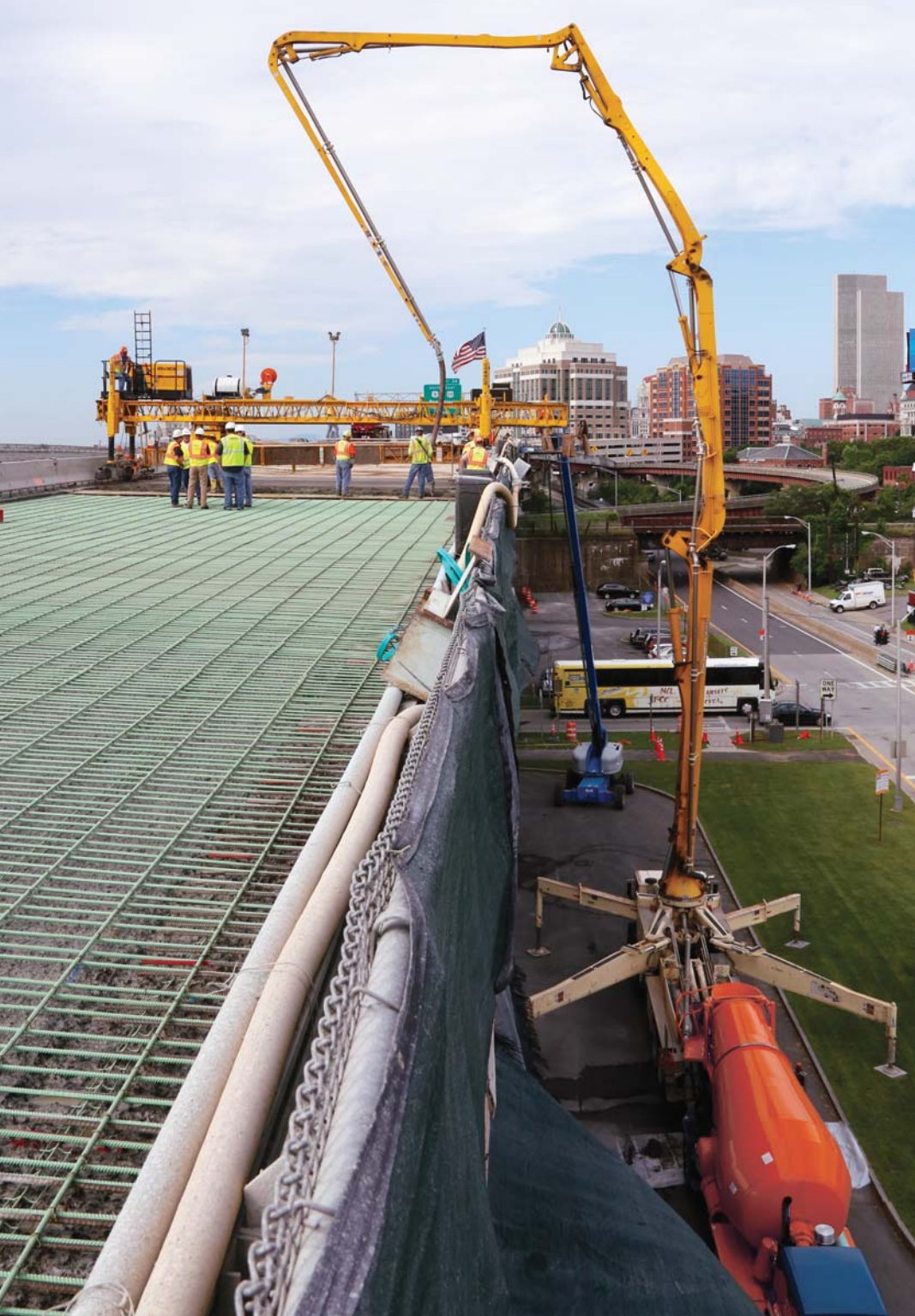
A concrete pump truck works below the bridge on Interstate 787, right next to the Hudson River, pumping the concrete with microsilica up to the GOMACO C-450 finisher.
