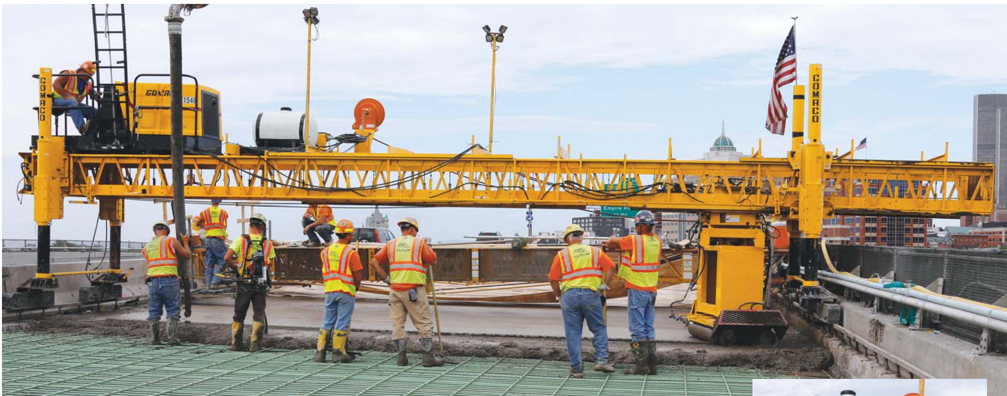
The C-450's undercarriage is equipped with a 36 inch (914 mm) lowering kit, dual augers, five foot (1.5 m) long externally-vibrating double cylinders, and double float pans with a double burlap drag. It also features a fogger system to keep the microsilica concrete from sticking to the finishing cylinders.
