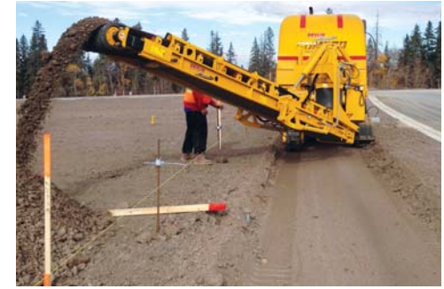
A GT-3400 trimmer's long placing belt moves the trimmed material away from the machine and over the stringline. It is trimming 1.9 meters (6.2 ft) wide on this project in Canada.
