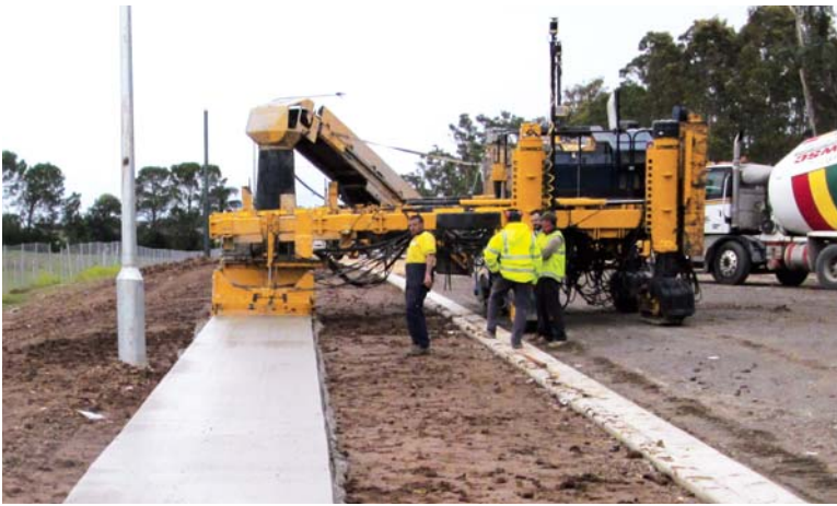
A four-track Commander III with a sidemounted mold slipforms tight-clearance sidewalk in Penrith, New South Wales, Australia.
