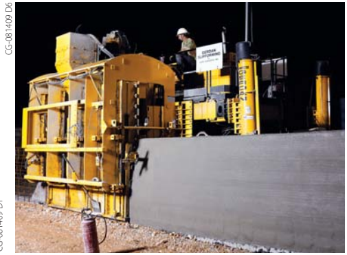
All of the barrier was slipformed at night because of the challenge of dealing with heavy traffic on I-49.
