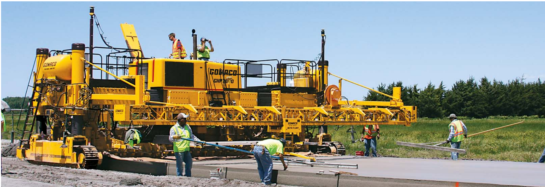
A two-track GHP-2800 slipform paver with Topcon mmGPS 3D guidance system slipforms a new bypass around the city of Columbus, Nebraska.
