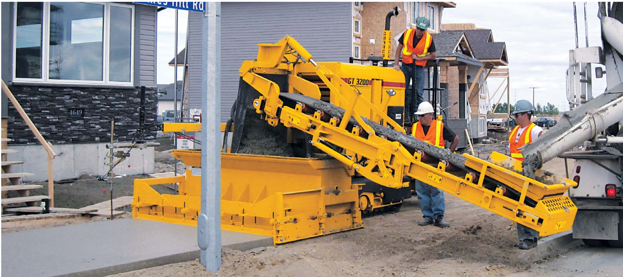
Loewenhardt Construction Ltd. and their new zero-clearance GT-3200 sidewalk paver is at work on a subdivision project in Regina, Saskatchewan, Canada, slipforming three different widths of sidewalk.
