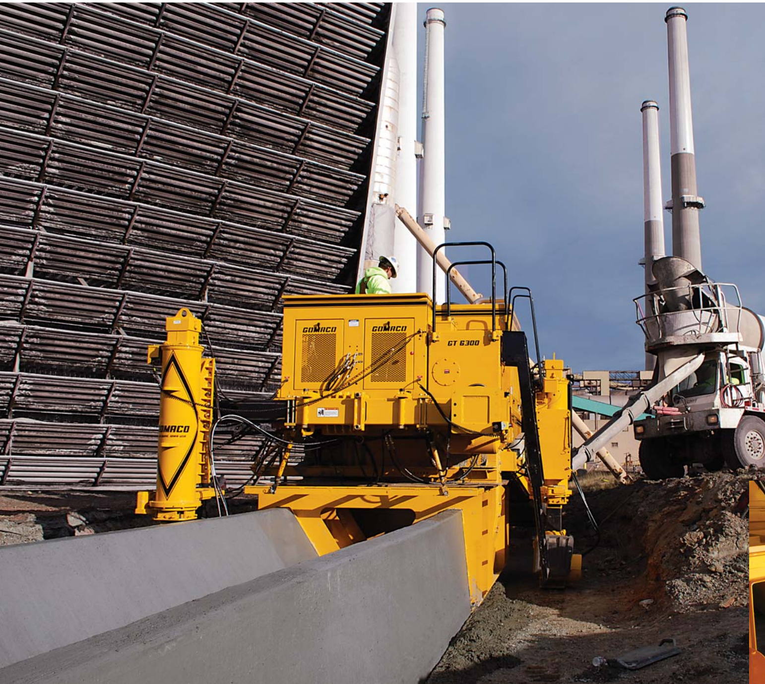
The water channel's large profile was designed to withstand ground movement caused by dynamite blasting from a nearby surface coal mine complex.
