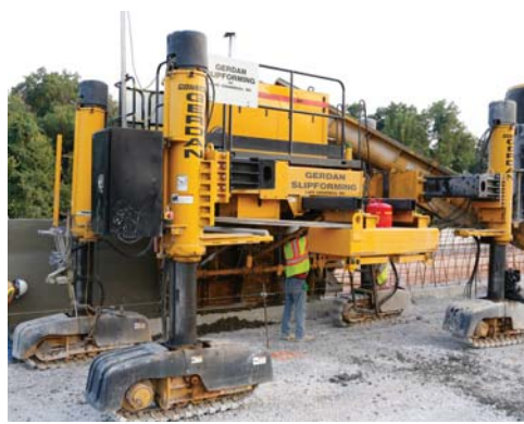
A 5000 pound (2268 kg) counterweight package is positioned on the right side of the paver.
