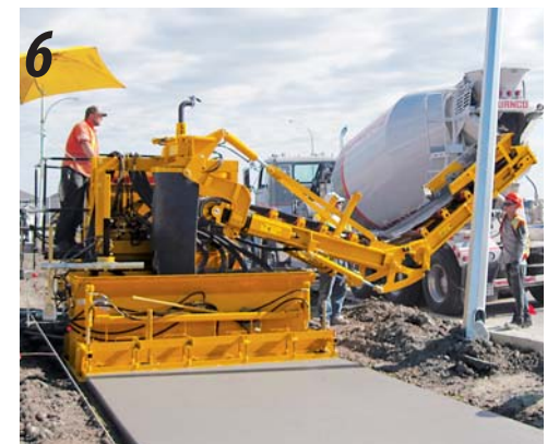
6 The conveyor belt is unfolded and the ready-mix truck, parked on the paved street, starts discharging concrete once again.
