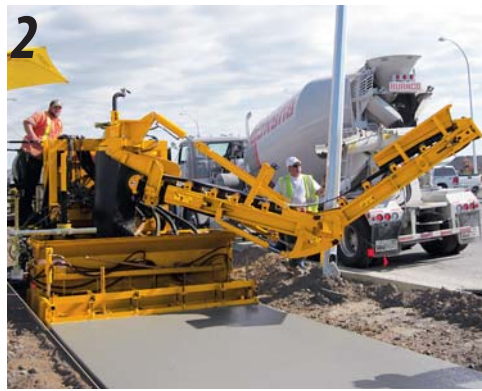
2 The paver keeps slipforming sidewalk as the ground person operates the conveyor belt and starts to fold it up.
