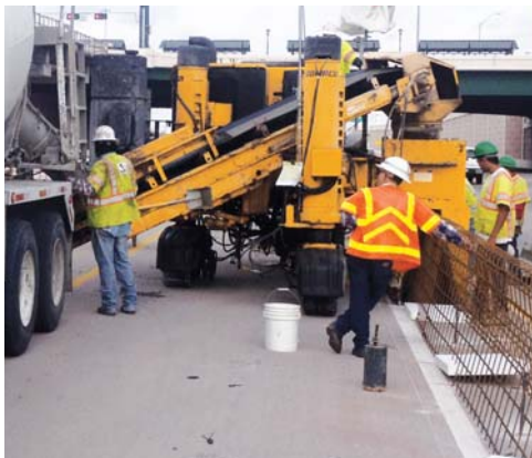
Austin Bridge & Road is slipforming over 18 miles (29 km) of barrier wall on a Texas interstate project with their GOMACO three-track Commander III.
