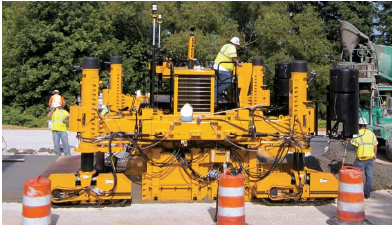
A four-track GP-2400 slipforms a county highway in Montgomery, Indiana, utilizing Trimble 3D guidance.
