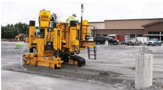
England approaches the island, puts the GT-360 into automatic, lowers the trimmerhead, and the 3D system takes over.
