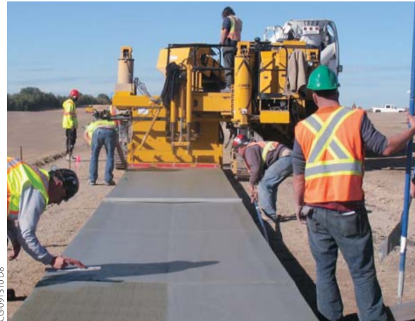
A GOMACO GT-3600 slipforms a six foot (1.8 m) wide, 10 inch (254 mm) thick swale curb in Edmonton, Alberta, Canada.
