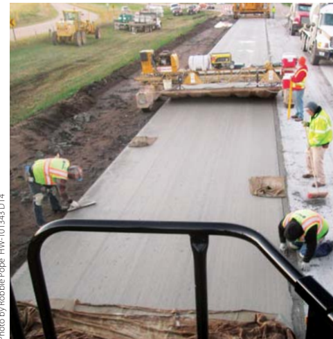
A GOMACO Spanit work bridge applies the burlap drag and white spray cure while a modified PS-30 applies the longitudinal tining to the new overlay.
