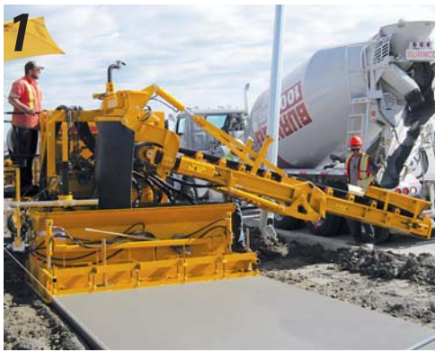
1 As the GT-3200 sidewalk paver approaches the obstacle, the operator loads the sidewalk hopper with concrete.
