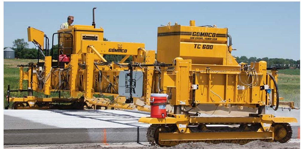
A T/C-600 texture/cure machine applies a longitudinal tining with double white spray cure finish. Sonic sensors are used to guide the texture/cure machine on the 3D stringless project.
