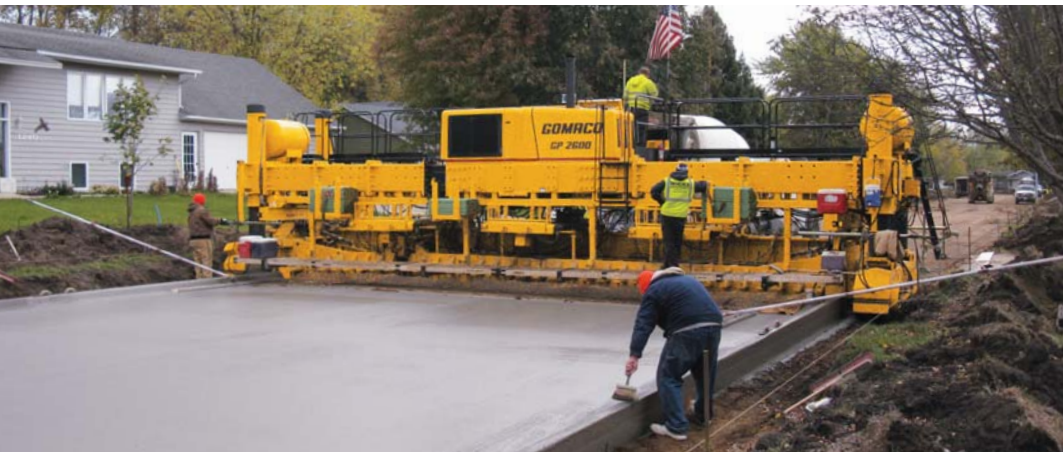
Wick's GOMACO GP-2600 paver is equipped with a 5000 series open front, auger forward mold and three 5400 series bar inserters. The bar inserters are loaded from the work bridge on the back of the paver and the bars are inserted in front of the mold. G+ control boxes manage the placement of the bars every 30 inches (762 mm) into the new city street.
