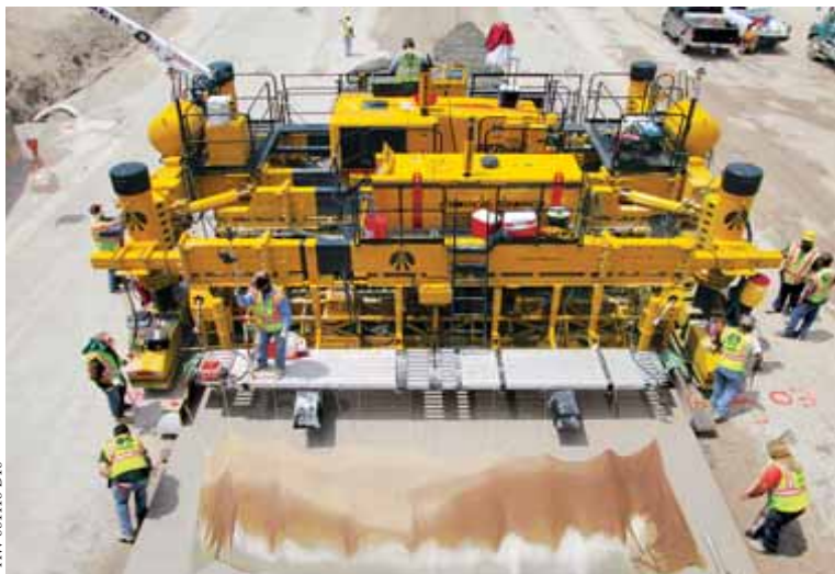
The four-track GOMACO GHP-2800 uses Leica Geosystems 3D guidance on this overlay project. Production on this project increased by 1000 feet (305 m) of paving per day with the introduction of the stringless system.
