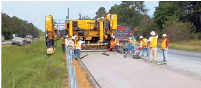
The two-track GHP-2800 paver is using Topcon 3D guidance to pave a single scab-on lane. The machine is straddling the cable guardrail next to the road.
