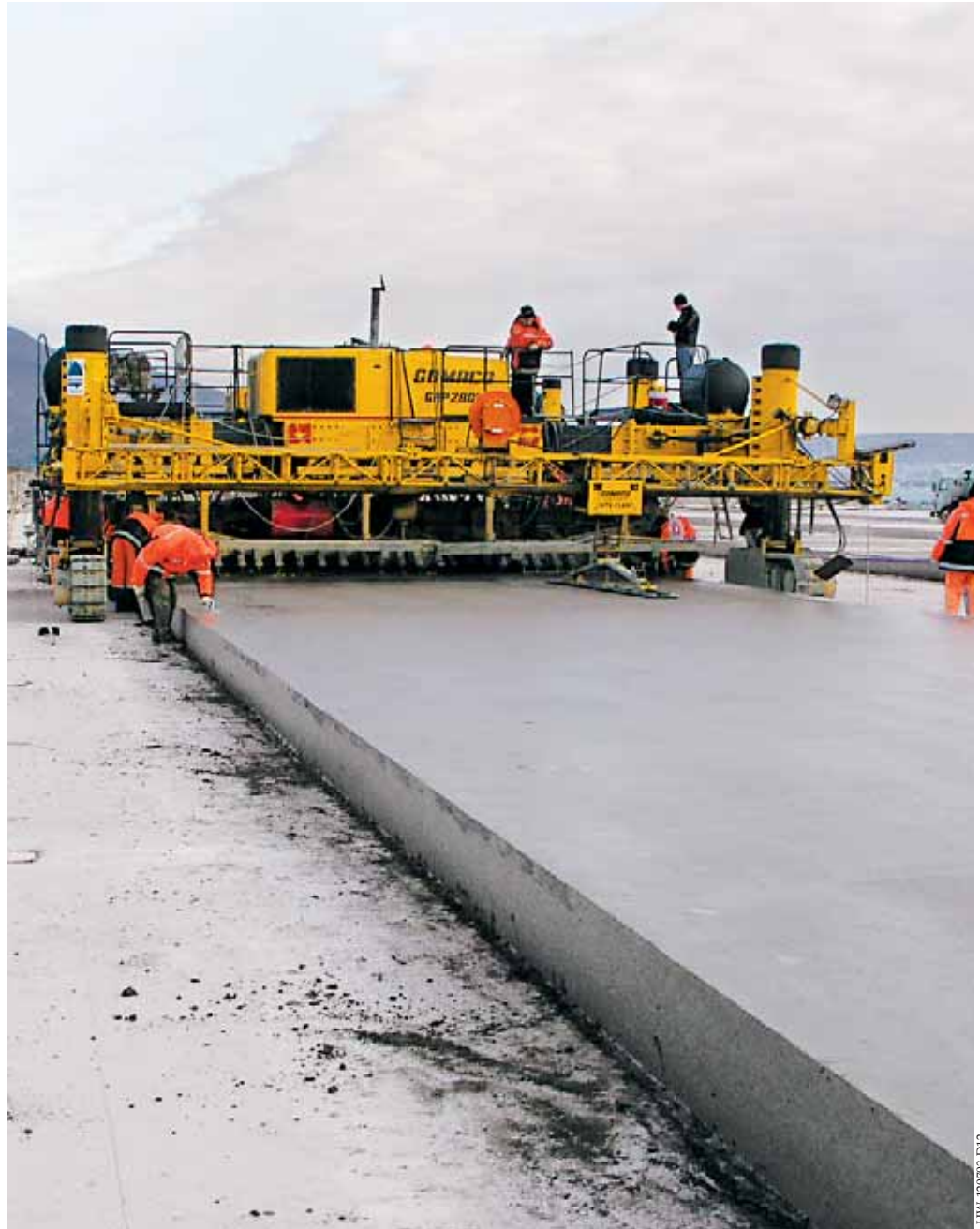
The four-track GOMACO GHP-2800 paver with the 5000 series auger/strike-off mold and Auto-Float slipform part of an airport runway.
