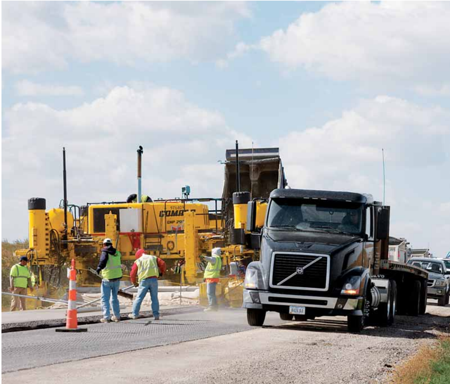
The four-track GOMACO GHP-2800 paver is equipped with two paver-mounted GOMACO Smoothness Indicator (GSI) units and Leica Geosystems 3D guidance. It is paving a half-width overlay 16 foot (4.88 m) wide, which includes a 12 foot (3.66 m) driving lane and a four foot (1.2 m) shoulder. Paving the overlay at half-width allows the road to remain open to traffic throughout construction.
