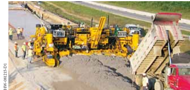
The GOMACO four-track GHP-2800 paver slipforms an interstate highway. The paver is equipped with GOMACO G+ controls, Leica Geosystems 3D guidance, and an IDBI.
