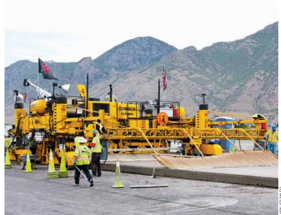
The GOMACO four track GHP-2800 is equipped with a 5400 series mold and Auto-Float to create the ultimate finish on a new roadway project.
