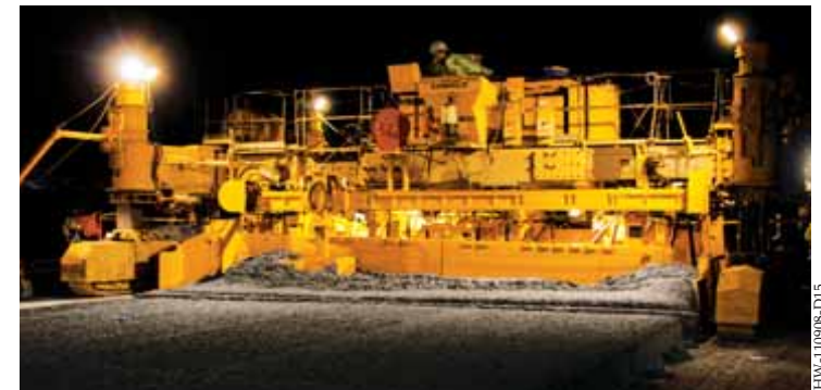
The GOMACO four-track GHP-2800 paver is equipped with a 5400 series paving mold featuring a spreader plow and also a rear loading, front inserting 5400 series bar inserter. It's paving the new highway at 25 feet (7.62 m) wide.
