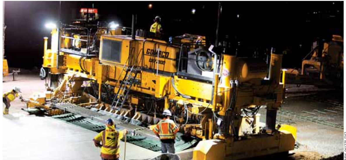
The two-track GHP-2800 paver is equipped with Leica Geosystems 3D guidance to slipform a new ramp underneath an interchange during a night pour.
