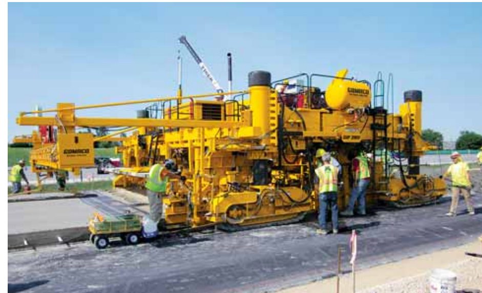
This four-track GHP-2800 slipform paver is equipped with a side bar inserter (SBI) and an Auto-Float while working on a highway system.
