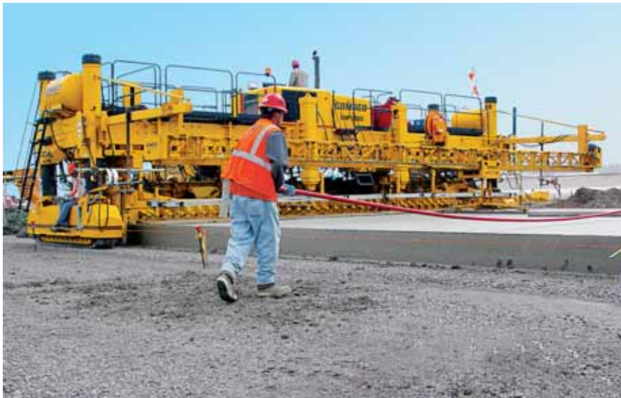
GOMACO's two-track GHP-2800 is equipped with an Auto-Float® and is paving a new runway.
