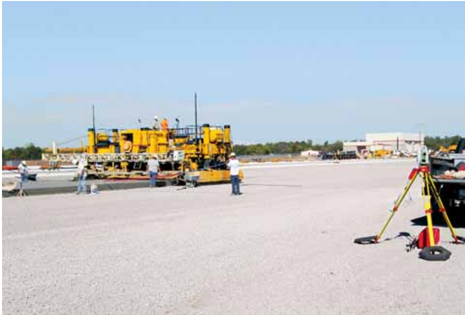
The two-track GHP-2800 paver with a 5000 series auger/strike-off mold and Leica Geosystems 3D guidance slipforms an airport parking apron and taxiway.
