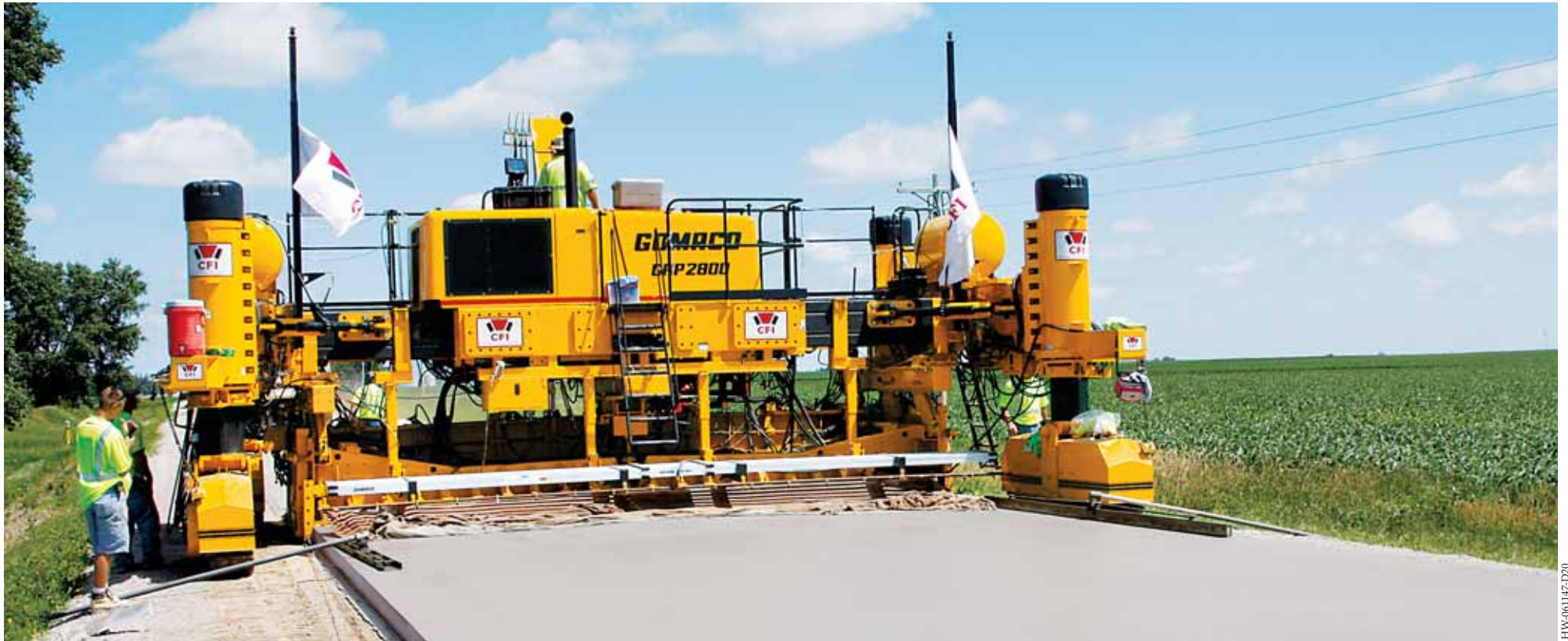
The four-track GOMACO GHP-2800 uses Leica Geosystems 3D guidance on this overlay project. Production on this project increased by 1000 feet (305 m) of paving per day with the introduction of the stringless system.
