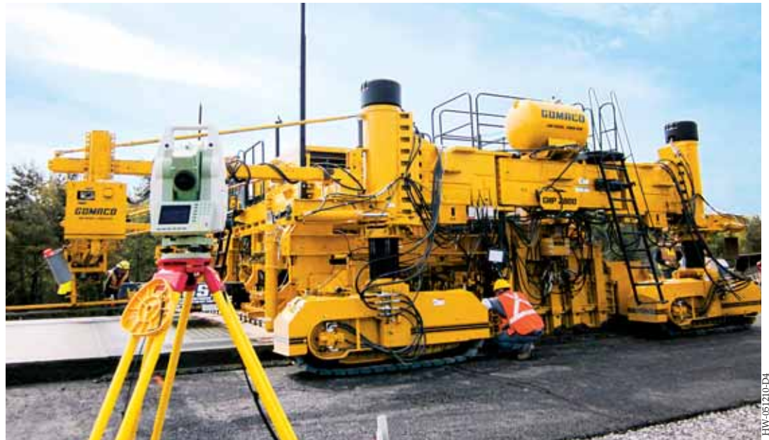
The GOMACO GHP-2800 paver is equipped with an IDBI attachment, two paver-mounted GOMACO Smoothness Indicator (GSI) units, and Leica Geosystems 3D guidance to pave the 25 foot (7.6 m) wide by nine inch (229 mm) deep overlay on top of the existing asphalt.
