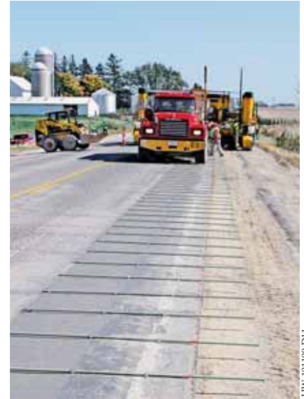
Six foot (1.8 m) long, #5 steel rebar, were placed on 30 inch (762 mm) centers on the existing roadway to tie on the new eight inch (203 mm) thick shoulder. The new road is 4.5 inches (114 mm) thick.
