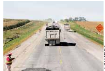
The existing asphalt surface was milled and swept clean to prepare for the unbonded concrete whitetopping. Trucks dump the concrete directly onto the grade in front of the paver.
