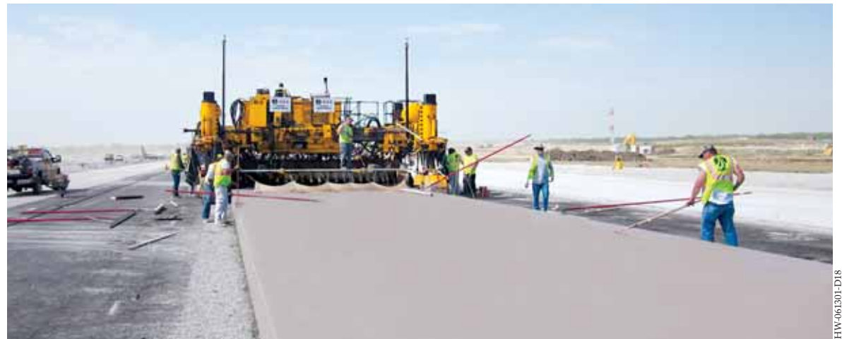
The four-track GHP-2800 is equipped with Trimble 3D stringless guidance while slipforming at an airport.
