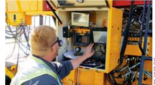
On the ground – personnel have the ability to monitor paving information and make adjustments to the PTAs, 3D systems, GSI units, and more.
