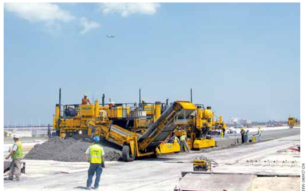
The GOMACO PS-2600 places concrete in front of a two-track GHP-2800 paver equipped with 3D guidance as it slipforms an airport runway.
