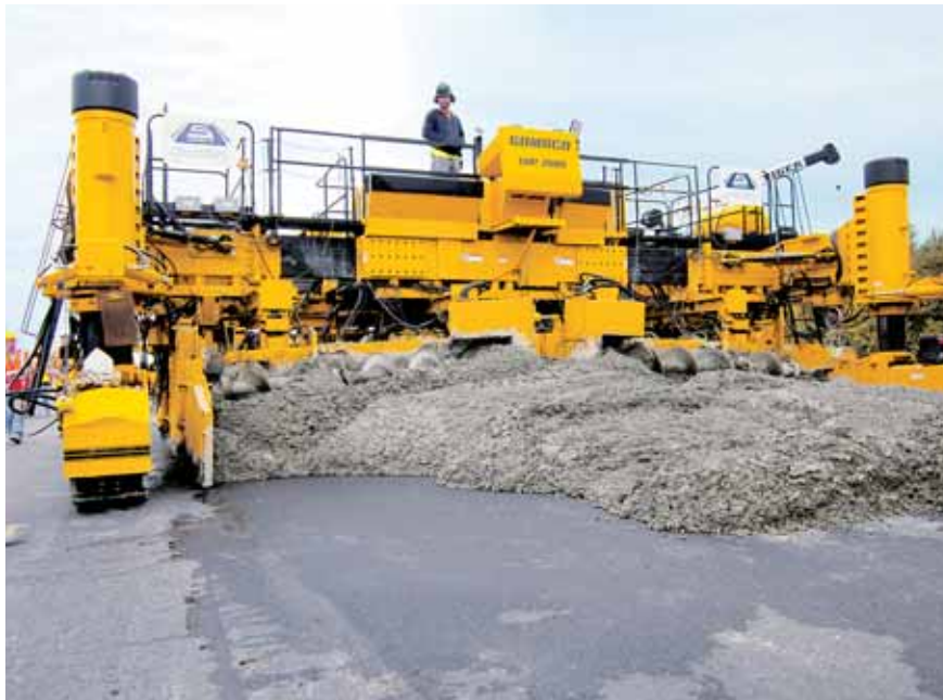
The GOMACO GHP-2800 paver is using Leica Geosystems 3D guidance to slipform the concrete overlay on top of the existing asphalt.
