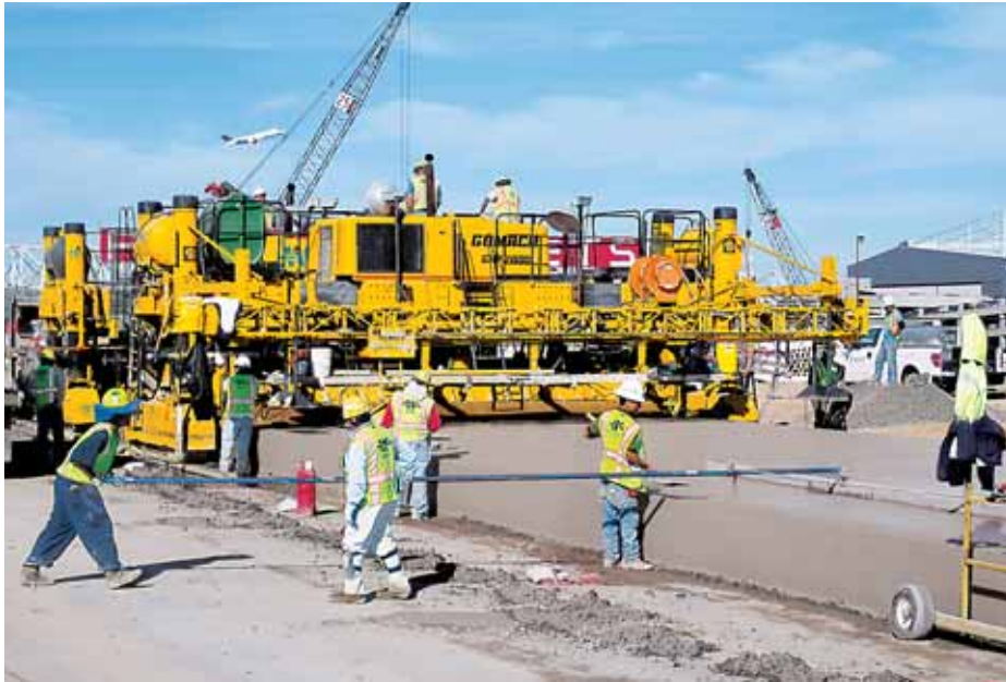
The two-track GOMACO GHP-2800 paver slipforms an airport apron 20 inches (508 mm) thick with some areas having 25 inch (635 mm) thickened edges.
