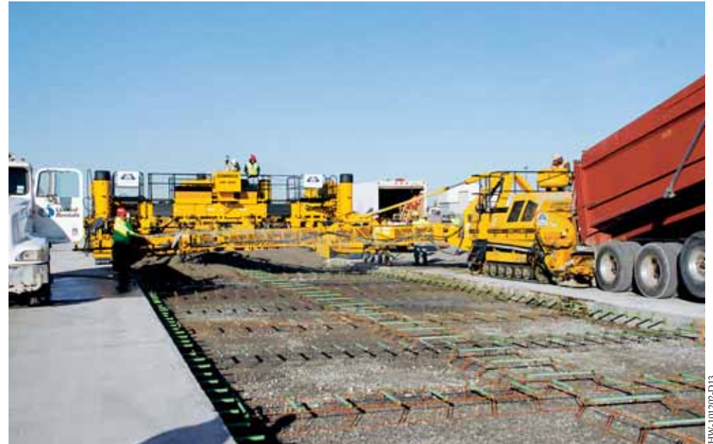
The GOMACO RTP-500 places concrete in front of the four-track GHP-2800. The paver is equipped with the 5400 series mold to create a smooth finish on the military air base's taxiways.
