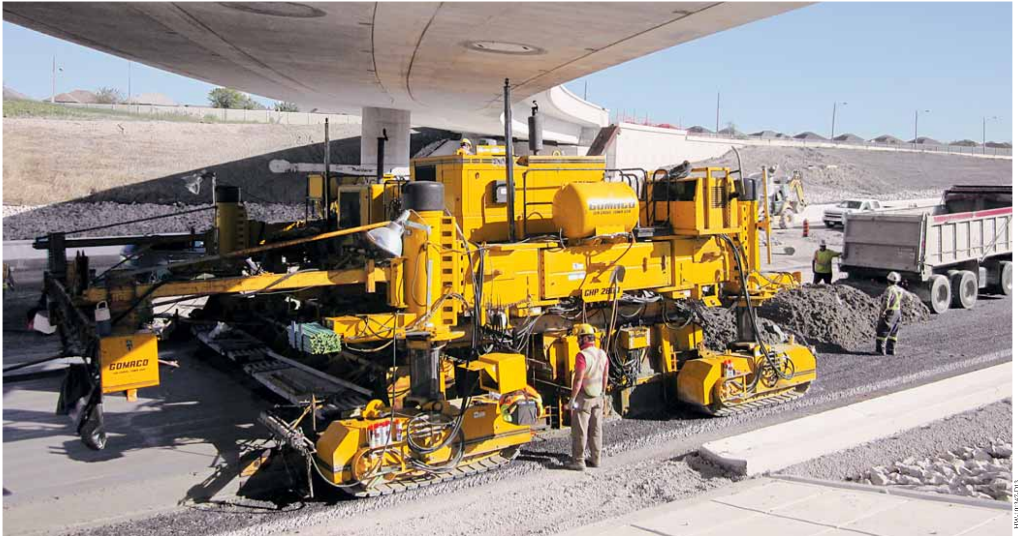
The four-track GHP-2800 paver is equipped with the Leica Geosystems 3D guidance, 5000 series auger/strike-off mold, IDBI, frame-mounted tie bar inserter (TBI), and side bar inserter (SBI) to efficiently slipform a new highway under the existing overpass.
