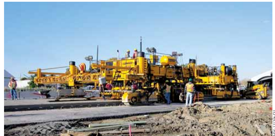
The four-track GOMACO GHP-2800 paver is equipped with an Auto-Float and Leica Geosystems 3D guidance while slipforming this highway.
