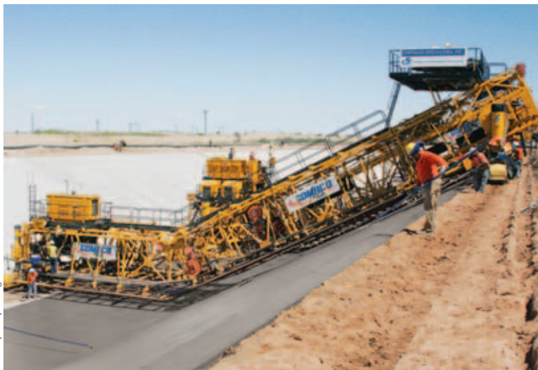
Each transverse joint had to be inserted in under three minutes to maintain a five foot (1.5 m) per minute paving production rate.
