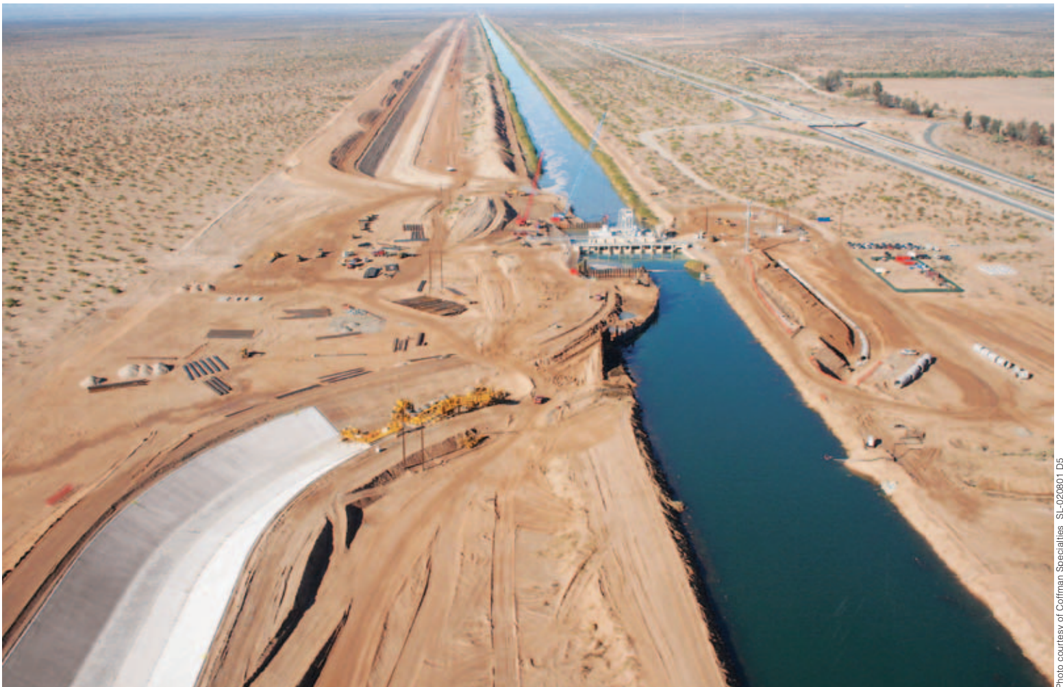
Coffman’s crew makes the second paving pass on Reach Three of the canal project. Just a few days of concrete paving was left for the crew when this photo was taken.
