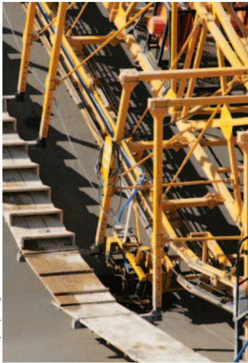
The transverse water stop inserter mechanism inserted the material as it made a run up the slope of the canal wall.
