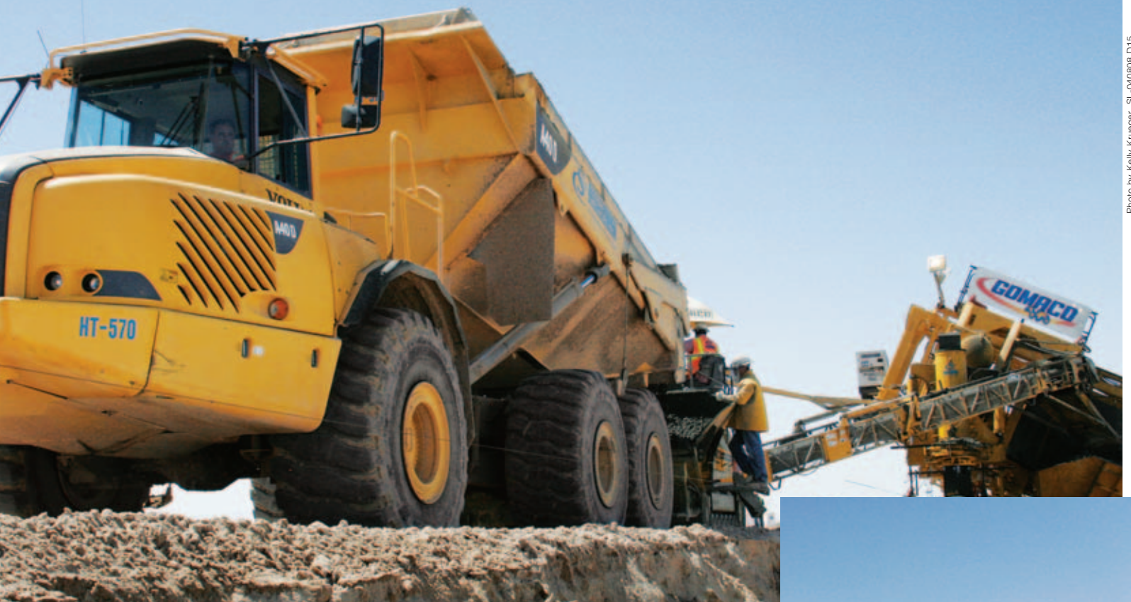
A truck dumps its load of concrete into the GOMACO RTP-500 as the paver continuously feeds the concrete into the handling system on the paver.
