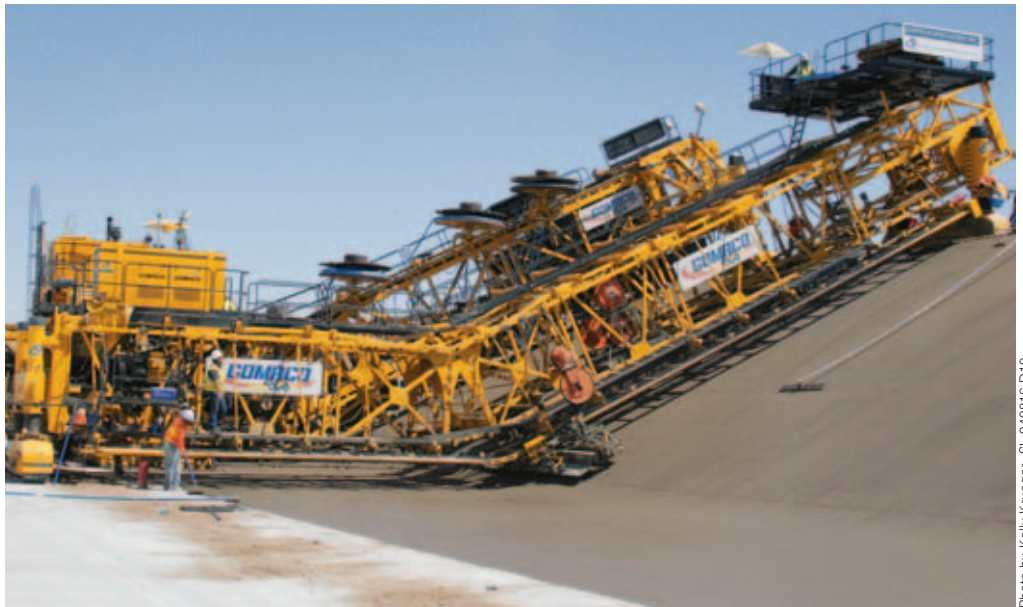
A float pan and 17 foot (5.2 m) long finishing cylinder working from the rear of the water stop machine helped repair and finish any wounds left over from inserting the water stop.
