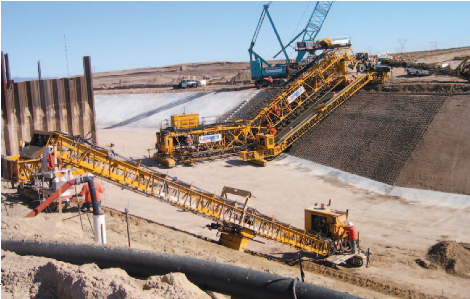
A GOMACO C-650 (pictured in the foreground), with a trimming undercarriage attachment, trimmed the final grade in the transition areas of the canal.
