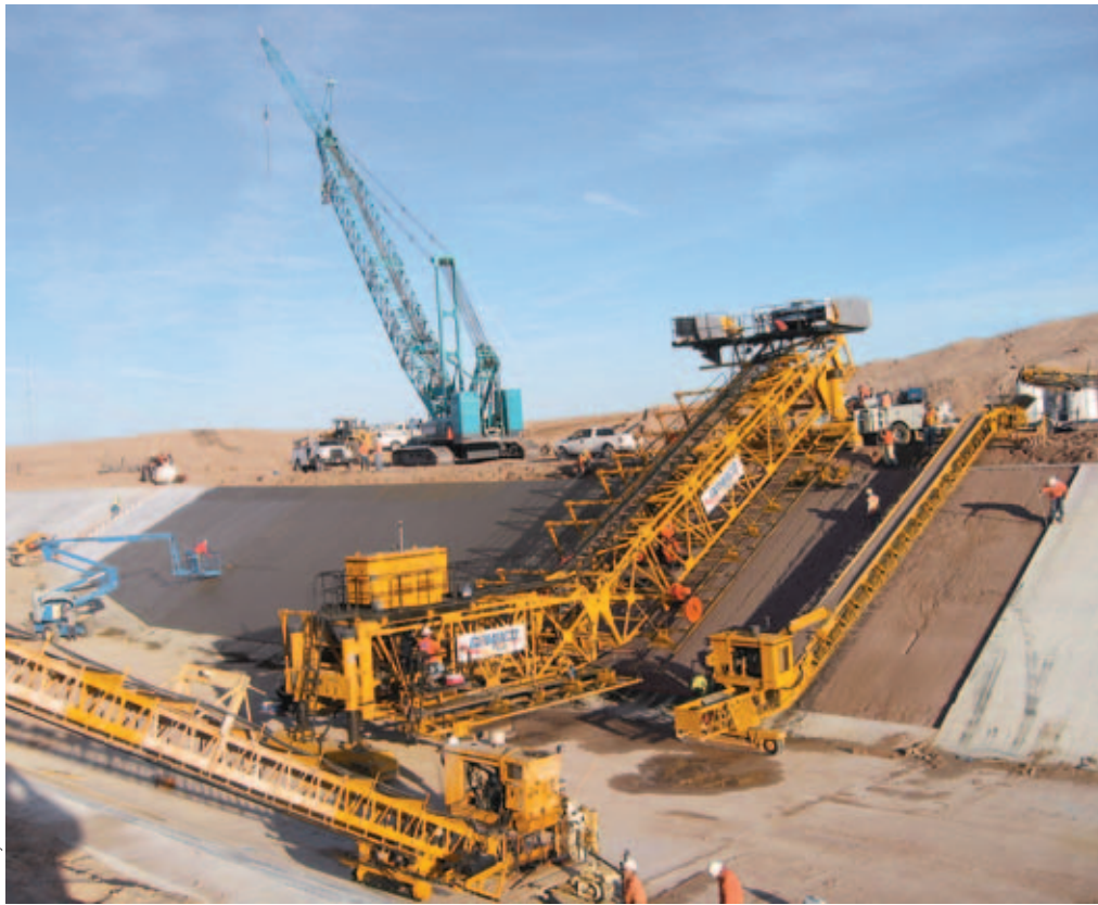
The water stop machine was equipped with a C-450 finishing cylinder and operated in reverse to finish the transition areas while inserting the material for the transverse water stop.
