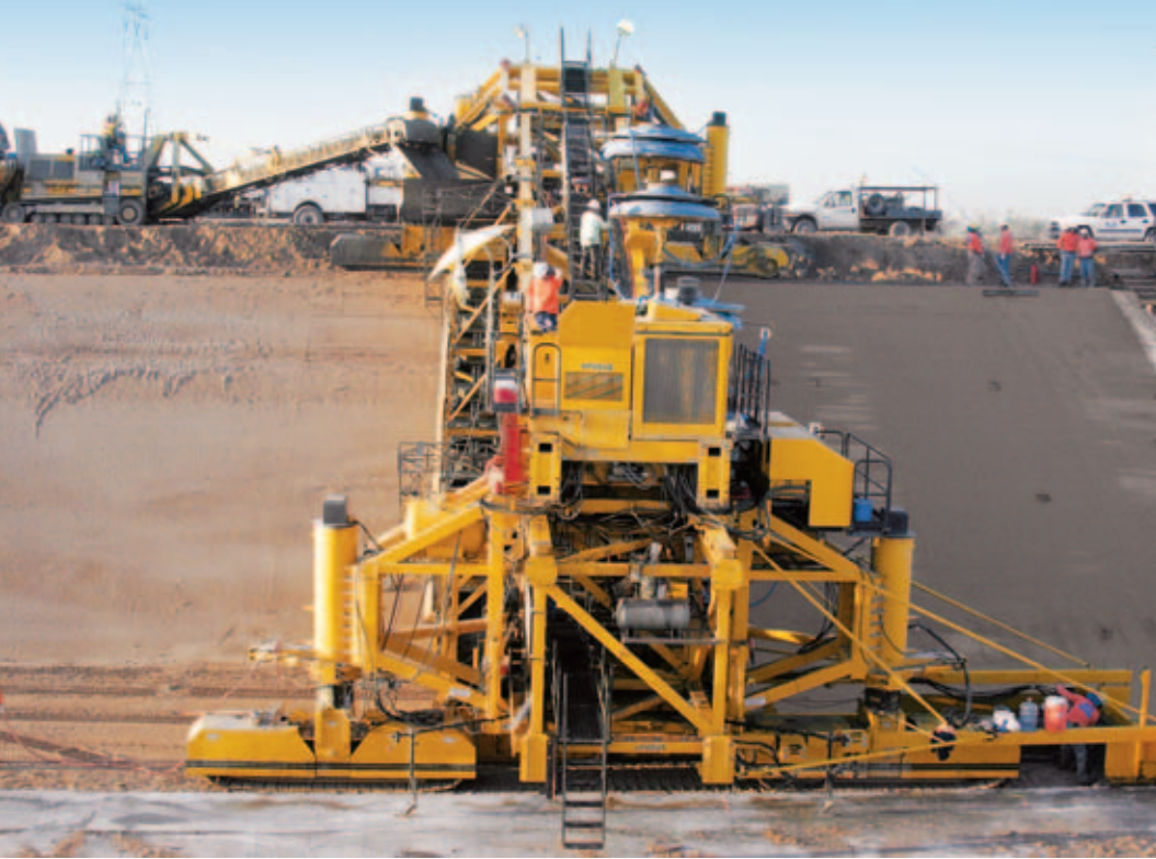
The All-American Canal paver, on the second paving pass, featured a zero-clearance trailing form to allow the tracks to travel on the grade and not the finished concrete.
