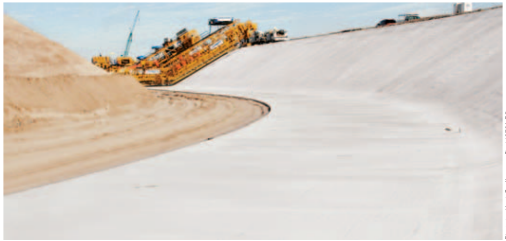
The concrete was a workable mix design for inserting the water stop material and closing up the void around the material.
