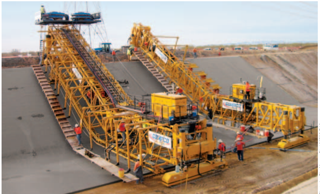
Two operators ran the water stop machine. One in front controlled the travel and water stop insertion, while the operator in back operated the carriage with finishing pan.
