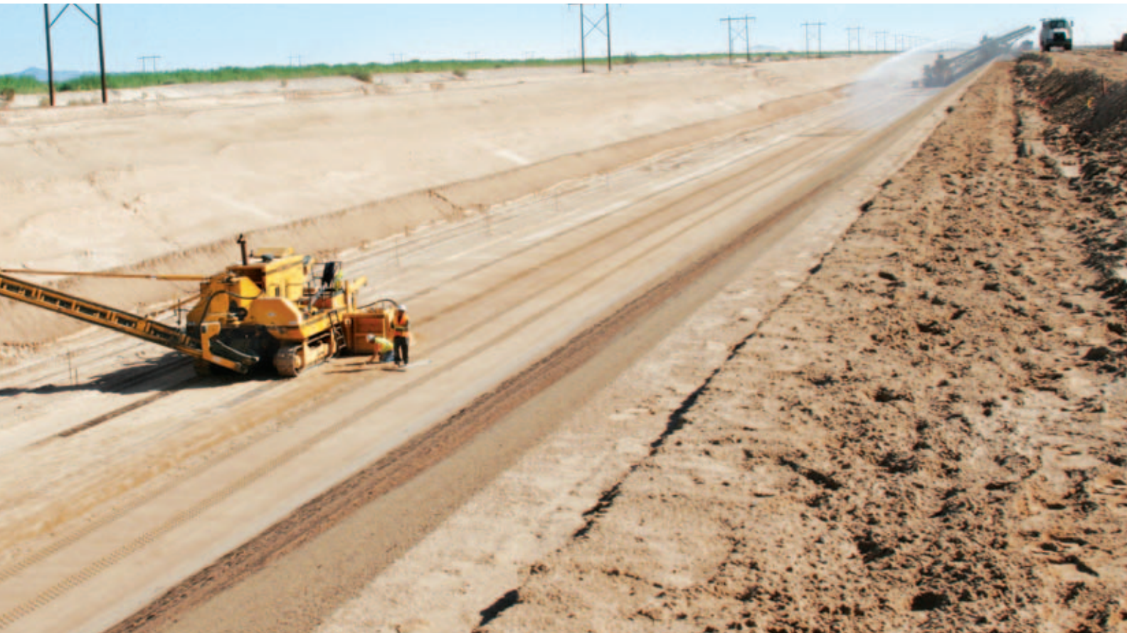
A GOMACO 9500 trimmer prepares the final grade on the 50 foot (15.2 m) wide floor of the All-American Canal.
