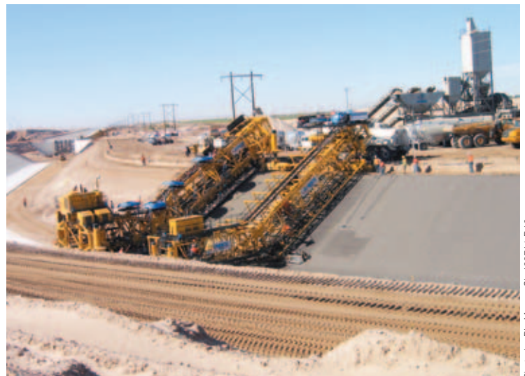
The paving train slipforms by the batch plant while paving Reach Two. The longest concrete haul was six miles (9.7 km).
