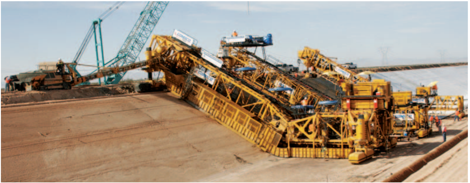
The exclusive GOMACO Powered Wedge on the canal equipment allowed them to match the canal's trimmed grade and changing angles.
