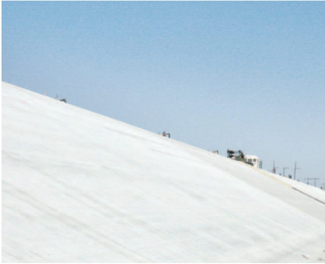
Coffman’s crew makes the second paving pass on Reach Three of the canal project. Just a few days of concrete paving was left for the crew when this photo was taken.
