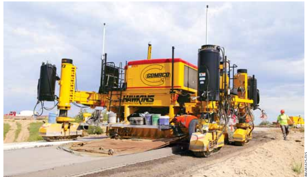
The GP3 with a 3D machine guidance system slipforms an eight foot (2.44 m) shoulder with a burlap finish onto a highway ramp.
