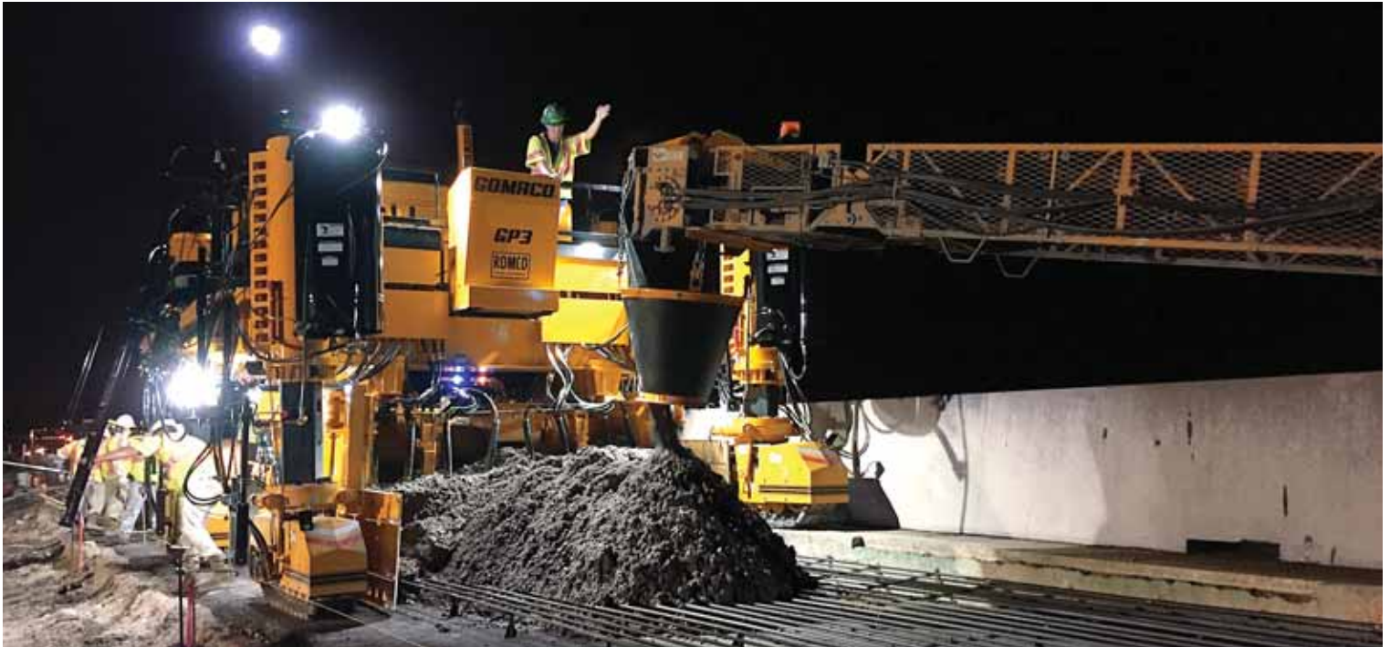
The GOMACO GP3 slipforms a scab-on lane over continuous steel during a night pour on an interstate project. A GOMACO RTP-500 places the concrete in front of the GP3.
