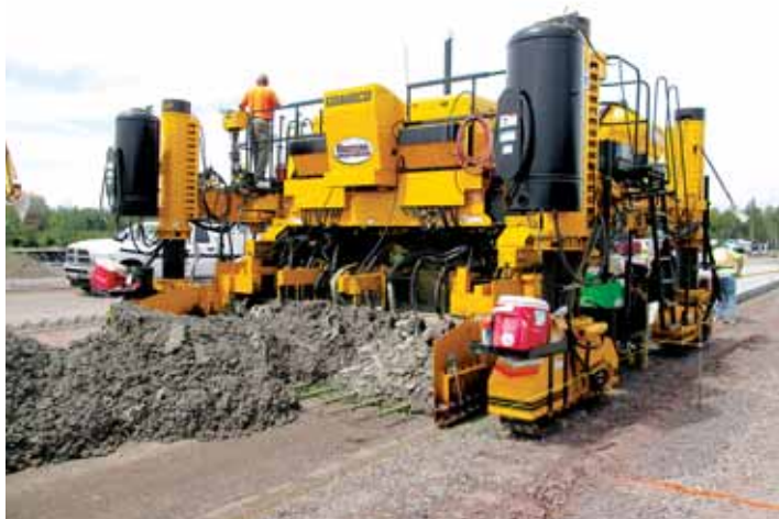
This GP3 is slipforming 15 feet (4.57 m) wide, 10 inches (254 mm) thick at a new weigh station.
