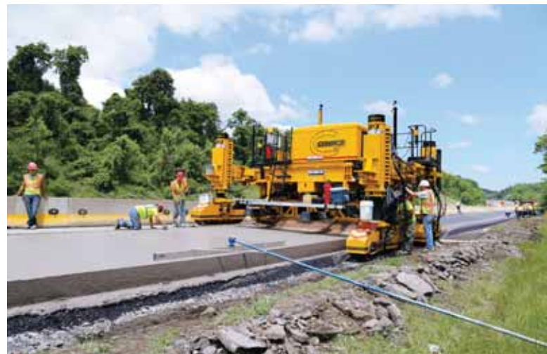
The smart width system provides easy, accurate width change setup and also a reference for G+ to control proper steering and track speeds at varying widths of the paver.
