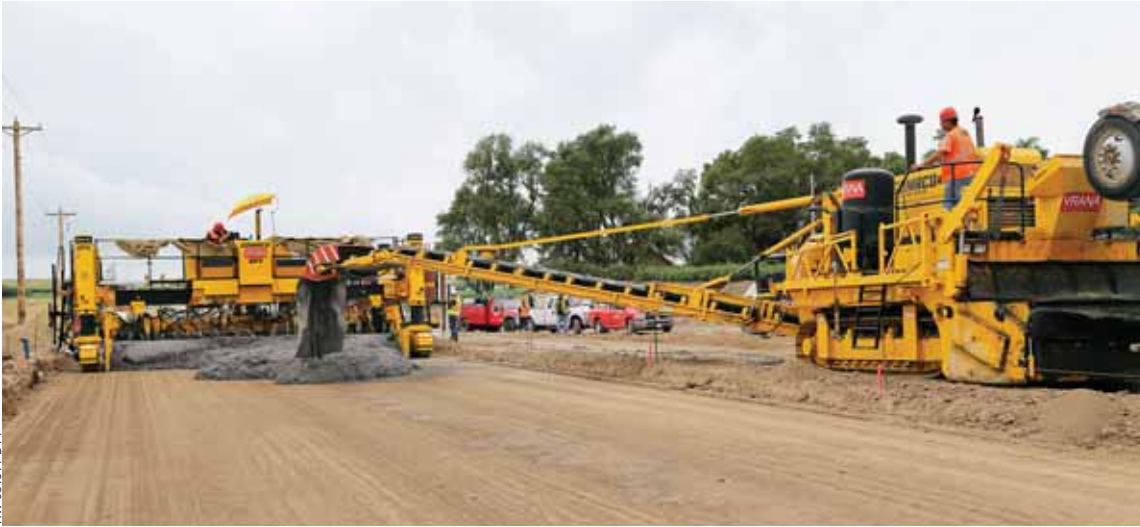
A GOMACO GP3 slipforms a 25 foot wide (7.62 m) road with the concrete being placed in front of the slipform paver by a GOMACO 9500 placer.
