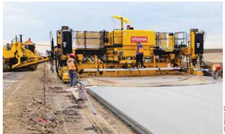
The 5400 series bar inserter is front or rear loading and front inserting for ease of use. It mounts to the mold's T-bar and allows on-the-go crown changes, while maintaining a constant depth. The bar box is mounted to the paver's rear T-beam mounting rail for easy access and loading of the bar magazine.
