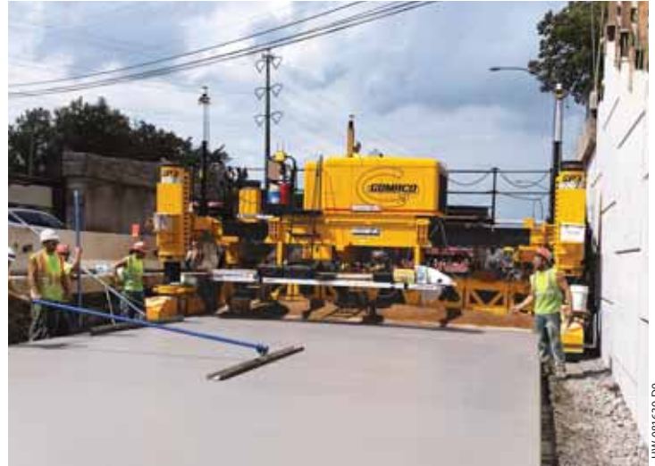
This GOMACO GP3 is equipped with a 5400 series paving mold and is slipforming a 22 foot (6.7 m) wide section of an interstate project. Minimum clearance is facilitated using 3D machine guidance.
