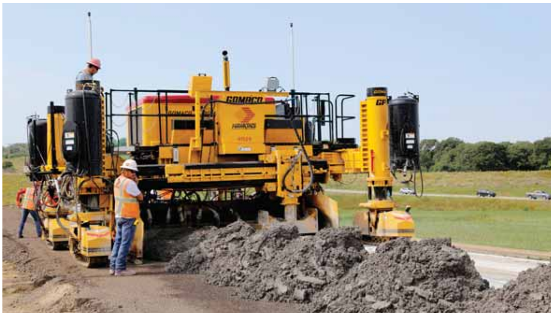
This GOMACO GP3 features a telescoping spreader plow on the front of the paver to spread the concrete ahead of the mold.
