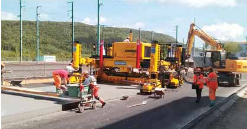
The GP3 slipforms a roadway that is 16.4 feet (5 m) wide. The GOMACO GP3 features an isolated operator's platform for optimum operator comfort. There is also easy access to the operator's platform from both sides of the machine.
