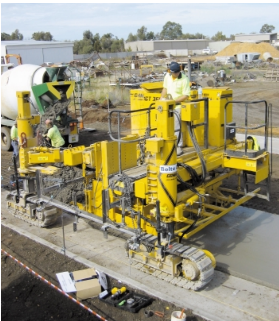
Bolte Civil undermounts a 9.8 foot (3 m) wide mold to their GT-3600 to slipform this section of roadway on a project in New South Wales, Australia.
