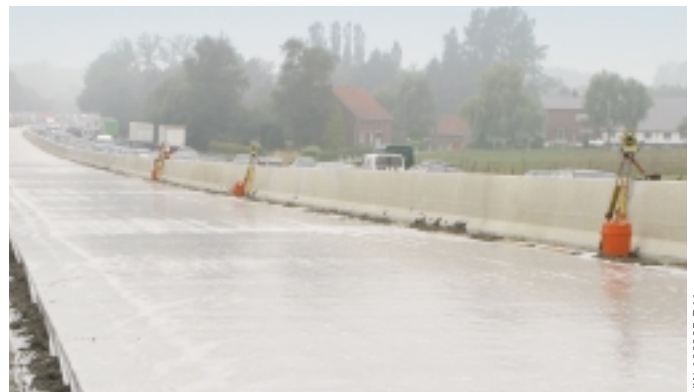
Two total stations work behind the paver sending measurements while the third measures the accuracy of the slab.
