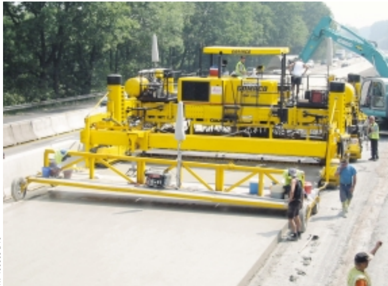
Project specifications required a ride of only 0.24 of an inch per 9.8 feet (6 mm/3 m). Betonac averaged 0.12 of an inch (3 mm).
