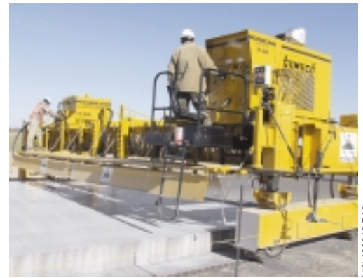
A T/C-400 follows the paver applying a transverse tine finish and spray cure to the new roadway.
