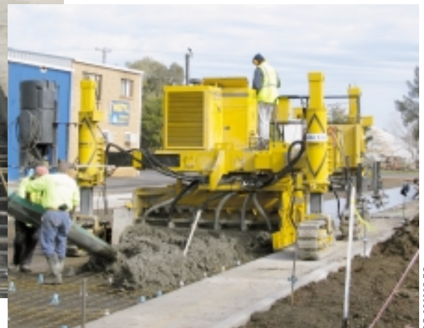
A majority of Bolte Civil's projects are slipformed over continuous steel reinforcing.
