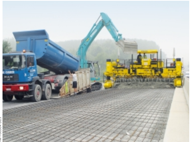
There was no room for a haul road, so concrete was first dumped into a holding container before an excavator placed it in front of the paver. 17
