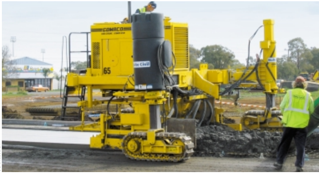
The GT-3600's All-Track Positioning allows Bolte Civil to position the legs in the necessary alignment to pave this section of new roadway.
