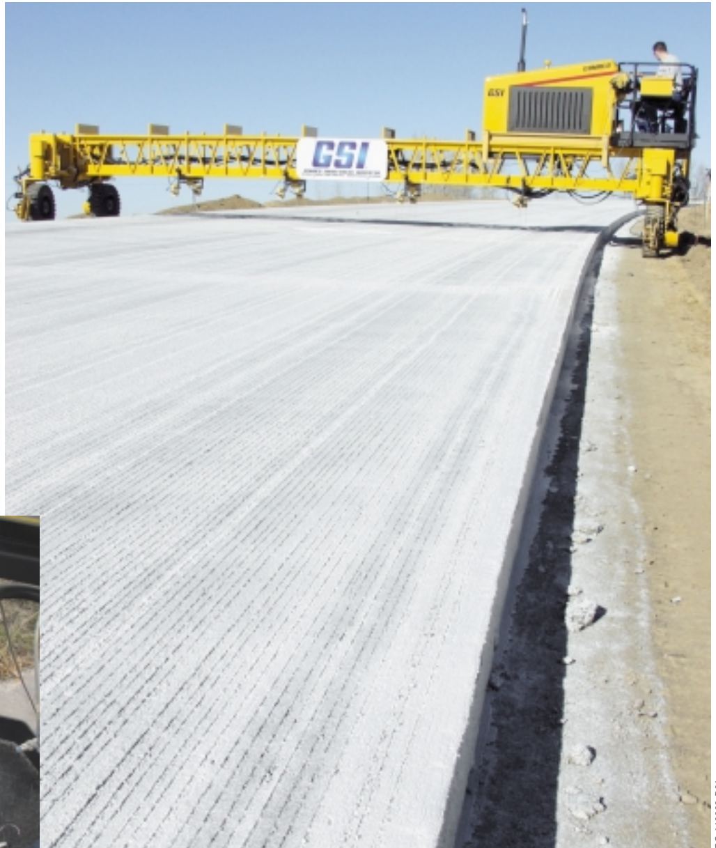
The GSI measures pavement smoothness behind the texture/cure machine on a project near Onawa, Iowa.
