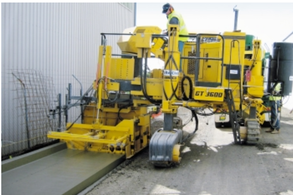
Bolte Civil sidemounts their mold to slipform 4.9 feet (1.5 m) wide flow path with integral curb.
