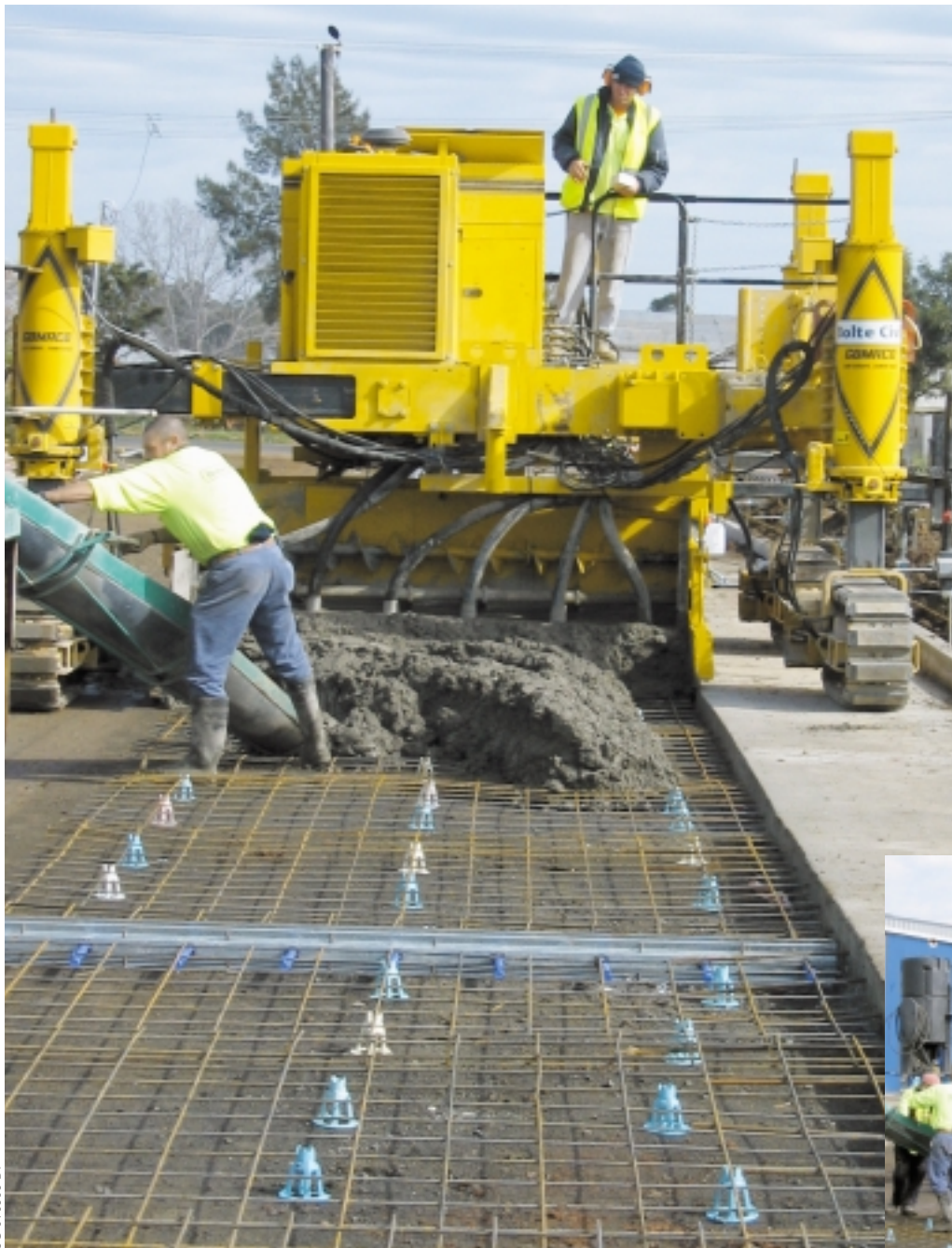
A majority of Bolte Civil's projects are slipformed over continuous steel reinforcing.
