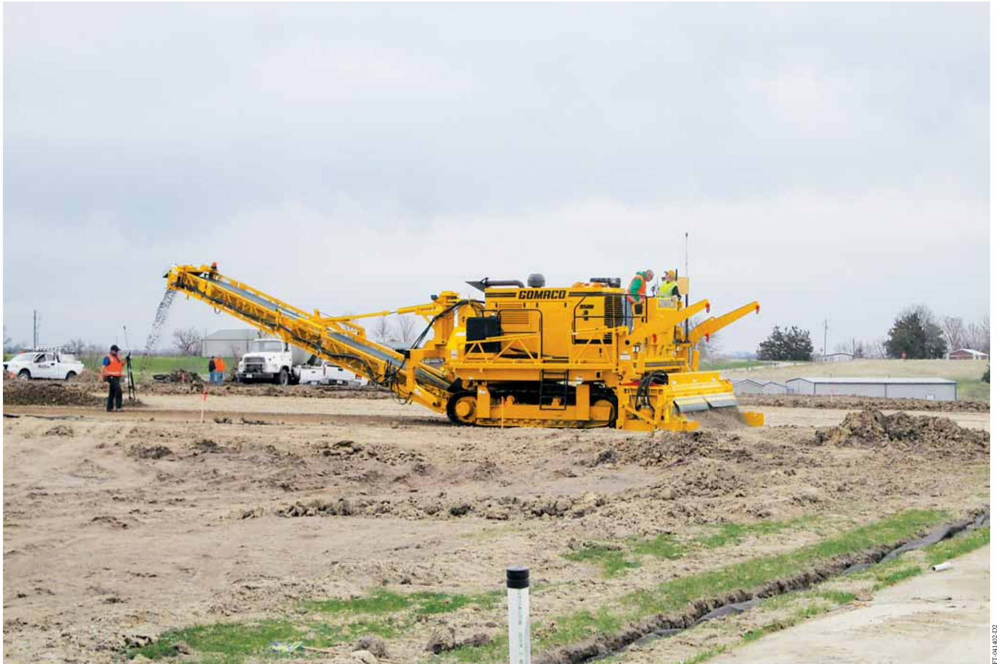
A GOMACO 9500 trimmer is equipped with a 14 foot (4.27 m) trimmerhead, G+ controls, and Leica Geosystems 3D machine guidance. The 9500 prepares the grade for 1000 feet (304.8 m) of airport runway and taxiway extensions.
