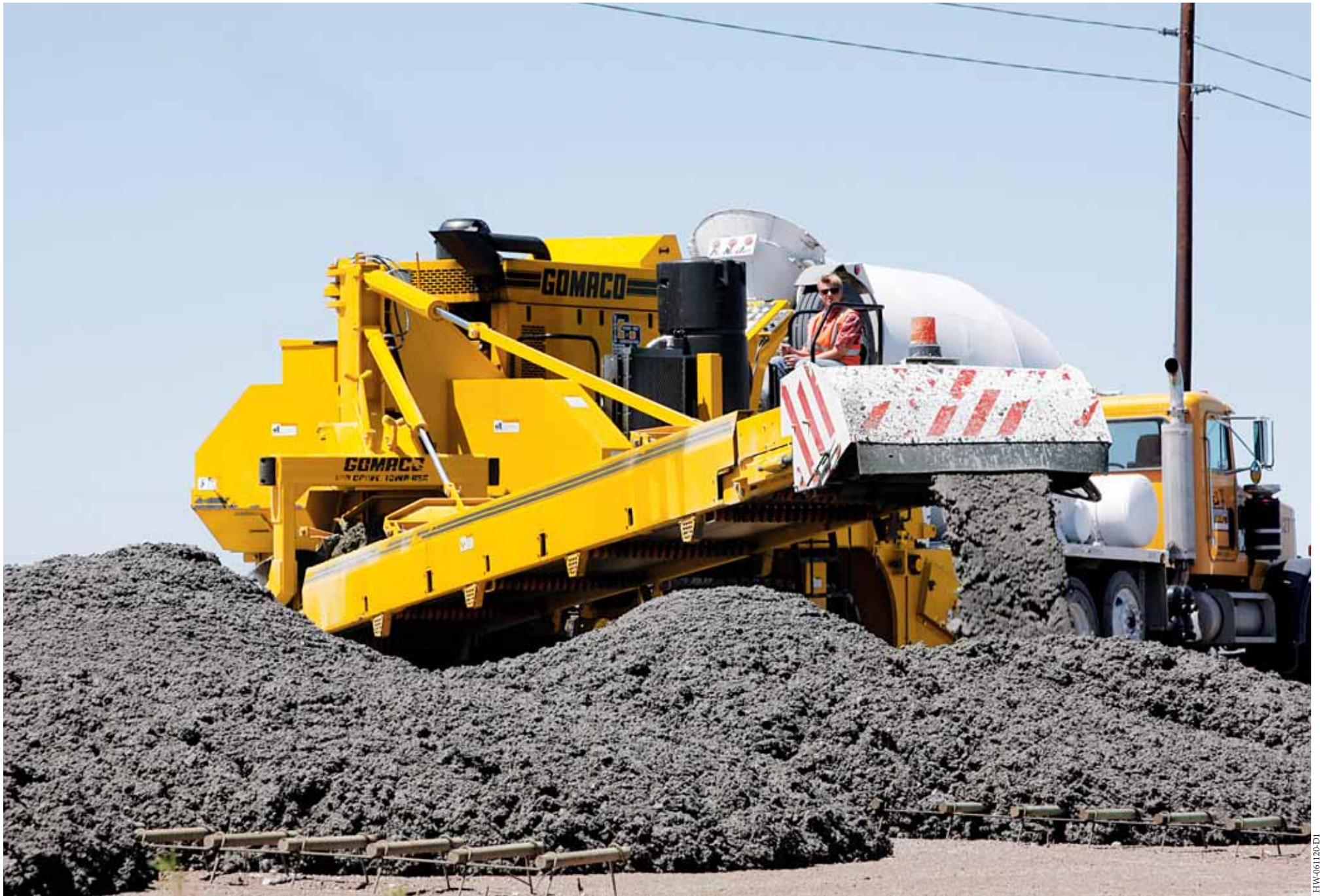
Placement of concrete with the 9500 is fast and accurate with the 35 foot (10.67 m) long conveyor.
