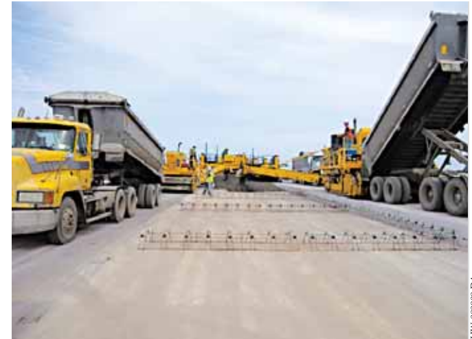
Two 9500 placers supply the concrete for the GOMACO paver on an airport runway.
