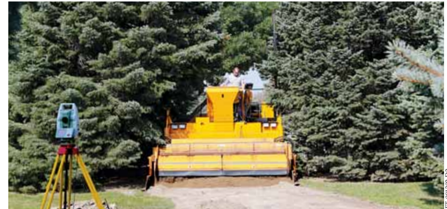
GOMACO's 9500 trimmer equipped with Leica Geosystems 3D guidance allows for the much needed minimal clearance while preparing the grade for a service road.
