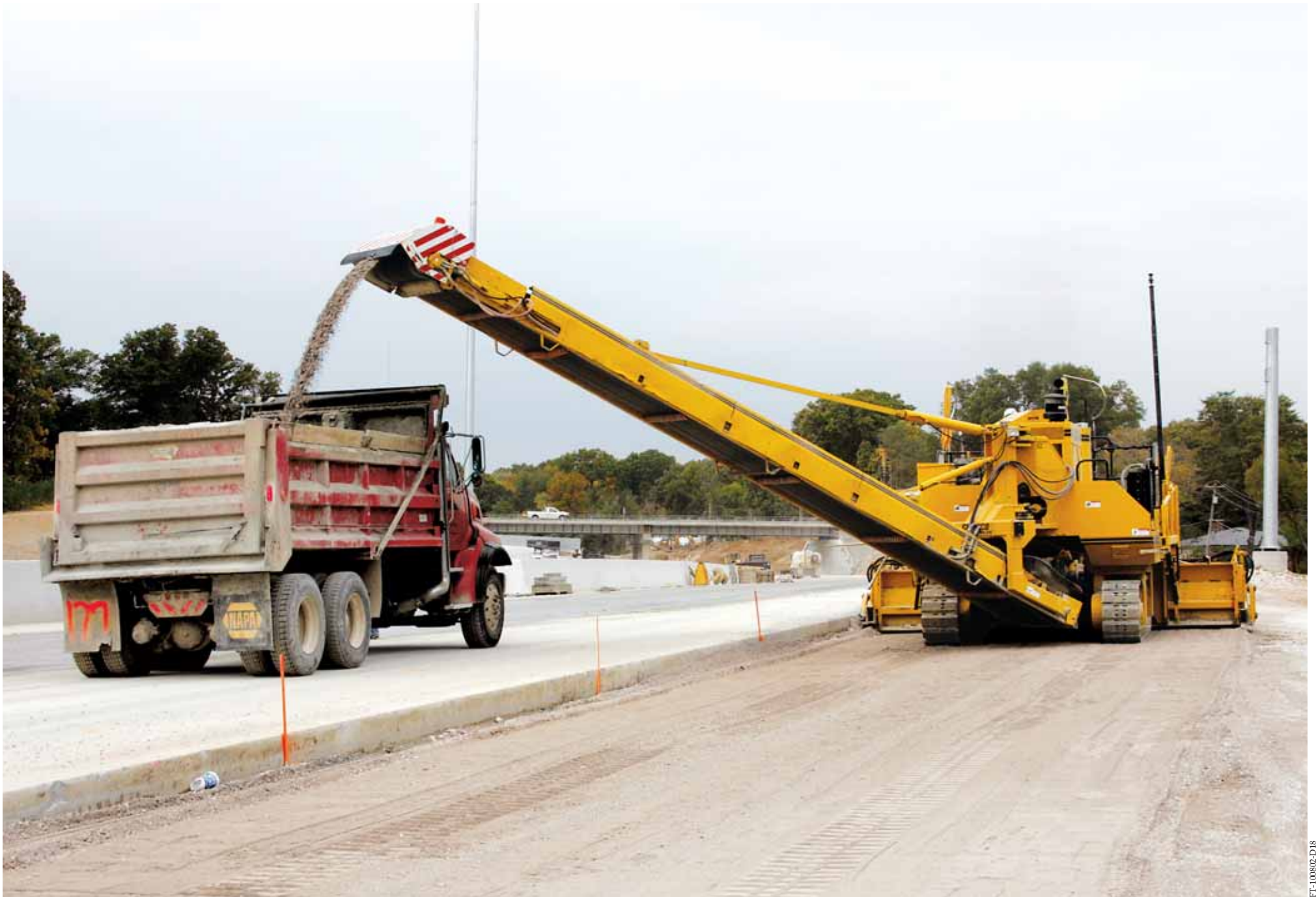
A GOMACO 9500 trims the grade and uses the conveyor to easily place the material into a haul unit for quick removal on an interstate project.
