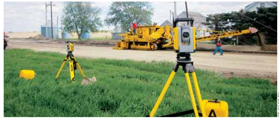
A 9500 trimmer equipped with Trimble 3D guidance creates a smooth grade in preparation for the concrete road.
