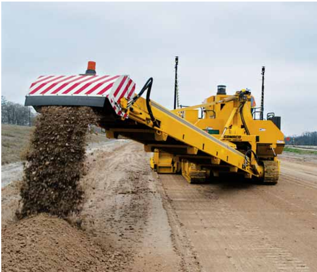
A 9500 trimmer is equipped with Topcon 3D guidance to trim the grade for a new highway system.
