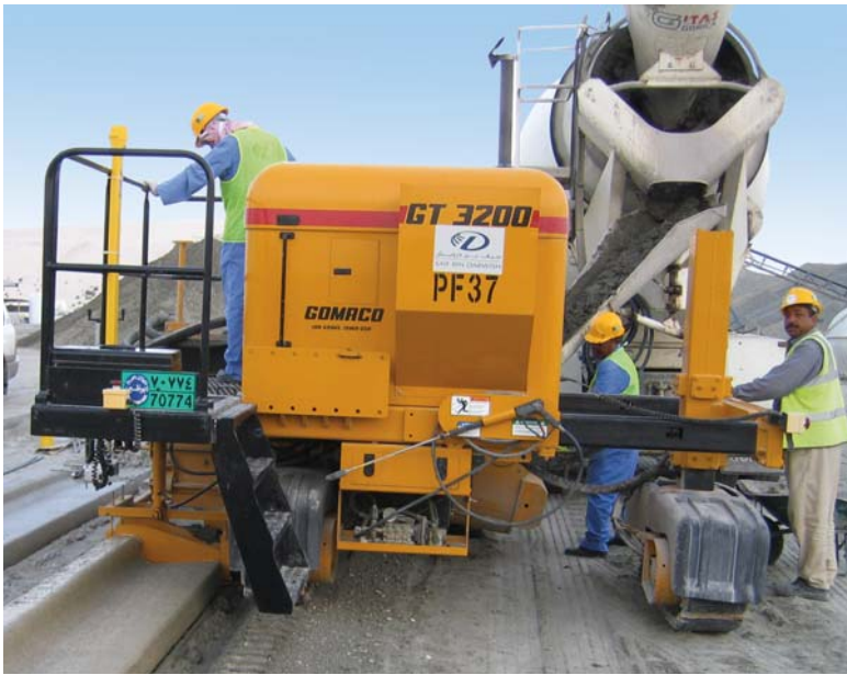
Saif Bin Darwish slipforms curb and gutter with their new GT-3200 in Abu Dhabi, United Arab Emirates.
