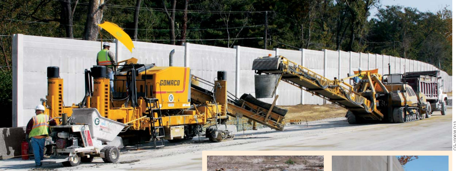
The Commander III slipforms barrier next to a section of already finished sound wall.
