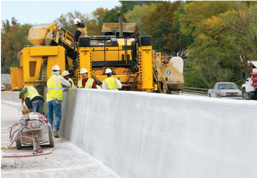
The Commander III is equipped with a variable-height mold for slipforming both the variable and non-variable center median barrier.
