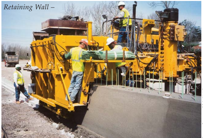
Two rebars at a time are hydraulically inserted into the top of this barrier. Another wall will be slipformed on top to form a retaining wall on the project.
