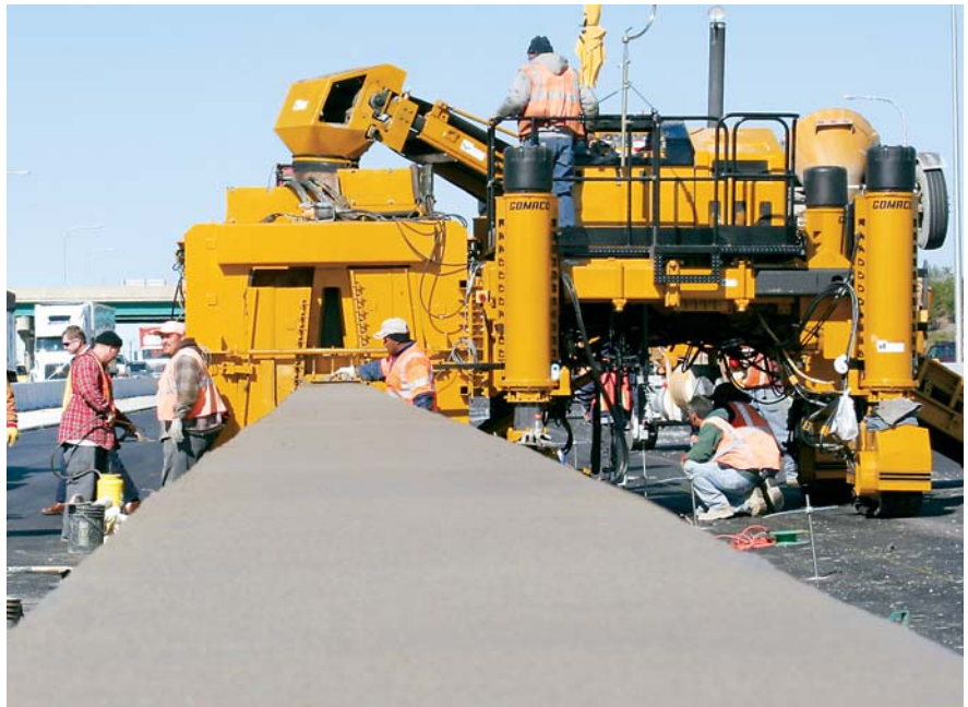
The wall has a 19 inch (483 mm) wide top, is 39.25 inches (997 mm) wide at the base and its sidewalls vary in height from 3.5 to 6.5 feet (1.1 to 2 m).
