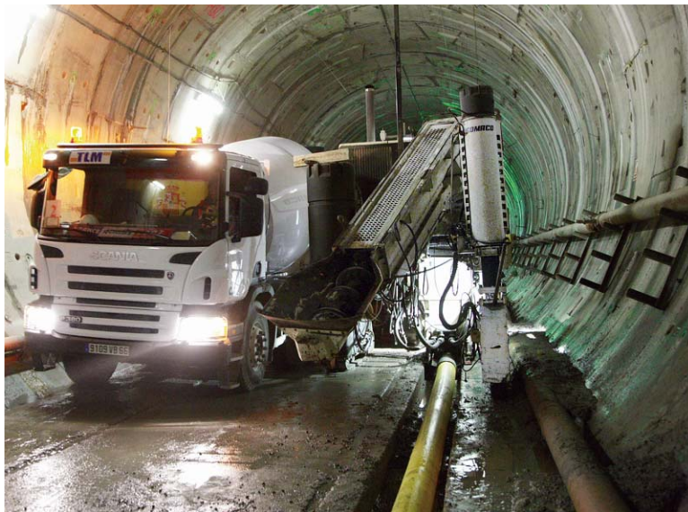
A high-drive track worked in the narrow spaces between the tubes and piping to be slipformed into the various profiles.
