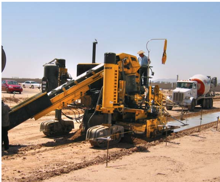
A total of 160,000 lineal feet (48,768 m) of curb and gutter and monolithic sidewalk and curb and gutter was slipformed on the project. All of the concrete was done with Commander IIIs.
