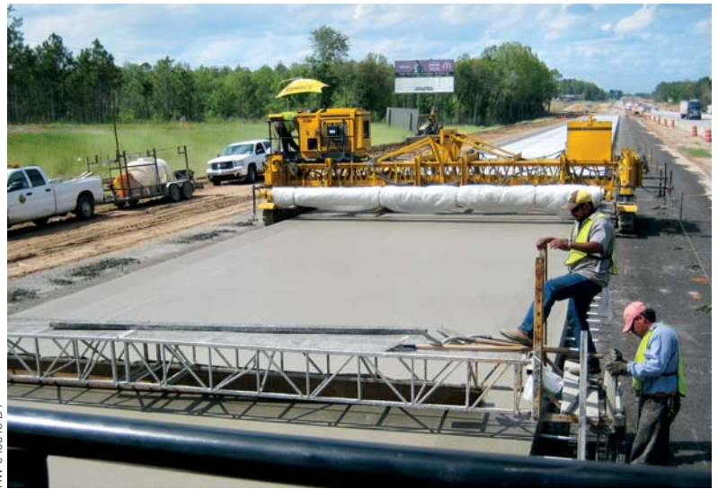
A T/C-600 texture/cure applied a tine finish and white spray cure.
