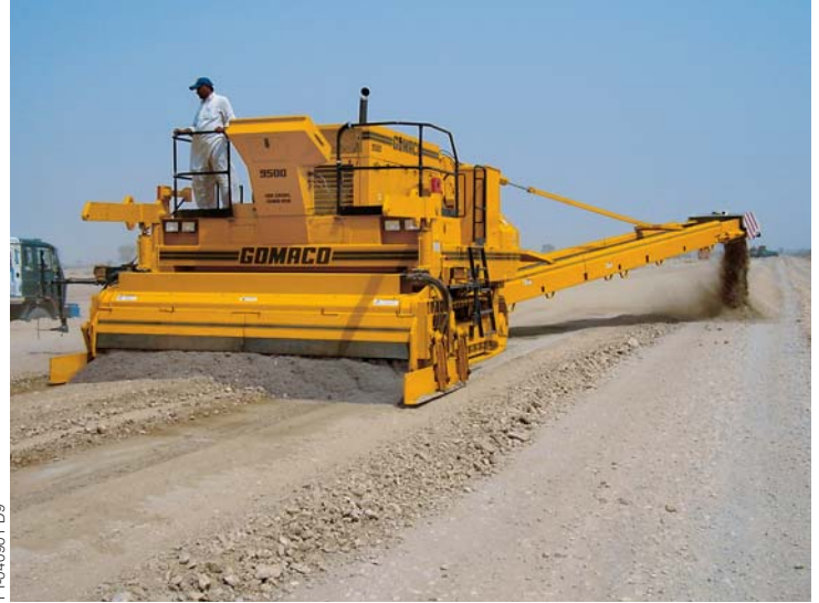
Giampietro Nasci trims grade with a GOMACO 9500 on a road project near Pezu, Pakistan.
