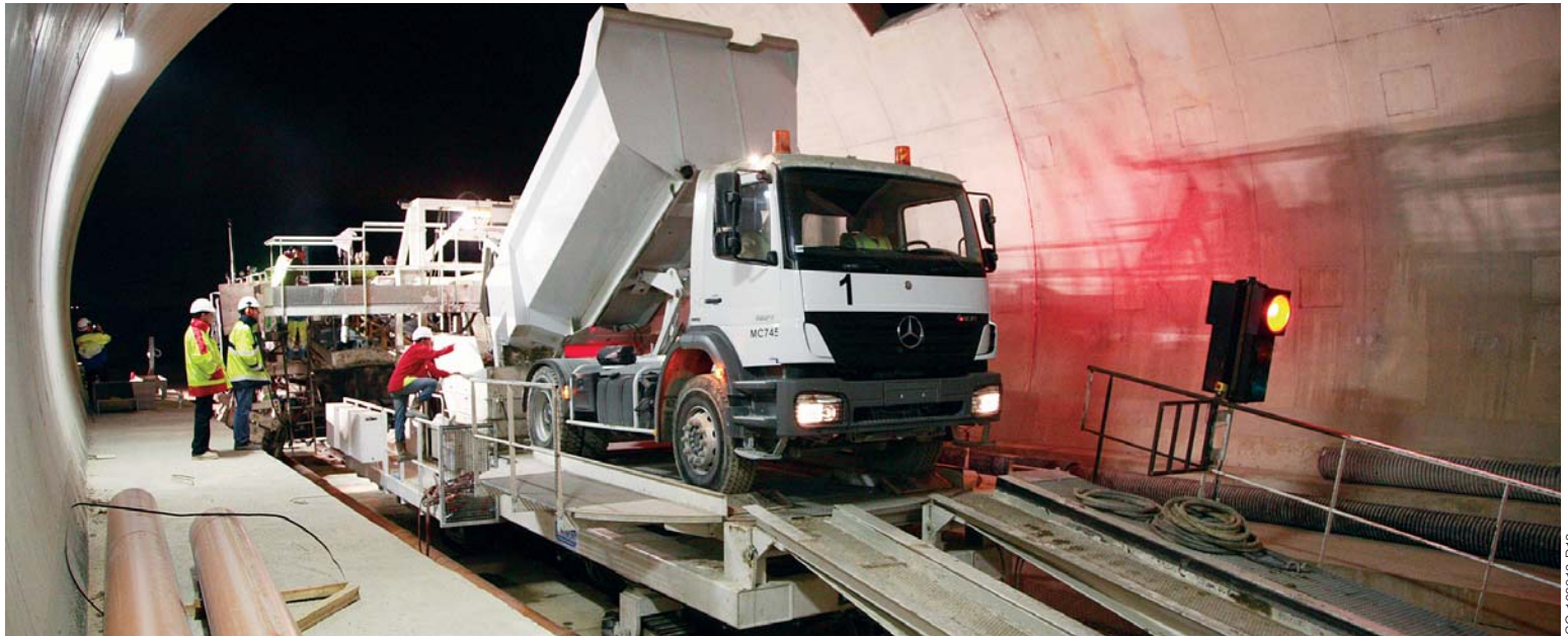
A turntable allowed trucks to rotate 180 degrees to dump their load of concrete into the hopper in front of the Commander III.
