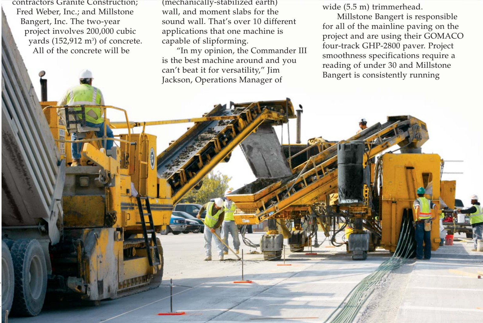
A GOMACO 9500 feeds concrete onto the belt of a four-track Commander III slipforming barrier wall on a project in St. Louis.
