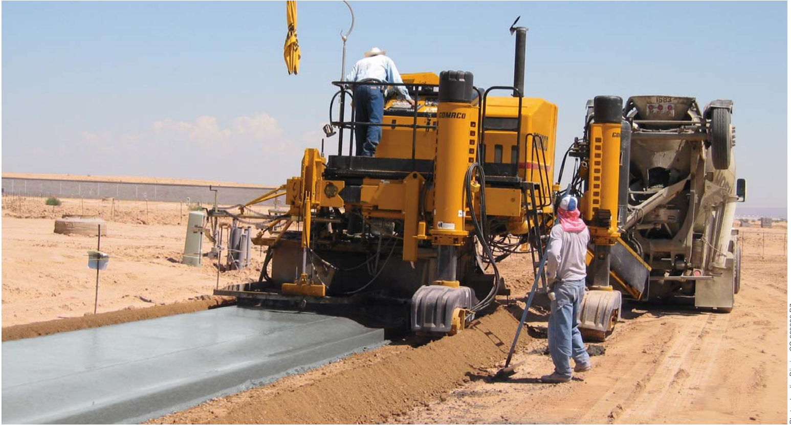
Petra Contracting slipformed two different profiles of monolithic sidewalk and curb and gutter at a business park in Arizona.
