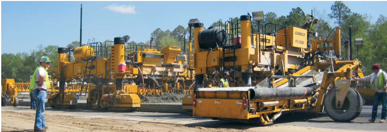
Scruggs PS-2600 placer/spreader and GHP-2800 paver are guided by the Leica stringless system. The GSI and T/C ran on stringline.
