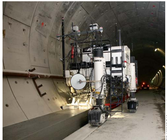
The Leica guidance system eliminated the hassle of stringline in the tunnel's tight paving conditions.
