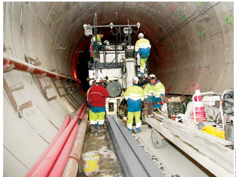
Slotted drain will remove any dangerous liquids that could potentially spill from the trains.
