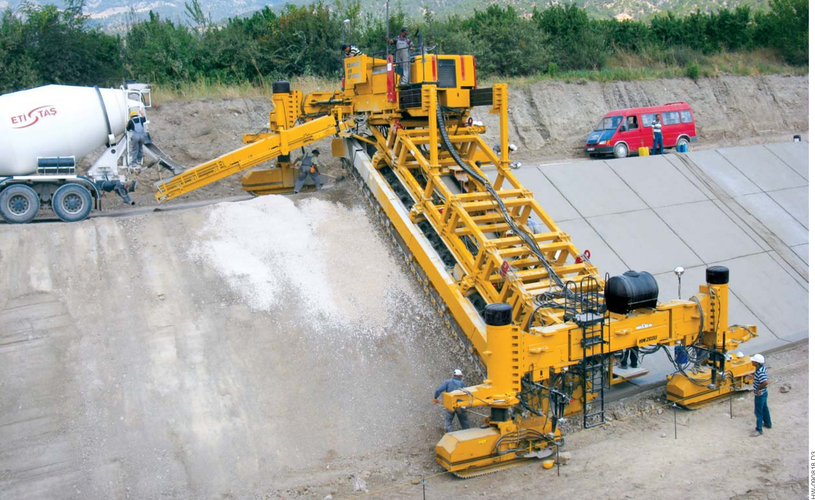
Concrete was discharged into the concrete feeding system with an auger and baffles that fed it down the slope of the canal.
