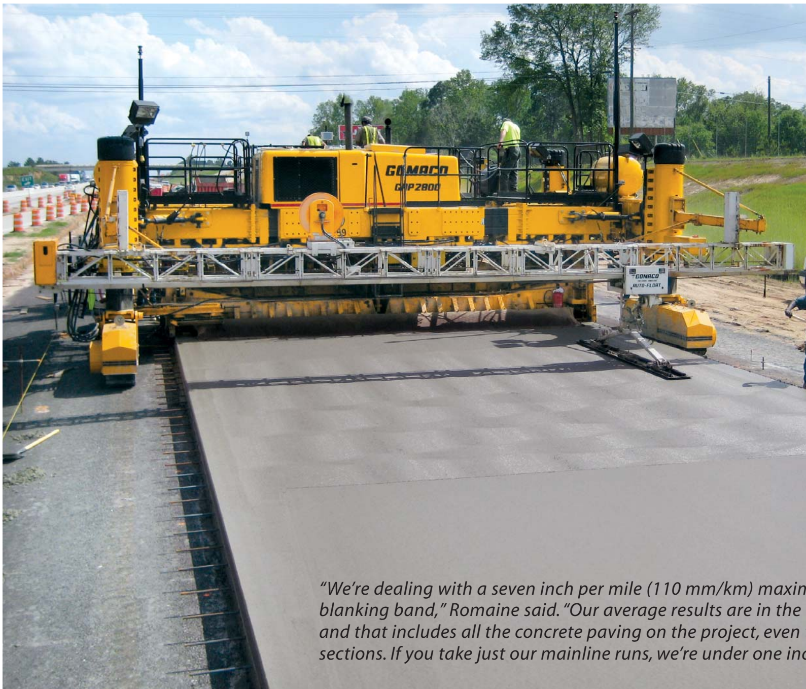
Rideability specifications were easily met with the four-track GHP-2800 paver. Scruggs has paved 99 lane miles (159 km) on the project with the GHP-2800 paver.
