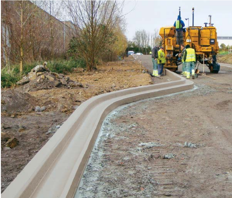
Tramo/TRBA slipforms curb and gutter with their GT-3600 and the TSD stringless system on a project near Peruwelz, Belgium.
