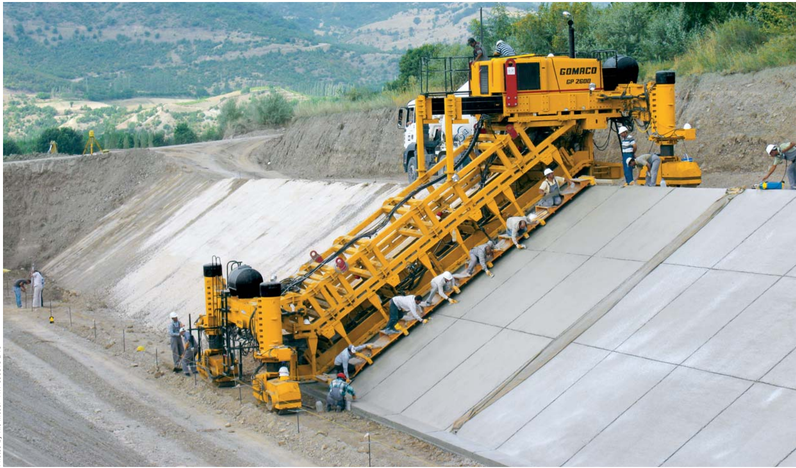
The GP-2600 with a front-mounted chain trimmer slipformed a new canal between Amasya and Tasova in northern Turkey.
