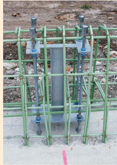
The first step to the sound wall is slipforming a moment slab. The slab features extra steel reinforcing slipformed into the concrete. The steel caging for the barrier wall is anchored to the steel in the slab. Extra supports for the sound wall are incorporated into the wall's steel cage. The posts that support and hold the sound wall panels are then bolted to the supports after the concrete wall has cured.
