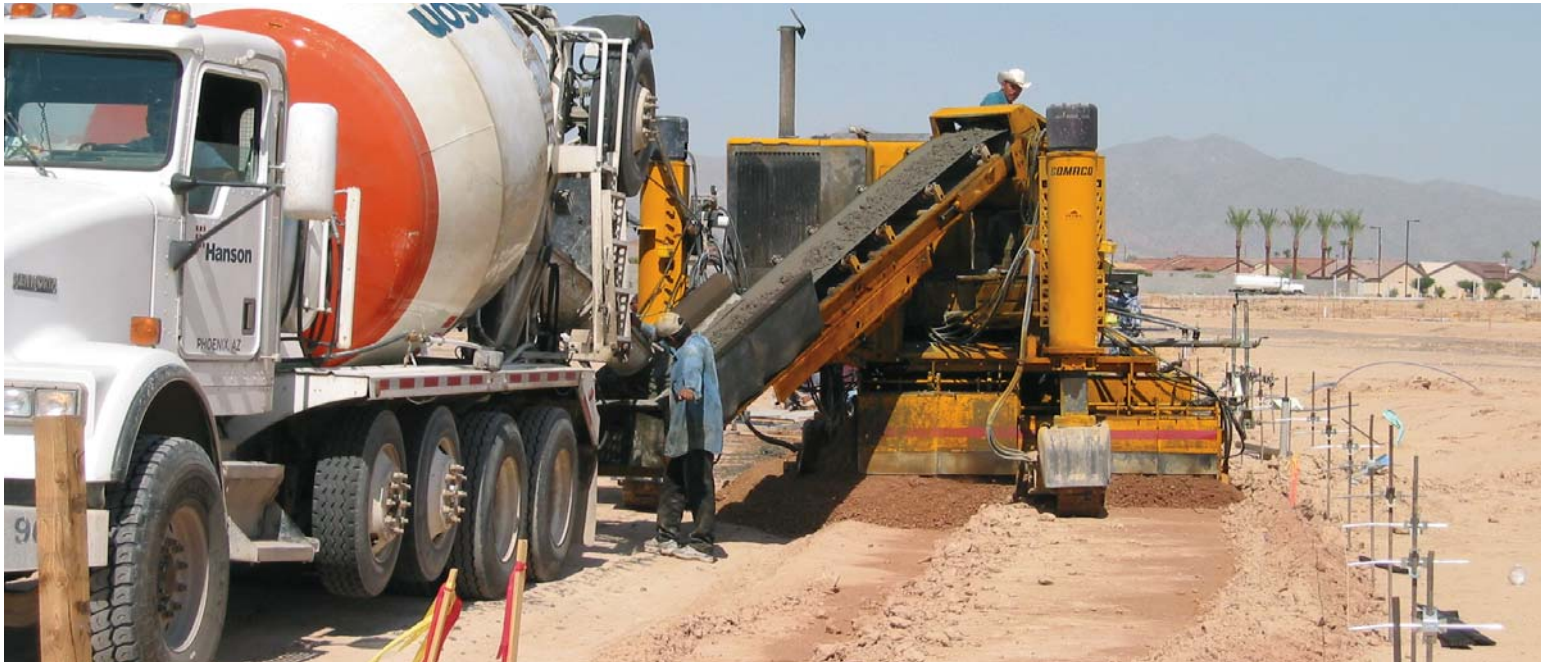
The Commander III's monolithic trimmerhead trims an extra six inches (152 mm) wider than the profile and moves the trimmed material out of the way with the side-discharge feature.
