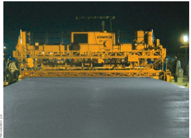
Orascom Construction Industries paves at night a new apron with their GP-2600 two-track paver at the Borg El Arab International Airport in Alexandria, Egypt.
