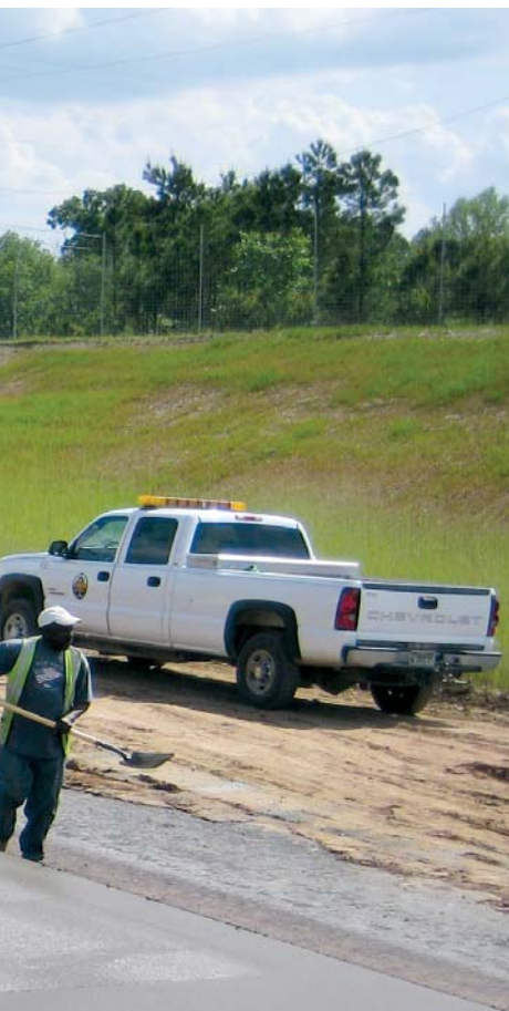
A GSI followed the paver providing instant rideability readings.
