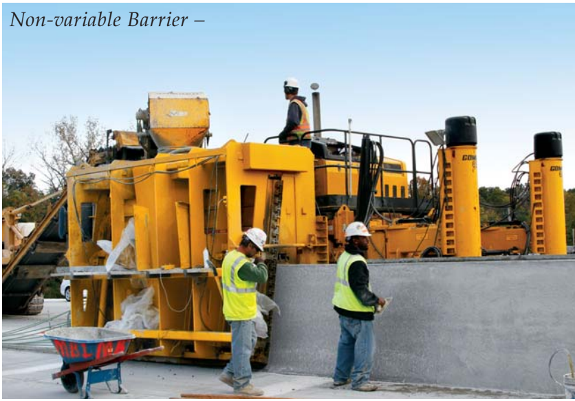
Ten longitudinal bars are fed into the front of the mold on the Commander III for the non-variable barrier wall.
