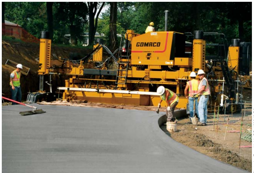
A roundabout on the project was slipformed 20 feet (6.1 m) wide with integral curb around a 45 foot (13.7 m) radius.
