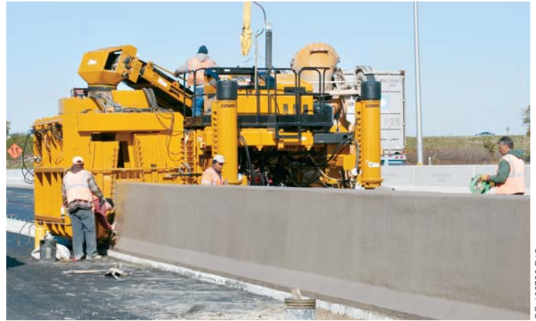
Slipforming successful wall, according to P.T. Ferro, is having the right concrete mix design delivered at the correct slump.
