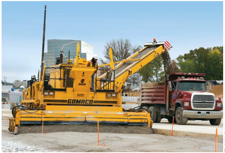
A 9500 trims grade for the mainline portion of the paving project. The trimmer is equipped with an 18 foot (5.5 m) wide trimmerhead.
