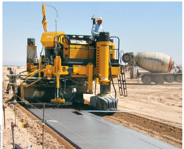
Production, on good days, would average around 6000 feet (1829 m) of monolithic in a 10 hour shift if the concrete supply was good and steady.
