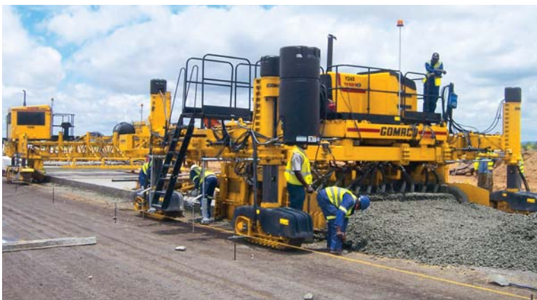
WBHO slipforms a new runway at the Sir Seretse Khama International Airport near Gaborone, Botswana. They are using a new Commander III four-track paver and a T/C-600 texture/cure machine to pave the five meter (16.4 ft) wide passes.
