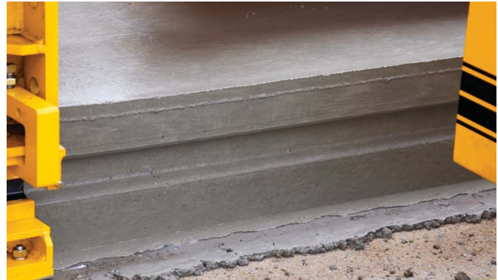
The new GP3 with 5400 series mold produces a smooth, clean and sharp edge and keyway on this new roadway project for a commercial development in Sarpy County, Nebraska.
