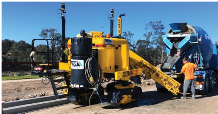
A GT-3200 with Topcon 3D guidance slipforms curb and gutter on a project in Glenfield, New South Wales, Australia.
