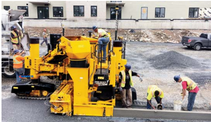
Twelve inch (305 mm) stand-up curb for a new apartment complex is slipformed with a GT-3600 and Topcon 3D guidance in Halifax, Nova Scotia, Canada.
