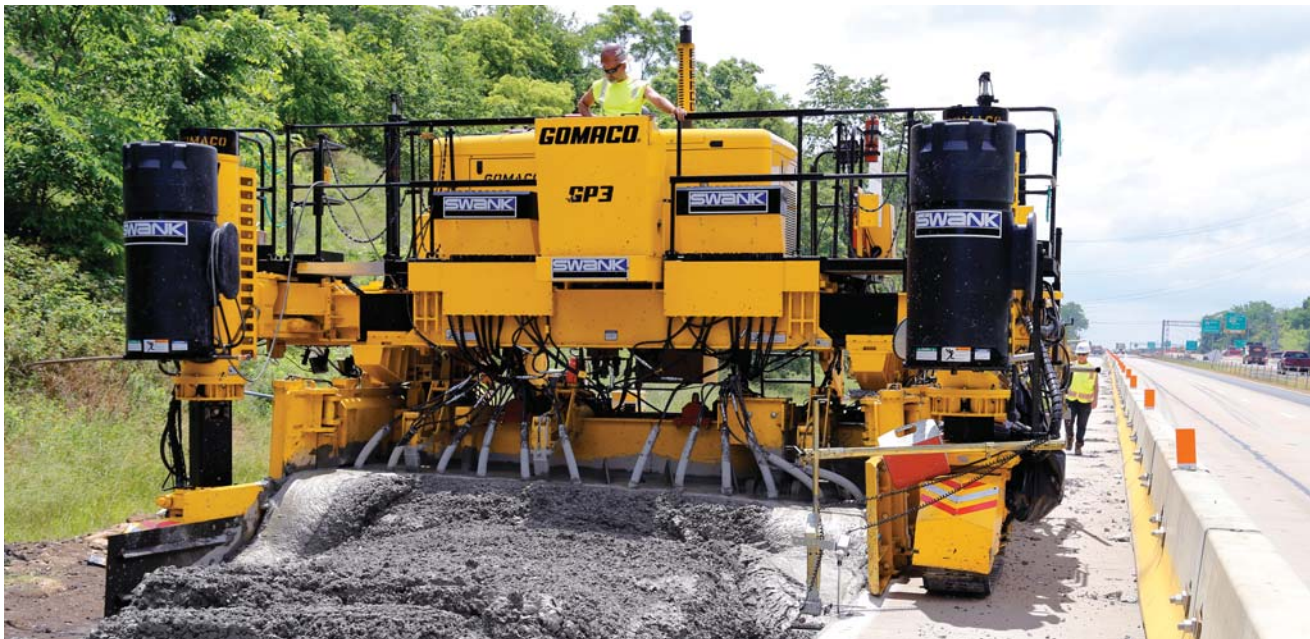
Swank's GP3 paver is equipped with a GOMACO 5400 series mold with a self-supported transition adjuster (TA). The 5400 series mold is also equipped with hydraulic vertical hinged sideplates for track clearance on this project with tight-clearance paving conditions.
