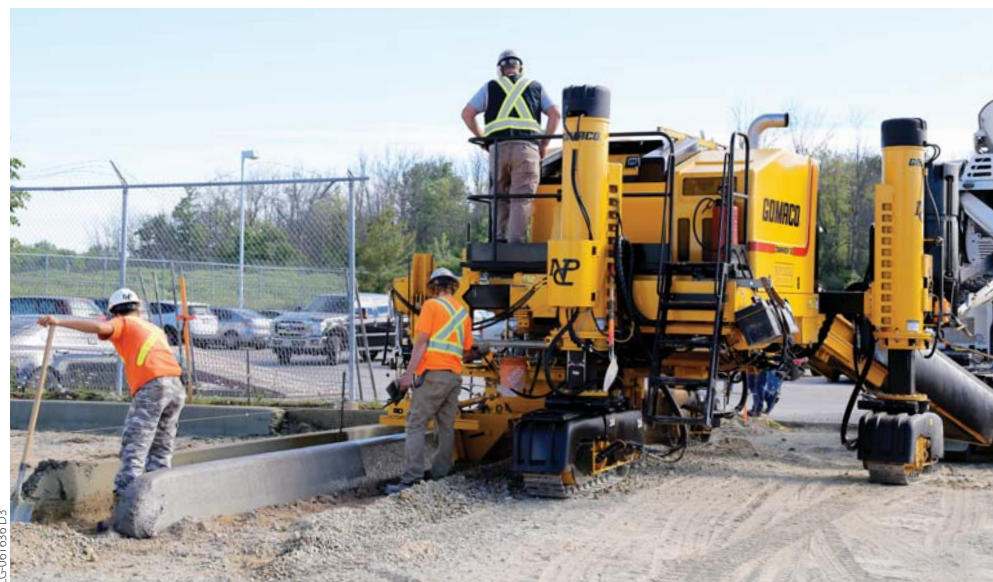
This parking lot project in London, Ontario, was a great test for the new Commander III and its tight turning abilities as it was maneuvered into and out of short curb runs in tight-clearance conditions.
