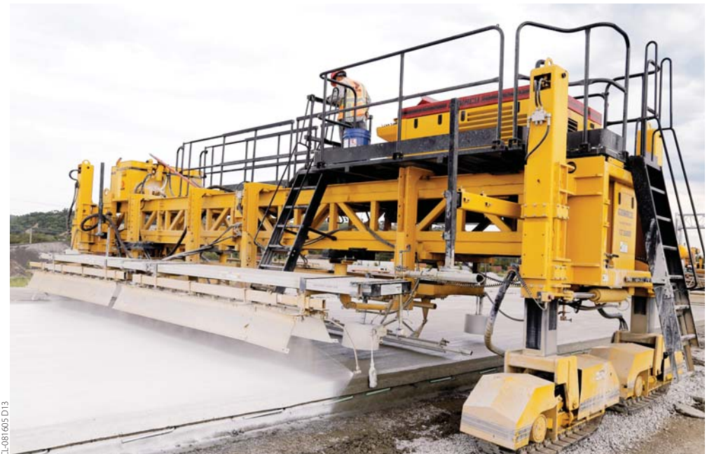
One pass texturing and curing is possible with the four-track T/C-5600. Covered sensors on the texture/cure machine follow the edge of the slab to steer it down the length of new interstate.
