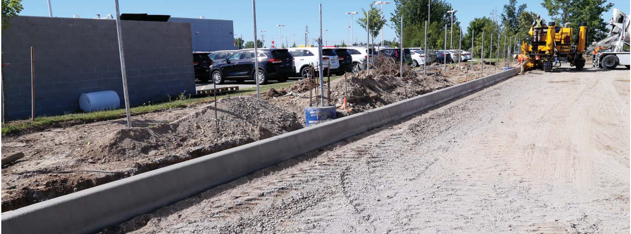
Straight curb is always the goal of Piccoli Construction, and the new Commander III has produced some of the straightest curb the company has ever slipformed.
