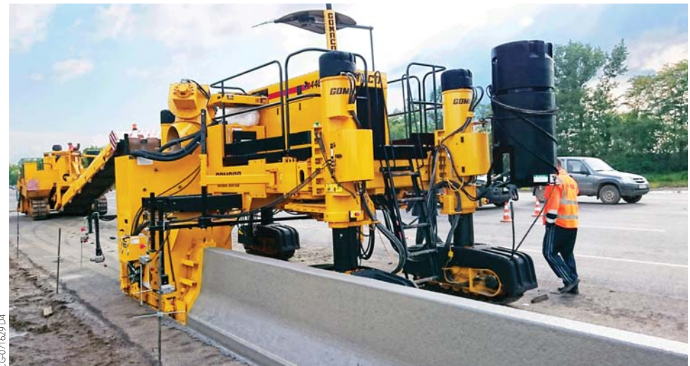
A 9500 placer works in front of a 4400 barrier paver on a project in southern Russia. The project is the M4 Don Federal Highway between the cities of Rostov-on-Don and Karasnodar in southern Russia.
