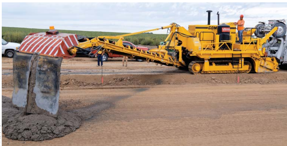
The operator of the 9500 uses the placer's remote control to move the placing belt as it puts concrete on the grade in front of the GP3 paver.
