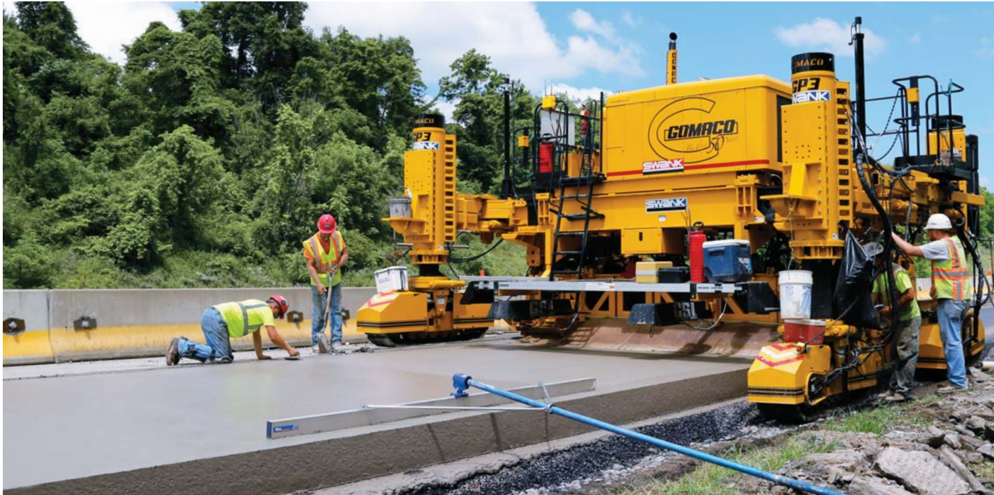
No stringline is necessary on Swank’s project. The paver is sensing off the existing slab for elevation control on this add-on lane and the G+ controller maintains the four percent cross slope.
