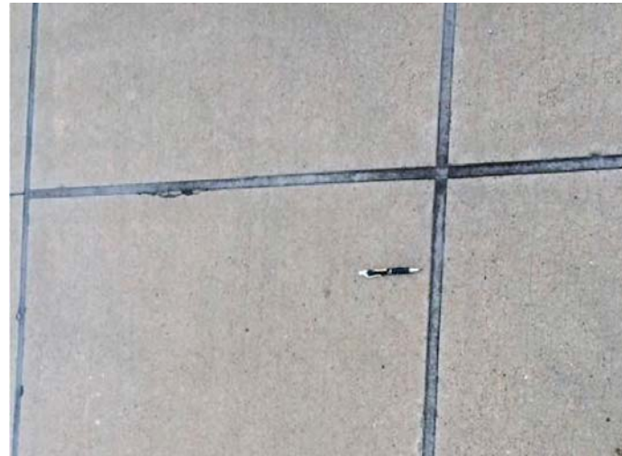
Figure 4. Current pavement condition (June 2015).
