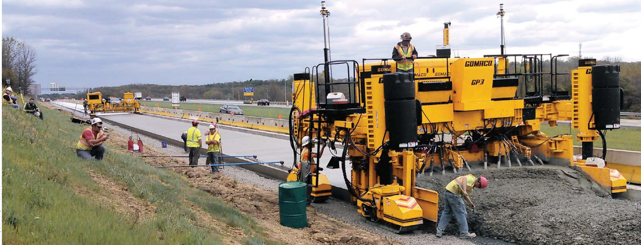
Swank Construction Company has a long-time roadbuilding history, and they chose the GOMACO GP3 with Trimble 3D guidance for their mainline paving projects around the Pittsburgh area of Pennsylvania.
