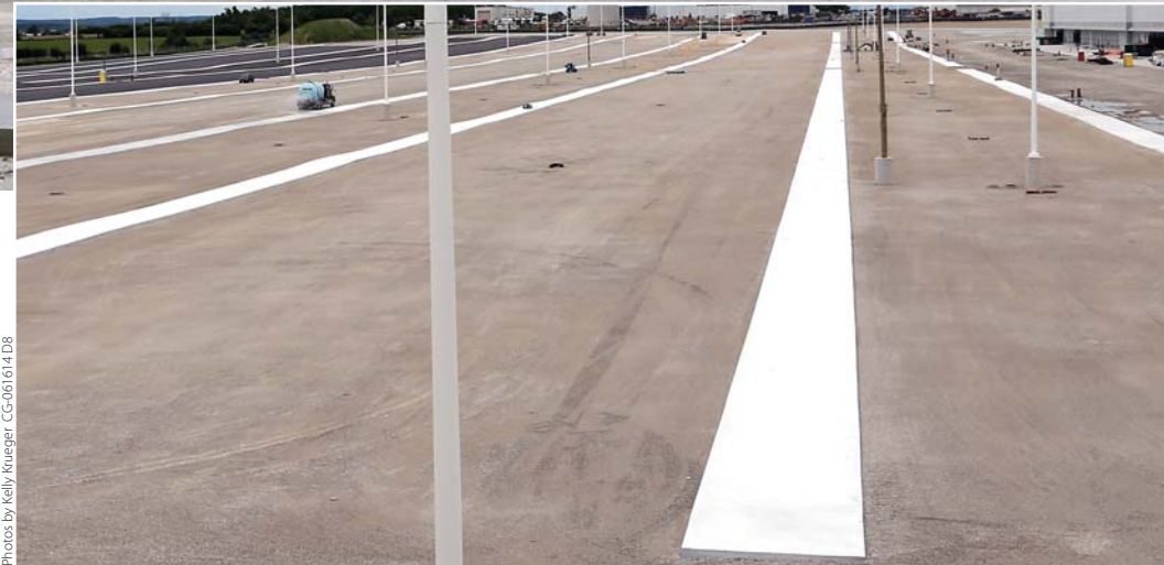
Curbside Construction is using their GOMACO GT-6300 with new 3100 series mold to slipform over 10 kilometers (6.2 mi) of three meter (9.8 ft) wide white dolly pads at a newly constructed distribution center in Toronto, Ontario, Canada.
