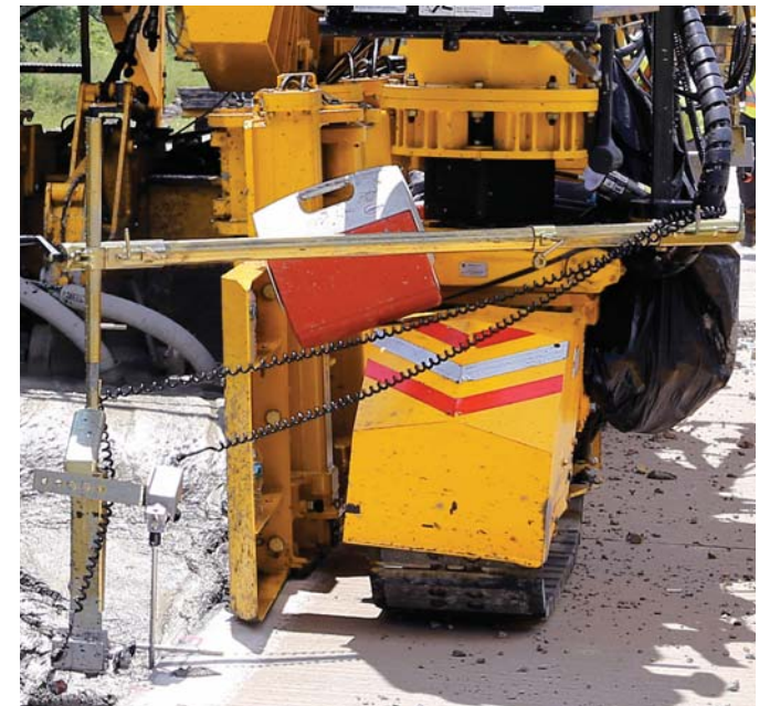
When scab-on paving, the GP3's steering wand on the front of the paver is sensing off the existing slab for grade and steering.
