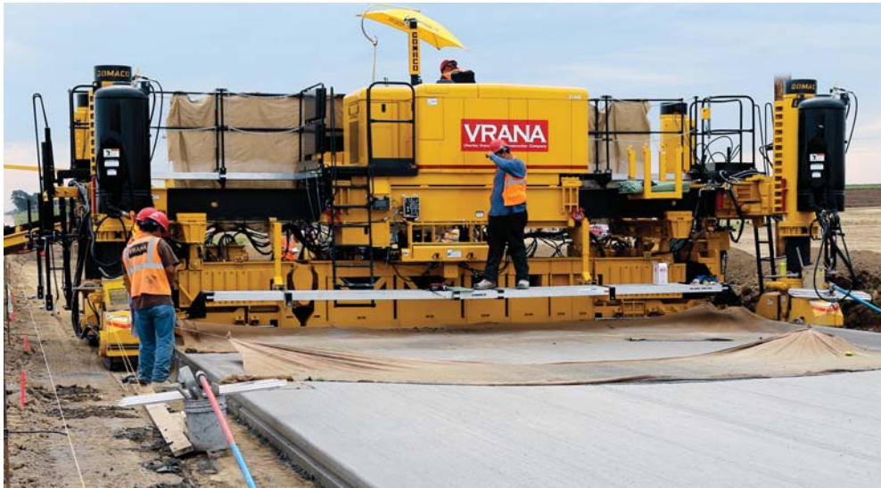
Vrana has equipped their GP3 with a 5400 series mold and bar inserter. The rear-loading, front inserting bar inserter is placing a 30 inch (762 mm) #5 bar every 33 inches (838 mm) into the new roadway.
