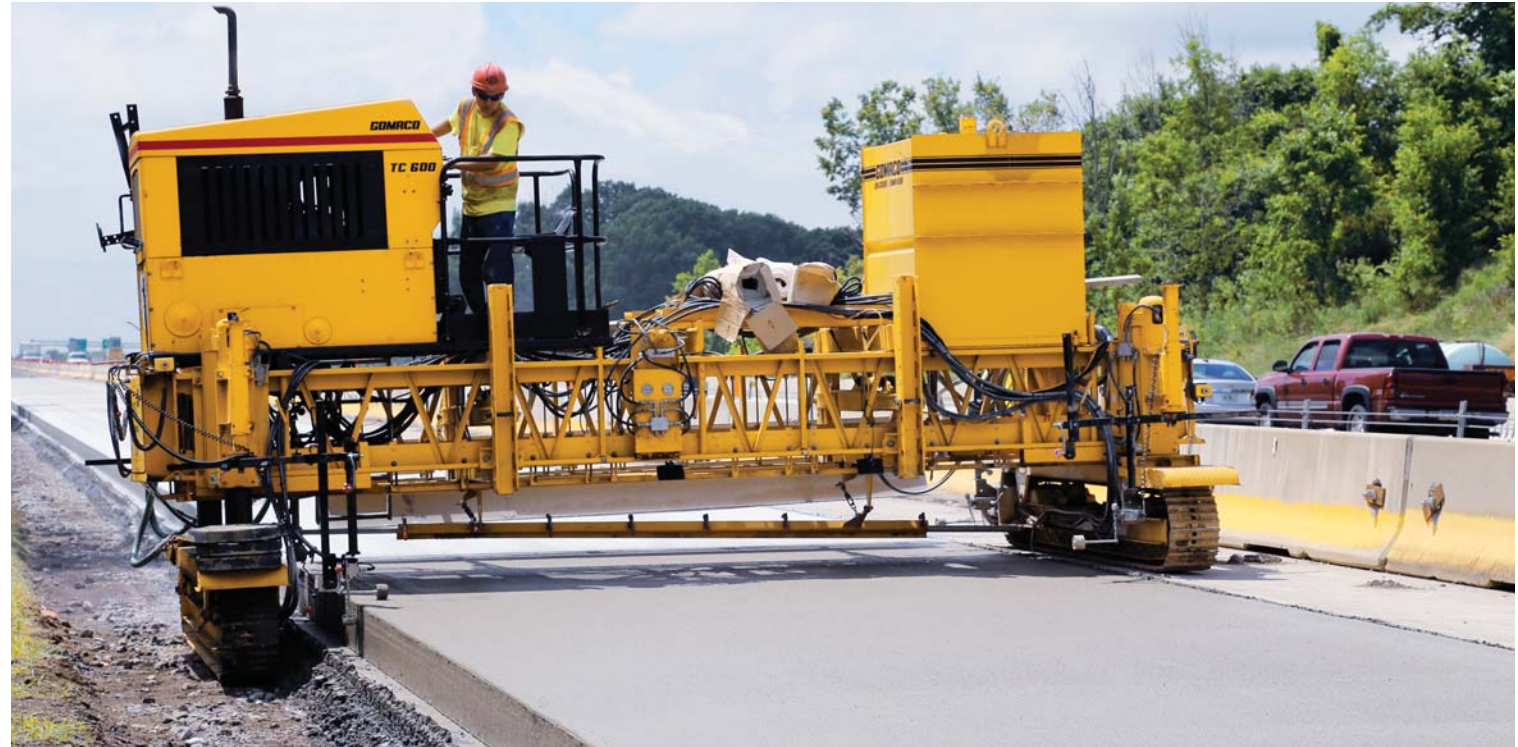
The T/C-600 machine applies a white spray cure and longitudinal tine finish to the new Interstate 376.
