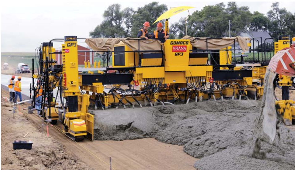
Vrana has to make one or two foot (0.3 to 0.6 m) width changes on many of their projects so they equipped their 5400 series mold with telescoping end sections to make the changes faster and easier.
