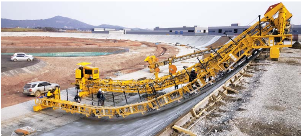
A new vehicle test track is under construction in Seosan, South Korea, using an RC Conveyor, SL-750 slope cylinder finisher, and 4000 series Spanit® work bridge. The undercarriage with finishing cylinder on the SL-750 is controlled with a Leica 3D guidance system. This is the second track they've finished with the equipment, with the first one built near Yantai, Shandong Province, China.
