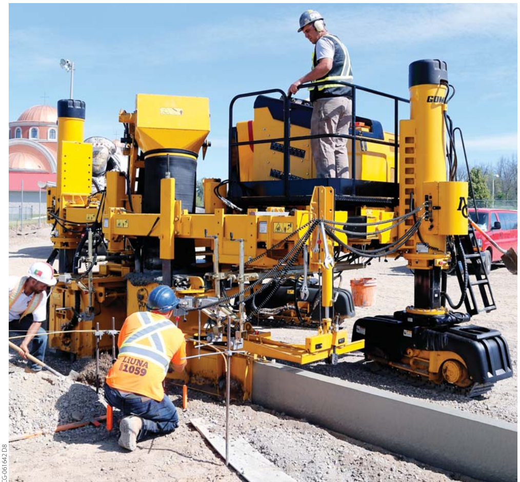
The operator and ground crew monitor the progress of the Commander III as it slipforms around a radius in the parking lot.
