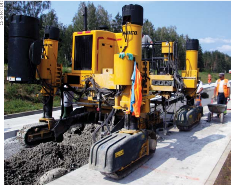
A GT-3600 with a center-mounted sidewalk mold is at work slipforming on a new project in Brest, Belarus, close to the border with the country of Poland.
