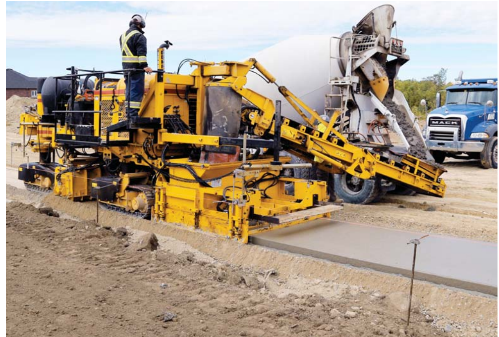
Curbside Construction says the GT-3200 sidewalk paver produces a high quality and precise sidewalk at a production rate far higher than what could be built by handforming.
