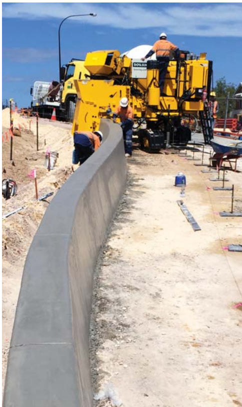
A GT-3600 slipforms variable barrier ranging in height between 885 to 1335 millimeter (34.8 to 52.6 in) on a project in Perth, Australia.
