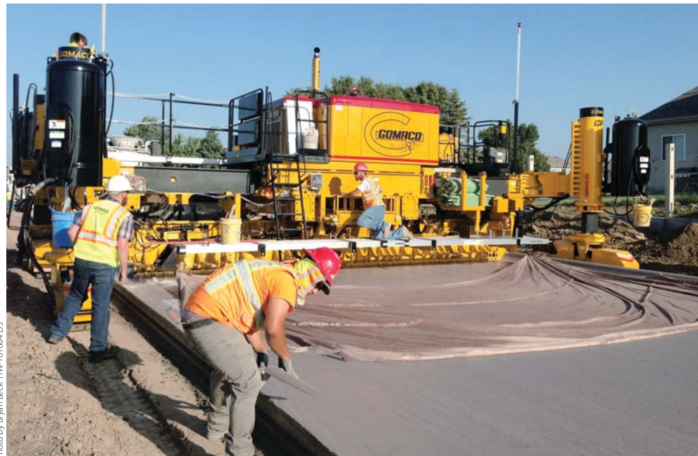
The first pour with the GP3 was slipformed 26 feet (7.9 m) wide with integral curb on both sides of the slab. The machine was delivered in the afternoon and early the very next morning was paving this project.
