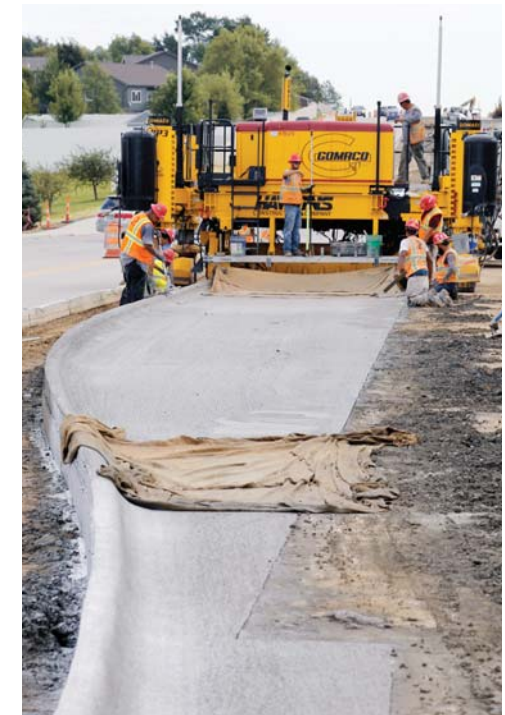
The GP3 slipforms a scab-on, tapered slab with integral curb in traffic in urban conditions.
