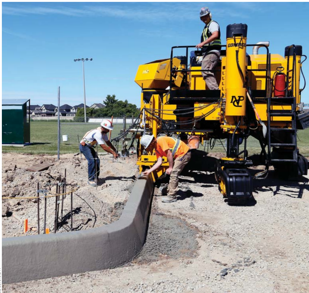
Piccoli's Commander III can slipform a 24 inch (610 mm) radius. The G+ controller, rotary-sensored slew drives, sensors on the sideshifting mold, and new radius software work together to easily slipform it.
