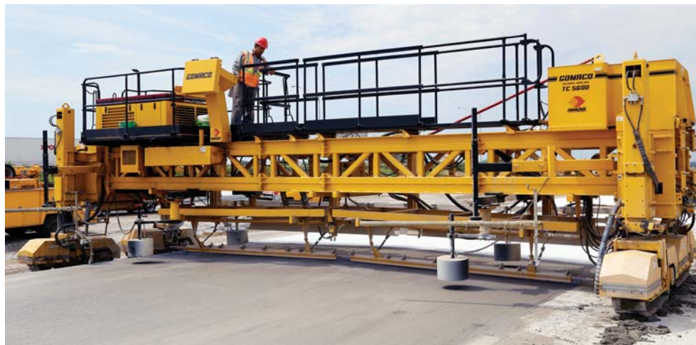
Sonic sensors on the T/C-5600, protected by black spray guards, control the machine’s elevation and crowning adjustments on this stringless paving project in Omaha, Nebraska.
