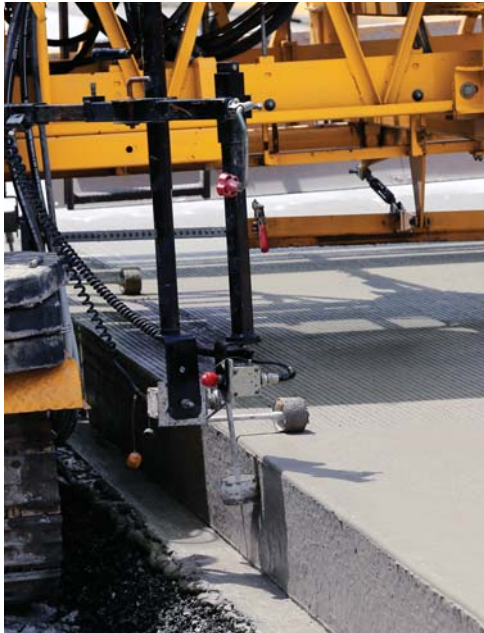
The GOMACO T/C-600 texture/cure machine has wheels attached to the sensors to steer it on the stringless project. Steering is referenced off the side and grade control is referenced off the top of the new concrete roadway.
