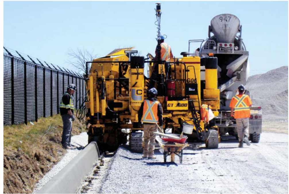
Curbside Construction is using their GT-3600 to slipform approximately eight kilometers (5 mi) of barrier curb around the perimeter of the distribution center.
