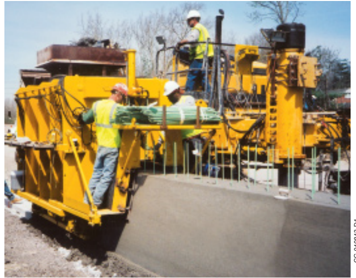
Rebars are hydraulically inserted into the 24 inch (610 mm) wide top of this barrier wall being slipformed by a four-track Commander III on a project in St. Louis, Missouri.
