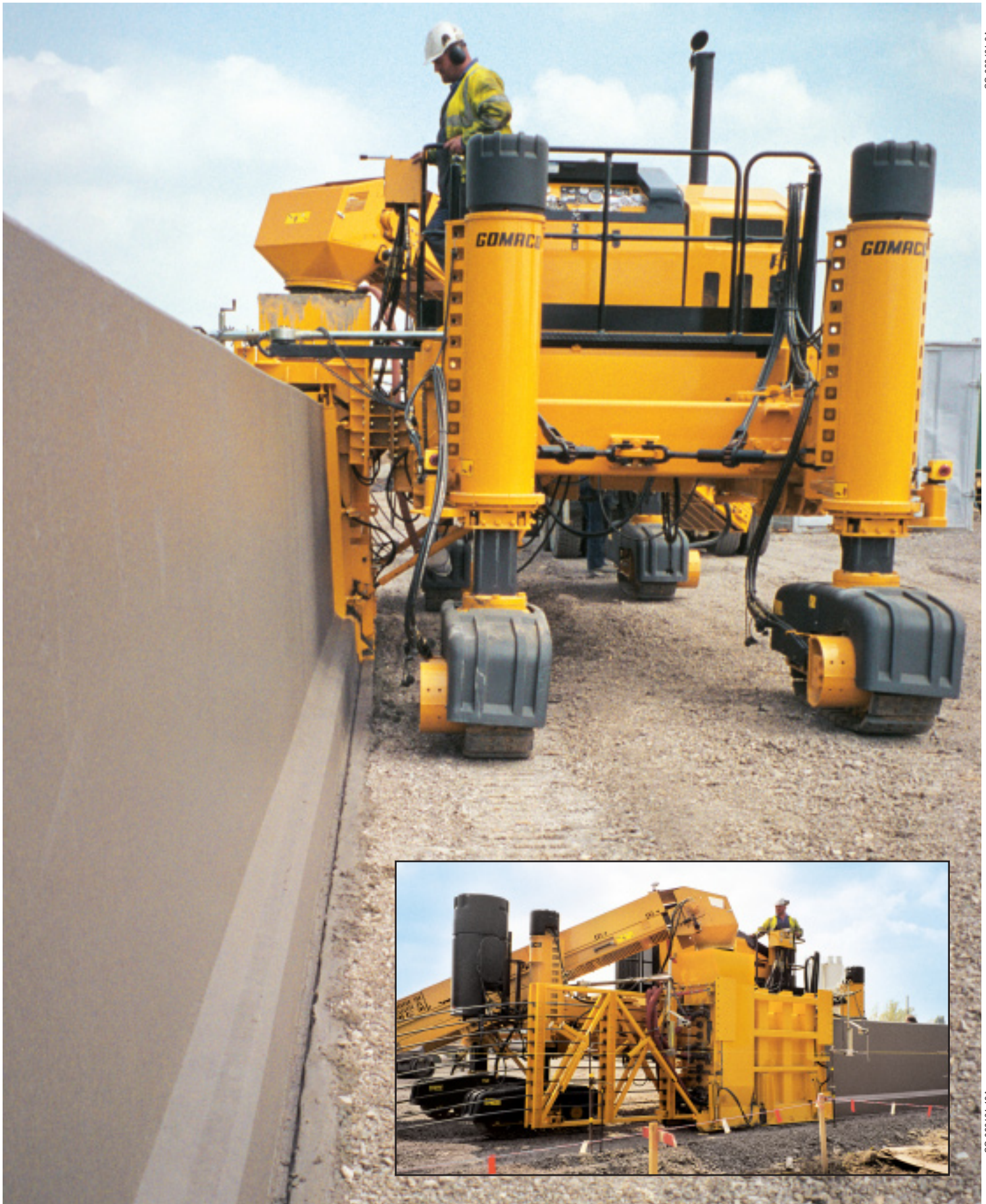
Steel reinforcing is fed into the front of the mold as this 5 ft. 7 in. (1.7 m) tall European-style step barrier is slipformed with a four-track Commander III on a project in London, England.
