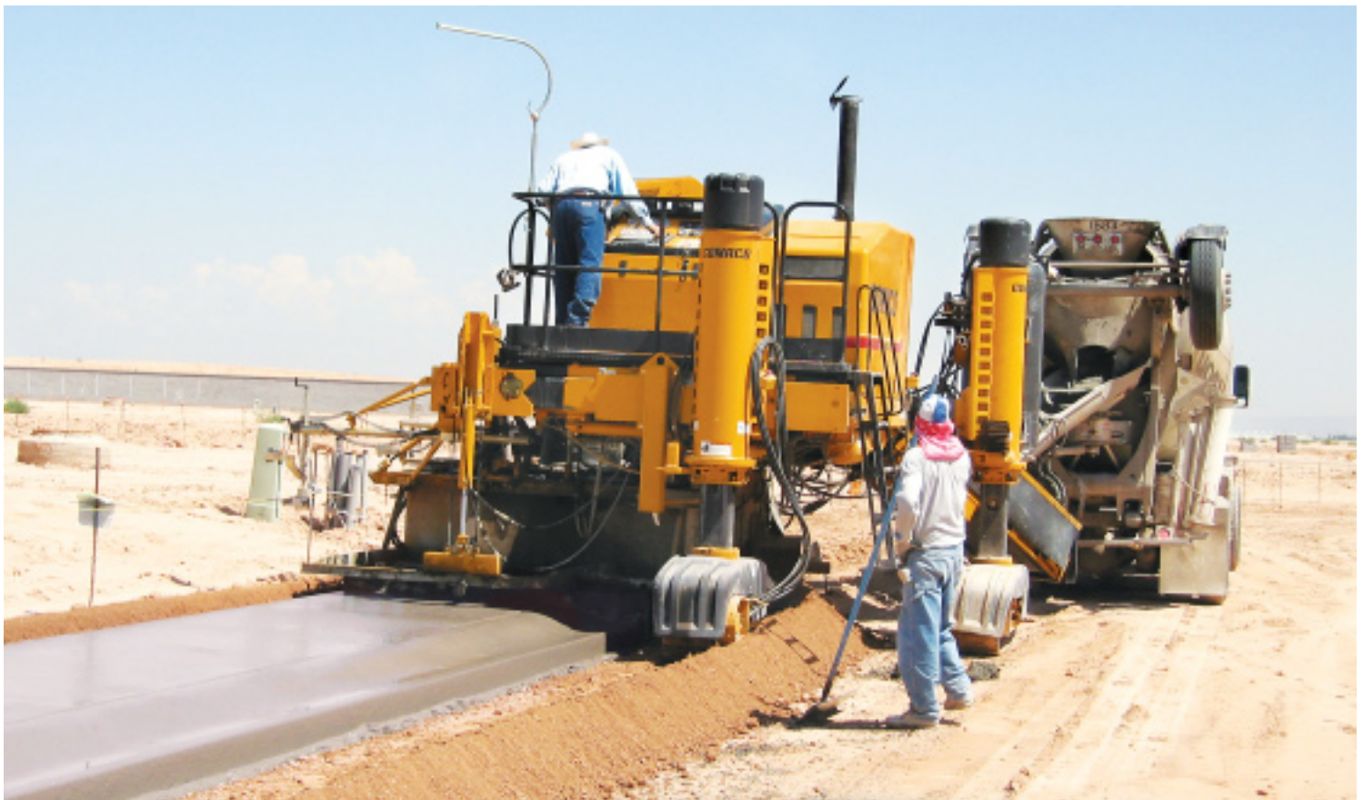
This Commander III is equipped with a monolithic trimmerhead and mold. It simultaneously trims the correct profile as the monolithic sidewalk and curb and gutter is slipformed. The monolithic profile is a 5 ft. (1.52 m) sidewalk with a 36 in. (914 mm) roll curb.
