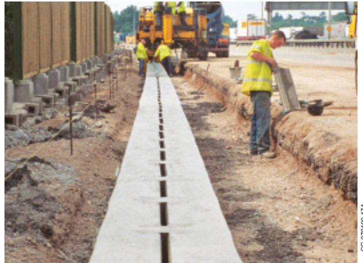
Slotted drain is slipformed by a three-track Commander III along the M25 Ring Road near London, England.
