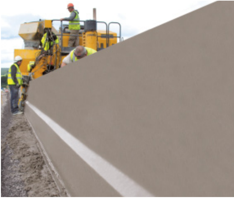
A GOMACO Commander III three-track slipforms 35 in. (900 mm) tall European step barrier on a project outside of Kilpedder, Ireland.
