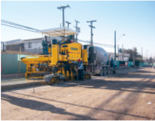
A contractor paves a single lane 11 ft. 6 in. (3.5 m) wide with a three-track Commander III equipped with a 12 ft. (3.66 m) paving package in Santiago, Chile.
