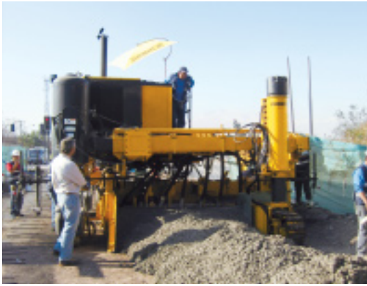
A contractor paves a single lane 11 ft. 6 in. (3.5 m) wide with a three-track Commander III equipped with a 12 ft. (3.66 m) paving package in Santiago, Chile.
