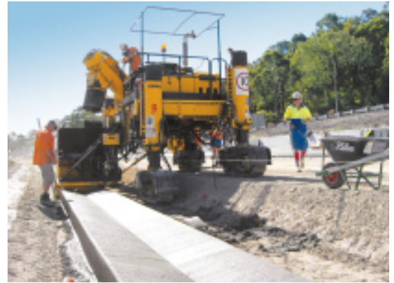
High-Production Slipforming
